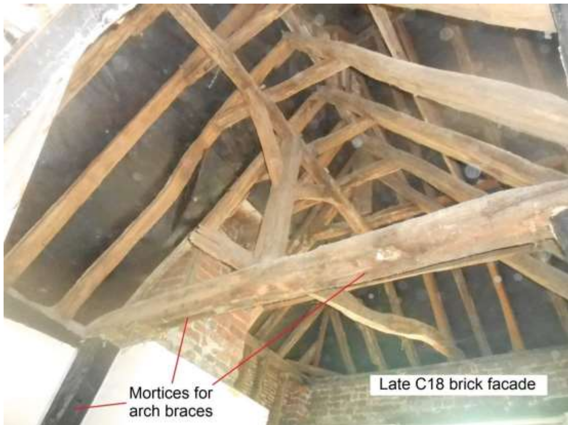
Crown-post roof in eastern crosswing
