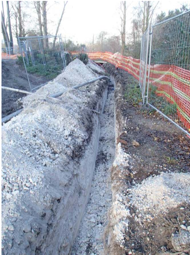
Cable trench looking north
