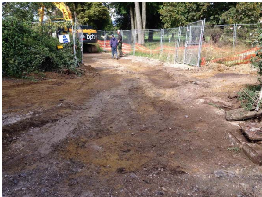
Removal of protective surface over Stane Street
