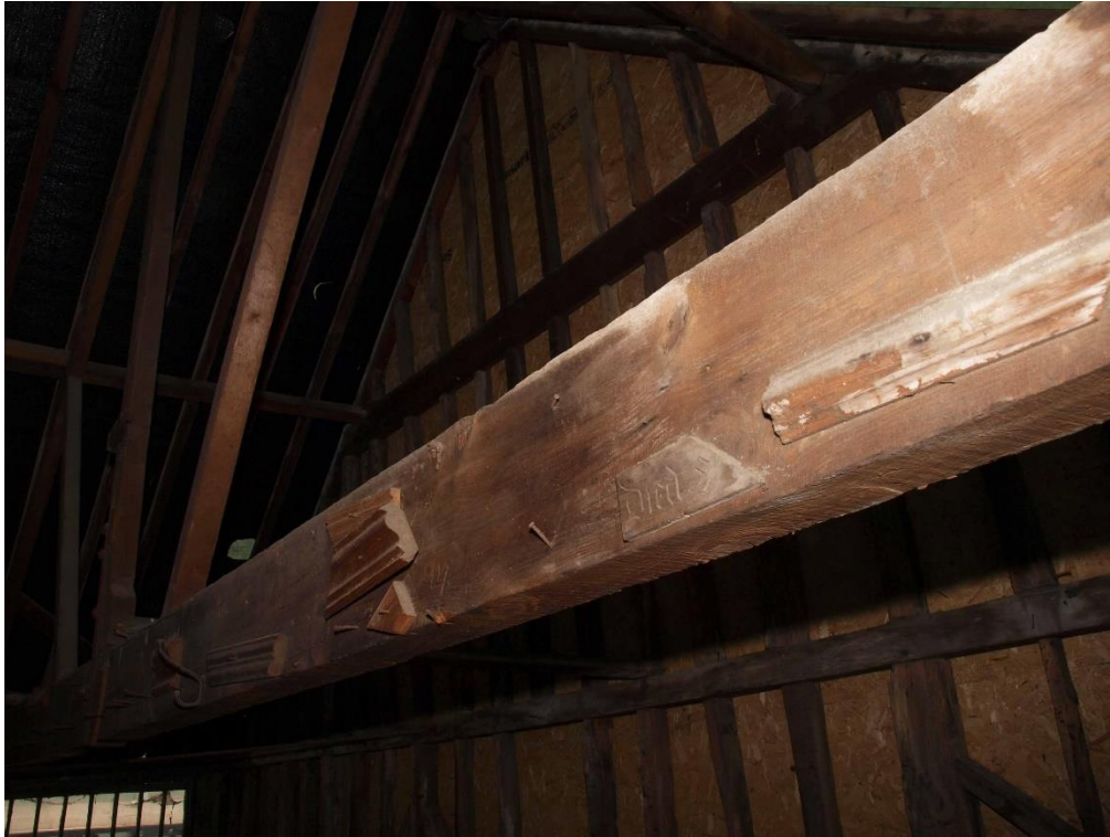
Plate 35: Detail of the retained coffin trimmings secured to the western roof truss, facing south-west (7790_028)
