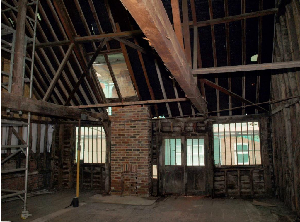
Plate 33: View of the south elevation at first floor level, facing south-east (7790_019)
