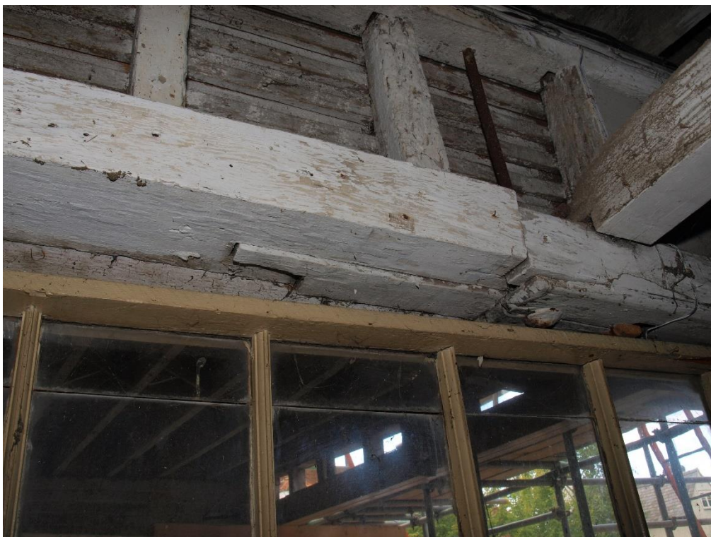
Plate 16: Detail of the face-halved scarf joint within the wall plate to the west of the eastern room, facing west (7790_050)
