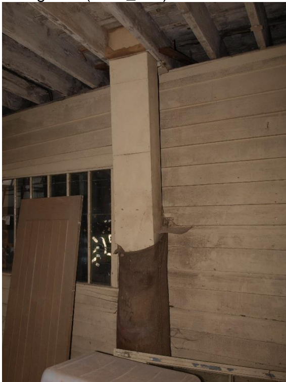
Plate 24: Detail of the chute within the former carriageway, facing north-east (7790_034)
