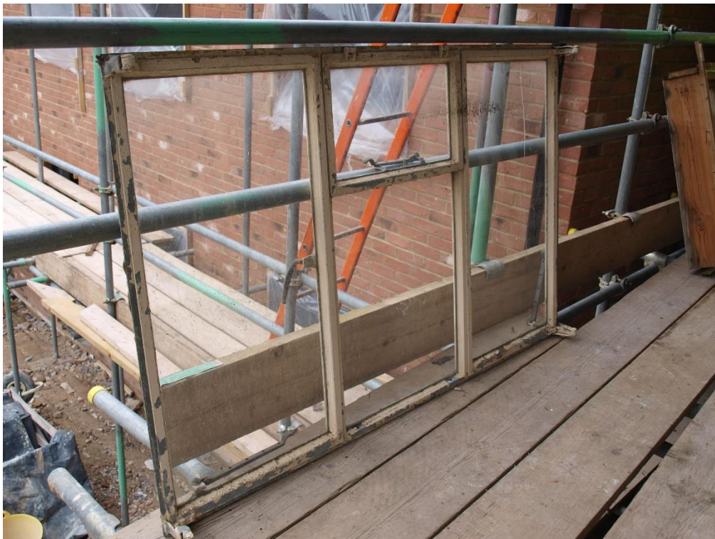
Plate 8: Detail of the Crittall style windows at first floor level within the north elevation, facing north (7790_012)
