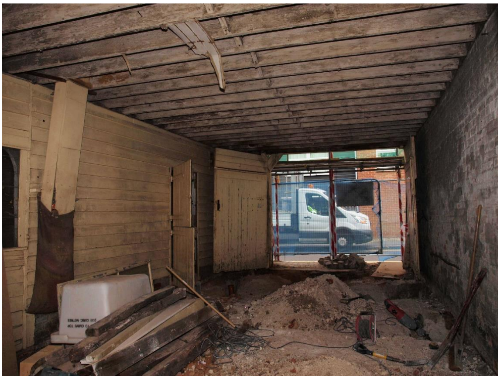
Plate 10: View of the former carriageway at ground floor level, facing south (7790_029)
