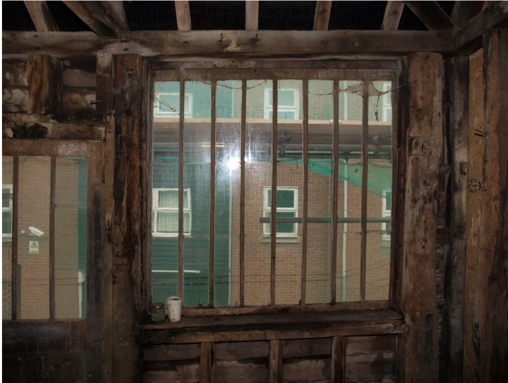
Plate 3: Window within the south elevation, facing south (7790_026)
