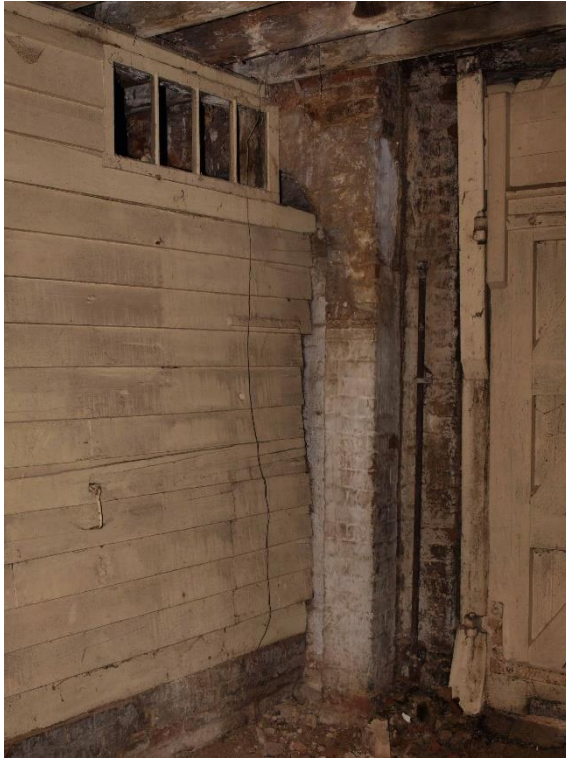
Plate 15: Detail of the four light window within the southern end of the partition wall, ground floor level, facing south-east (7790_039)
