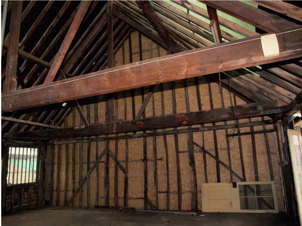
Plate 31: View of the west elevation at first floor level, facing south-west (7790_021)
