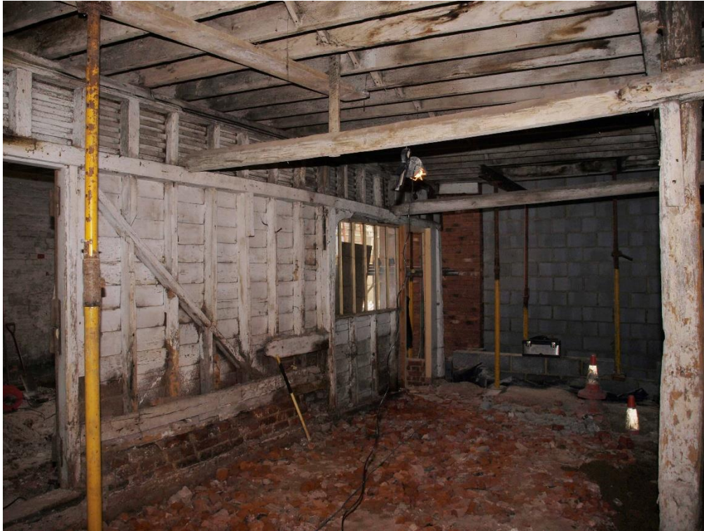
Plate 11: View of the eastern room at ground floor level, facing north-west (7790_041)
