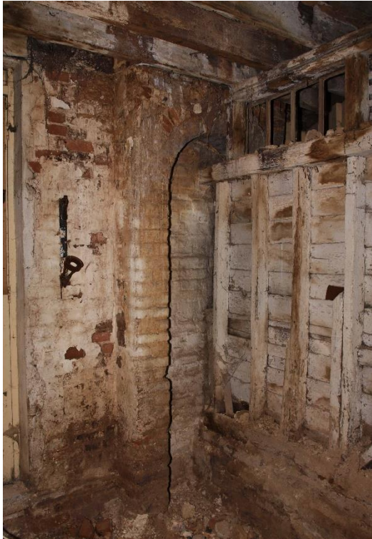
Plate 21: Detail of the relieving arch at ground floor level to the chimney above, south wall, facing south-west (7790_048)
