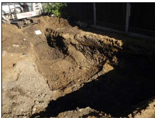
General view of monitored area looking north
