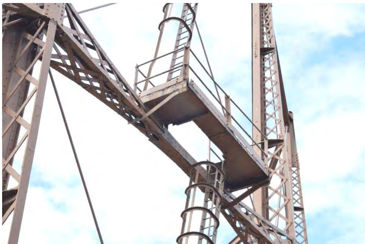
Plate 36: Gasholder No. 1, detail of the ladder platform, facing west (216)
