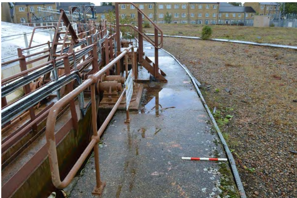
Plate 53: Gasholder No. 2, concrete tank surround and guard rail, facing south-west (13)
