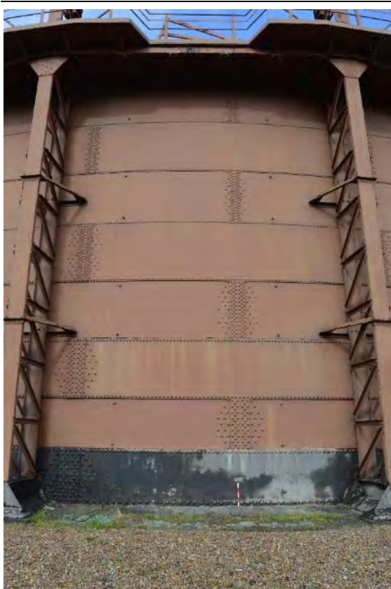
Plate 59: Gasholder No. 3, tank sheeting arrangement and vertical upright supports, facing west (80)
