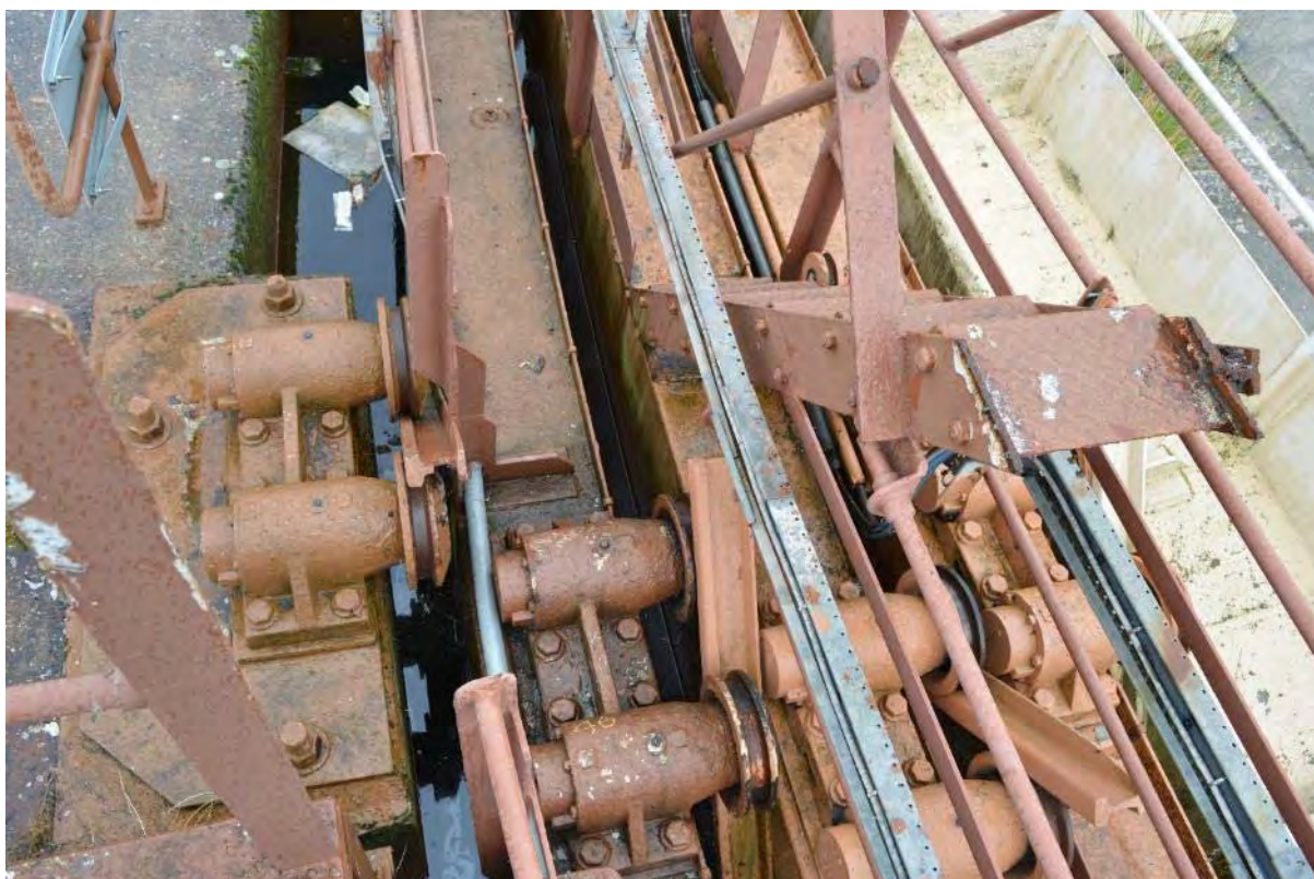
Plate 49: Gasholder No. 2, detail of roller-carriage arrangement on each lift, facing north (9)
