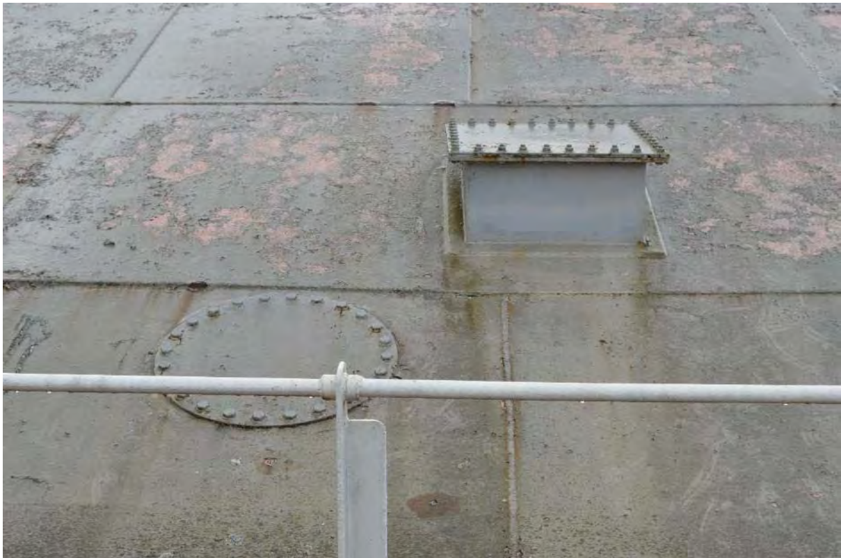
Plate 39: Gasholder No. 2, detail of bell inspection hatches, facing south-east (24)
