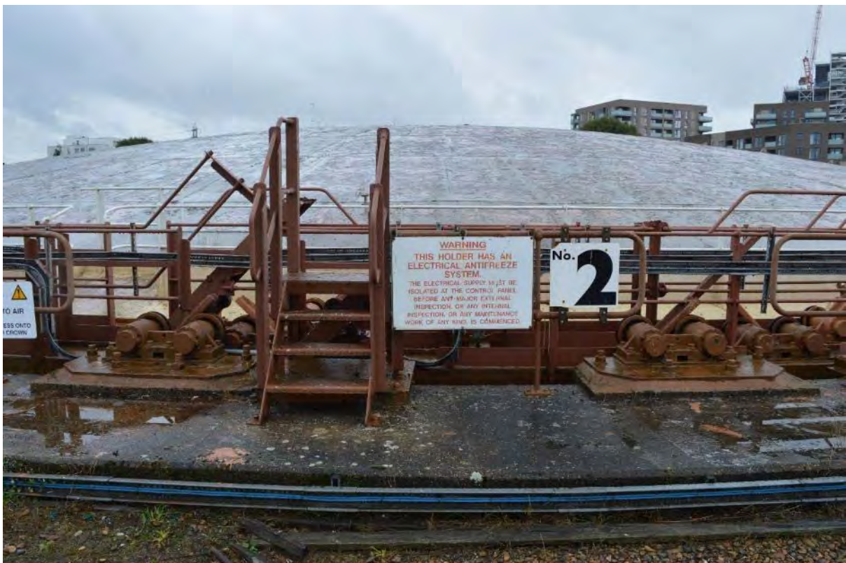
Plate 52: Gasholder No. 2, detail of tank access stair to first lift, facing east (5)
