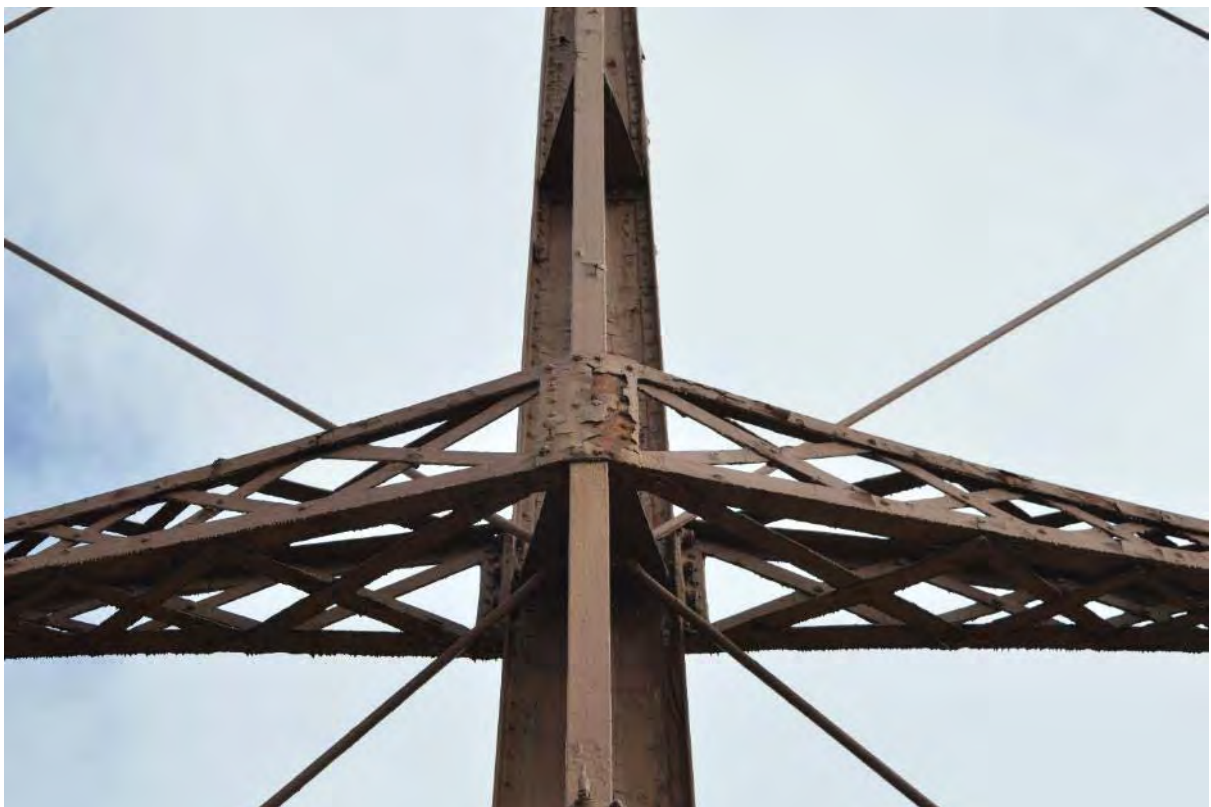
Plate 8: Gasholder No. 1, detailed arrangement of the girder and standard joining components, facing east (207)
