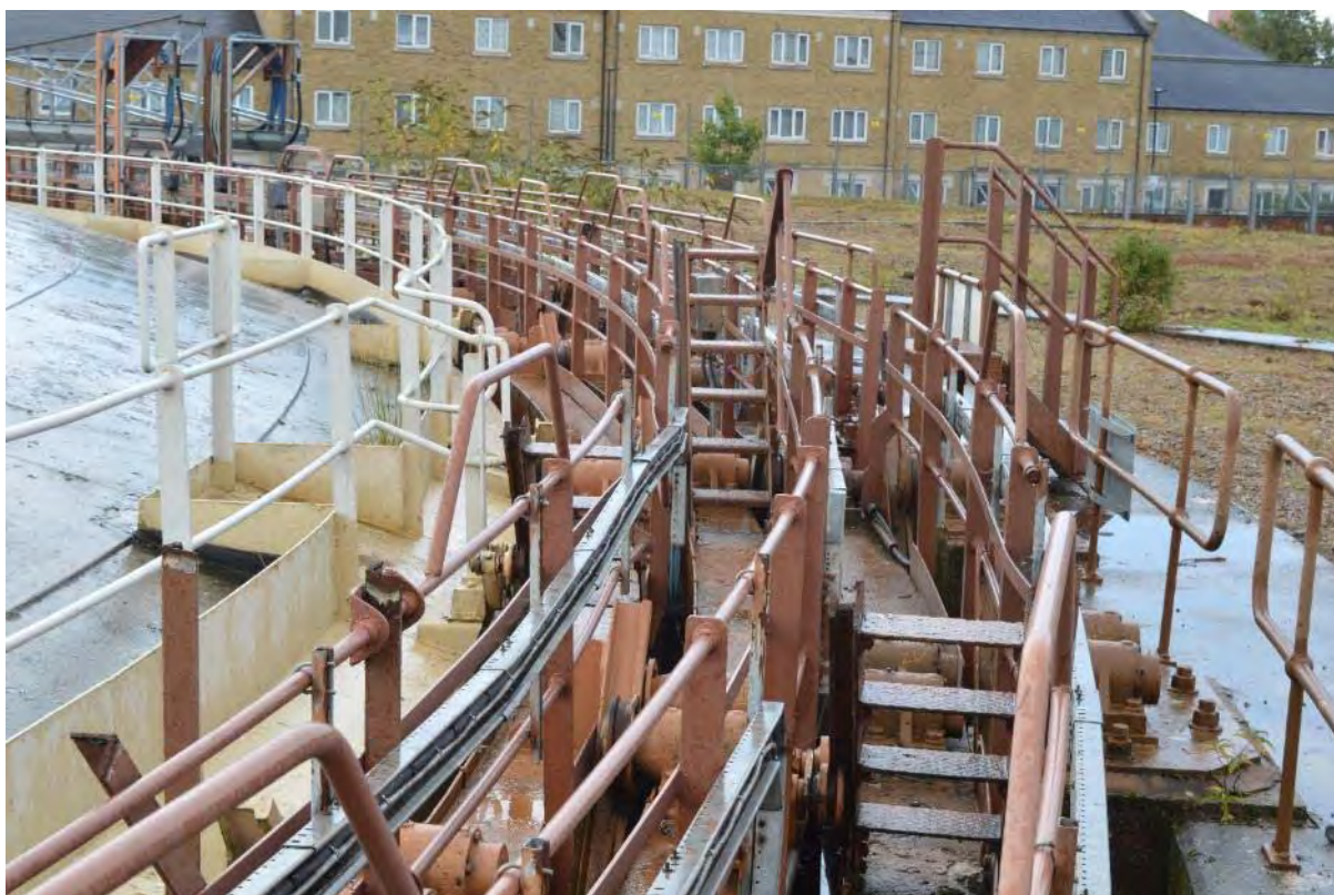
Plate 50: Gasholder No. 2, access stair arrangement, facing south (25)
