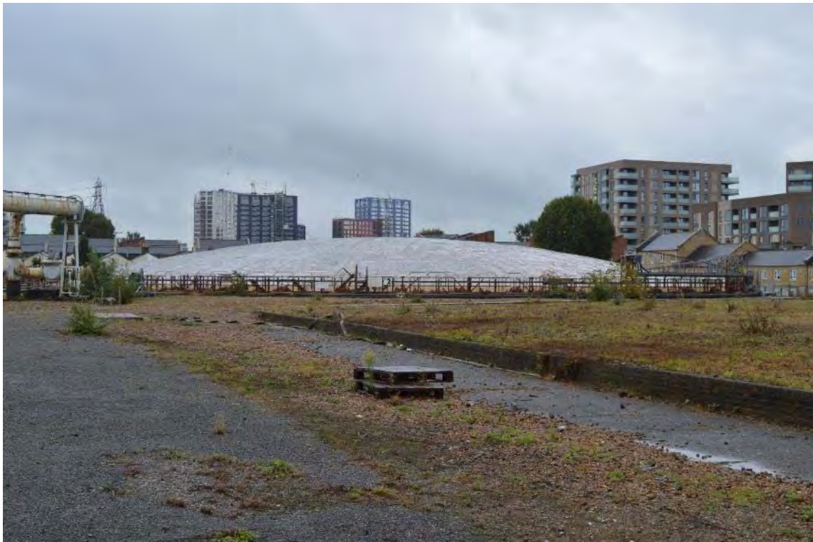
Plate 37: Gasholder No. 2, general view of bell, facing south-east (1)
