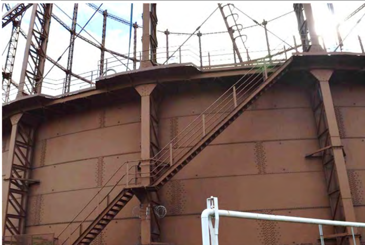
Plate 67: Gasholder No. 3, tank access stair arrangement, facing south-east (220)
