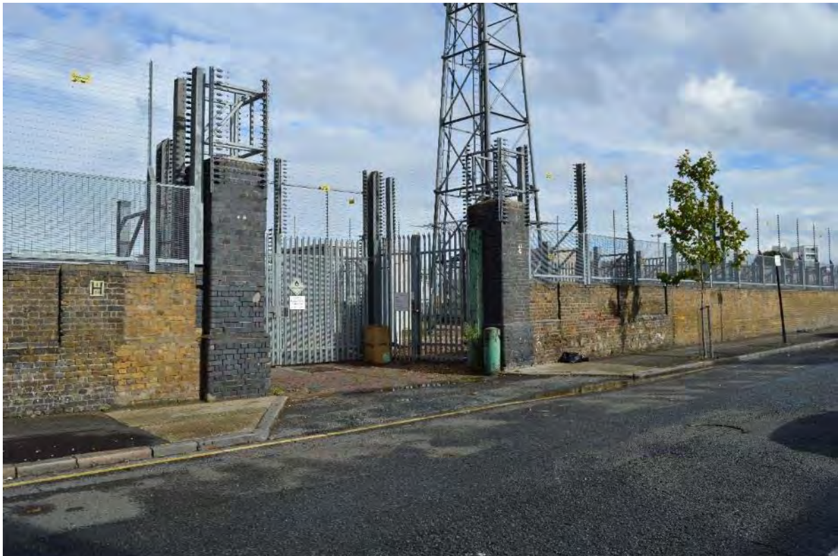
Plate 1: Original boundary wall to the south of the site, facing north-east (223)
