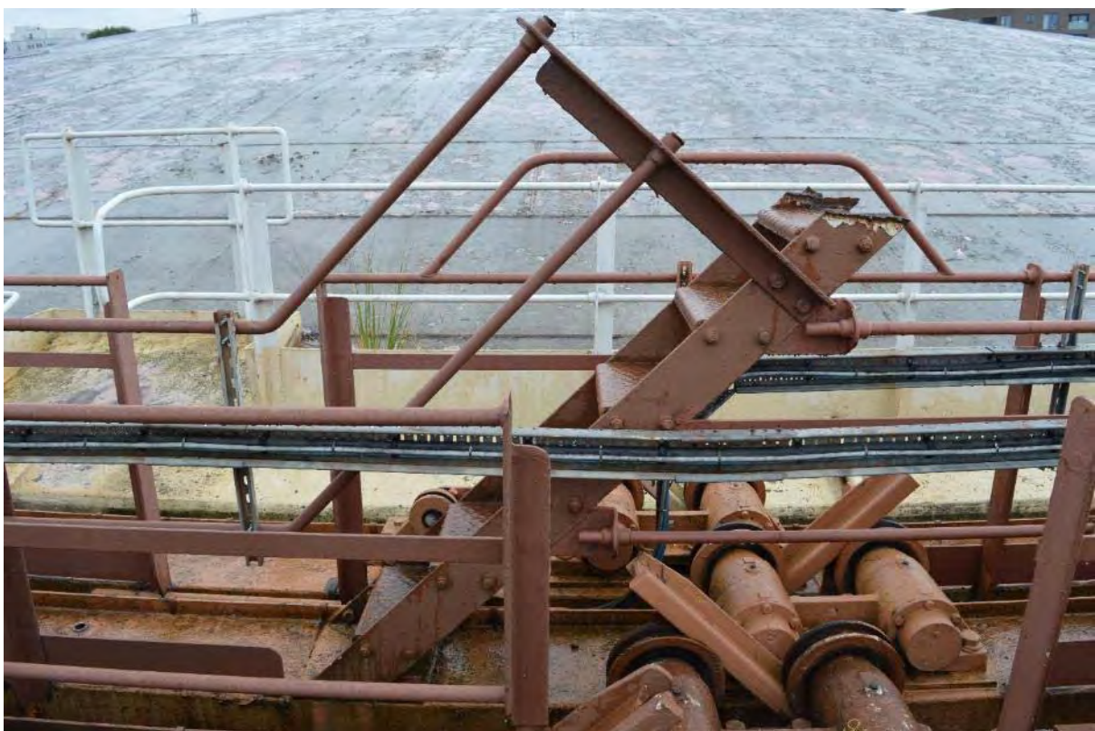
Plate 51: Gasholder No. 2, detail of lift stair and handrail, facing east (8)
