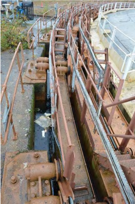
Plate 43: Gasholder No. 2, detail of lift and lute arrangement, facing north (10)
