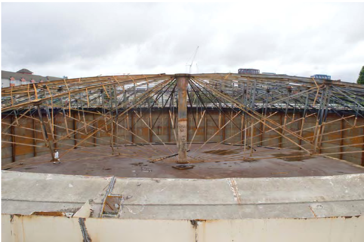
Plate 40: Gasholder No. 2, view of the framework supporting the bell, facing south-west (308)
