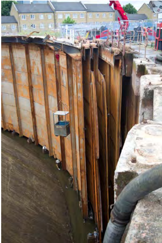
Plate 44: Gasholder No. 2, detail of the inner lift walls and concrete bases, facing west (270)
