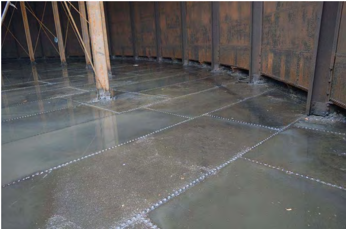
Plate 61: Gasholder No. 3, detail of the tank floor sheeting, facing south-east (350)
