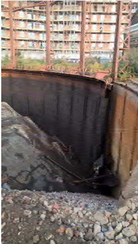
Plate 29: Gasholder No. 1, view of the inner lift wall sheeting, facing north-west (488)
