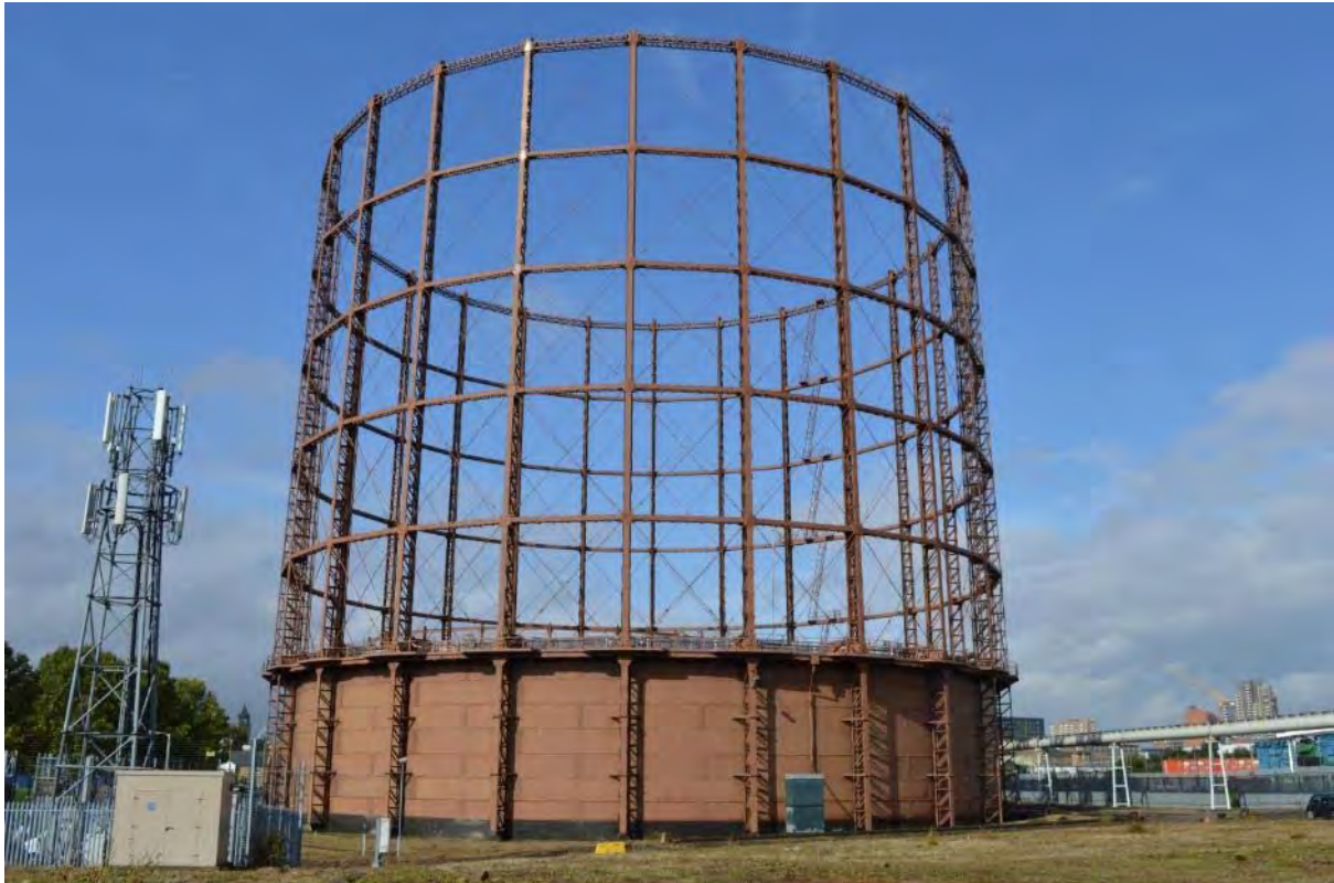
Plate 57: Gasholder No. 3, general view of the holder, facing west (70)
