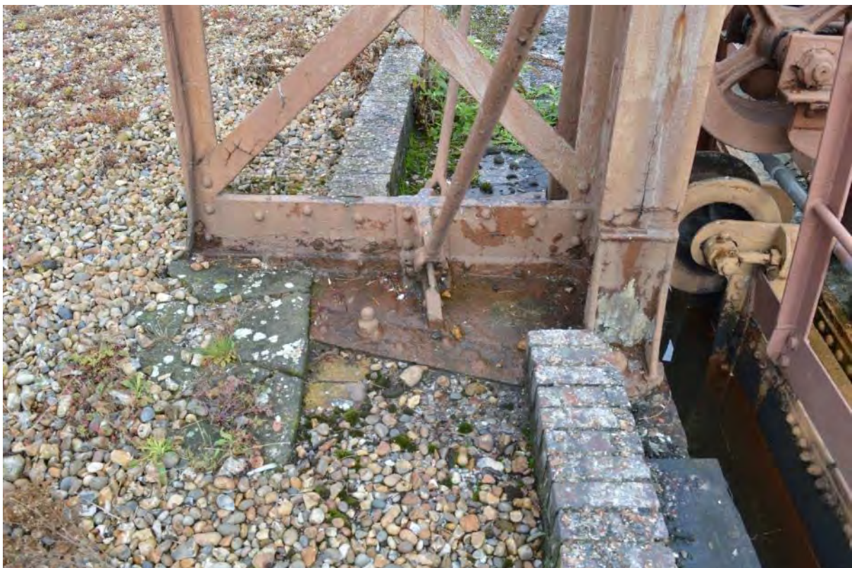
Plate 10: Gasholder No. 1, detail of a standard base arrangement, facing north (199)
