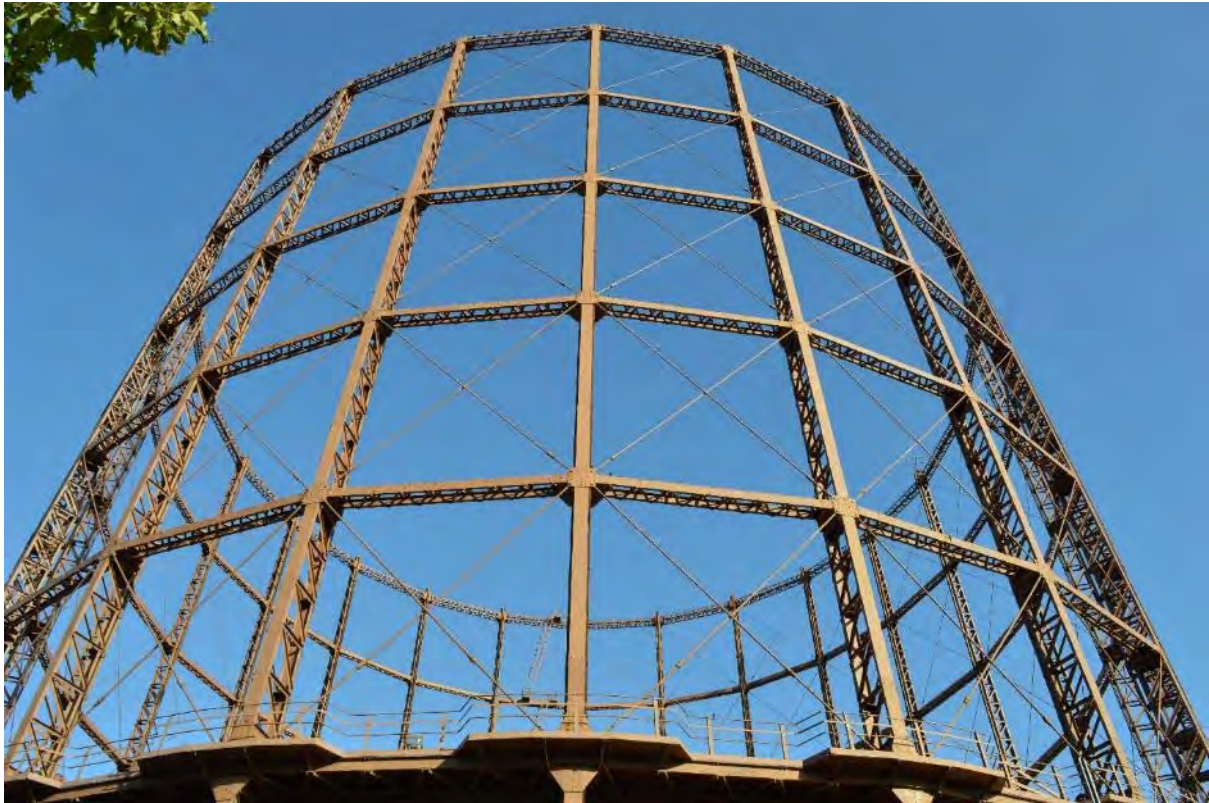
Plate 71: Gasholder No. 3, detail of the guide frame standards, facing north-west (52)
