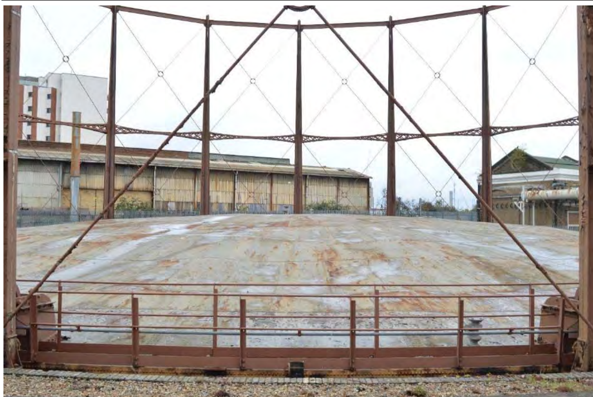
Plate 21: Gasholder No. 1, general view of the Armco bell sheeting, facing north-west (163)
