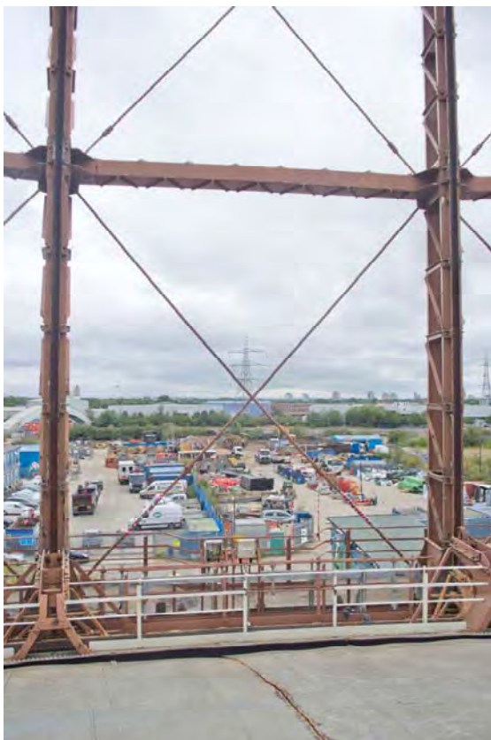
Plate 78: Gasholder No. 3, detail of the guide frame tension rods, facing north (241)
