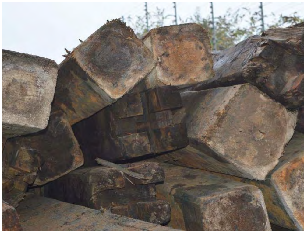
Plate 24: Gasholder No. 1, detail of the cross-section mortices cut within the top end of each post supporting the underside of the crown (post-deconstruction), facing west (455)
