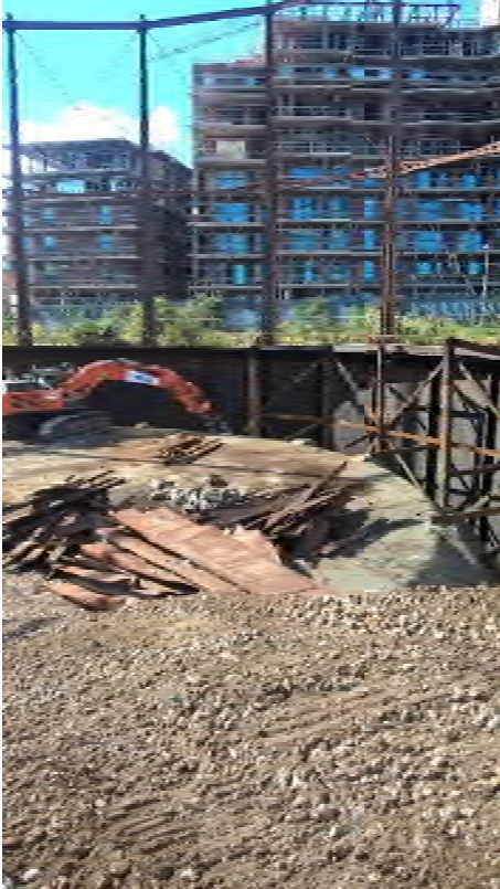
Plate 25: Gasholder No. 1, View of the outer rim of posts which frame the inner lift perimeter, note the board-like beam lattice, facing west (486)
