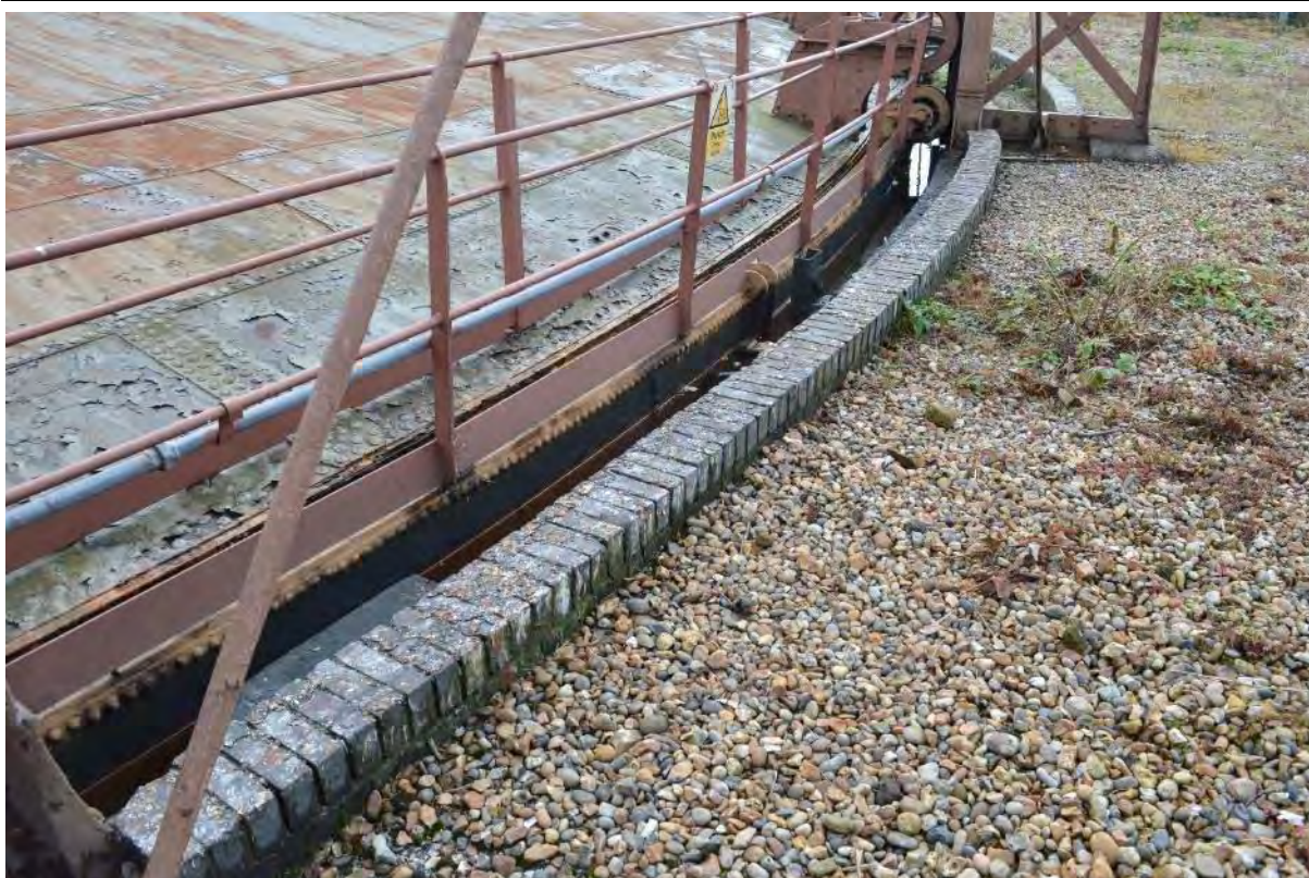
Plate 13: Gasholder No. 1, brick curb surround to the western edge, facing south-east (200)
