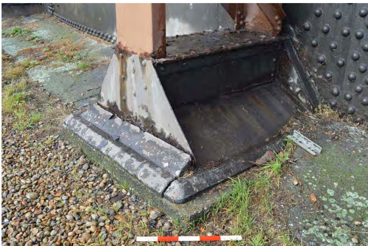
Plate 60: Gasholder No. 3, detail of vertical upright base construction, facing south-west (75)
