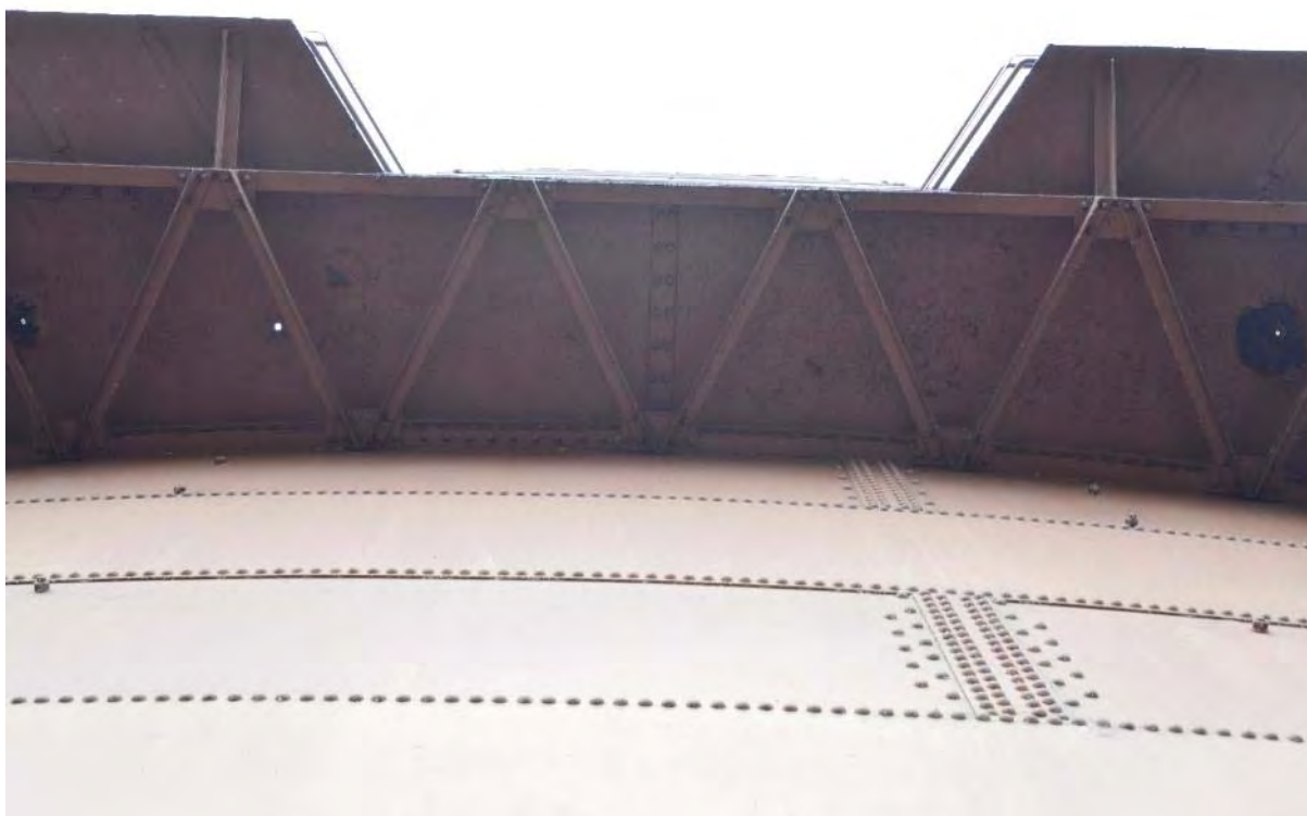
Plate 70: Gasholder No. 3, detail of the tank platform underside supports, facing east (84)
