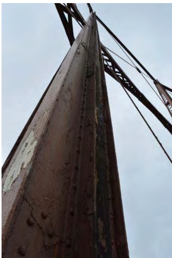
Plate 6: Gasholder No. 1, rolled 'I' section guide rail, facing east (178)
