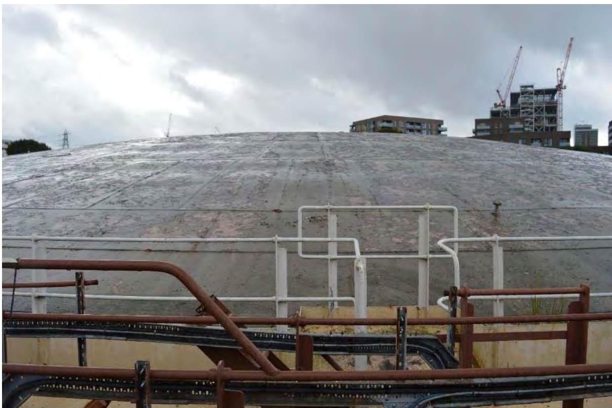
Plate 38: Gasholder No. 2, detail of bell sheeting, facing east (14)
