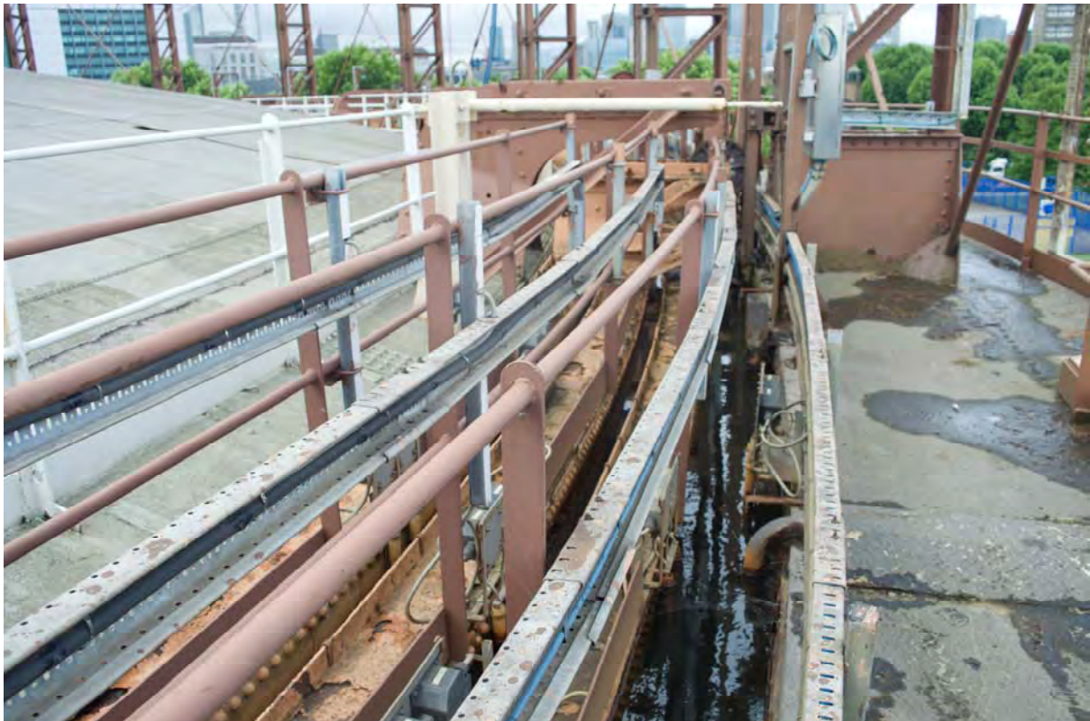
Plate 84: Gasholder No. 3, detail of the lifts and lutes, facing west (324)
