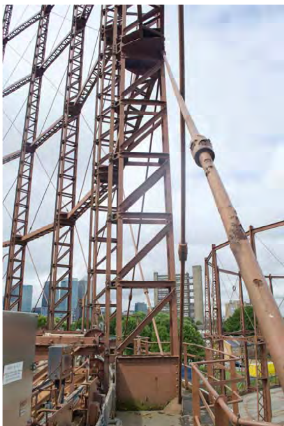
Plate 75: Gasholder No. 3, detail of the guide frame stanchion bases, facing south-west (327)
