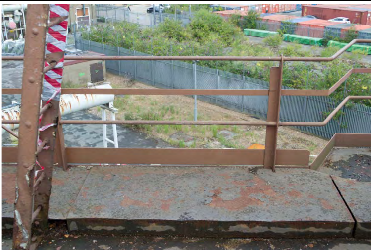
Plate 69: Gasholder No. 3, detail of the tank platform, facing north (333)
