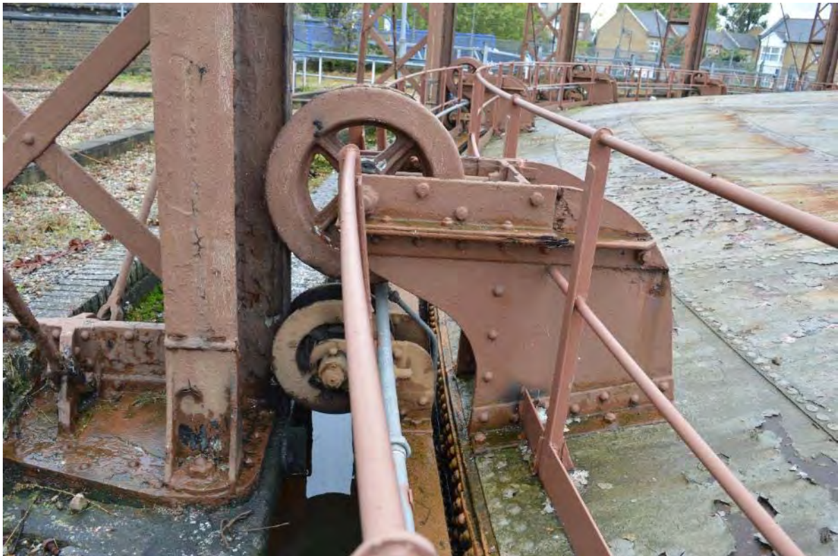
Plate 31: Gasholder No. 1, radial guide roller arrangement engaged with the rolled 'I' section guide rail, facing south-east (170)
