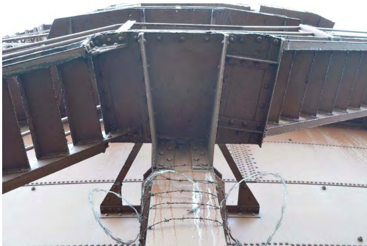
Plate 68: Gasholder No. 3, construction detail of tank stair half-landing, facing east (102)
