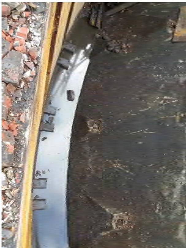
Plate 15: Gasholder No. 1, detail of the dumping outer edge, facing south-west (462)
