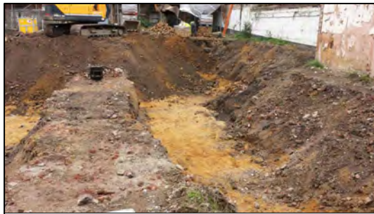
View east across site
