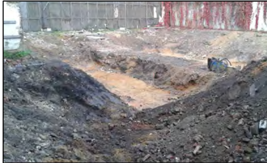
View north-west across site
