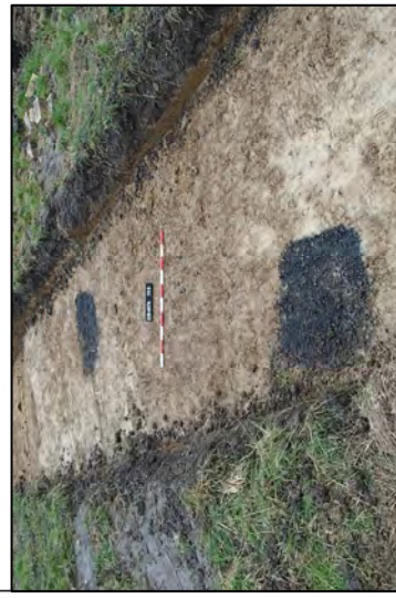
Asphalt bedding for brick plinths 5/005, looking north-west (1m scale)
