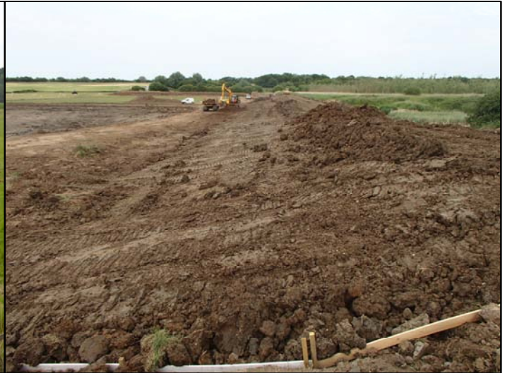
Fig.3b. The new and built-up north embankment, Areas 1 and 2, looking west
