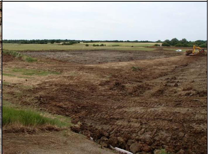
Fig. 3d. Area 3 excavated borrow pit, looking south-west
