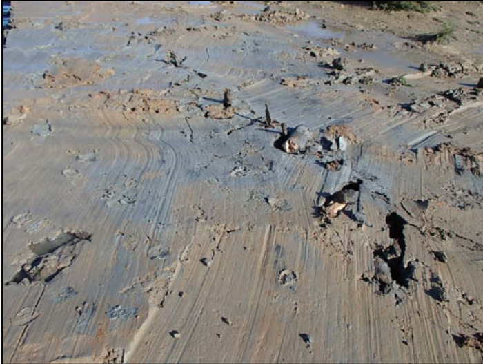
Fig.5c. Line of stakes 106 in the south breach Area 9, looking north-east
