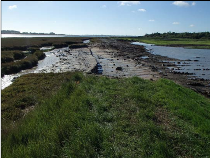
Fig.5a. The south breach of of the sea wall looking south, Area 9. The water to the right was the result of the first tidal influx after the breach was cut.
