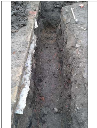
Foundation trench, view looking north west
