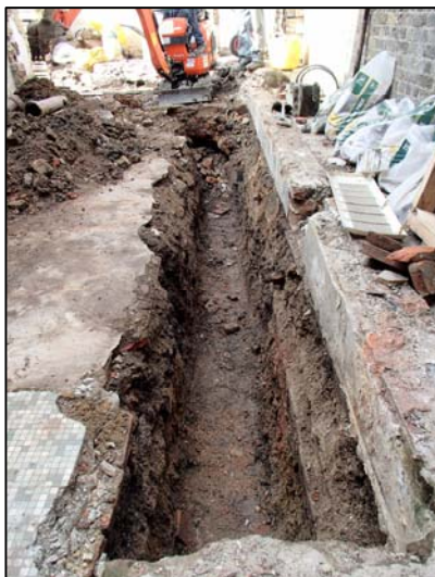
Foundation trench, view looking north west
