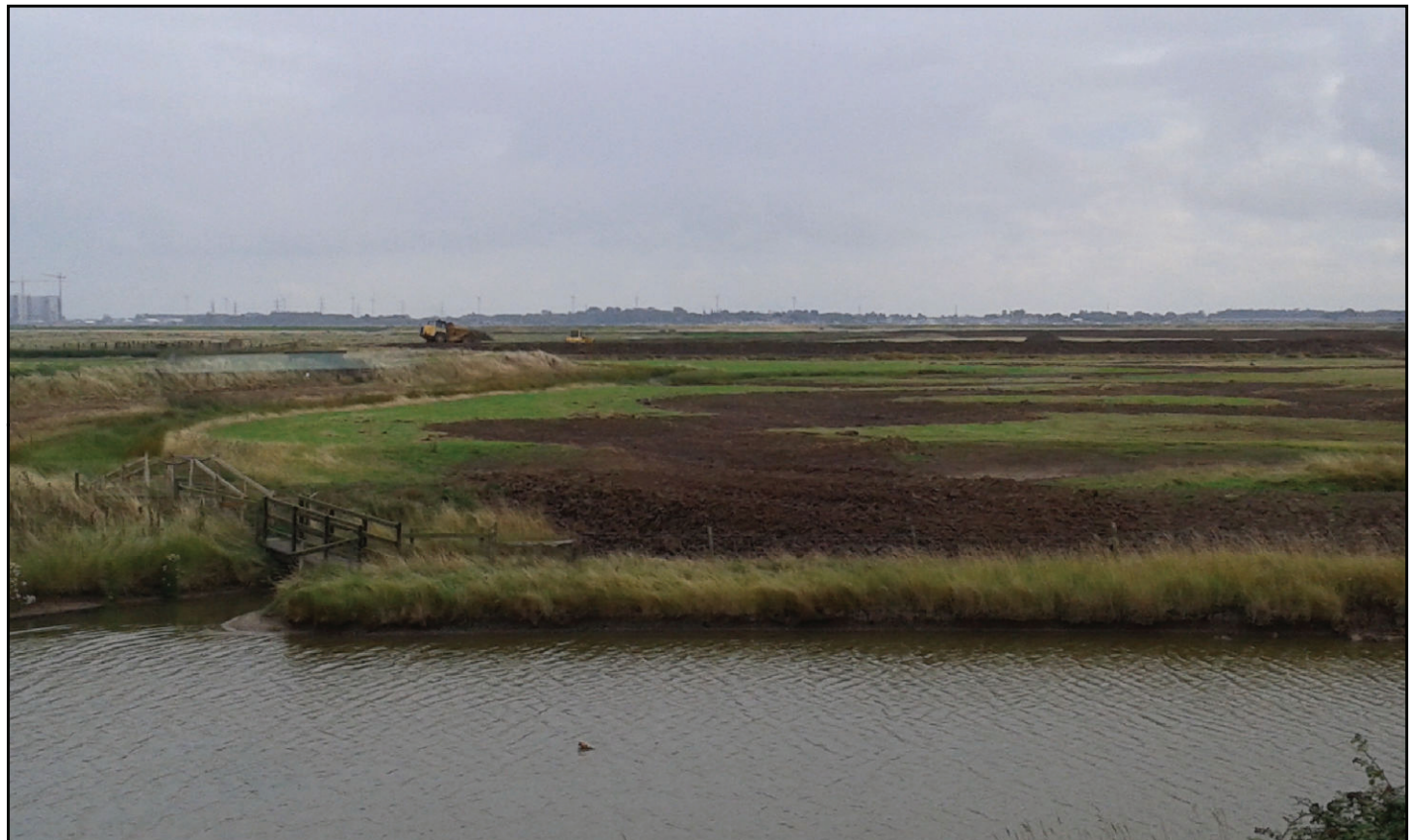
View south across the reserve showing new creeks. The recently constructed counterwall is on the left. Bradwell Power Station can be seen in the distance.
