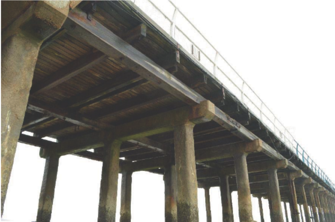
Plate 5: Outer pier substructure, looking east (66)
