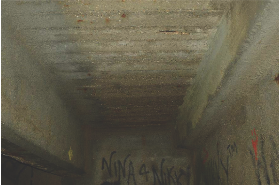
Plate 3: Amusement hall substructure, looking north-west (53)
