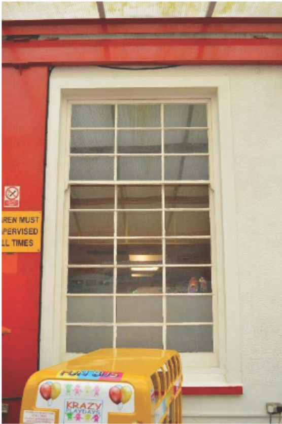
Plate 9: Former external window on original west elevation, looking east (3)
