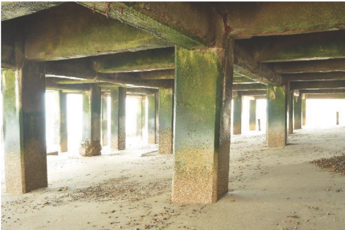
Plate 2: Amusement hall substructure, looking south (50)
