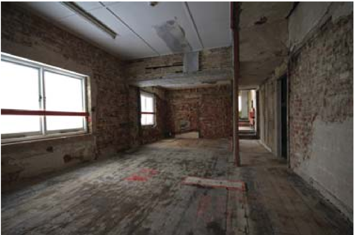
Plate 83: Overview of Room 14. (#222)
