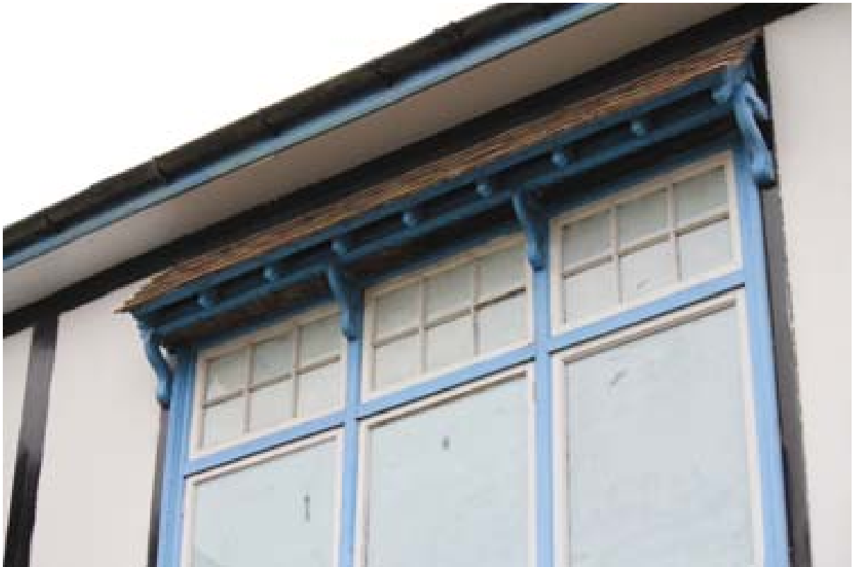
Plate 4: Tiled hoods and moulded brackets above window in the north elevation of the Old Hall. (#55)
