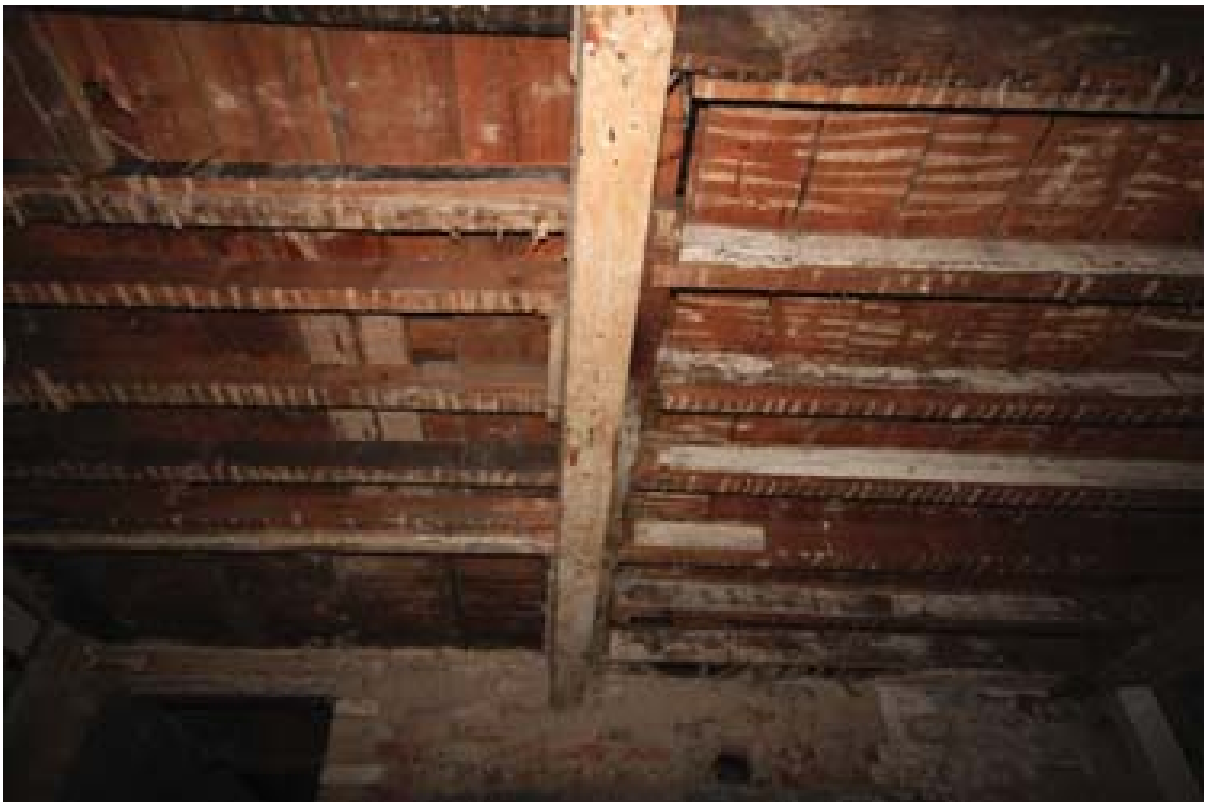
Plate 53: Ceiling construction in the east end of Room 6. (#153)
