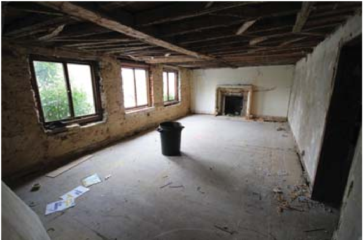
Plate 19: Overview of Room 1. (#63)
