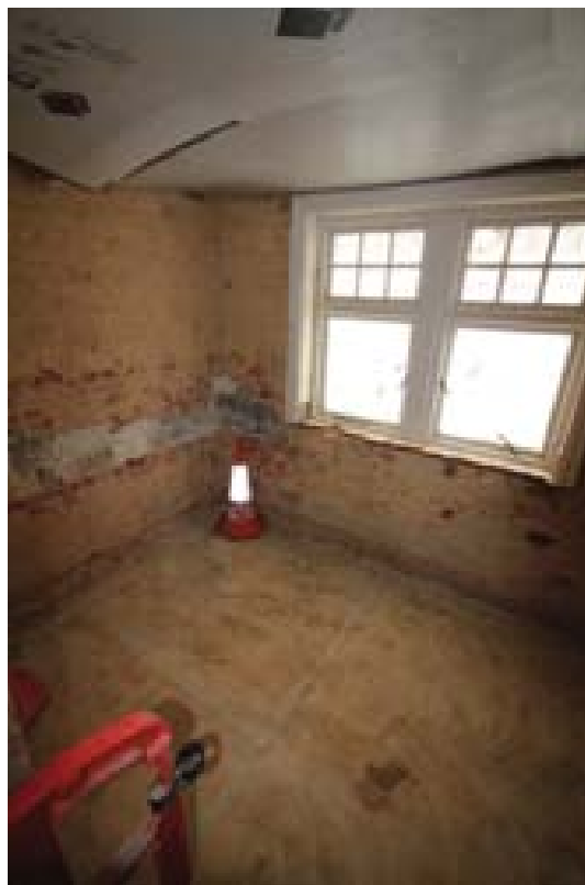
Plate 90: Fireplace at the west end of Room 14. Note the difference in construction between the chimney stack and wall to its north (right). (#224)
