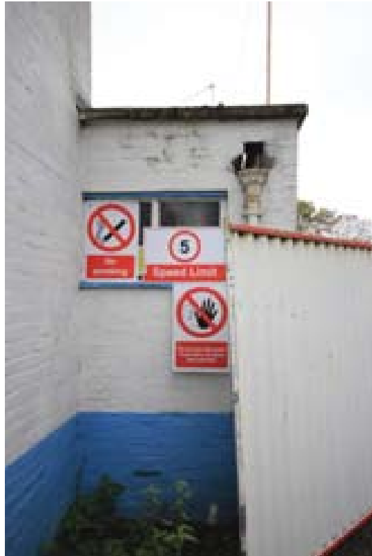
Plate 130: Window and downpipe, east elevation of Block D. (#346)
