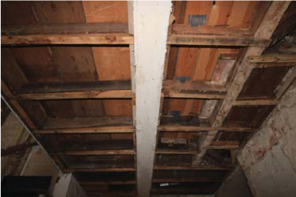
Plate 28: Ceiling construction in the hall, Room 2. (#88)
