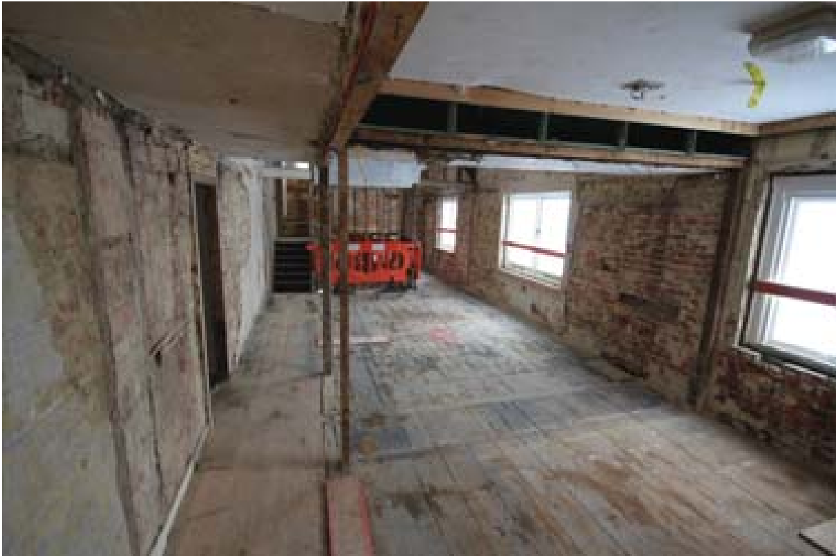
Plate 84: Overview of Room 14. (#303)
