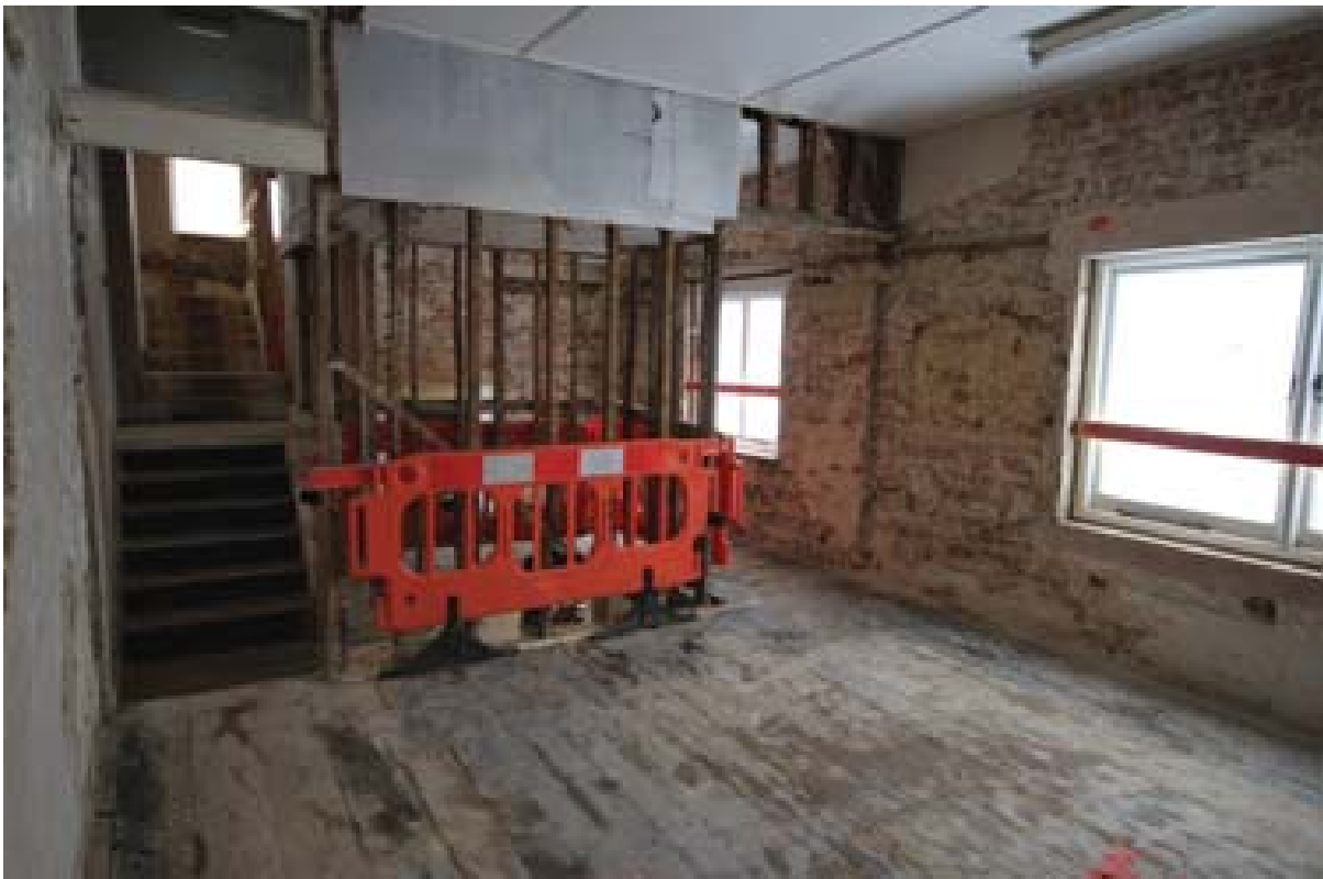
Plate 85: Studs walls encompassing the main stair, Room 14. (#288)
