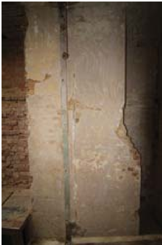
Plate 69: Chimney stack, Room 10. Note the wall scar. (#319)
