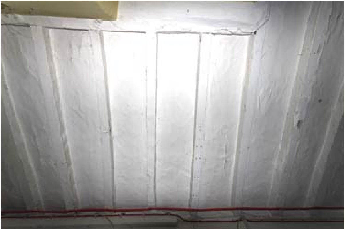
Plate 52: Joists above the west end of Room 6. (#149)
