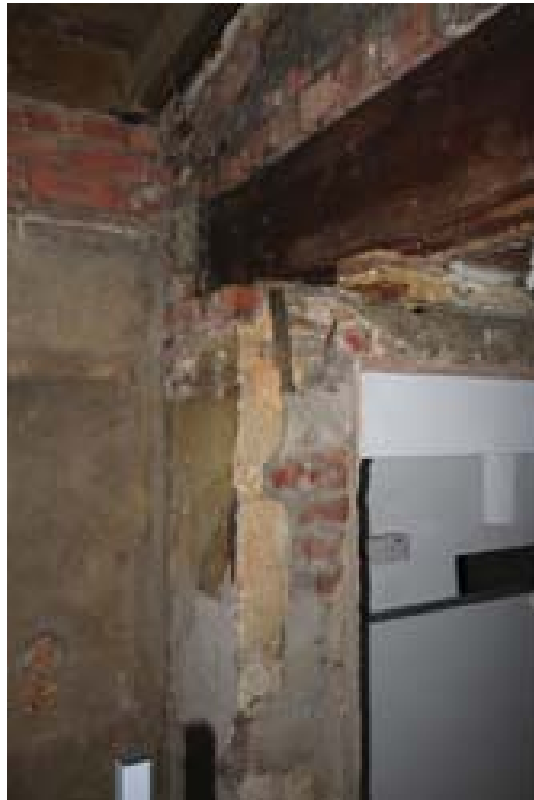
Plate 57: Removed wall, inserted beam, and obsolete girder in Room 7. (#324)
