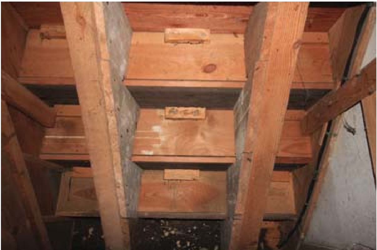
Plate 31: Construction of the stair, Room 2. (#94)
