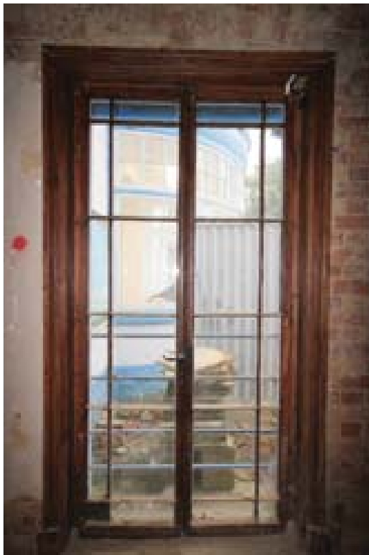
Plate 33: Inserted French door, Room 3. (#324)
