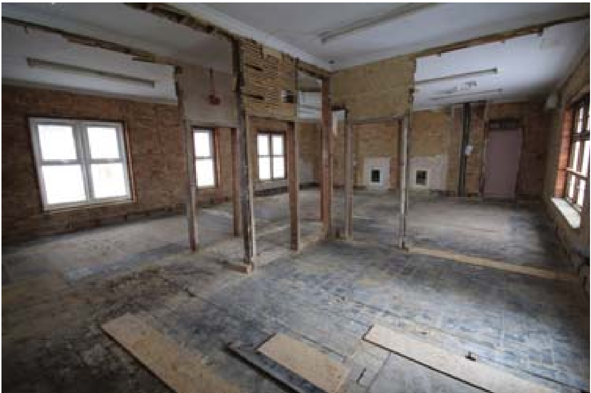
Plate 107: Overview of Room 21. (#267)
