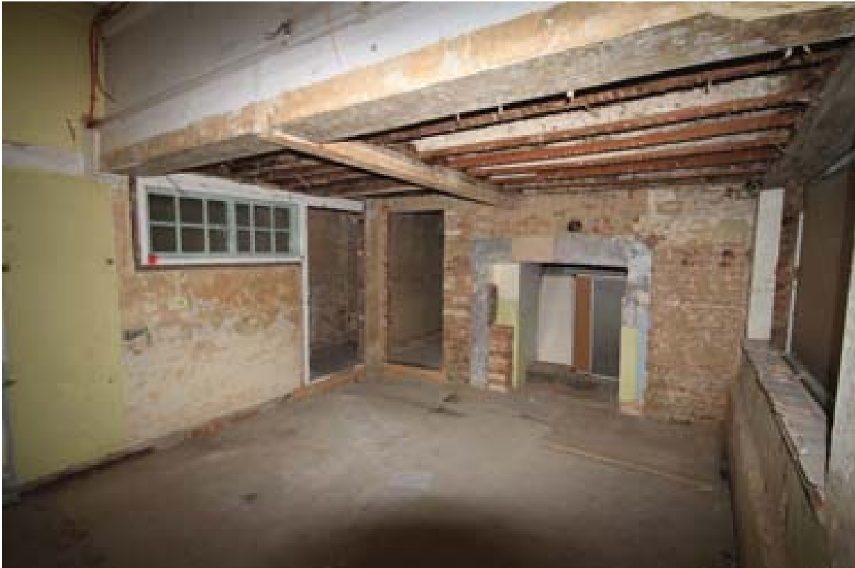
Plate 46: Overview of Room 6. (#151)
