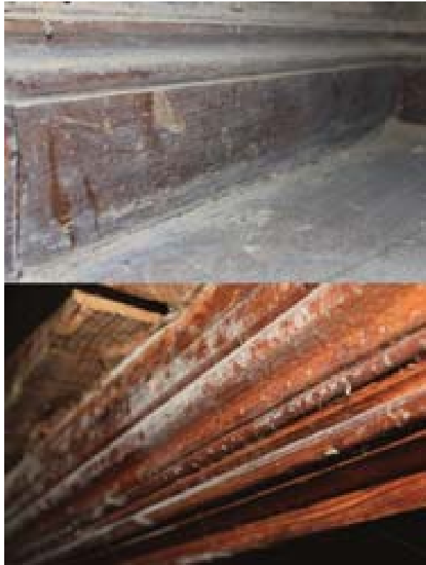
Plate 18: Detailed examples of extant architrave and skirting form, Room 2. (#103 and #104)
