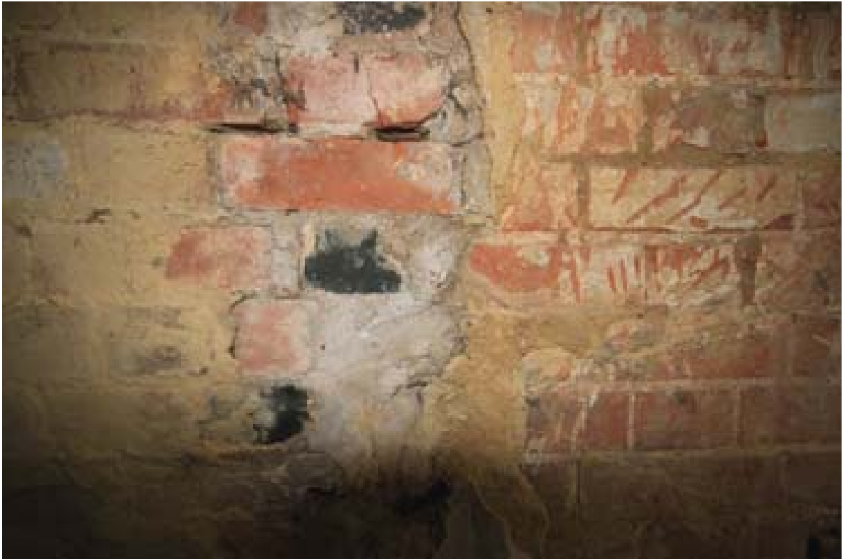
Plate 106: Intersection of brickwork of Rooms 10 (right) and 20 (left). (#307)
