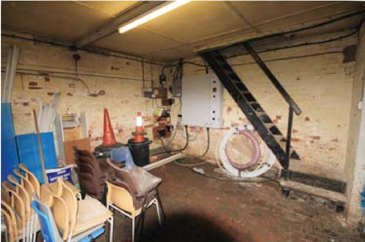
Plate 132: Overview of the cart room, Block D. (#399)
