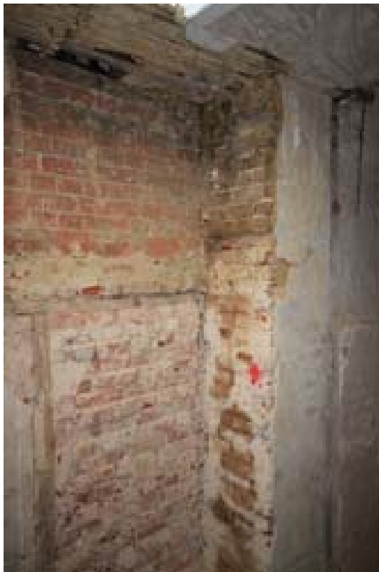
Plate 71: Inserted chimney stack, Room 10. (#308)
