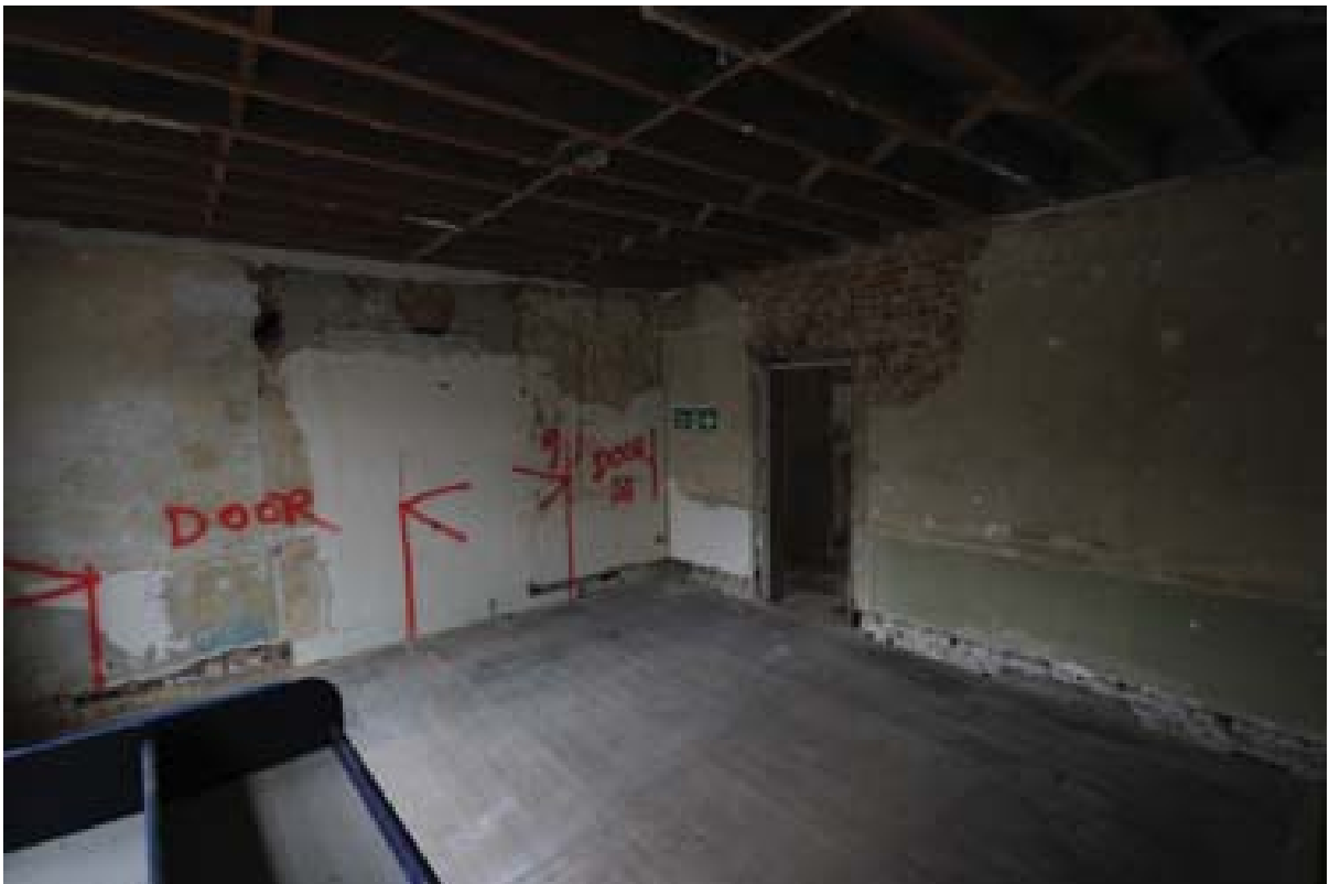
Plate 41: Overview of Room 5. (#124)
