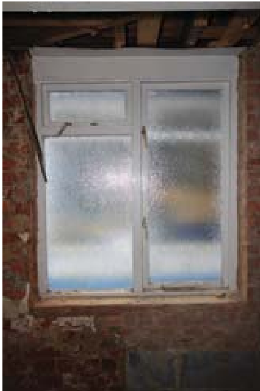
Plate 61: Inserted window in the south wall of Room 8. (#209)
