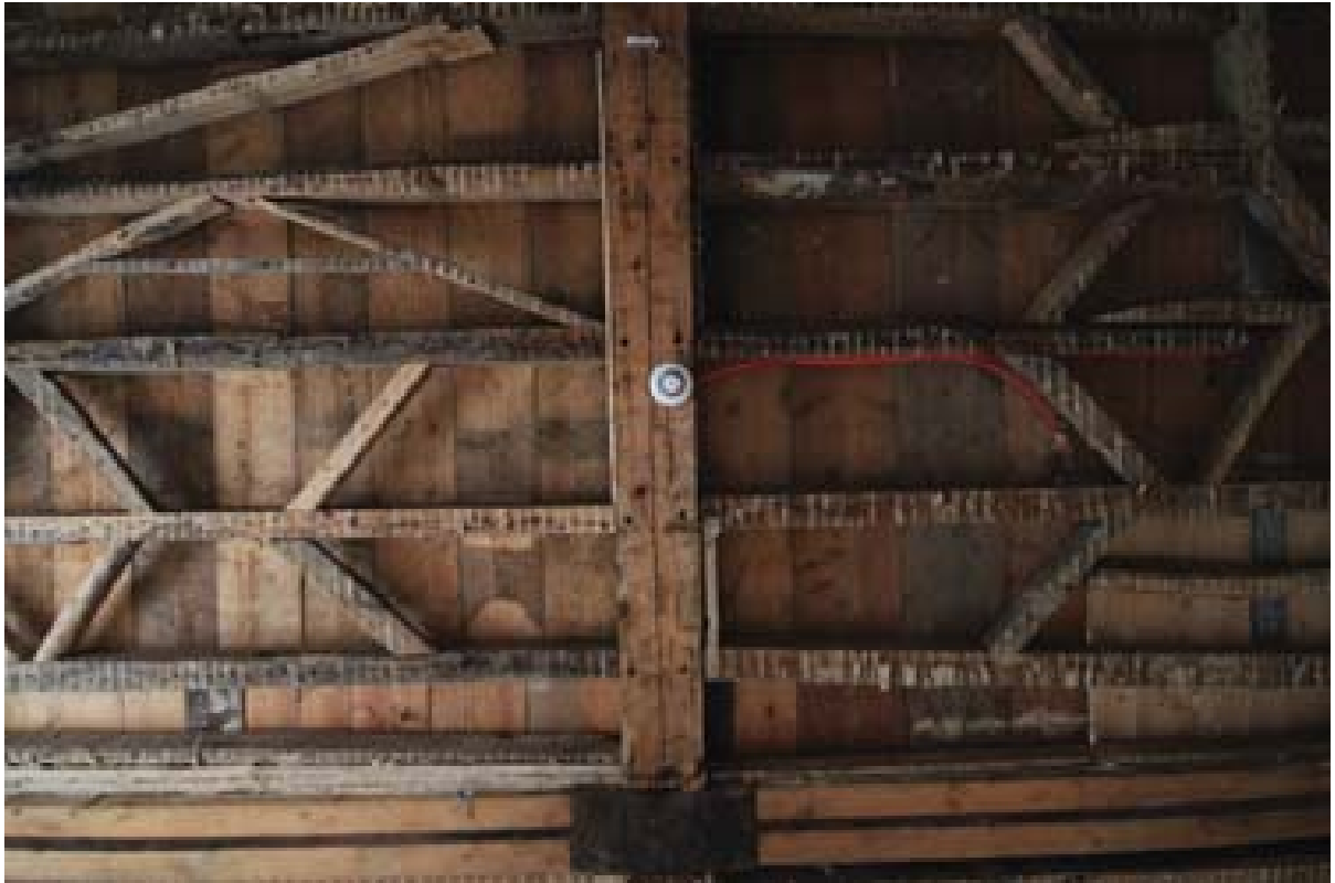
Plate 22: Construction of the ceiling in Room 1. (#70)
