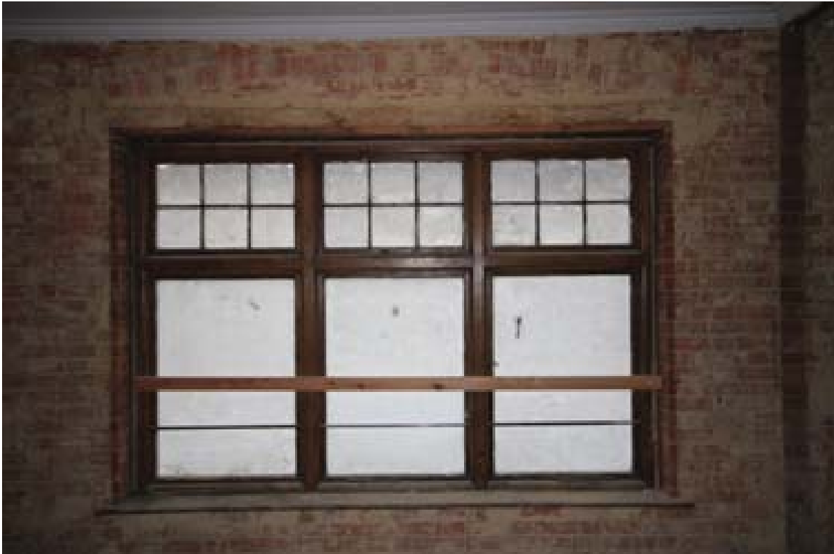
Plate 110: Triple-casement window in the north wall of Room 21. (#273)
