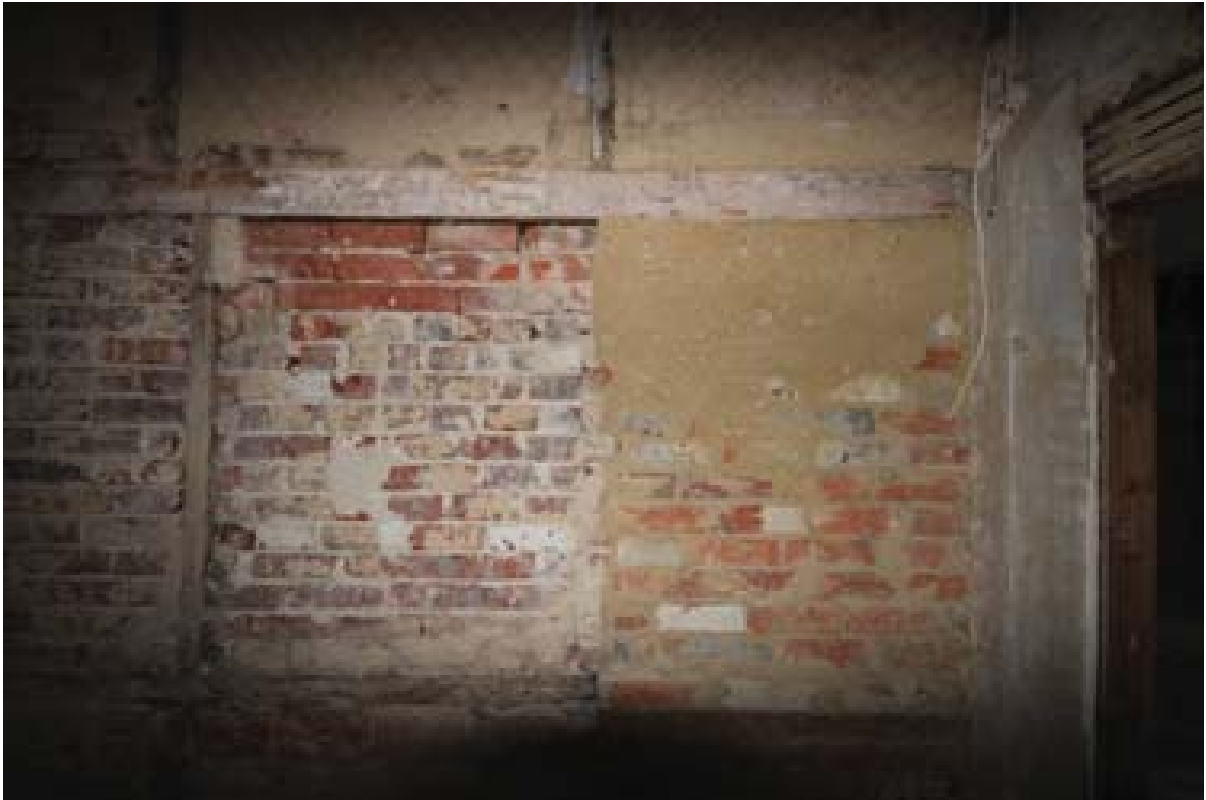
Plate 102: Blocked doorway west to Room 17, Room 18. (#293)
