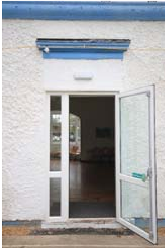
Plate 12: Inserted doorway in the south elevation of the Old Hall. (#37)
