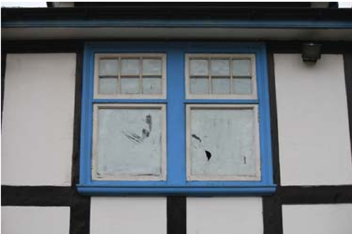
Plate 3: Presumed early 20 th -century windows in north elevation of Block A. (#60)
