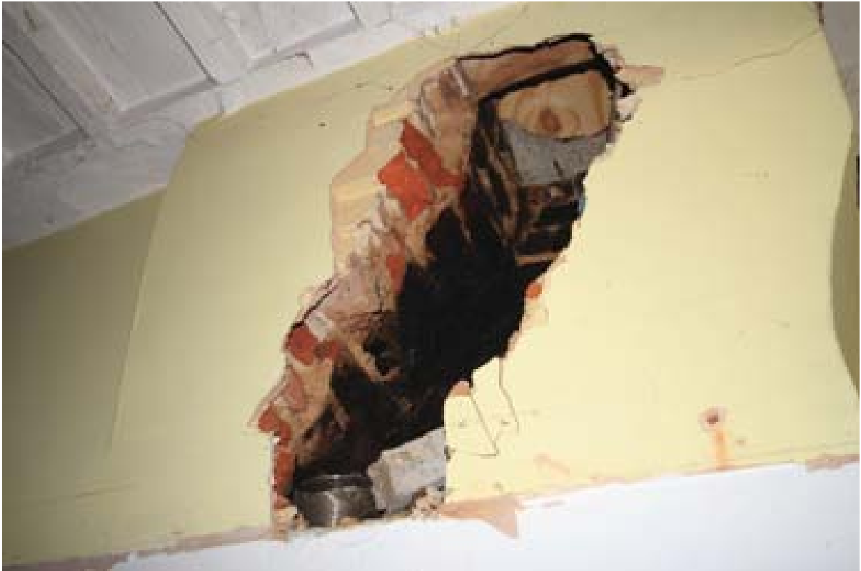
Plate 50: Exposed flue, Room 6. (#145)
