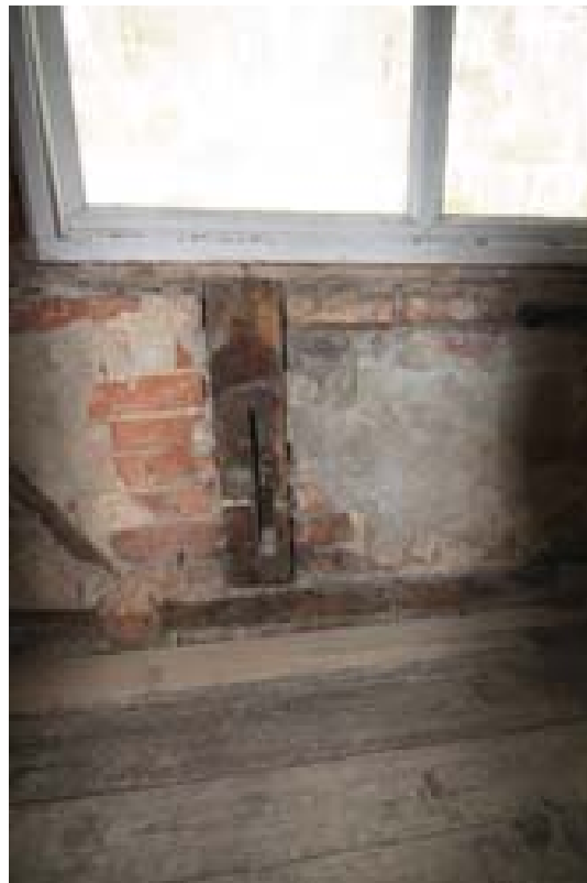
Plate 97: Reused timber with defunct mortice, Room 17. (#260)
