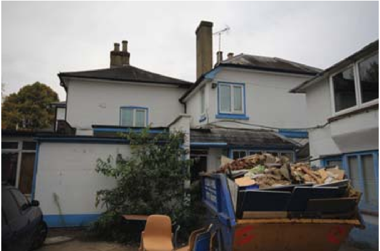
Plate 14: East elevation of the core building. (#7)
