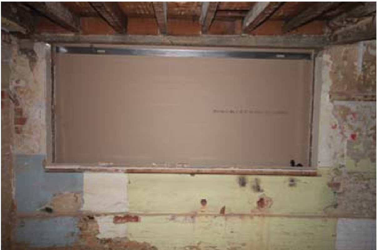
Plate 49: Blocked window in south wall of Room 6. (#155)
