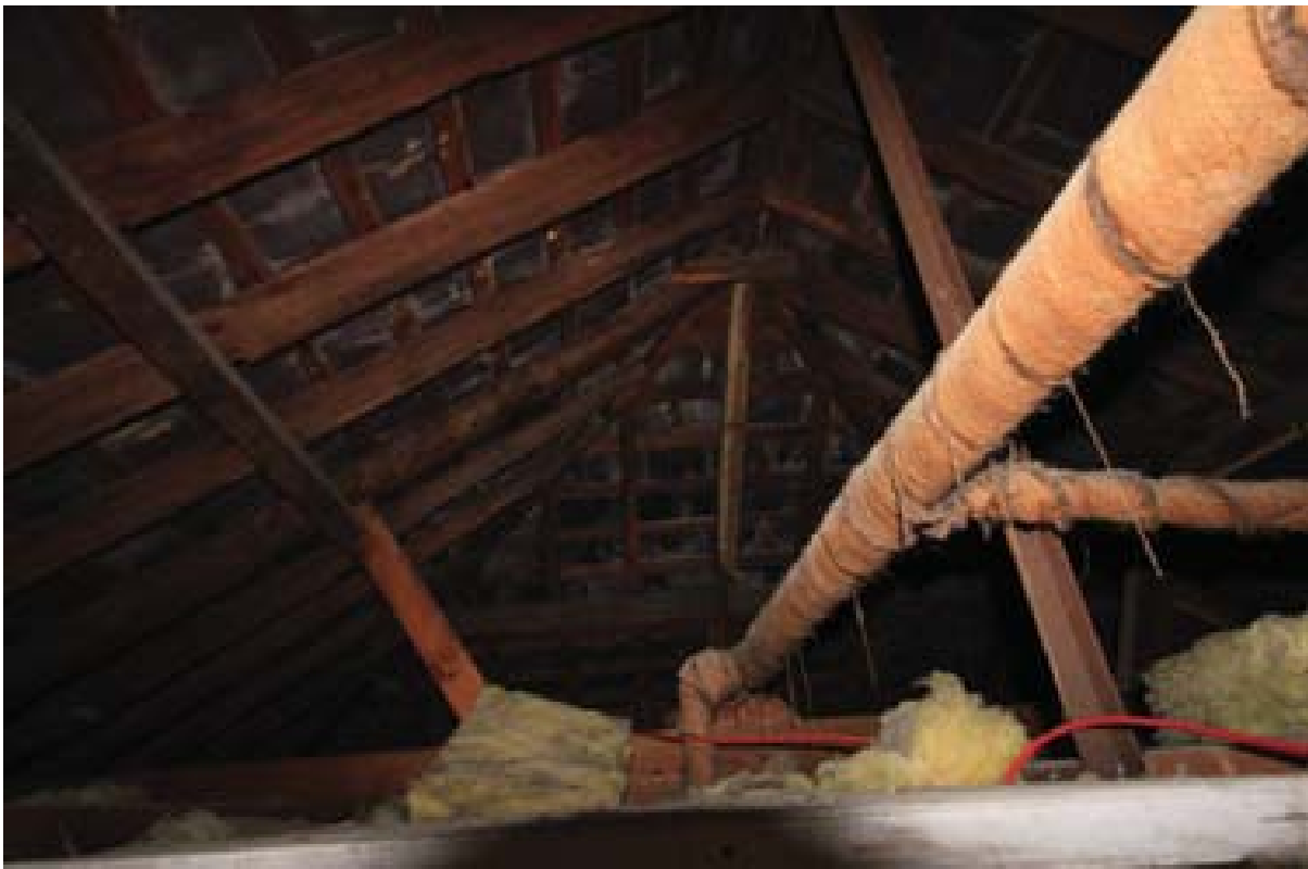
Plate 115: Roof space above Room 17. (#235)
