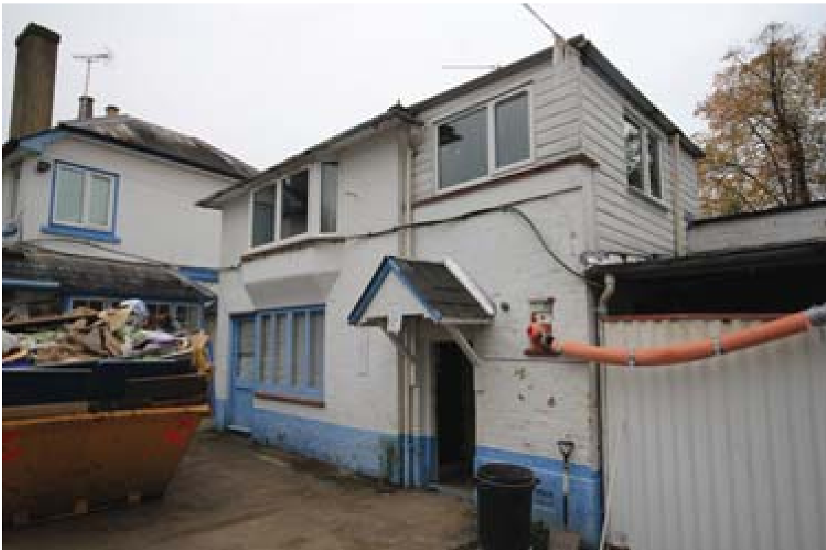
Plate 119: Principal (south) and east elevations of Block C. (#341)
