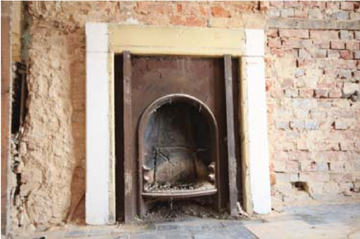
Plate 90: Fireplace at the west end of Room 14. Note the difference in construction between the chimney stack and wall to its north (right). (#224)
