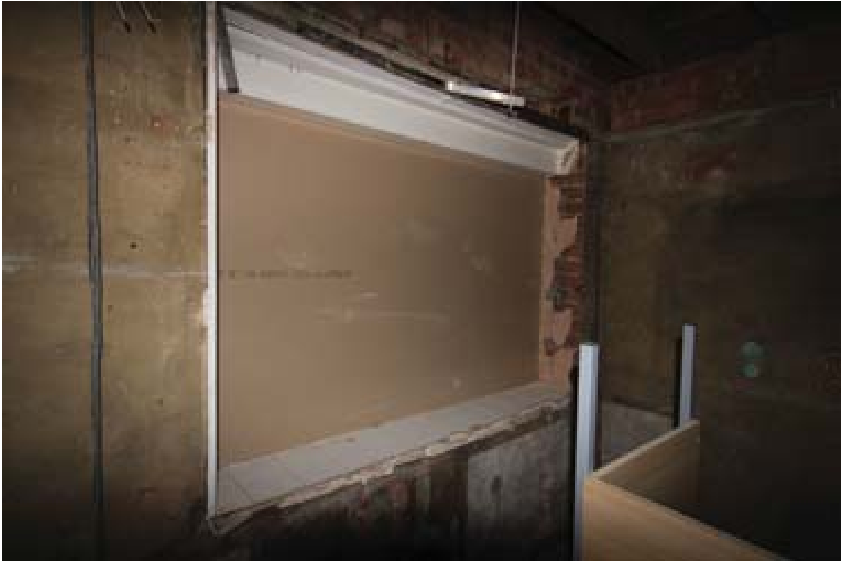
Plate 56: Service hatch extension at south end of Room 7. (#168)
