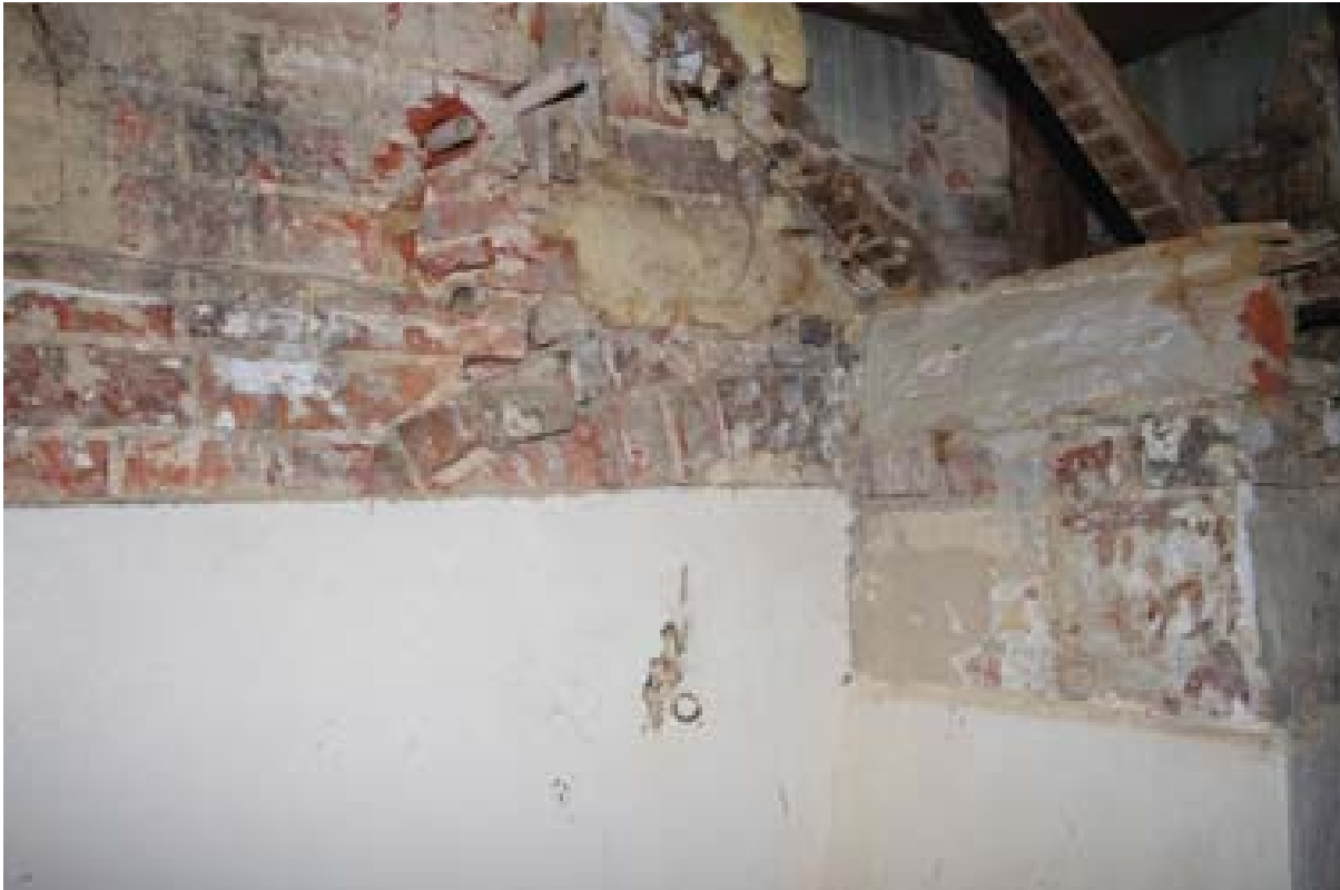
Plate 72: Inserted chimney stack and blocked opening, Room 10. (#185)
