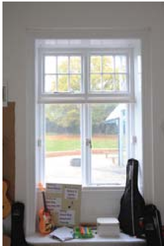
Plate 81: Overview of window in south wall of Room 13. (#218)
