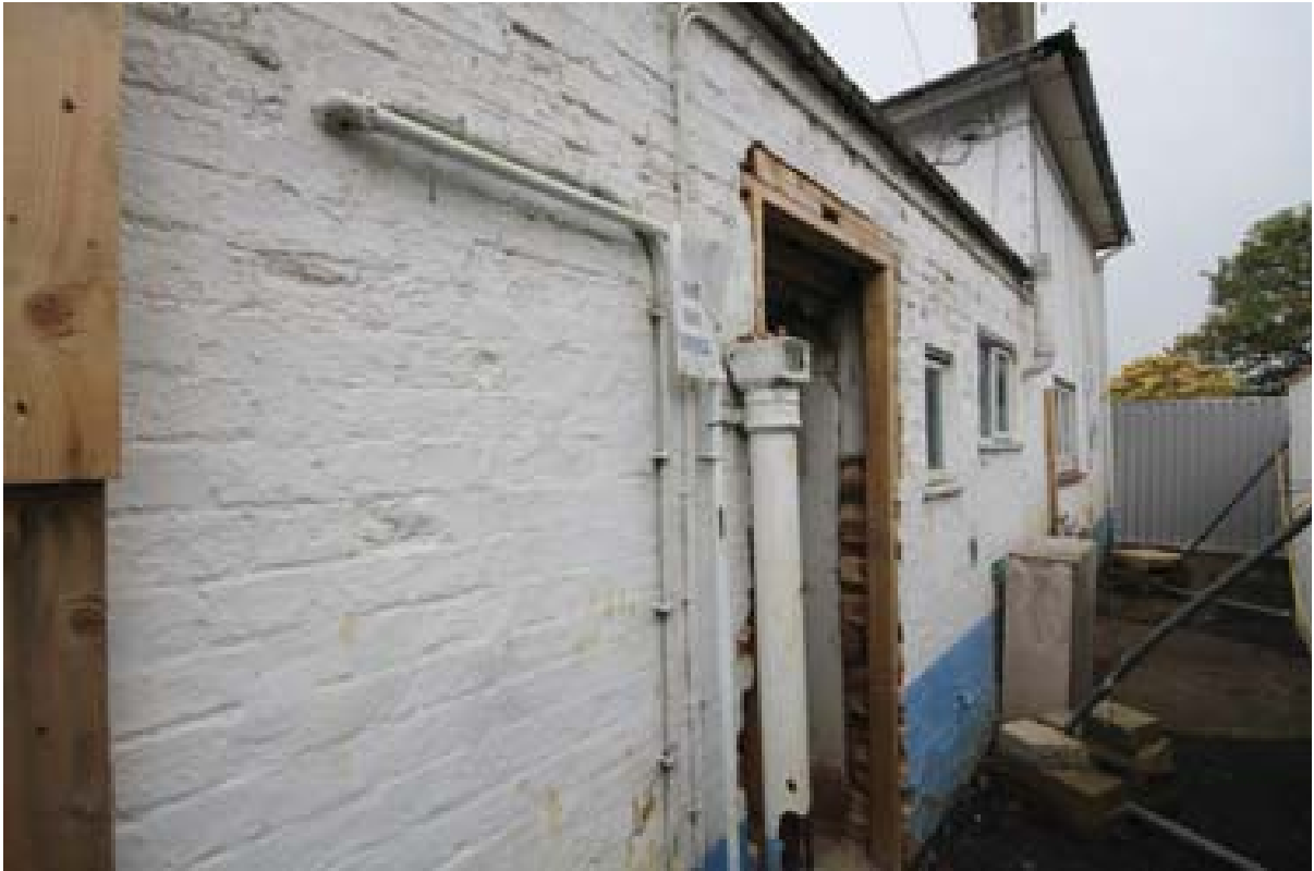
Plate 120: North elevation of Block C. (#382)
