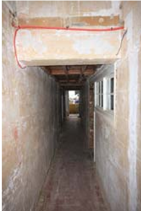
Plate 62: Overview of the servants' corridor (Room 9). (#139)
