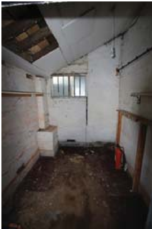
Plate 137: Storage room, Block D. (#415)
