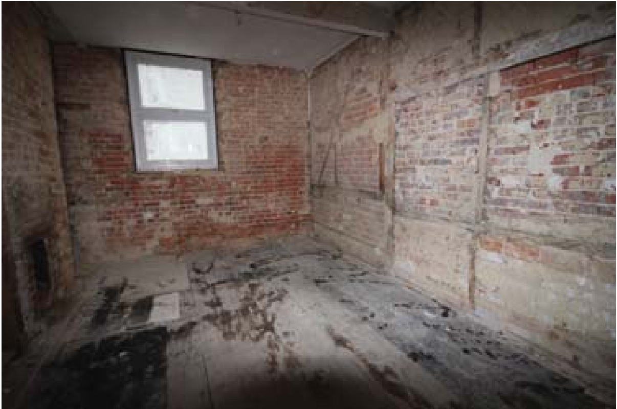
Plate 100: Overview of Room 18. (#292)
