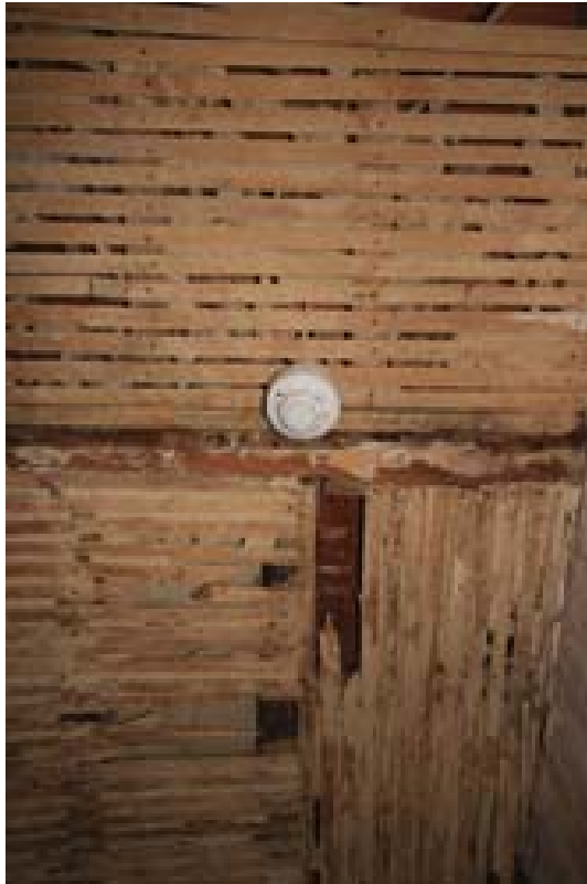
Plate 64: Lath-and-plaster ceiling at the west end of the corridor (Room 9). (#138)
