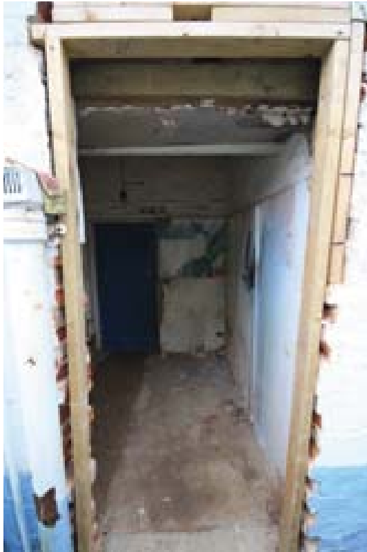
Plate 136: Cross passage, Block D. (#418)
