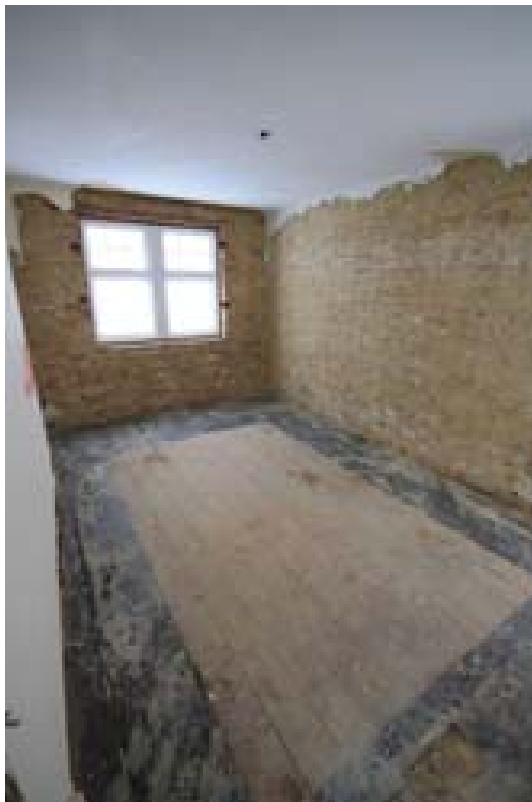
Plate 105: Overview of Room 20. (#304)
