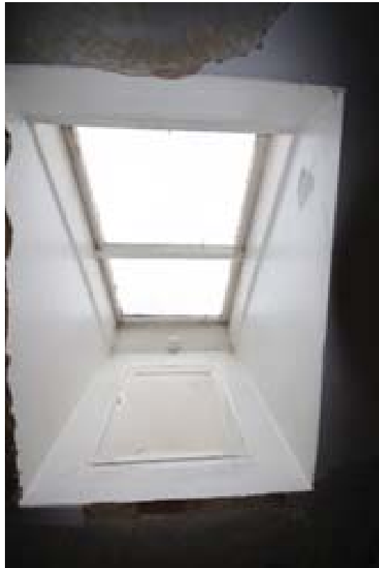
Plate 75: Skylight above Room 10. (#316)
