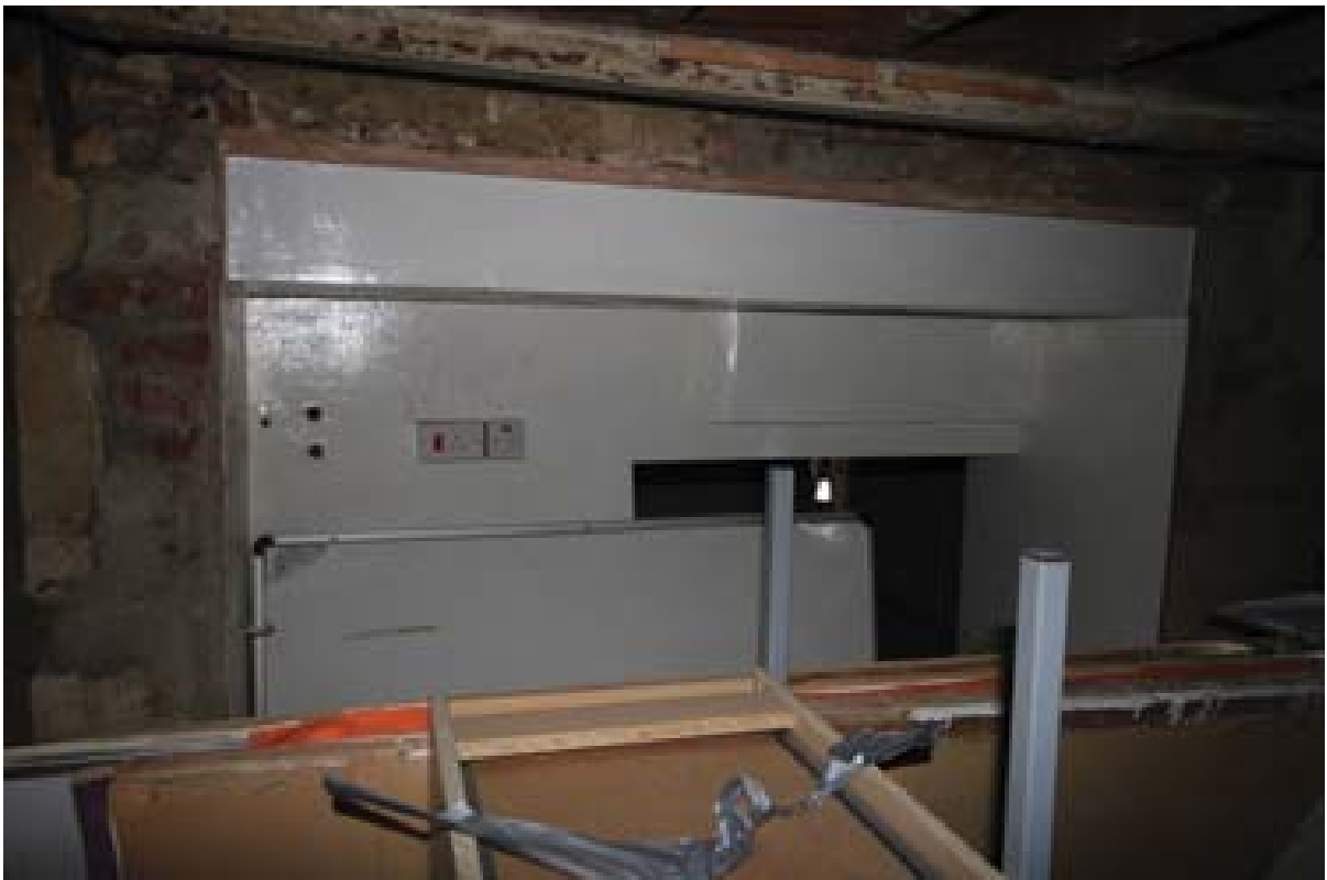
Plate 55: Altered fireplace, Room 7. (#167)
