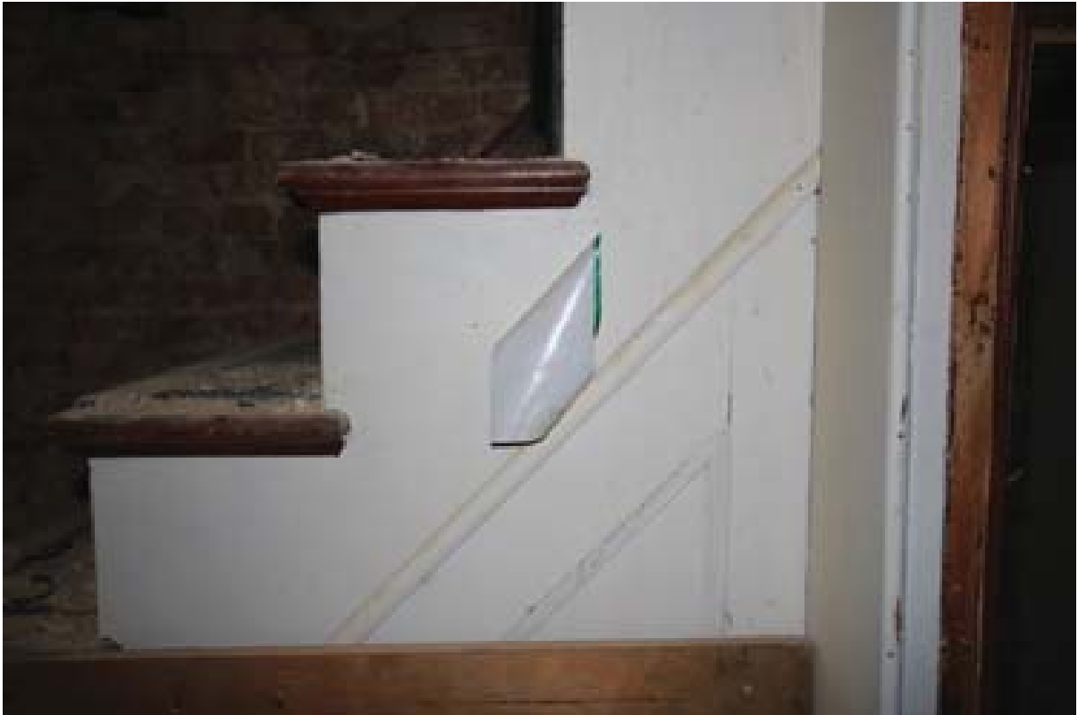
Plate 30: Stair trim and beaded spandrel, Room 2. (#120)
