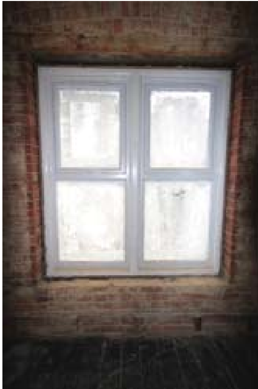
Plate 108: Window in the south wall of Room 21. (#272)
