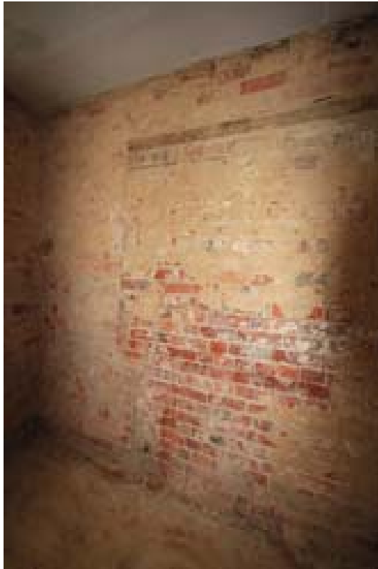
Plate 92: Change in wall construction and height, Room 15. (#255)
