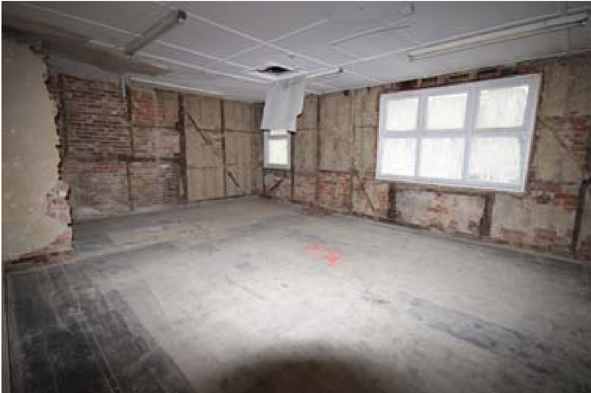
Plate 96: Overview of Room 17. (#228)
