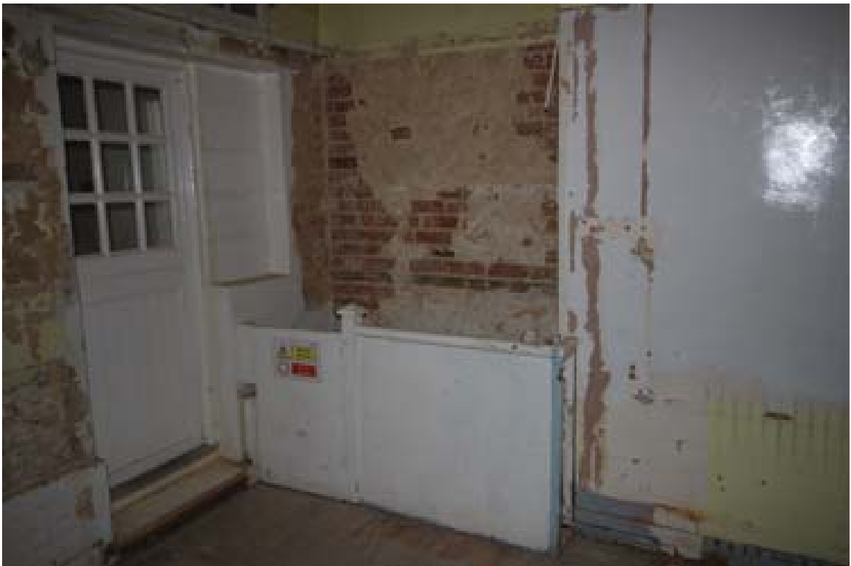
Plate 51: Bond timbers in west wall of Room 6. (#147)
