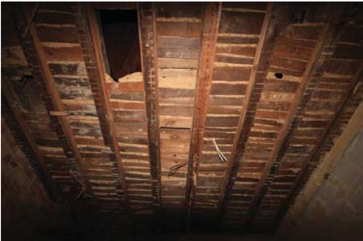
Plate 35: Ceiling construction, Room 3. (#119)
