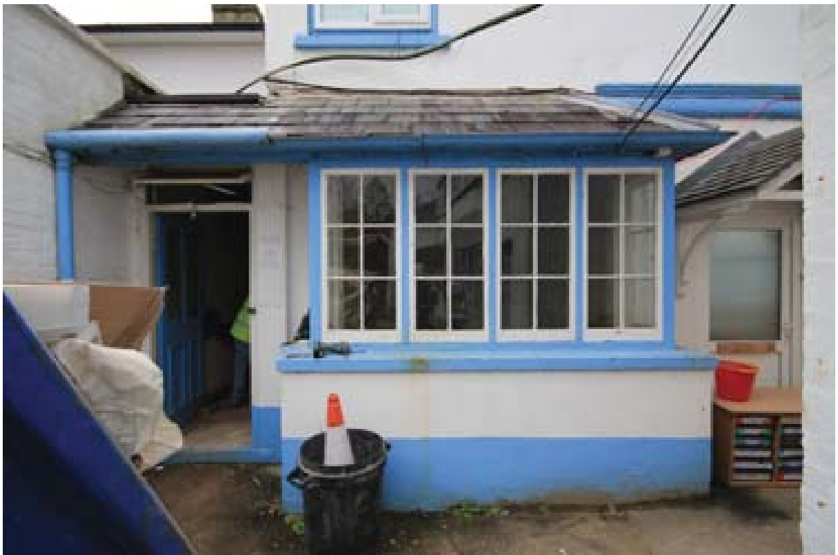
Plate 15: Bay window in east elevation of the core building. (#3)
