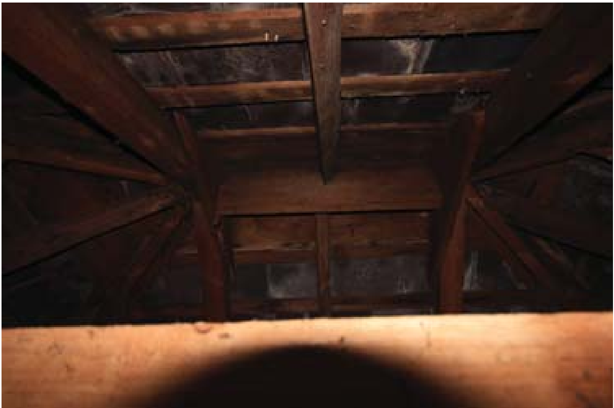
Plate 127: Roof space, Block C. (#368)
