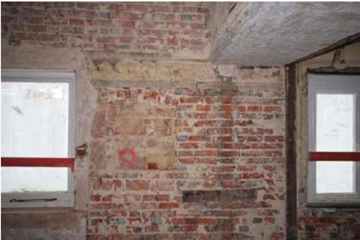
Plate 89: Blocked window opening and bond timbers, Room 14. (#289)
