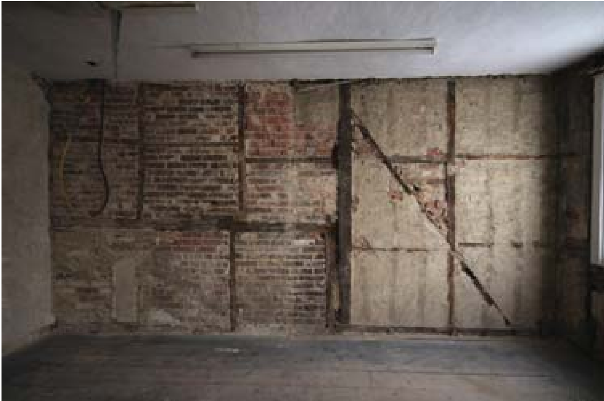
Plate 98: Intersection of construction phases in the east wall of Room 17. (#232)
