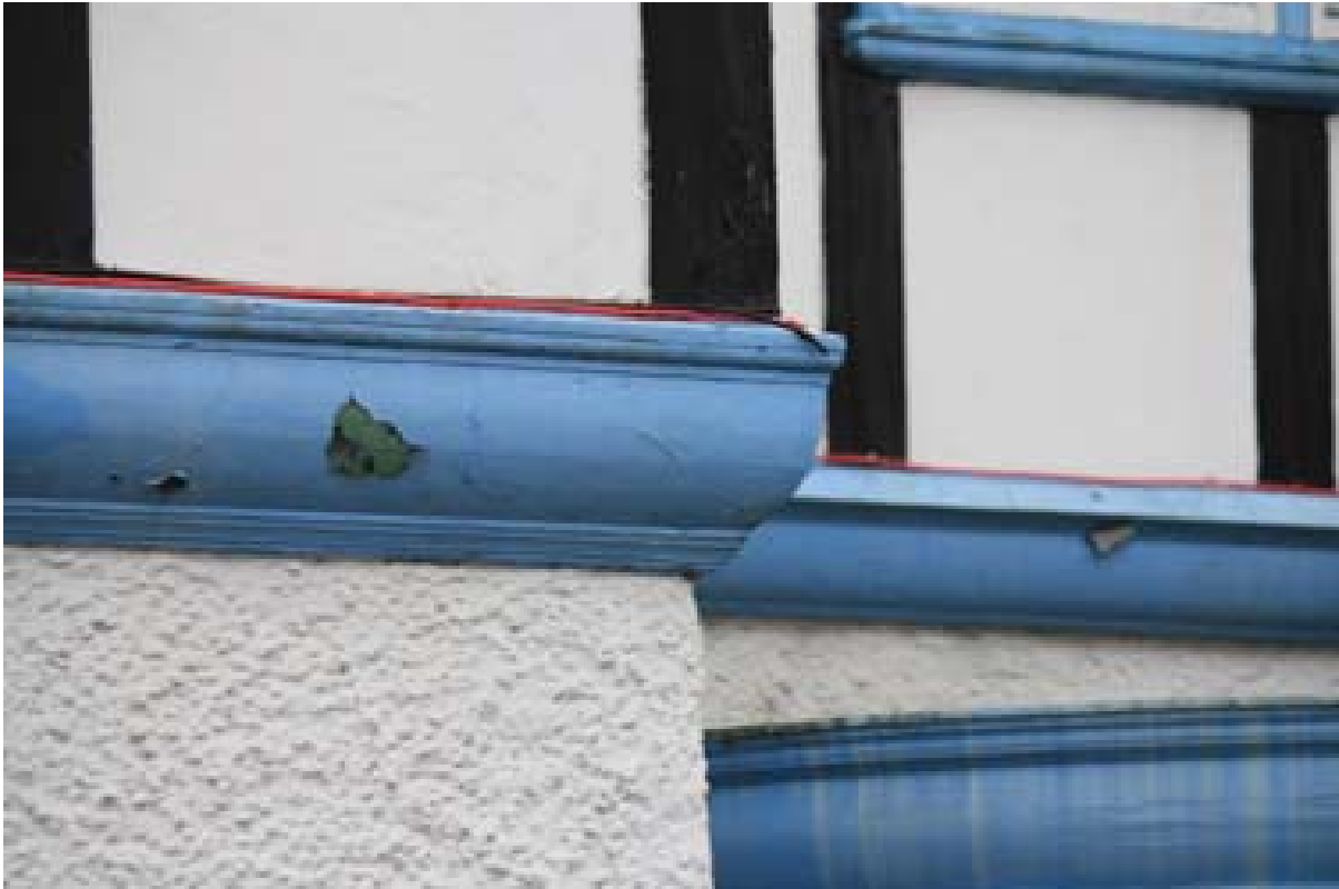
Plate 6: Moulded cornice on north elevation of Block A. (#61)
