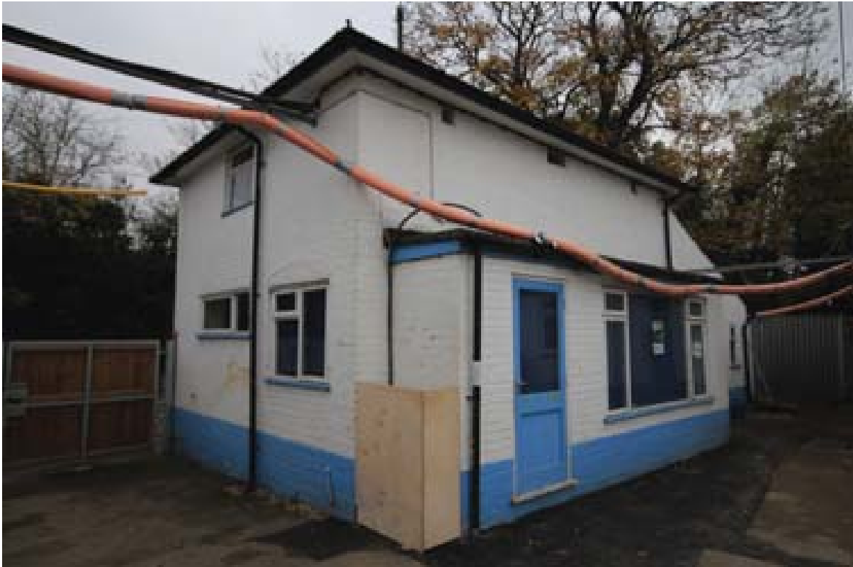
Plate 138: Principal (west) and north elevations of Block E. (#420)
