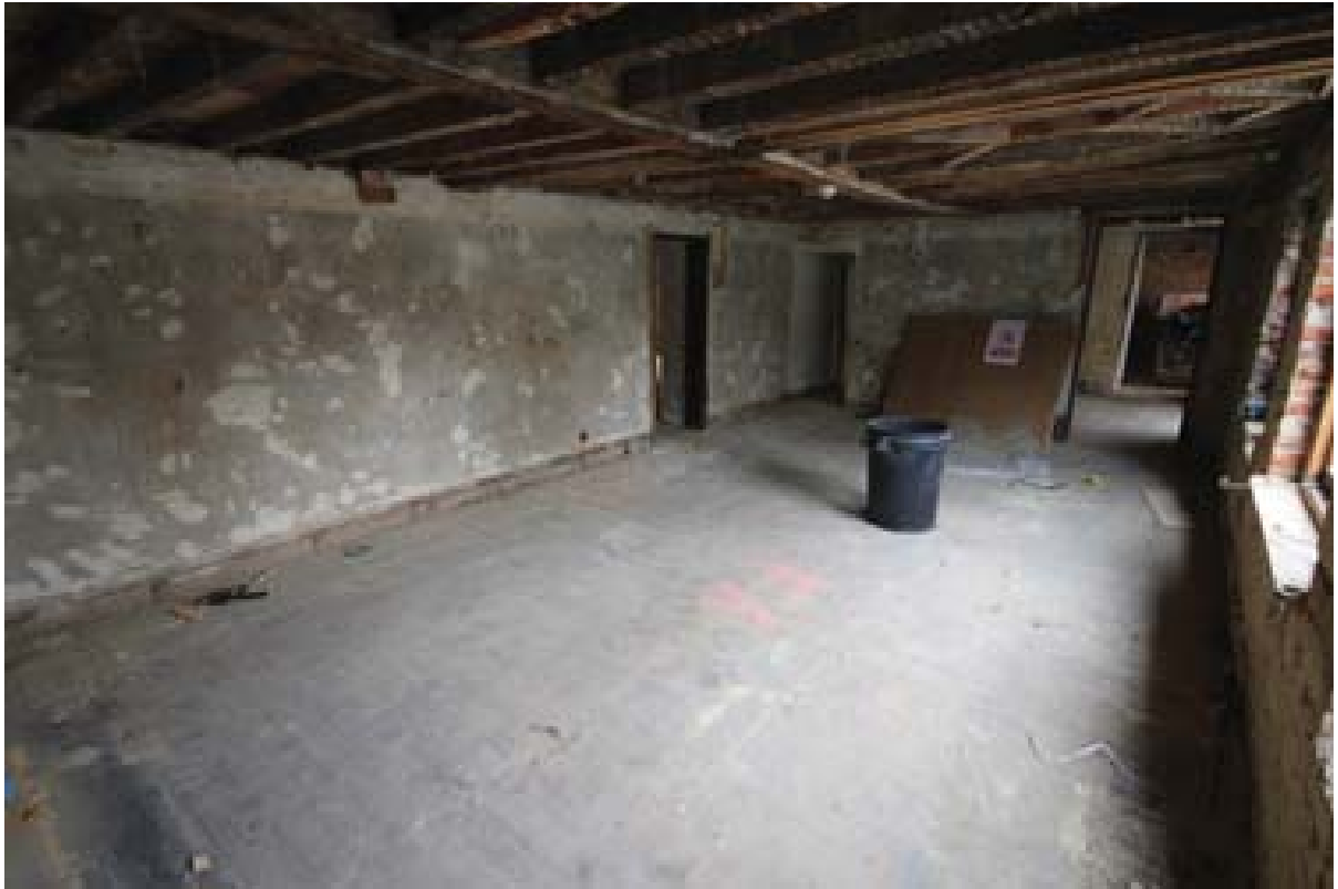
Plate 20: Overview of Room 1. (#65)
