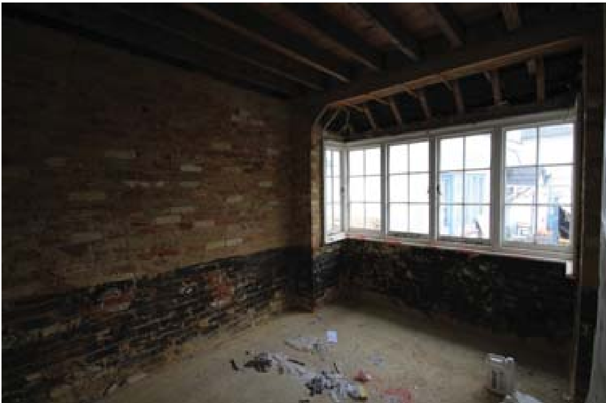
Plate 77: Overview of Room 12. (#195)
