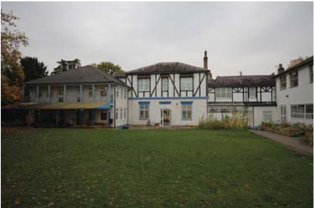
Plate 9: South elevation of Block A, with the Old Hall to the centre. (#35)
