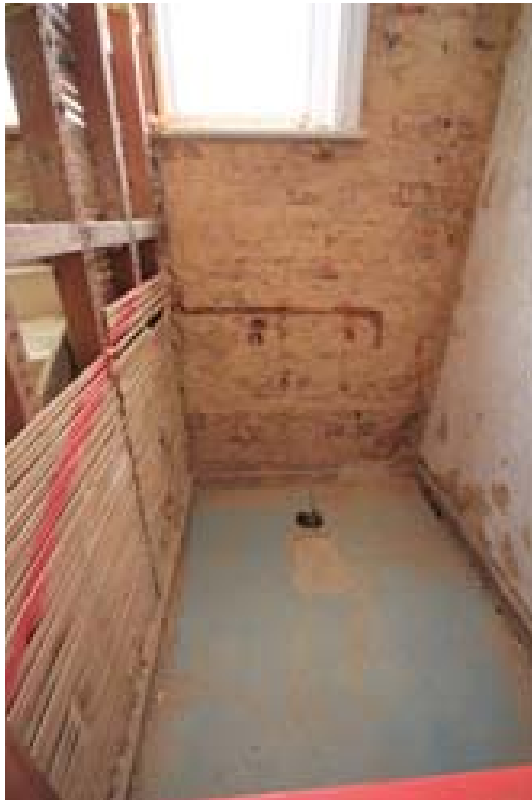
Plate 92: Change in wall construction and height, Room 15. (#255)
