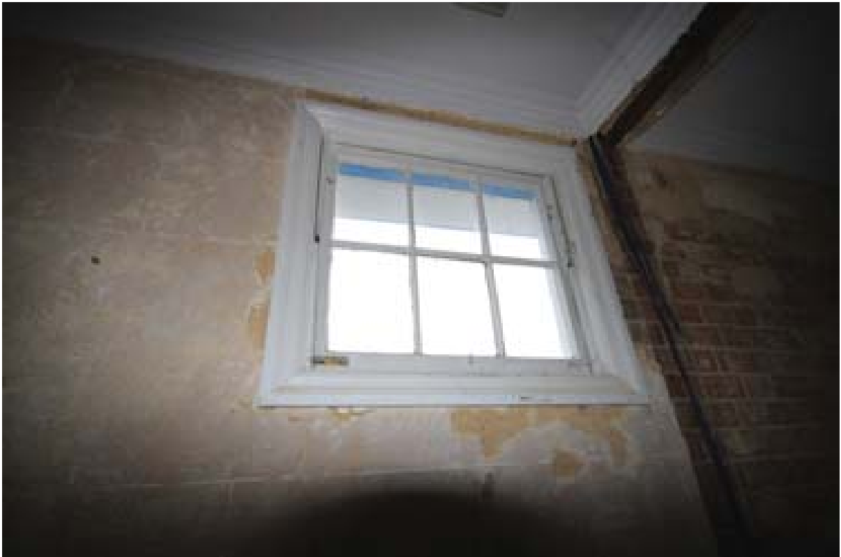
Plate 109: Small window in east wall of Room 21. (#268)
