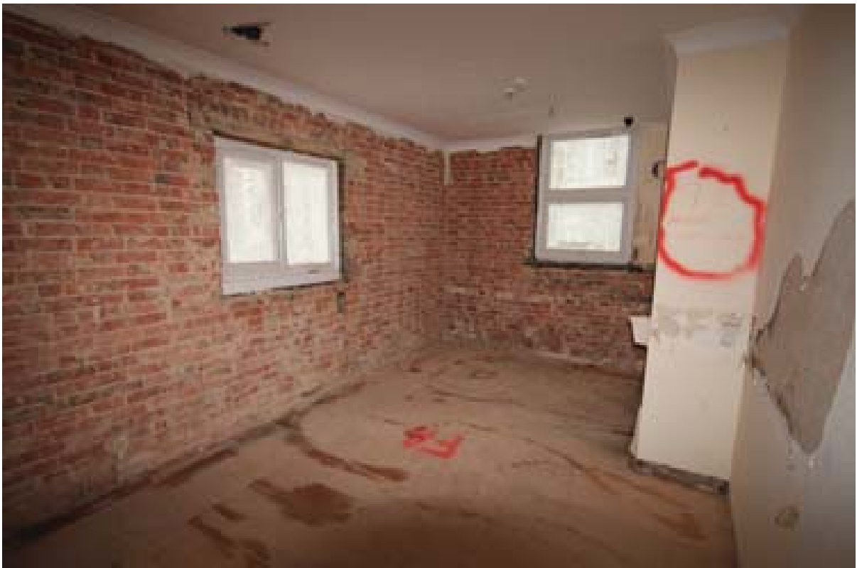
Plate 103: Overview of Room 19. (#295)
