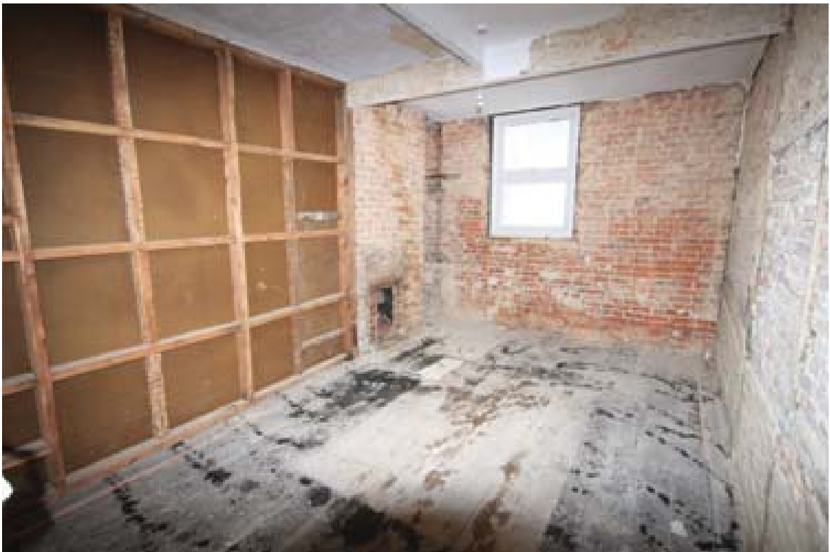
Plate 101: Overview of Room 18. (#291)
