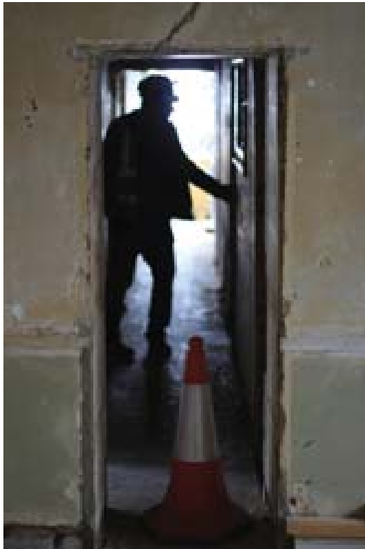
Plate 43: Small door to servants' corridor, Room 5. (#134)
