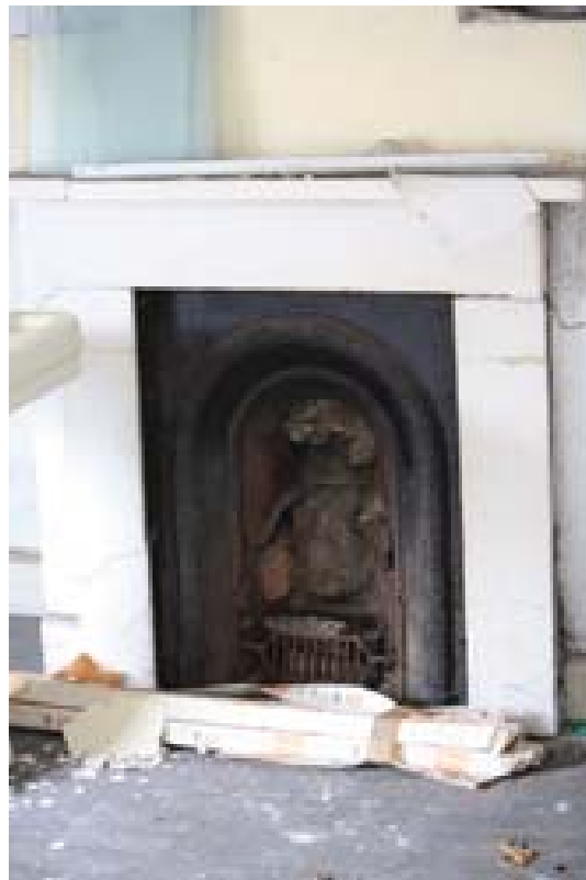
Plate 135: Fireplace in the first floor room, Block D. (#408)
