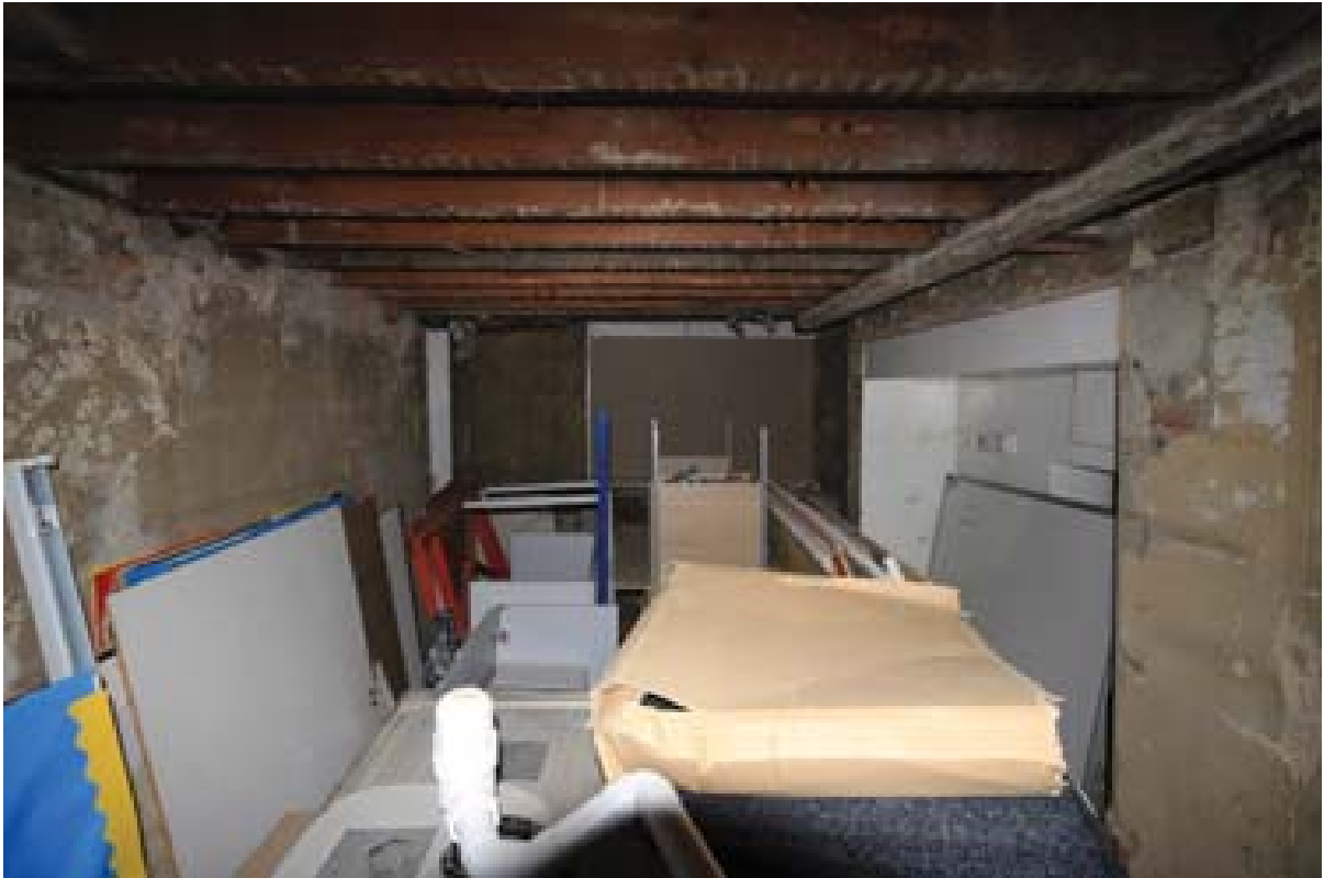
Plate 54: Overview of Room 7. (#161)
