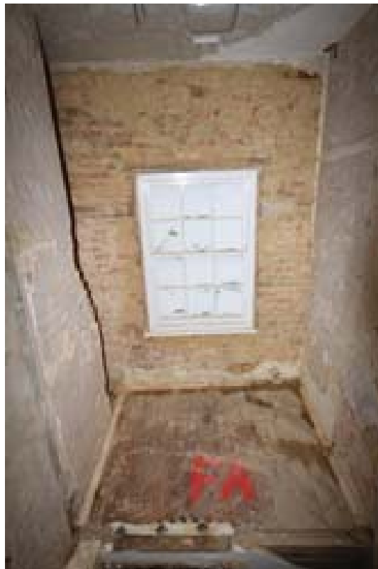
Plate 73: Overview of the former bathroom. Note the bond timbers and sash window in the north wall, Room 10. (#318)
