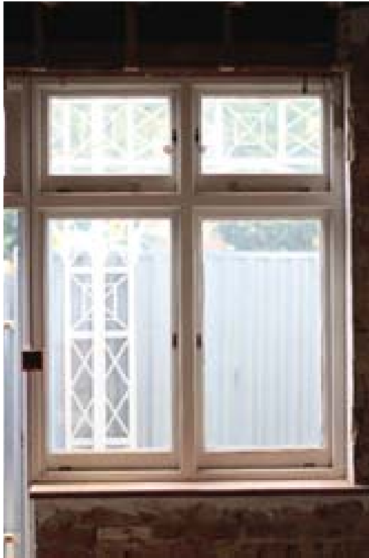
Plate 42: Window detail, Room 5. (#133)
