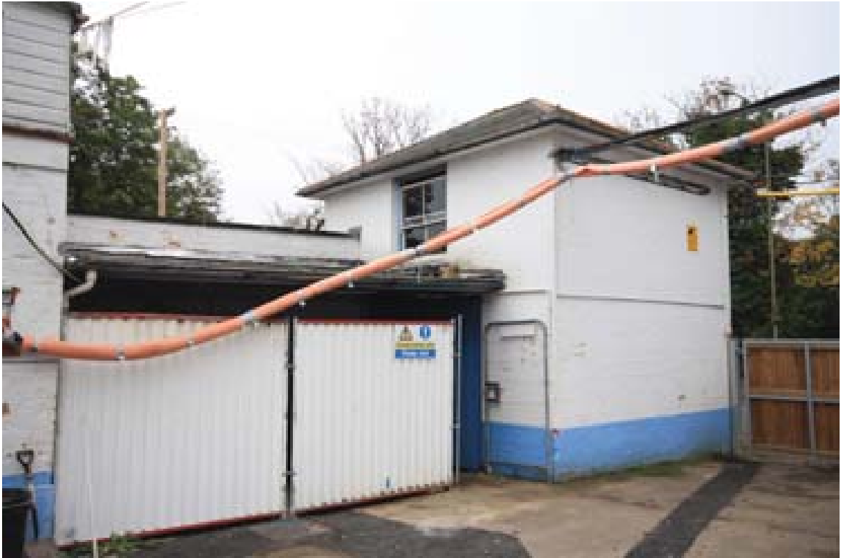
Plate 128: Principal (south) and west elevations of Block D. (#393)
