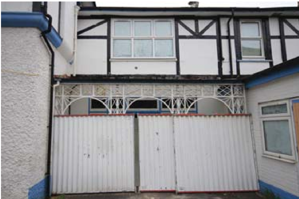
Plate 13: Remnant veranda on south elevation of the core building. (#28)
