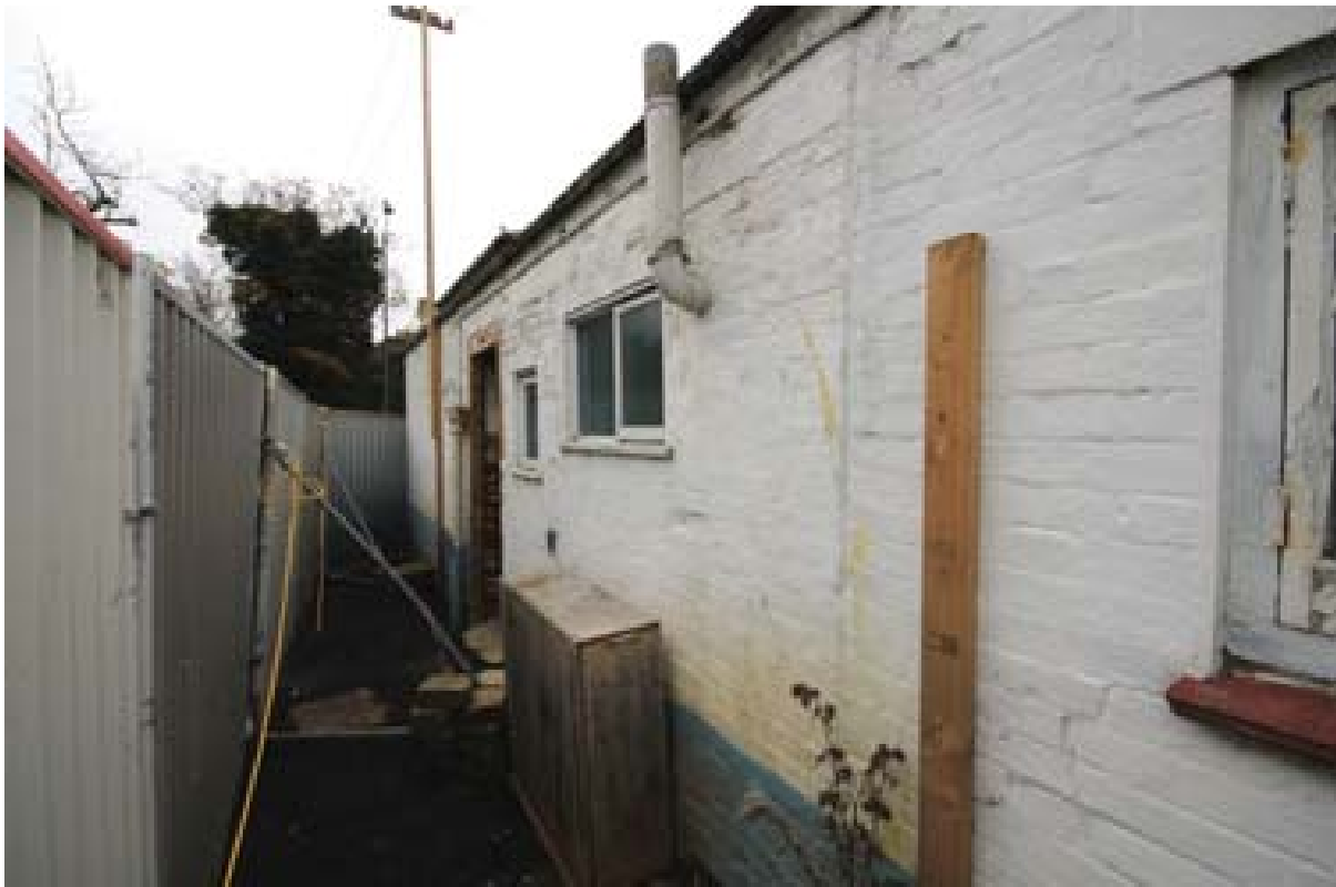
Plate 131: North elevation of Block D. (#384)
