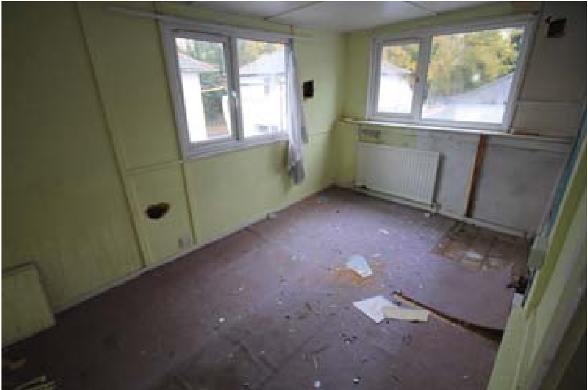
Plate 126: First floor extension, Block C. (#366)
