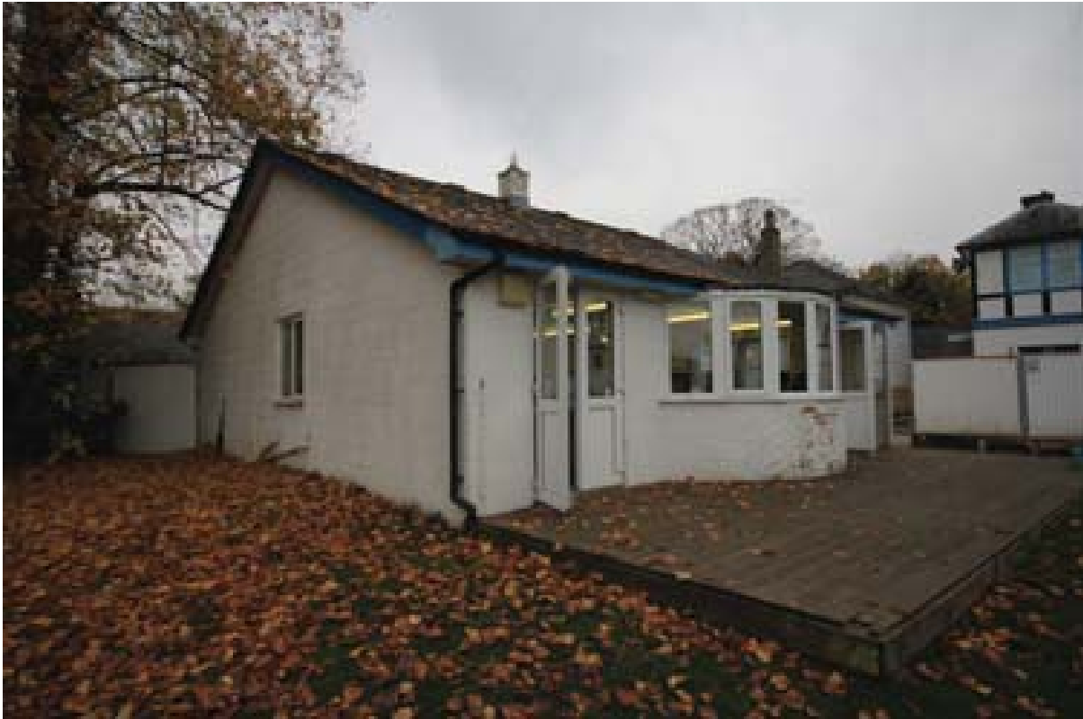
Plate 116: Principal (west) and north elevations of Block B. (#329)
