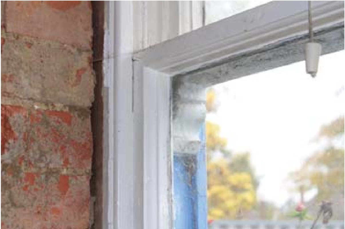
Plate 38: Horned sash window detail, Room 4. (#108)
