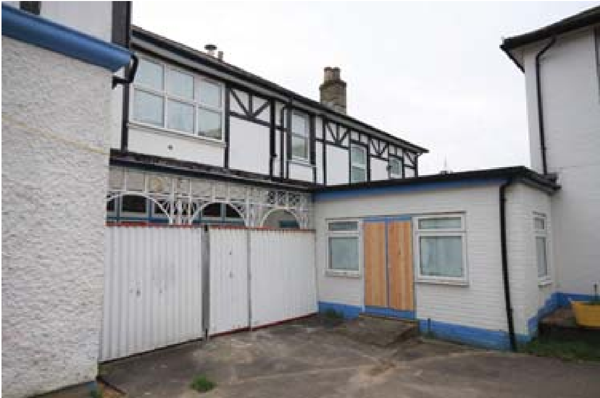
Plate 10: South elevation of the core building. (#29)
