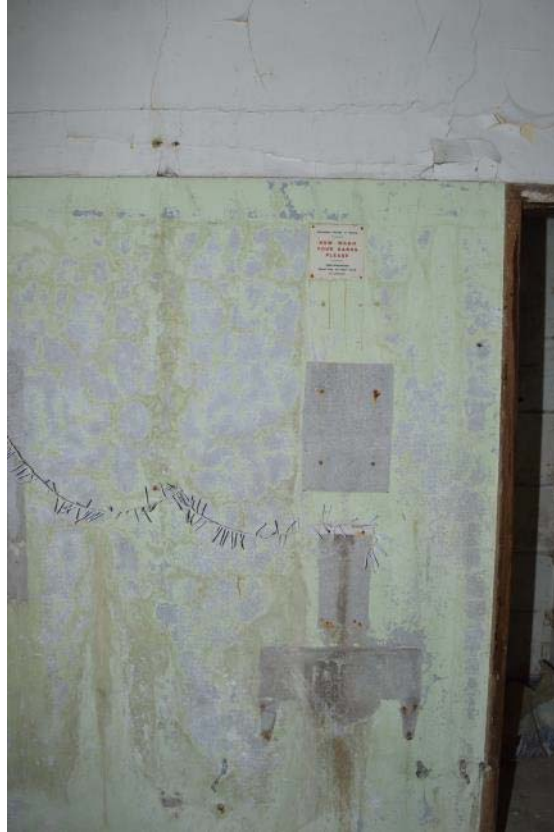
Plate 19: Room 5, looking west (53)
