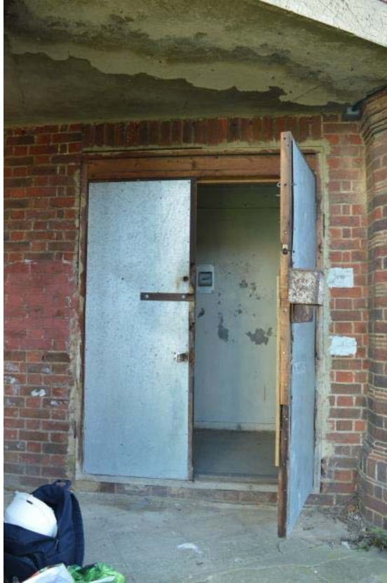
Plate 3: Inserted entrance to Room 1, looking east (16)
