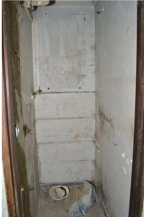
Plate 21: Room 7, looking west (54)
