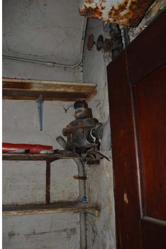
Plate 13: Room 3, looking west (31)
