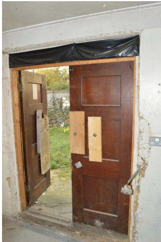
Plate 10: Room 1, looking west (21)
