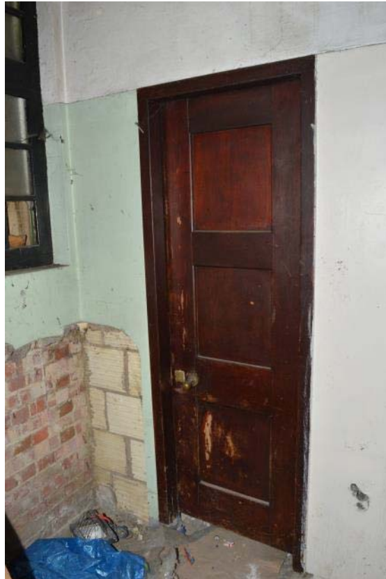
Plate 14: Room 2, looking west (30)
