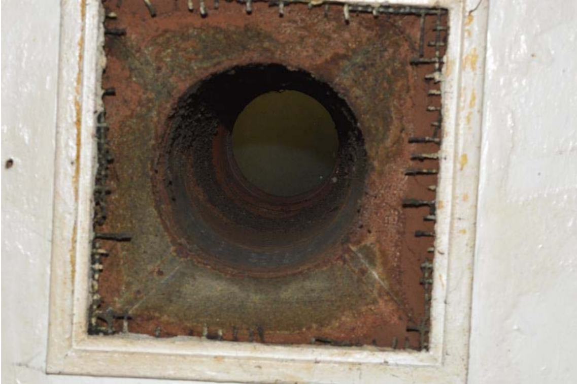
Plate 17: Room 4 looking up (40)
