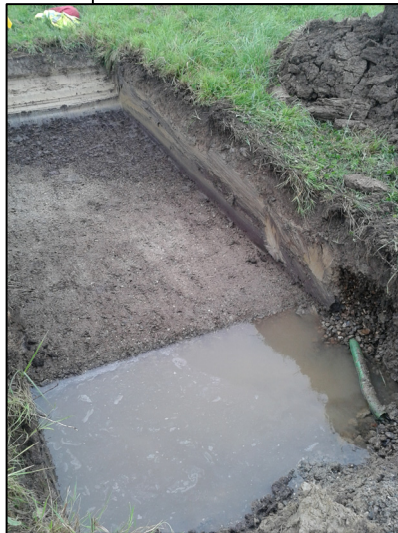
Trench 11, part during machine excavations, view south-west
