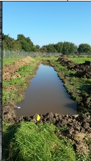
Trench 14, before pumping, view north
