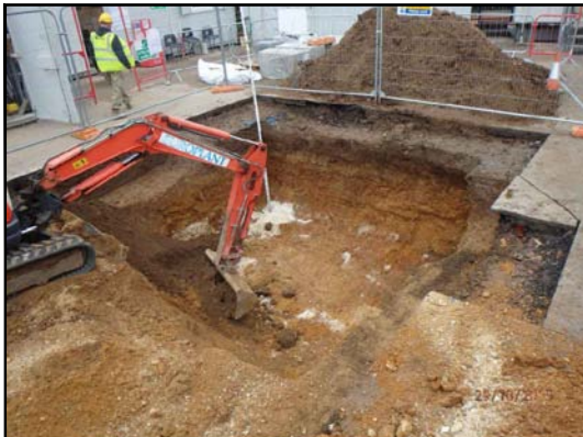
Area under excavation
