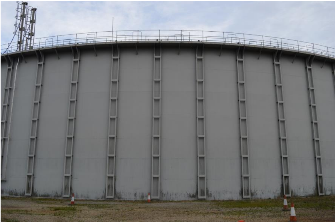
Plate 51: Gasholder No. 7, view of the tank construction, facing north-east (ARG15-0012)
