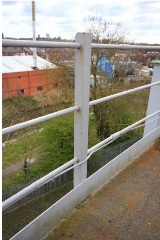
Plate 22: Gasholder No. 5, view handrail arrangement (ARG15-0164)
