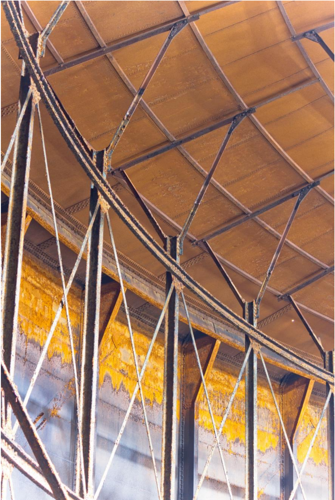
Plate 5: Gas holder No. 5, crown supports and framework (ARG15-0285)
