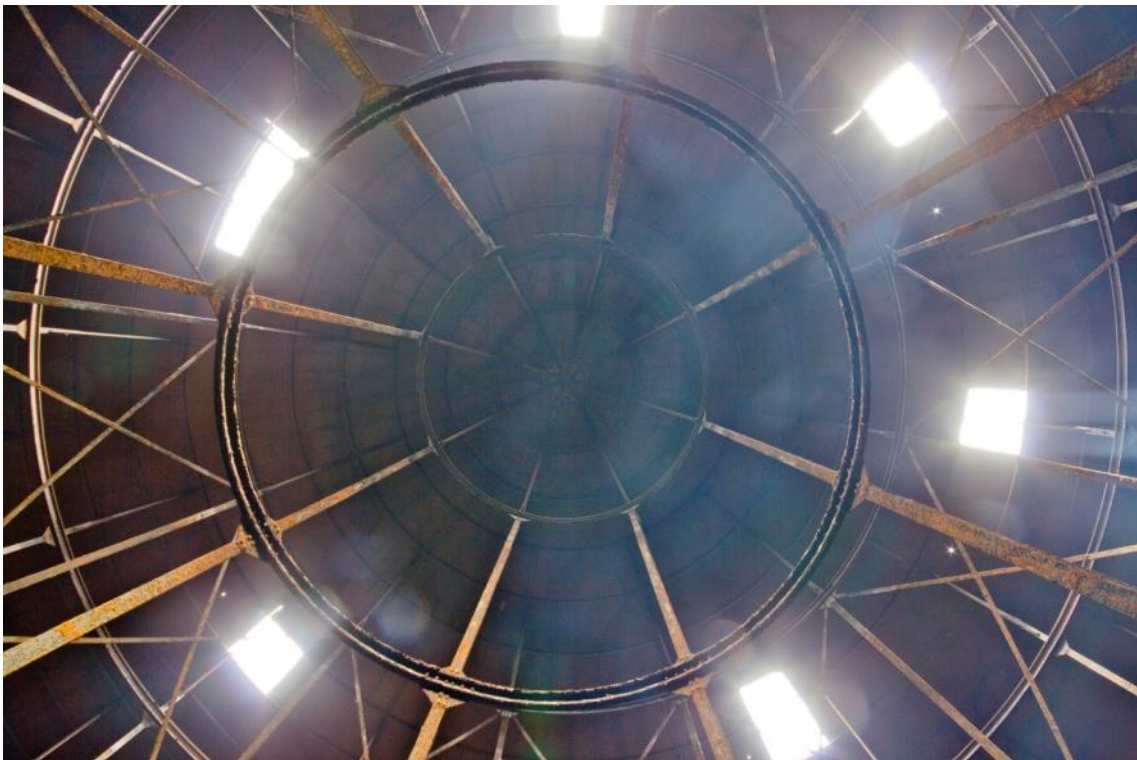
Plate 10: Gasholder No. 5, the apex of the crown and framework (ARG15-0265)
