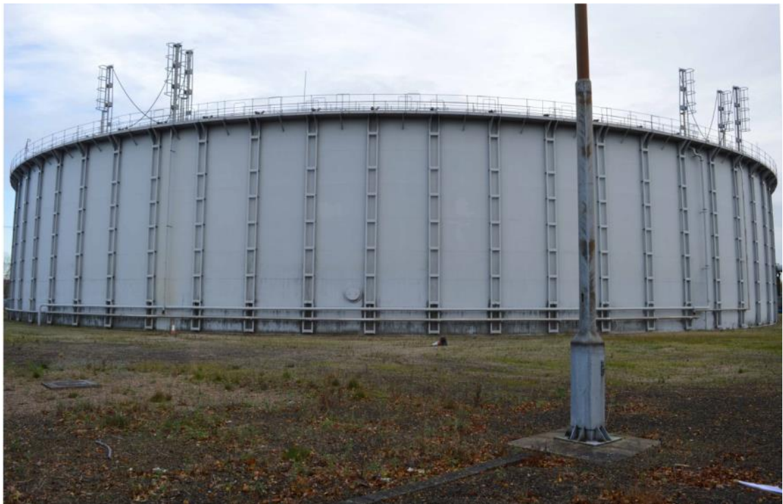
Plate 42: Gasholder No. 7, view of tank construction, facing north-east (ARG15-0014)
