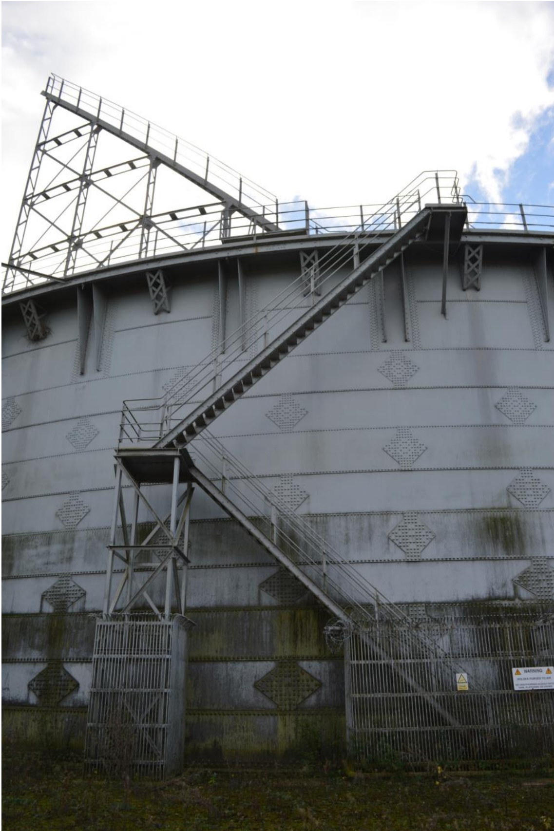
Plate 38: Gasholder No. 5, view of tank access stair, facing south (ARG15-0124)
