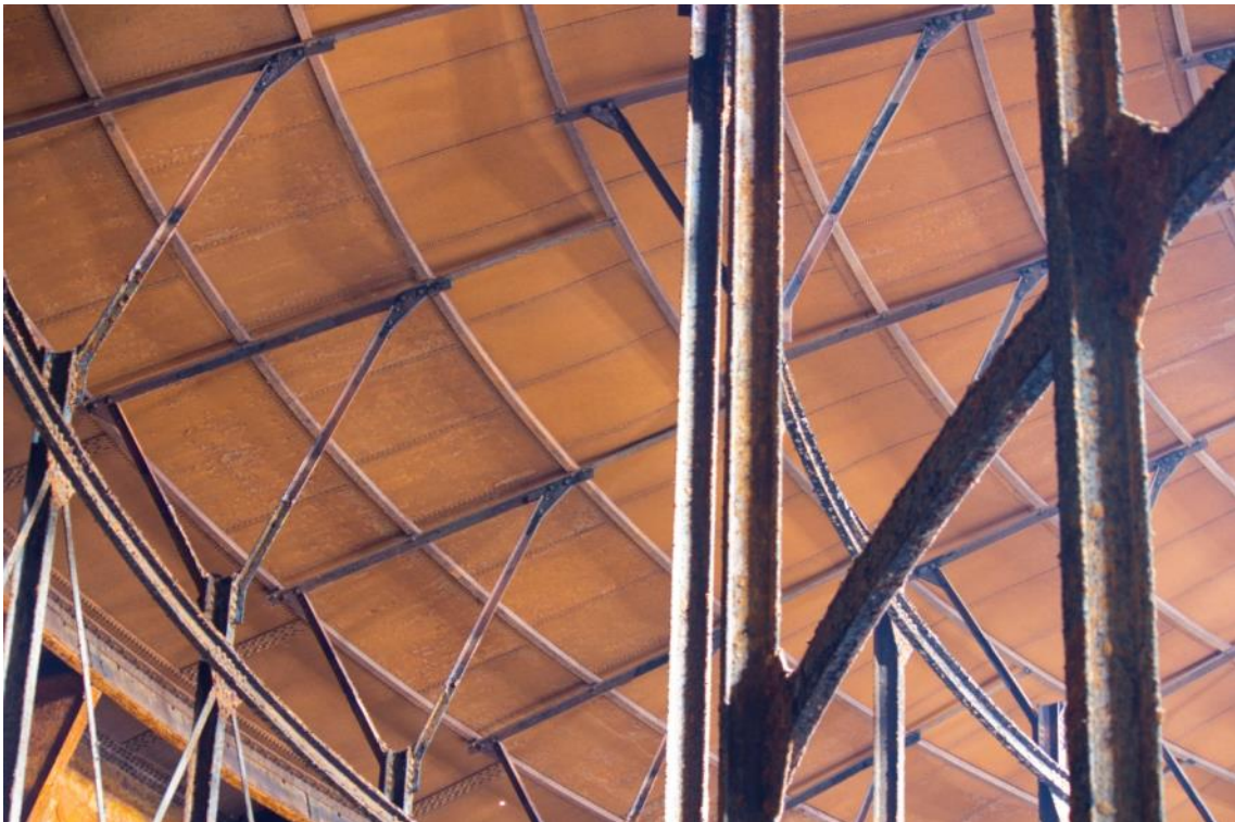
Plate 4: Gasholder No. 5, Interior of the crown (ARG15-0284)
