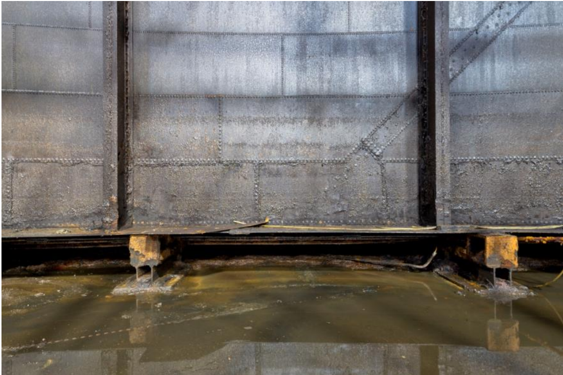
Plate 15: Gasholder No. 5, lift walls resting atop steel chocks (ARG15-0256)
