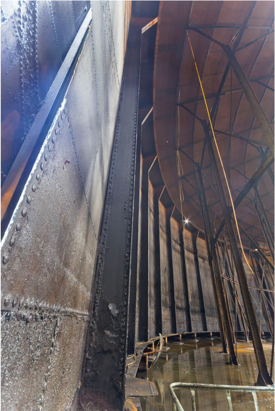
Plate 14: Gasholder No. 5, walls of the first lift (ARG15-0249)
