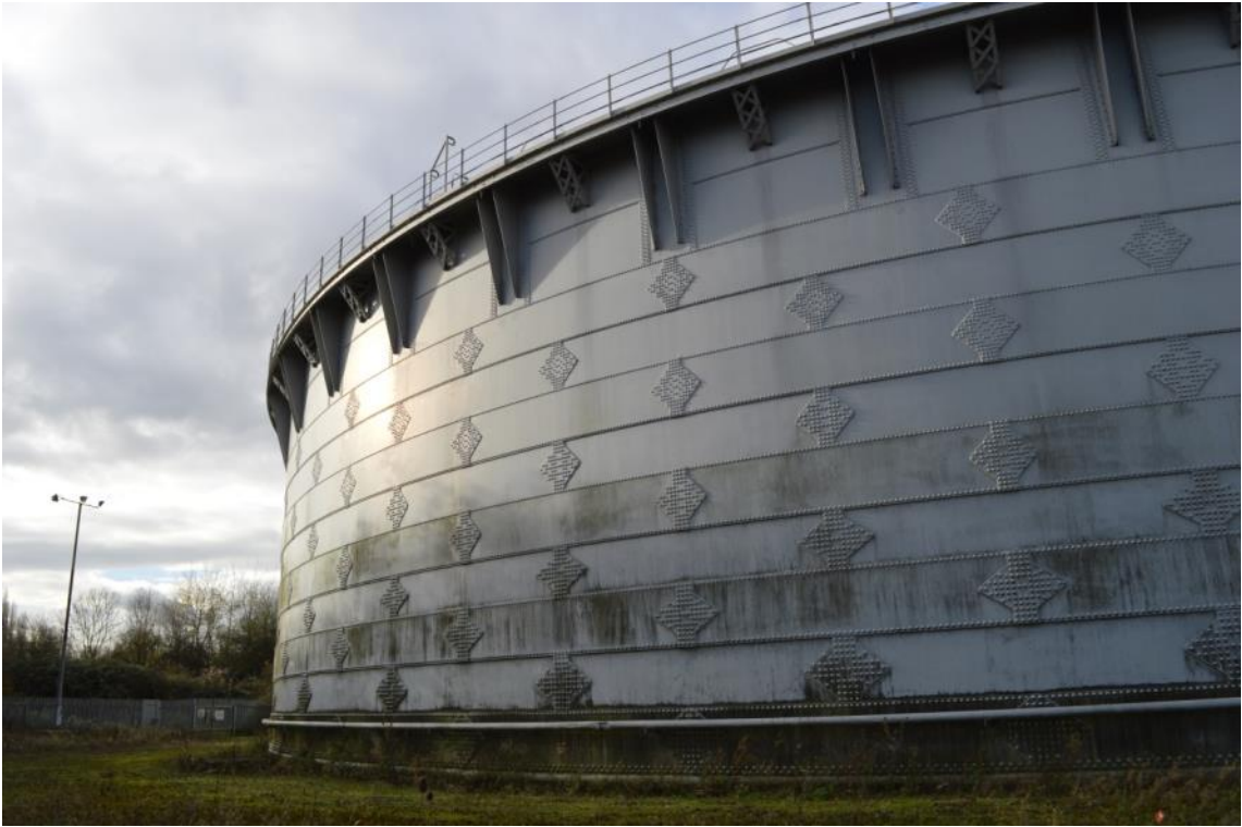
Plate 25: Gasholder No. 5, general view of tank construction, facing south-west (ARG15-0086)
