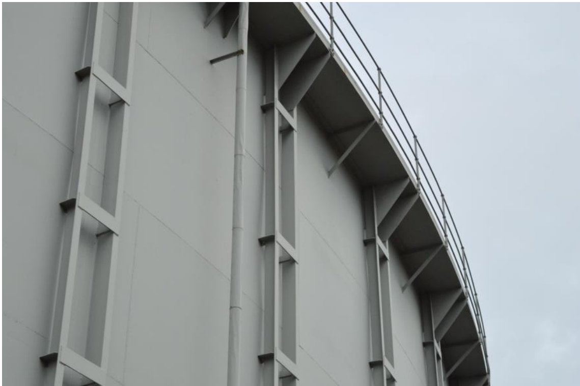
Plate 53: Gasholder No. 7, detail of tank platform support brackets, facing north-west (ARG15-0005)
