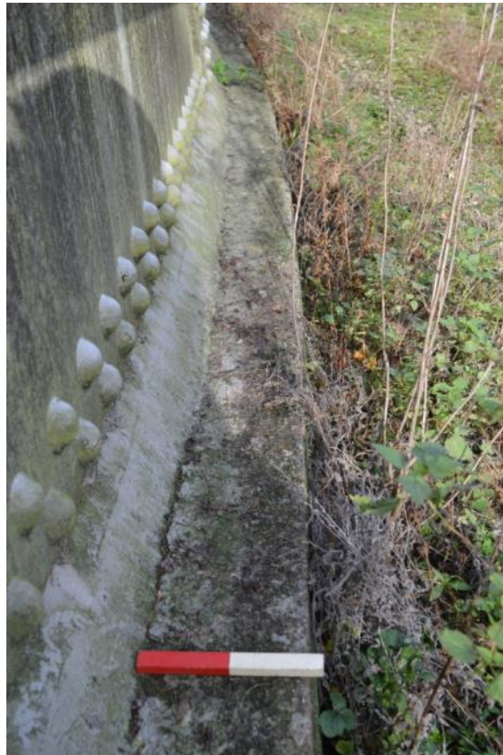
Plate 30: Gasholder No. 5, concrete tank base, facing north-east (ARG15-0087)
