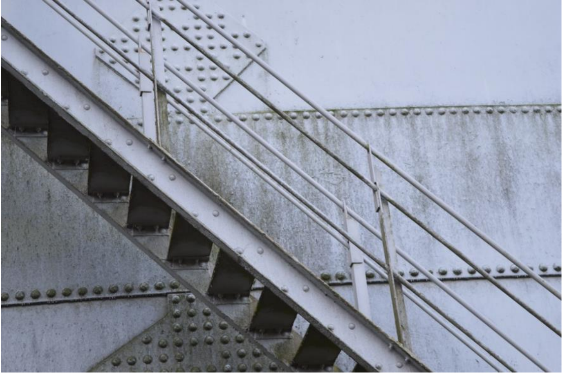
Plate 39: Gasholder No. 5, detail of tank access stair construction, facing south (ARG15-0127)
