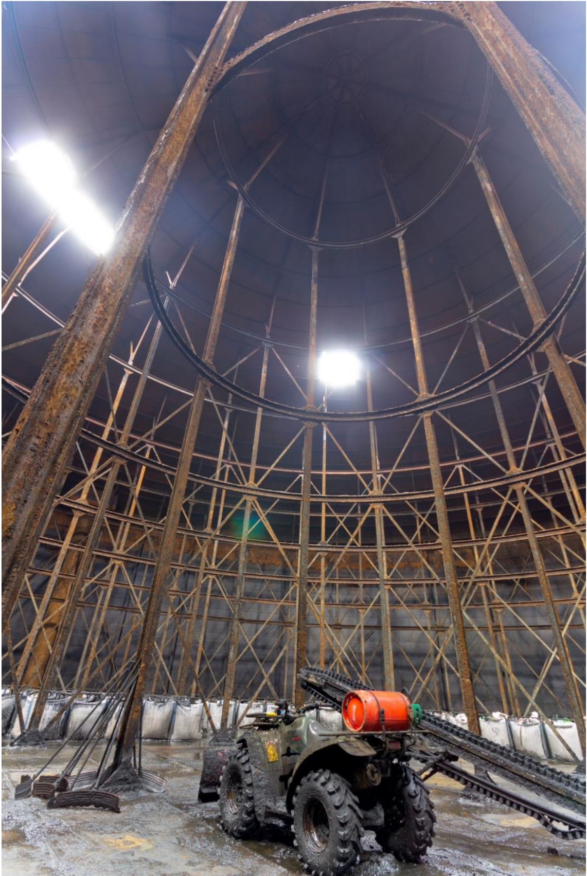
Plate 6: Gasholder No. 5, Interior framework (ARG15-0269)
