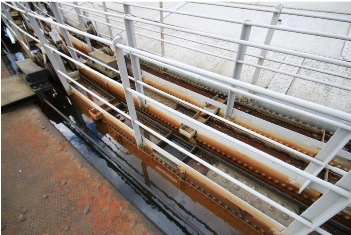
Plate 12: Gasholder No. 5, Interior of the crown (ARG15-0170)
