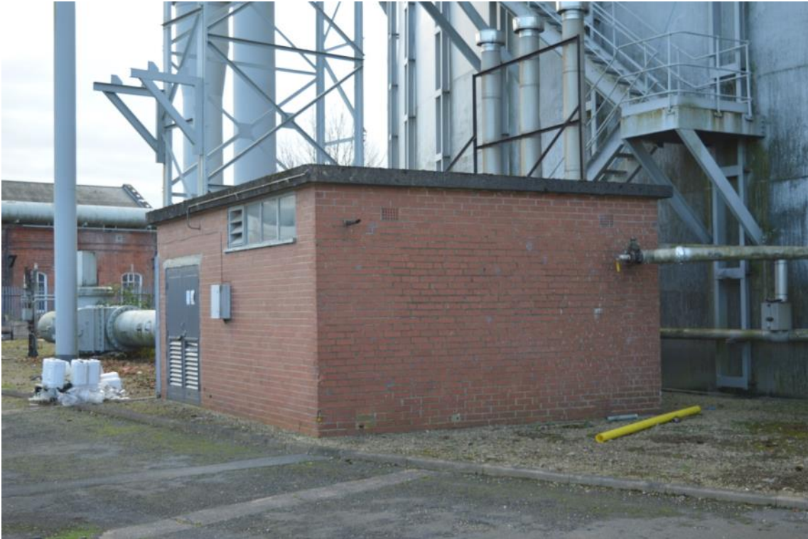
Plate 60: View of the Boiler House within the northern compound, facing south-east (ARG15-0035)
