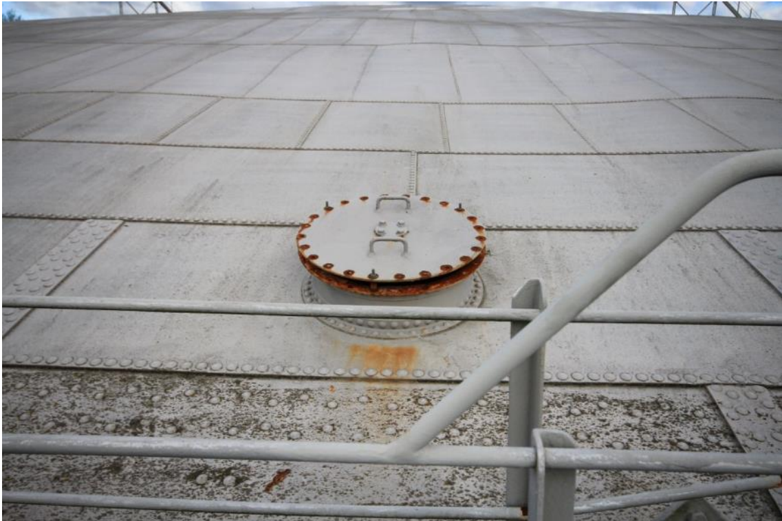
Plate 3: Gasholder No. 5, representative hatch access (ARG15-0182)
