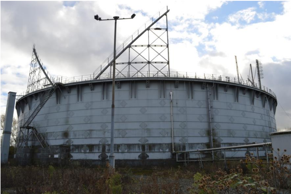
Plate 1: General view of Gasholder No. 5, facing south-east (ARG15-0121)
