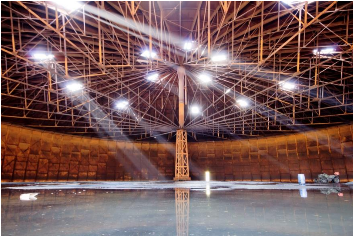
Plate 44: Gasholder No. 7, interior of the bell (ARG15-0213)
