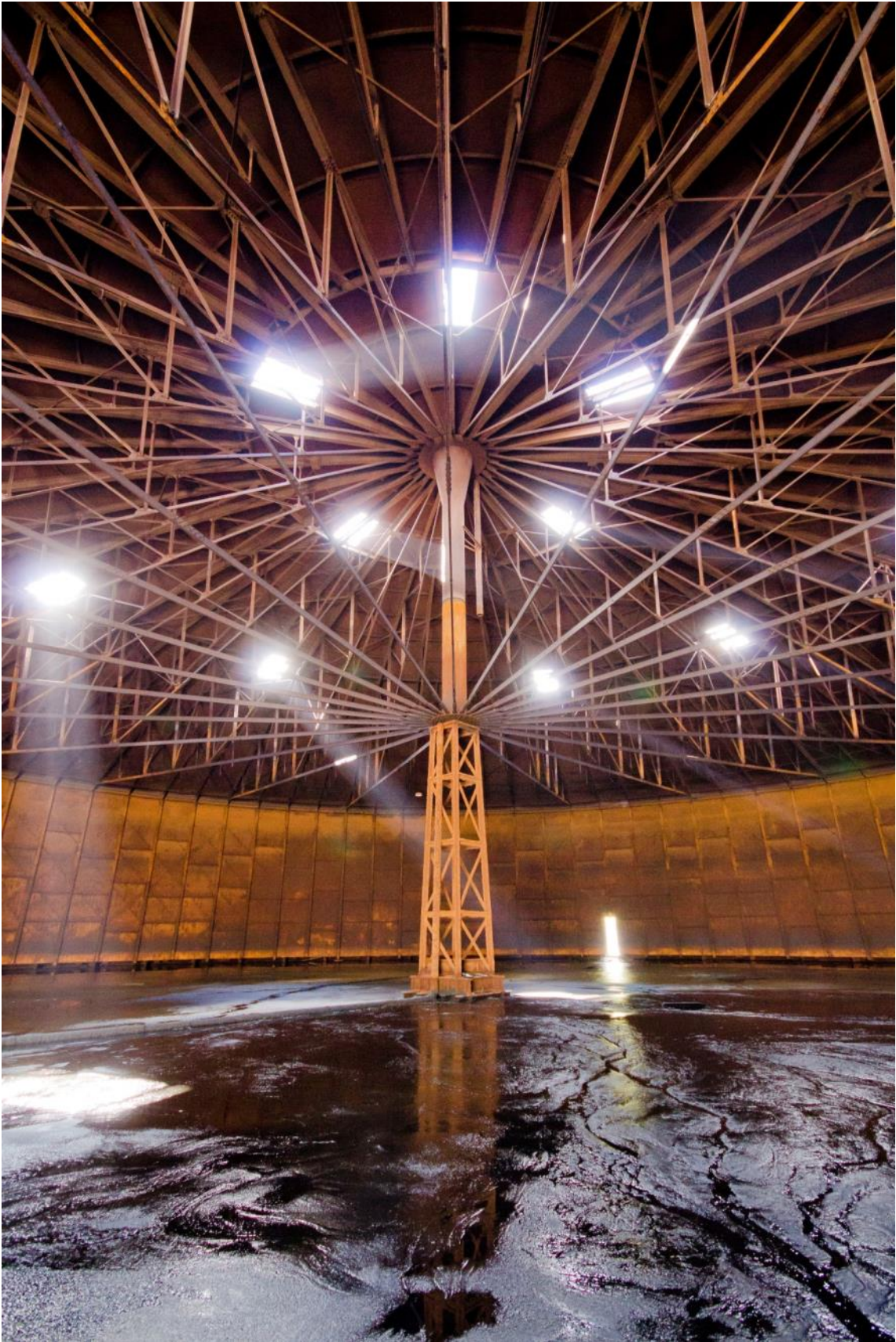
Plate 45: Gasholder No. 7, interior of the bell, plinth and crown stanchion (ARG15-0220)
