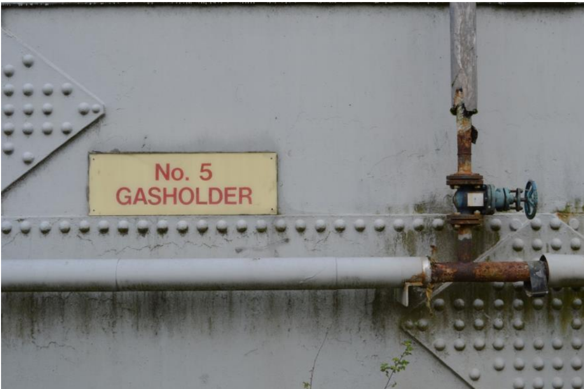
Plate 32: Gasholder No. 5, modern 'No. 5 Gasholder' identification signage, facing north (ARG15-0099)
