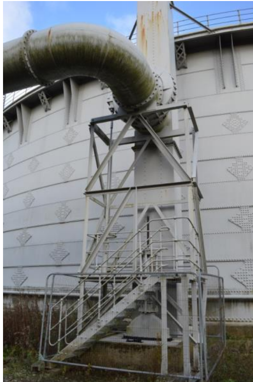
Plate 36: Gasholder No. 5, detail of the stair serving the southern gas inlet/outlet syphon, facing north-west (ARG15-0101)
