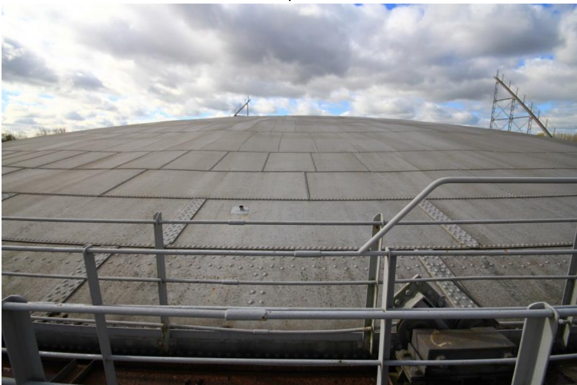
Plate 2: Gasholder No. 5, view of the crown (ARG15-0158)
