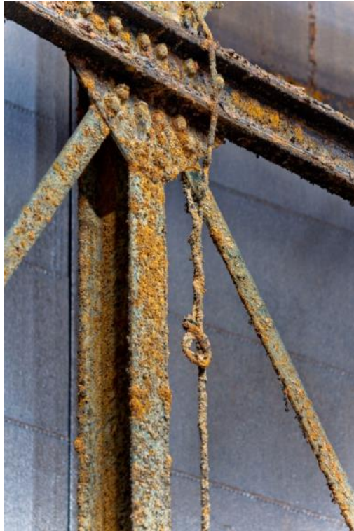
Plate 11: Gasholder No. 5, remnant rope on framework (ARG15-0288)
