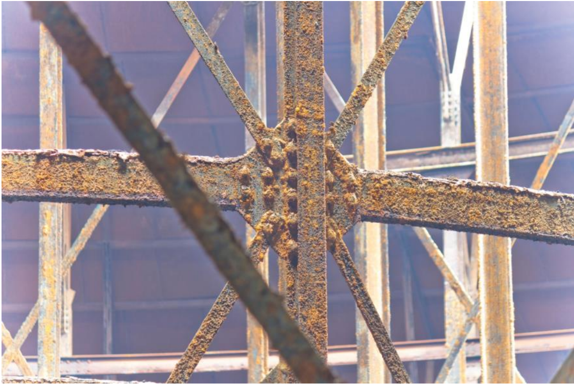
Plate 9: Gasholder No. 5, interior framework detail (ARG15-0283)
