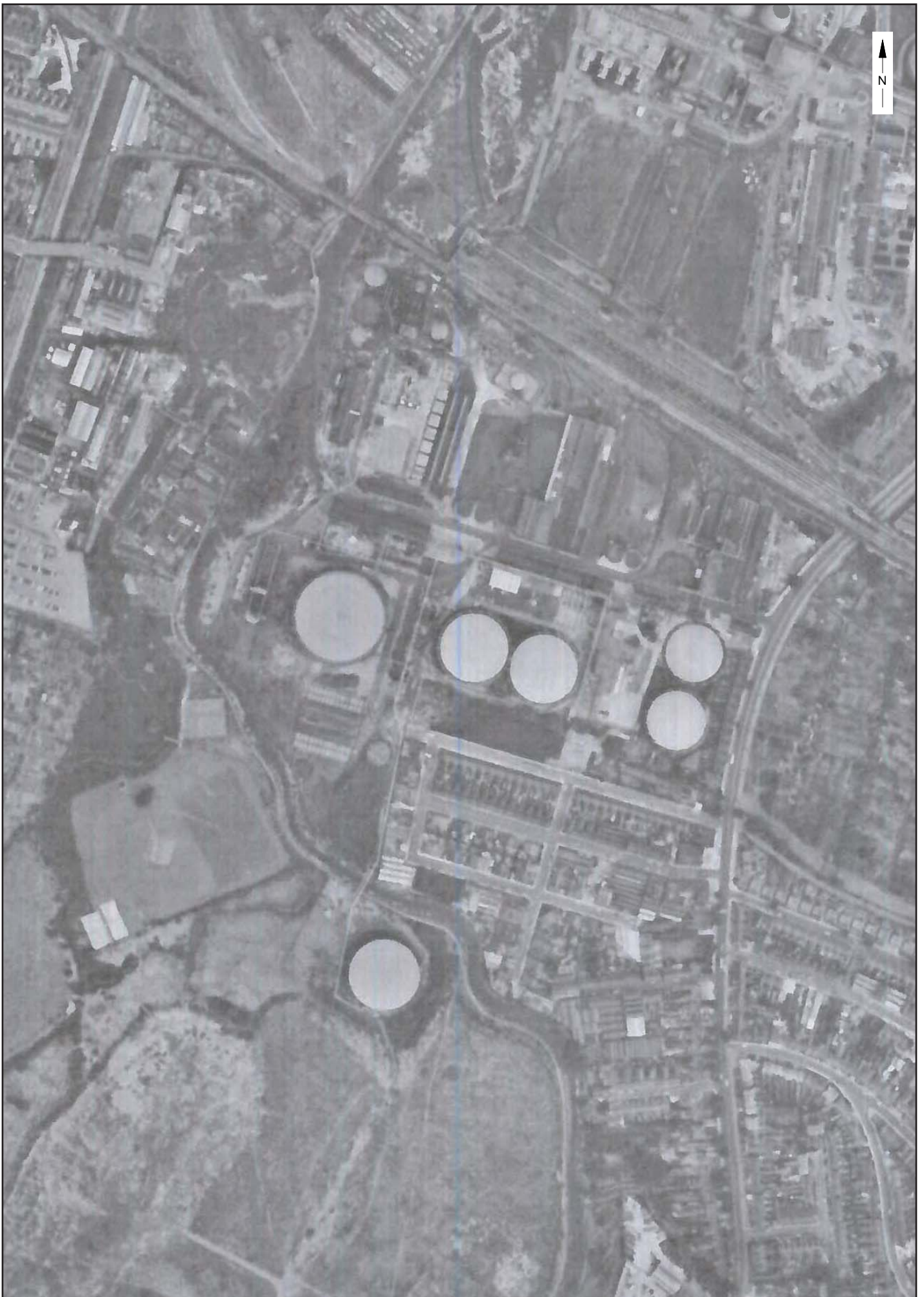
© Archaeology South-East Former Gasworks at Aylestone Road, Leicester Fig. 16 Project Ref: 7912 January 2016 Aerial view of Aylestone Road Gasworks, Leicester (07 AUG 1967) (HE) Report Ref: 2015449 Drawn by: HG
