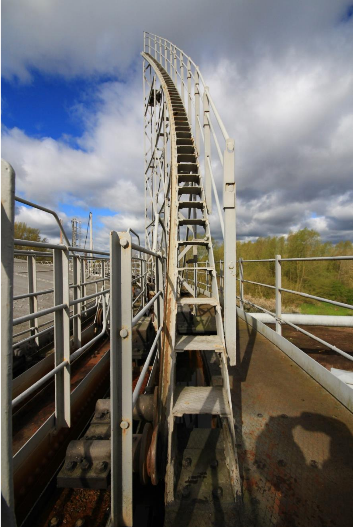
Plate 24: Gasholder No. 5, lift stair (ARG15-0160)
