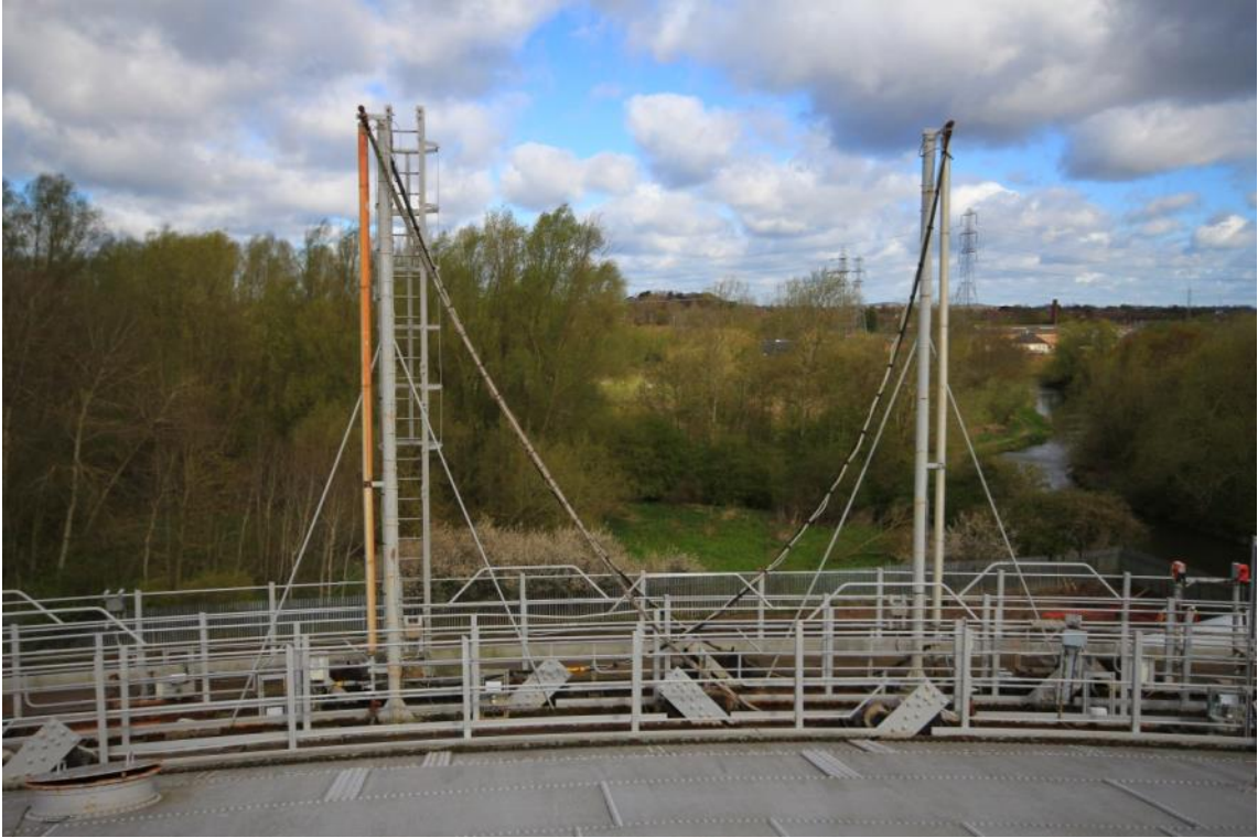
Plate 17: Gasholder No. 5, hose guides(ARG15-0196)
