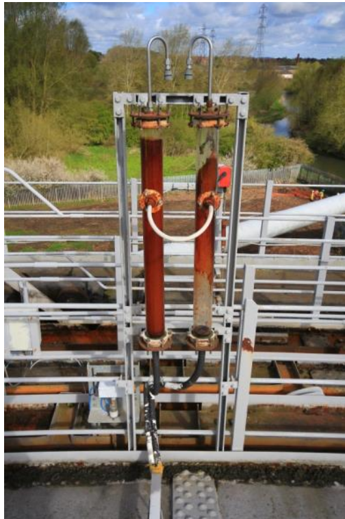
Plate 18: Gasholder No. 5, oil monitoring apparatus (ARG15-0202)
