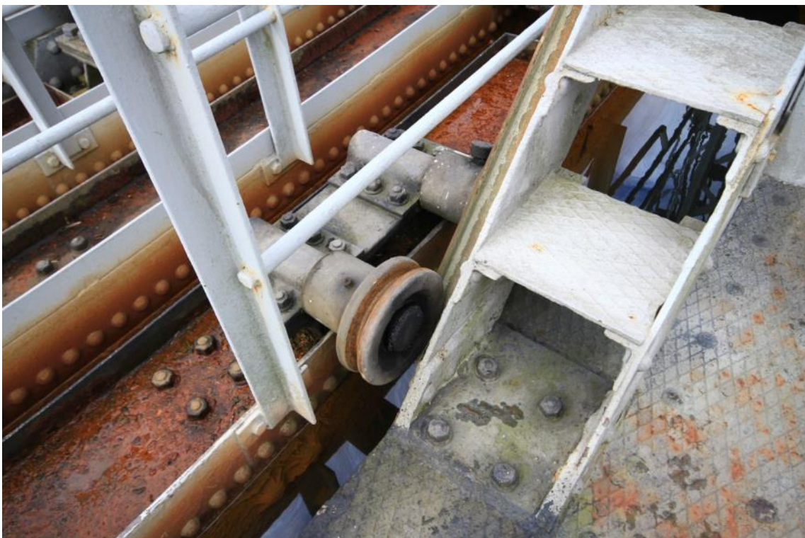
Plate 23: Gasholder No. 5, guide rail on lift stair (ARG15-0161)
