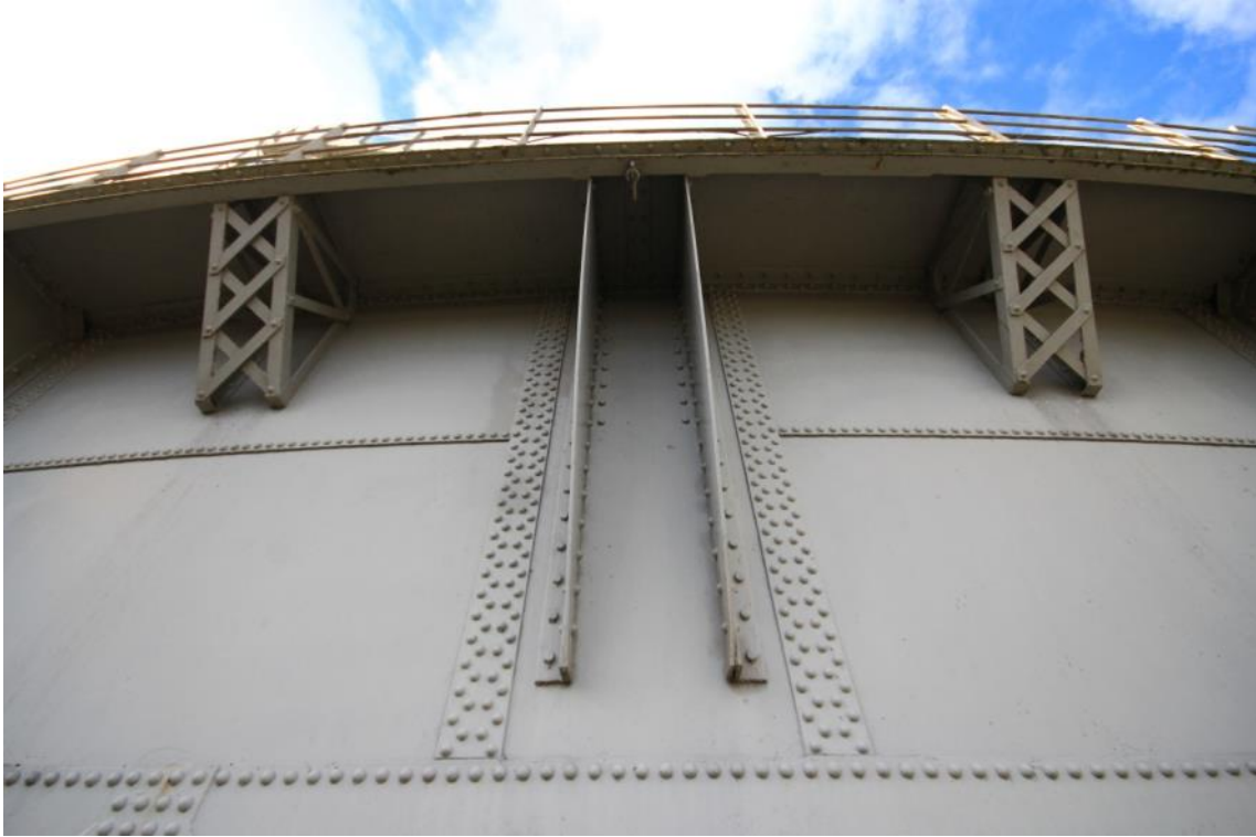
Plate 29: Gasholder No. 5, Support brackets to the tank platform (ARG15-0146)
