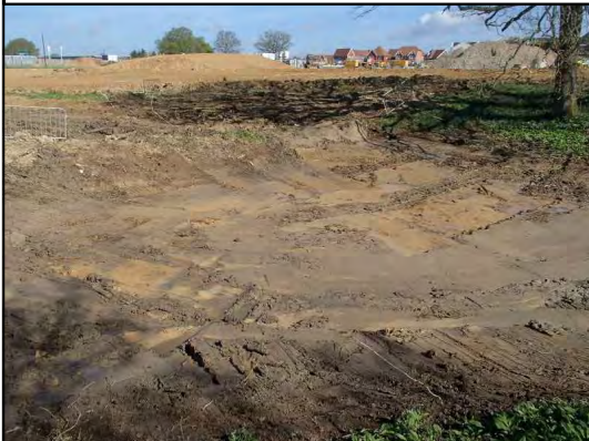
Pond after topsoil removal
