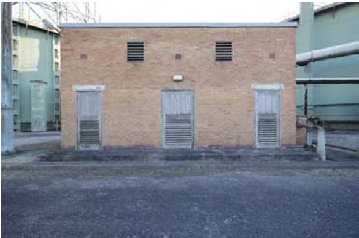
Plate 38: Boiler house (PPD16-0030)
