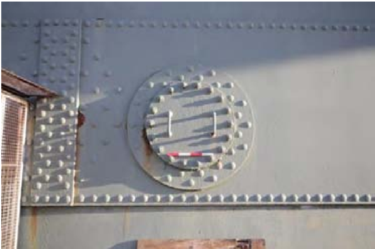
Plate 4: Access hatch in tank wall, Gasholder 6 (PPD16-0007)
