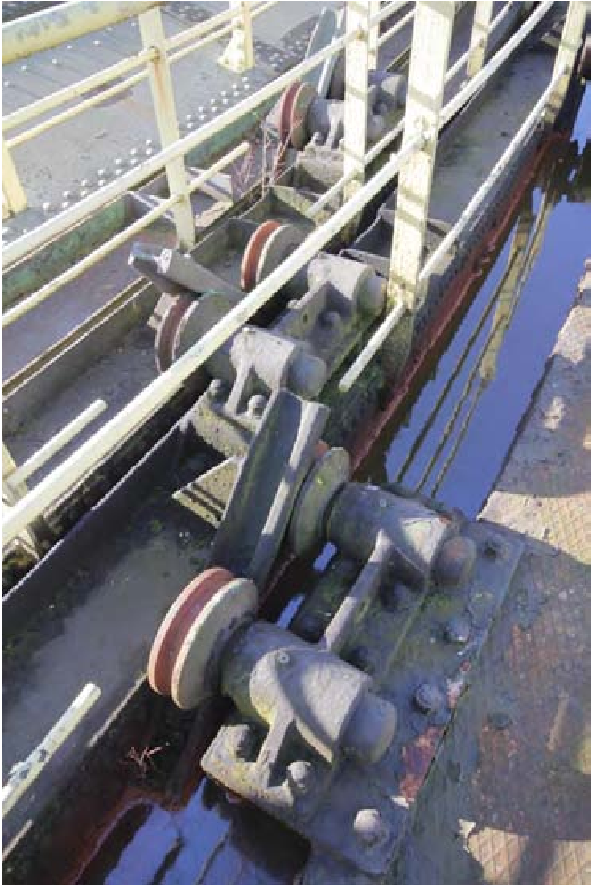
Plate 8: Guide carriages, Gasholder 6 (PPD16-0116)
