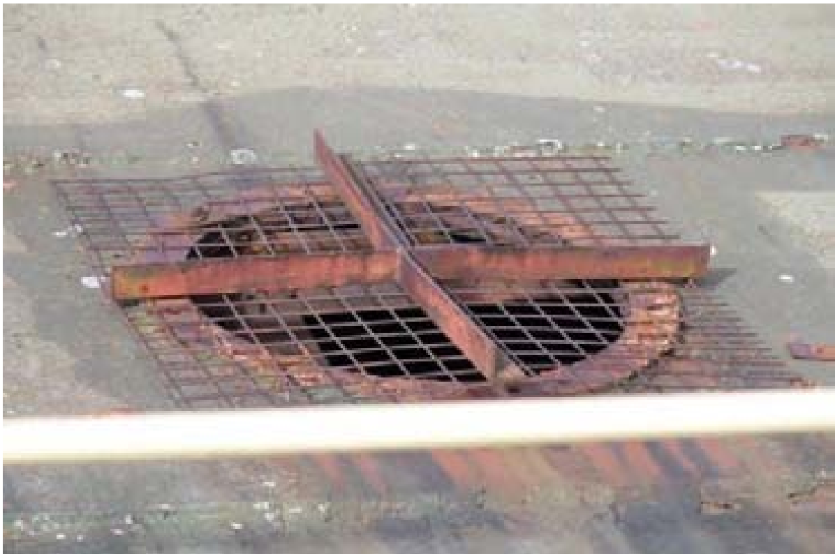
Plate 22: Access hatch in the crown of Gasholder 7 (PPD16-0214)
