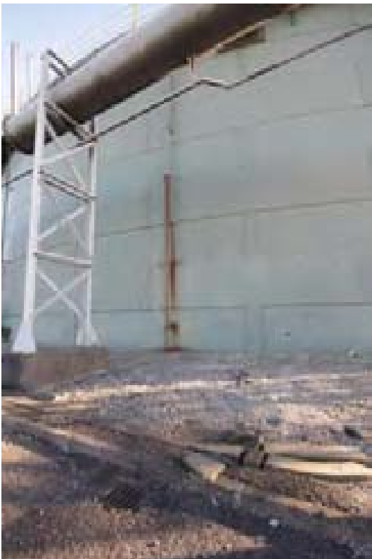
Plate 16: Downpipe, Gasholder 6 (PPD16-0015)
