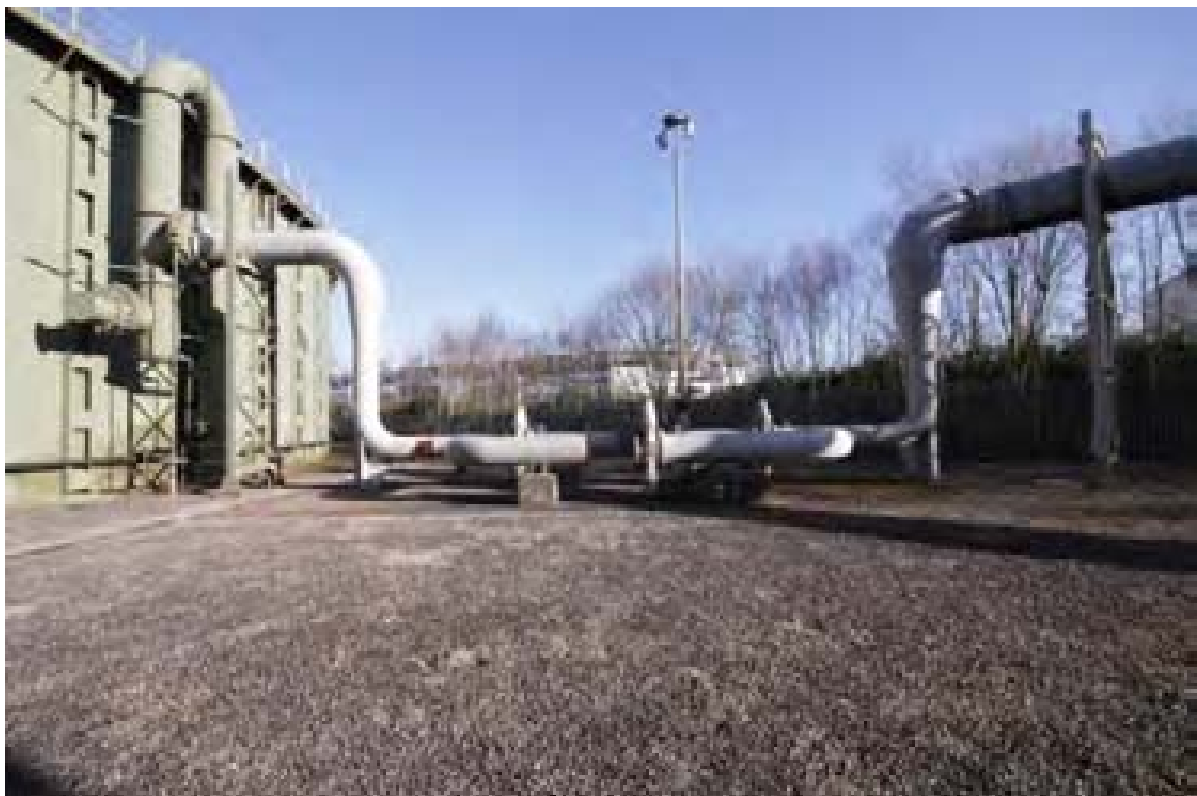
Plate 36: Siphon pit and volumetric governor, Gasholder 7 (PPD16-0076)
