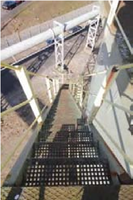
Plate 15: Looking down the staircase from the tank platform, Gasholder 6 (PPD16-0088)
