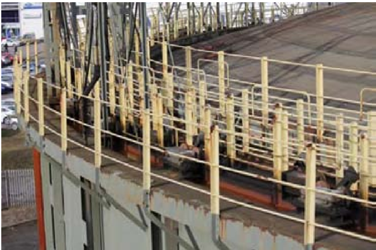
Plate 28: Tank platform walkway and supporting handrails/brackets, Gasholder 7 (PPD16-0222)
