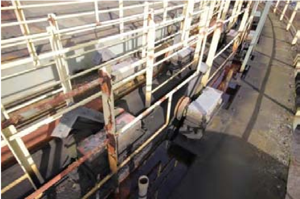
Plate 27: Guide carriages, Gasholder 7 (PPD16-0191)
