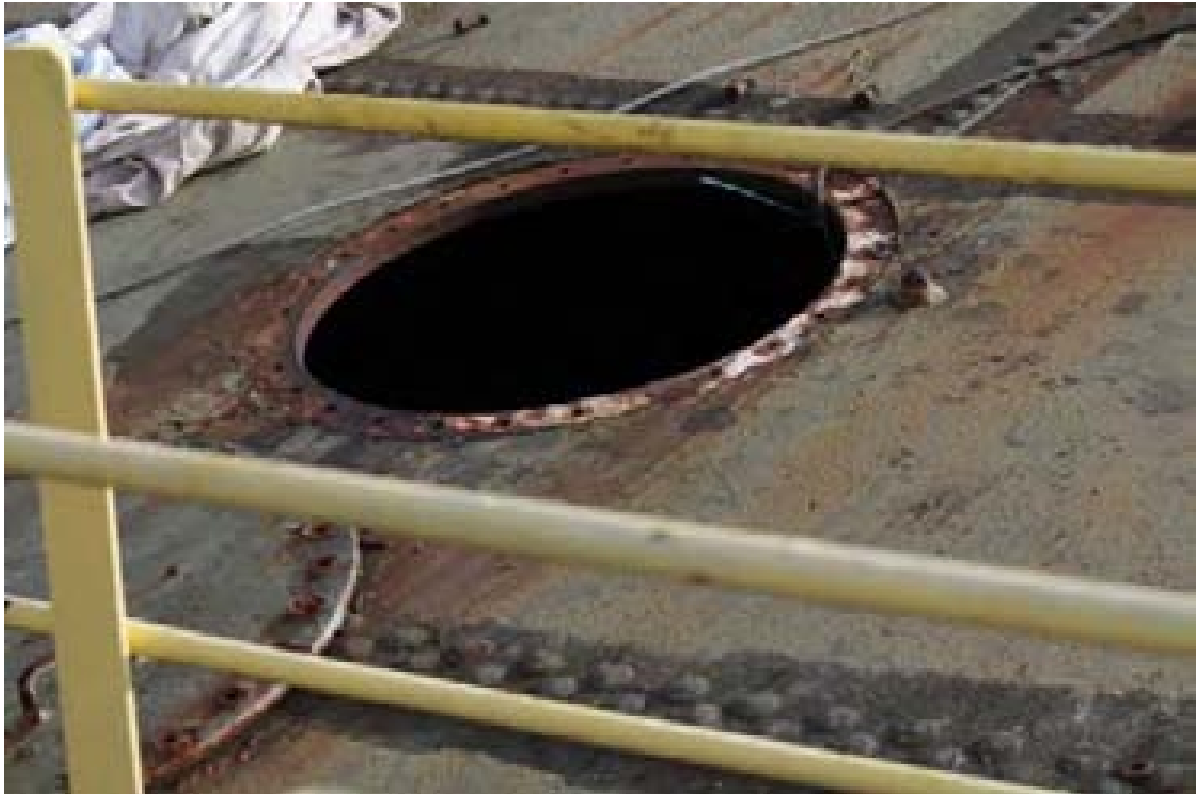
Plate 3: Access hatch in crown of Gasholder 6 (PPD16-0224)
