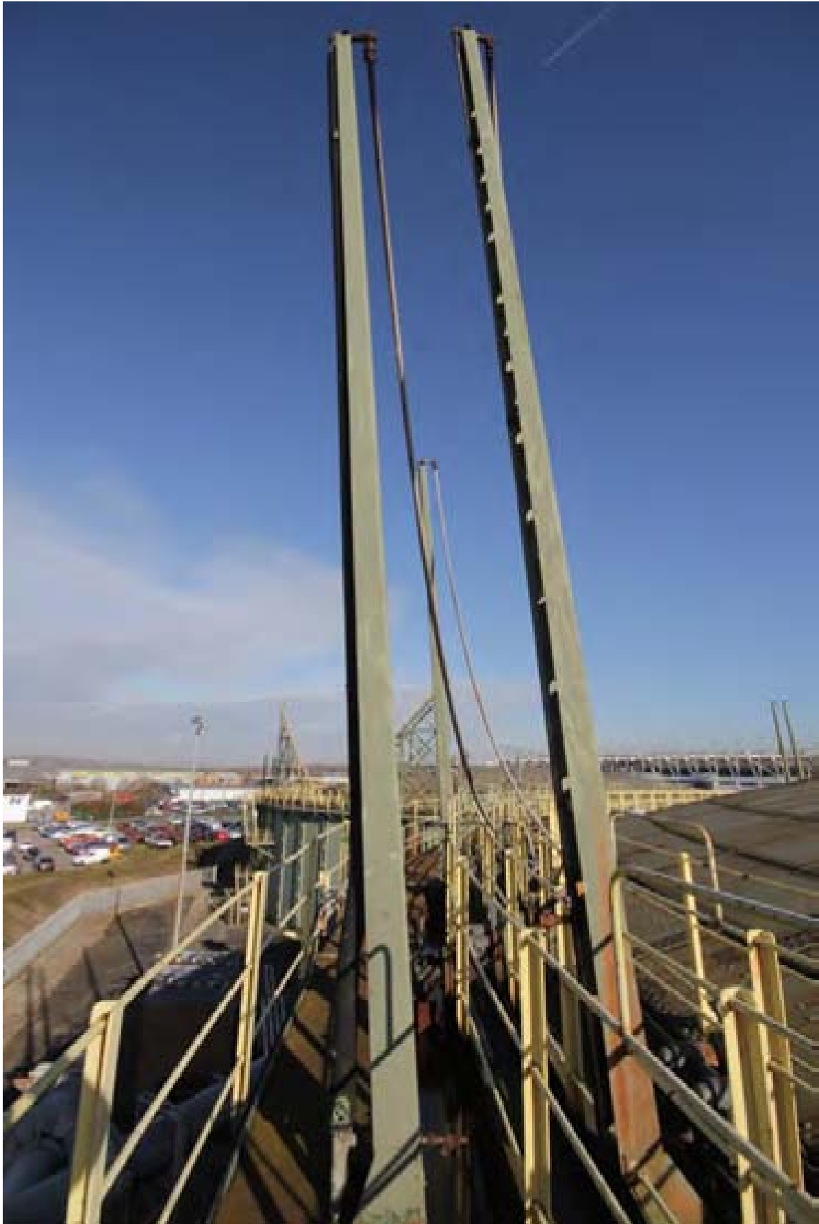
Plate 7: Guide masts for antifreeze distribution hoses, Gasholder 6 (PPD16-0125)
