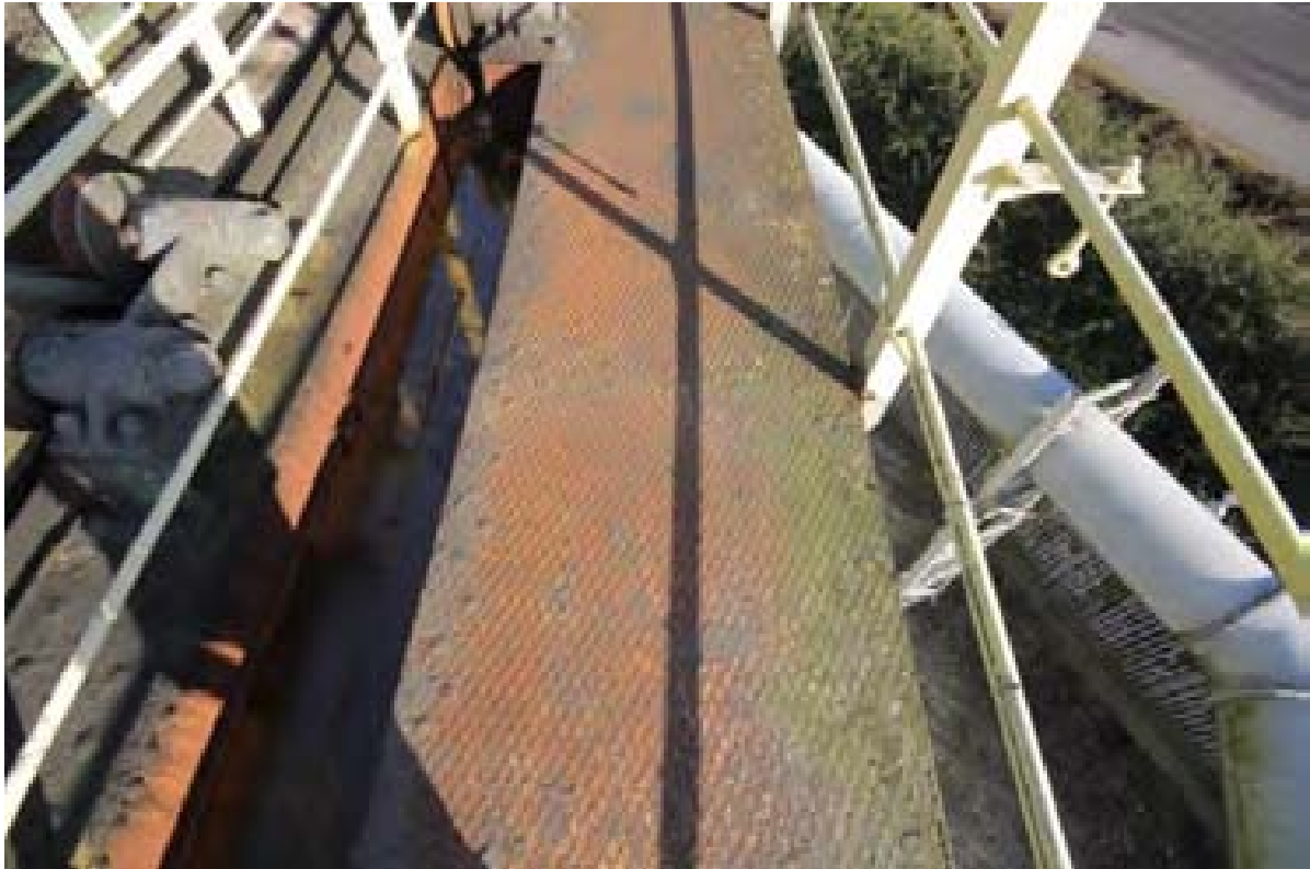
Plate 9: Tank platform walkway (PPD16-0108)
