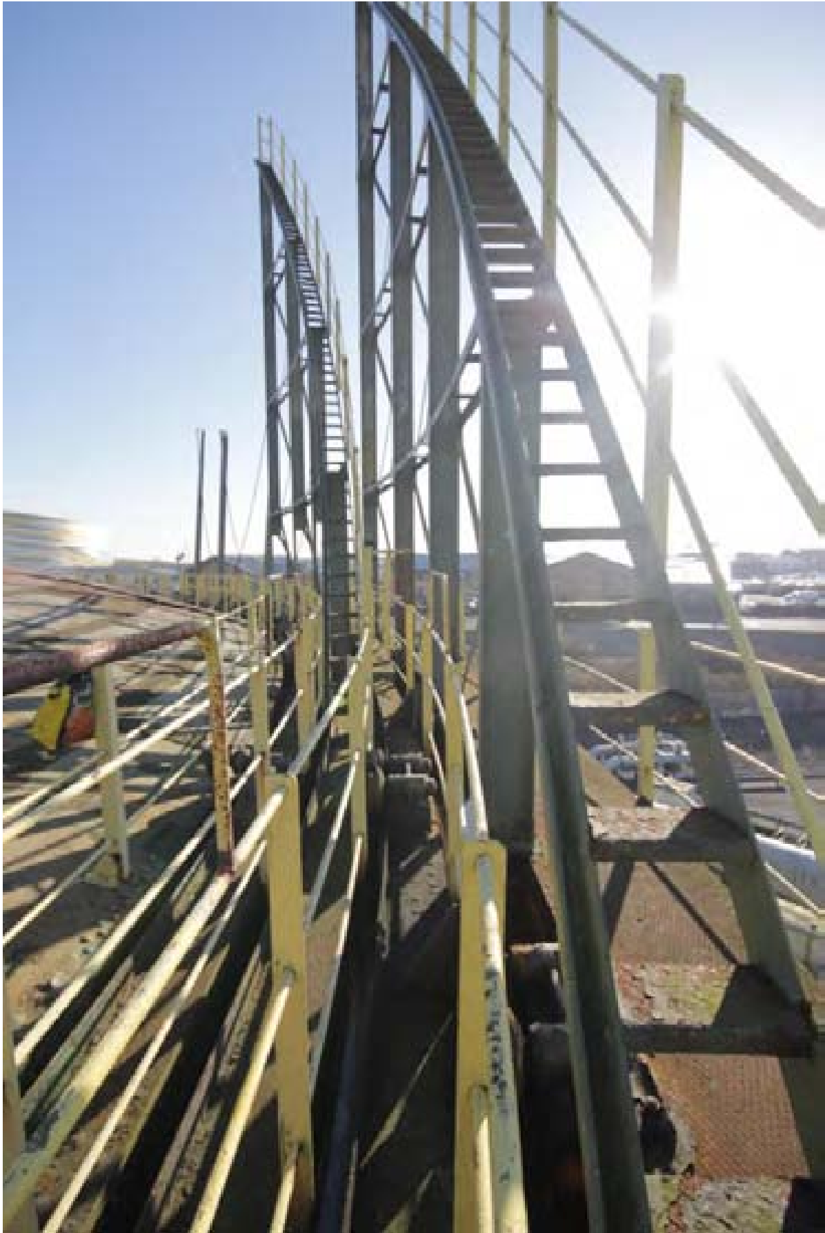
Plate 11: Lift stairs on Gasholder 6, note the grooved guide rail (PPD16-0083)
