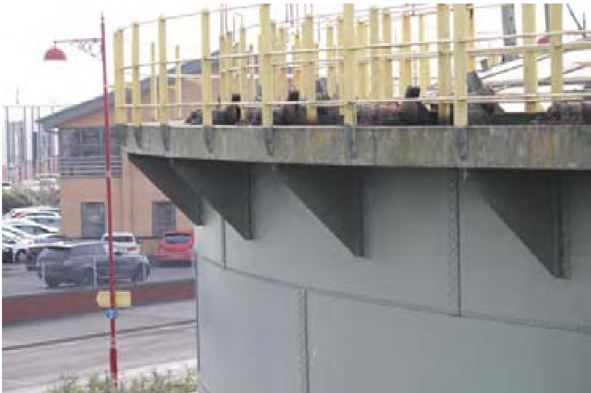
Plate 10: Brackets and rim to tank platform walkway (PPD16-0217)
