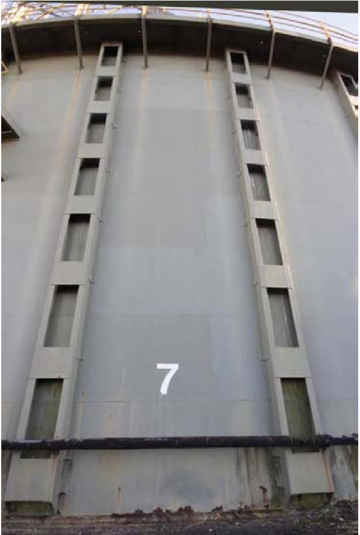
Plate 33: Stanchions on the side of Gasholder 7 (PPD16-0059)
