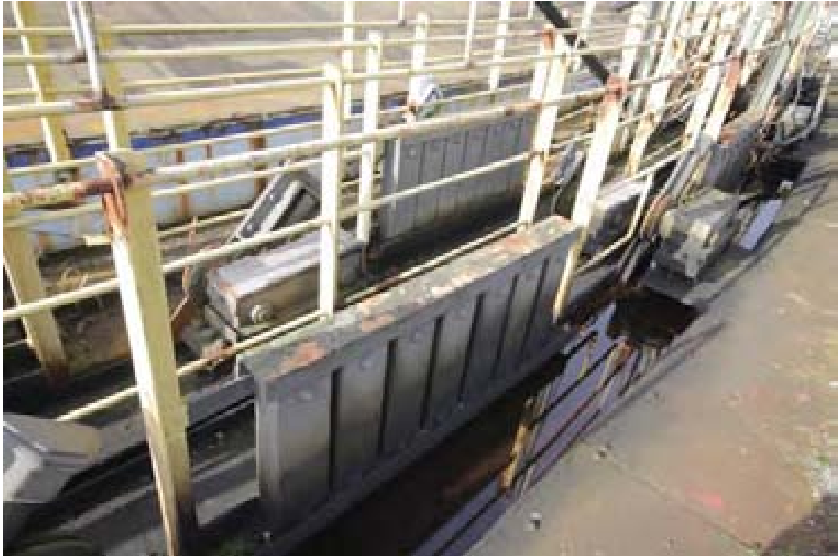
Plate 29: Counterweights diametrically opposite the lift stairs, Gasholder 7 (PPD16-0196)
