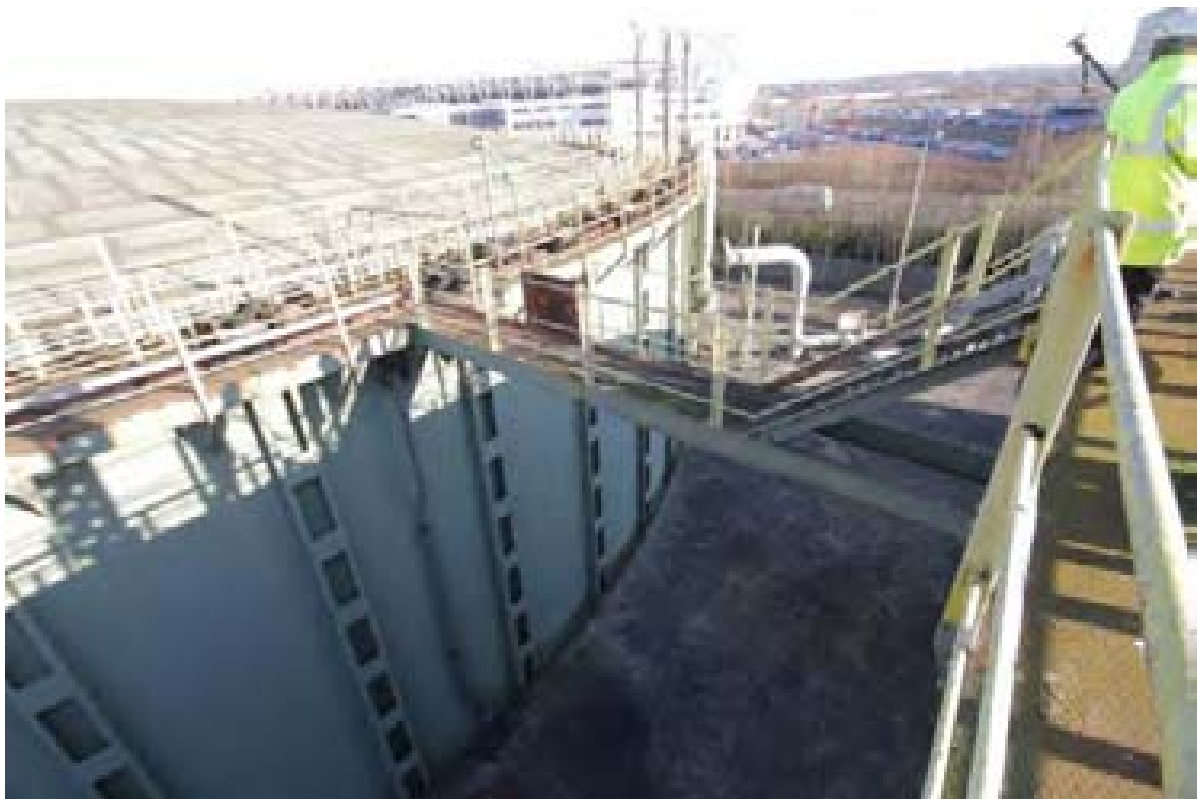
Plate 35: Bridge between the gasholders (PPD16-0134)
