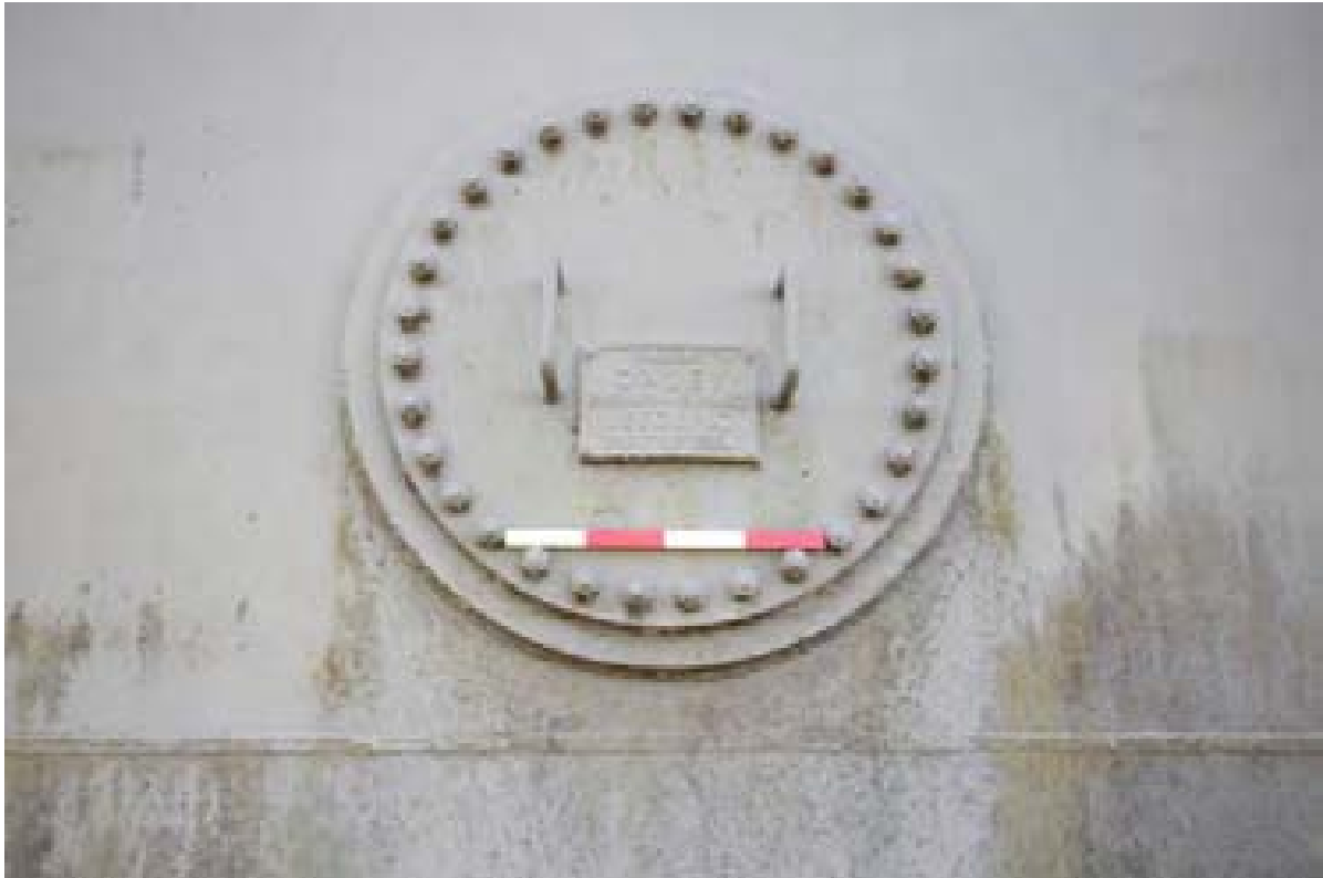
Plate 23: Access hatch in tank wall displaying makers marks, Gasholder 7 (PPD16-0068)
