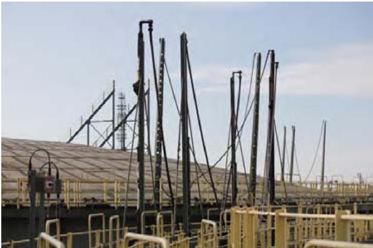
Plate 26: Guide masts, Gasholder 7 (PPD16-0209)
