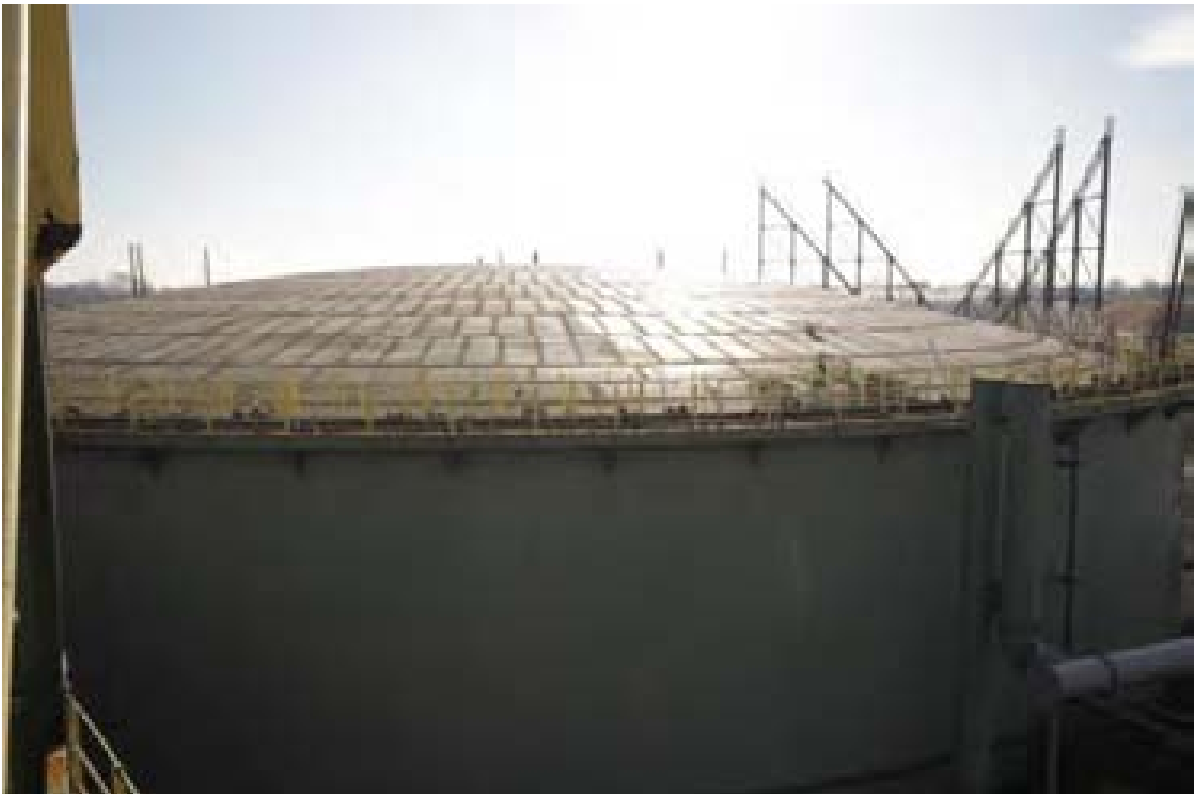
Plate 2: The crown of Gasholder 6 as seen from Gasholder 7 (PPD16-0170)
