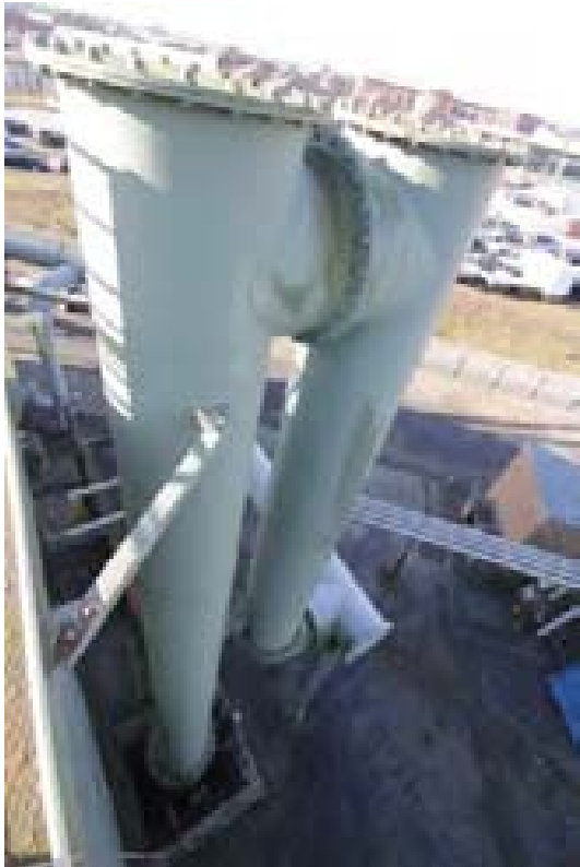
Plate 17: Pipework and siphon pit, Gasholder 6 (PPD16-0130)
