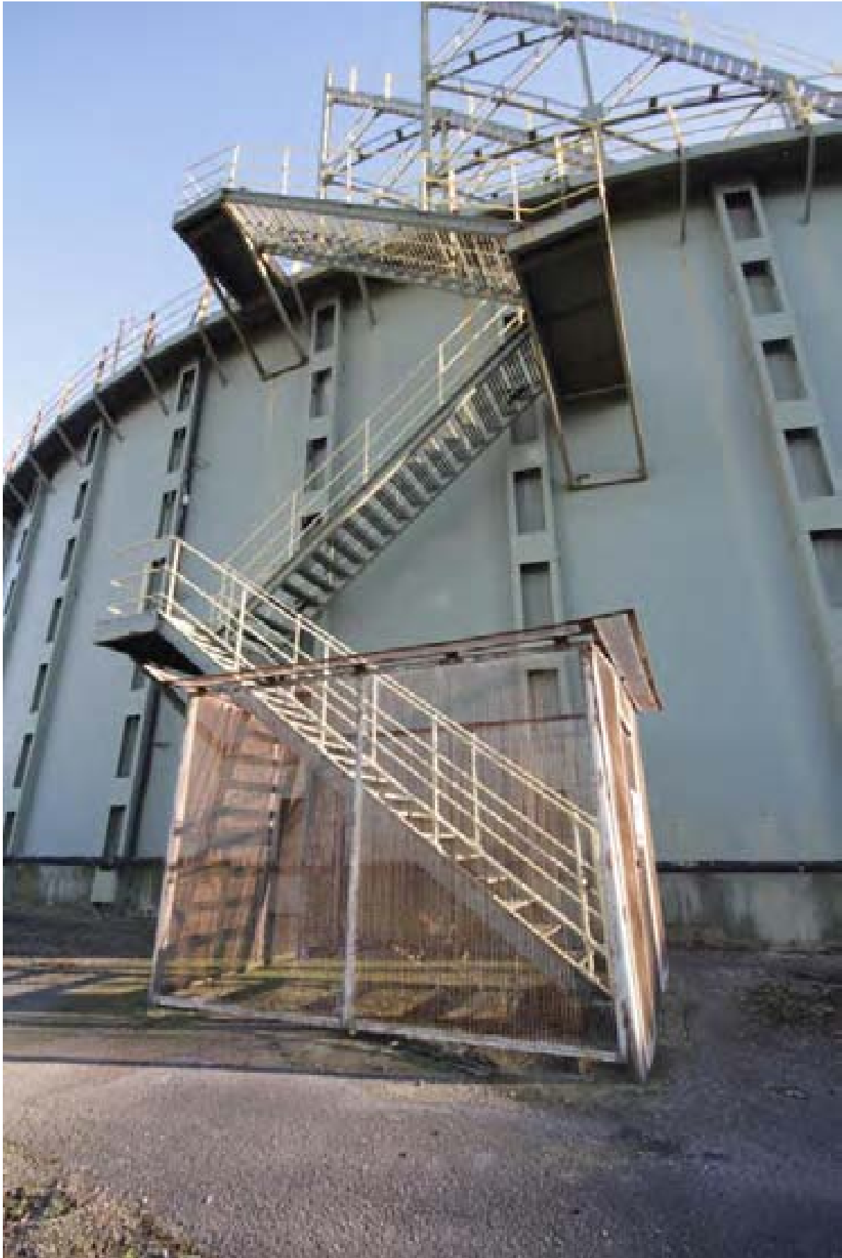
Plate 34: Staircase to tank platform, Gasholder 7 (PPD16-0061)
