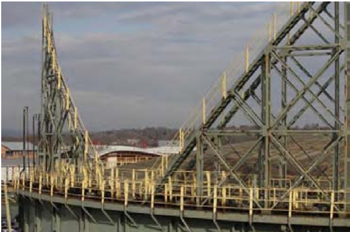
Plate 30: Lift stairs, Gasholder 7 (PPD16-0227)
