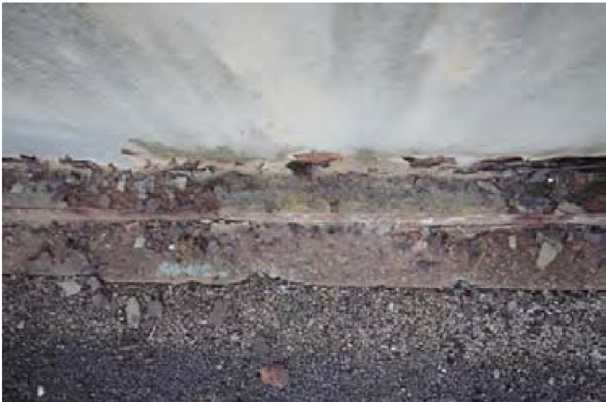
Plate 32: Concrete base to Gasholder 7 (PPD16-0053)
