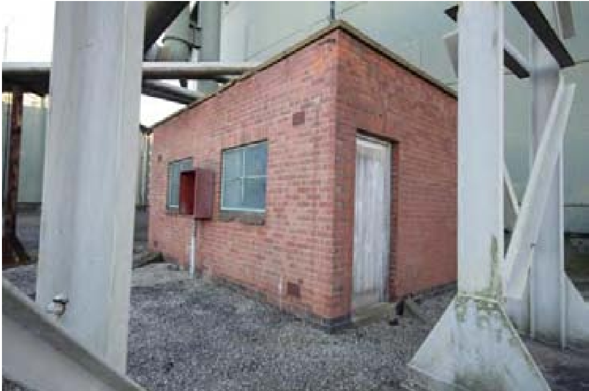
Plate 37: Antifreeze pump house (PPD16-0024)
