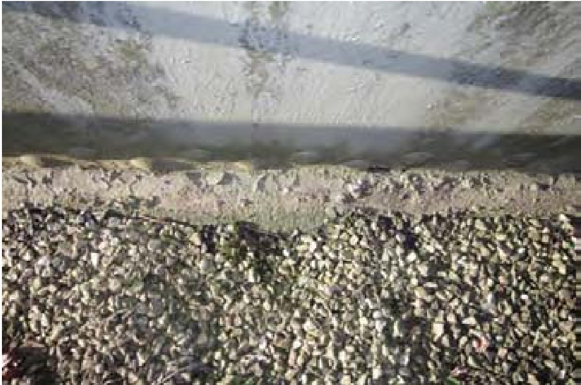
Plate 12: Detail shot of the concrete base to Gasholder 6 (PPD16-0045)
