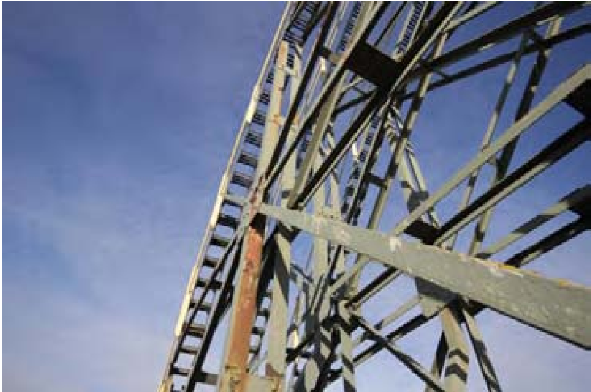
Plate 31: Construction of the lift stairs, Gasholder 7 (PPD16-0155)
