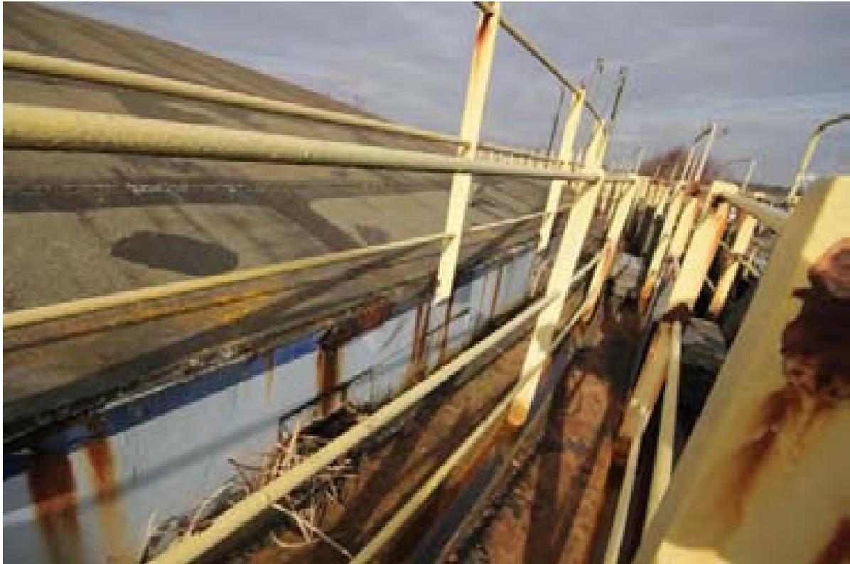
Plate 21: The raised rim to the first lift and crown of Gasholder 7 (PPD16-0200)
