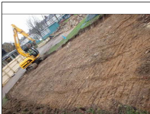
Excavated ramp area, facing north west
