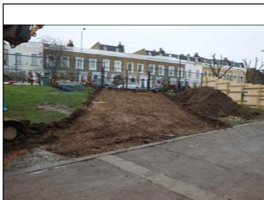
Excavated ramp area, facing east
