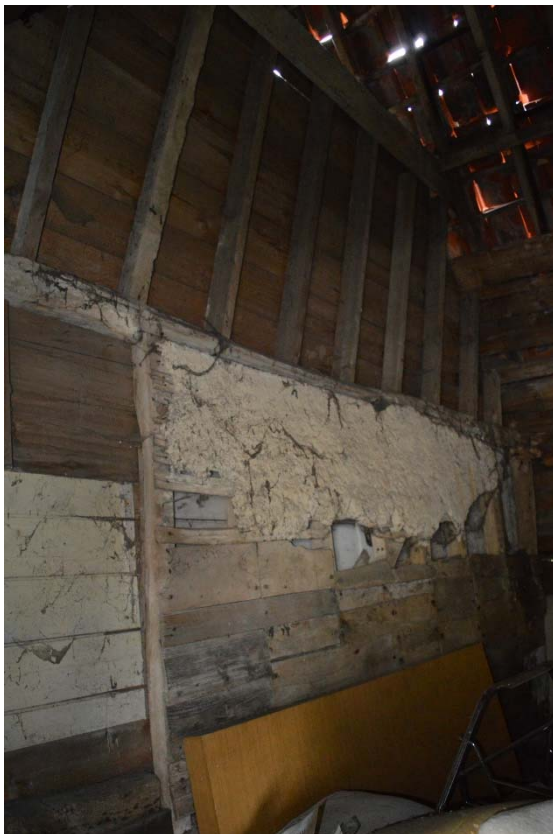
Plate 22: Interior of stable, Bay 3. Remains of daub partition, looking south-east (HRWF_065)
