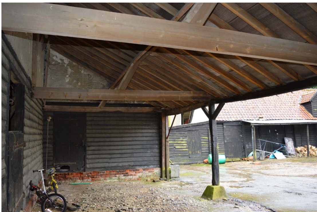
Plate 2: Interior of barn shelter, looking south (HRWF_021)
