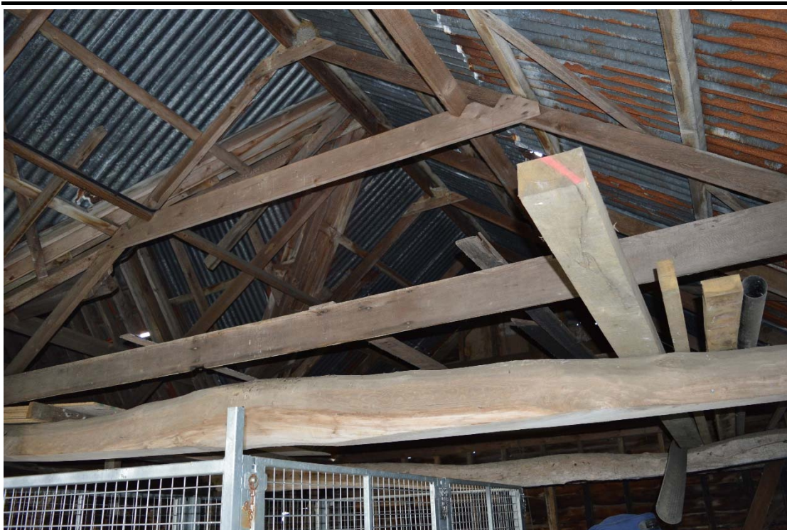
Plate 27: Interior of stable, Bay 5 roof, looking south (HRWF_072)
