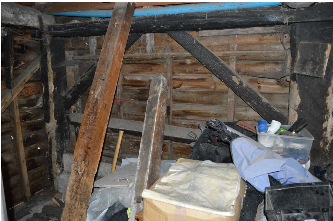
Plate 26: Interior of stable, Bay 5, looking west (HRWF_074)
