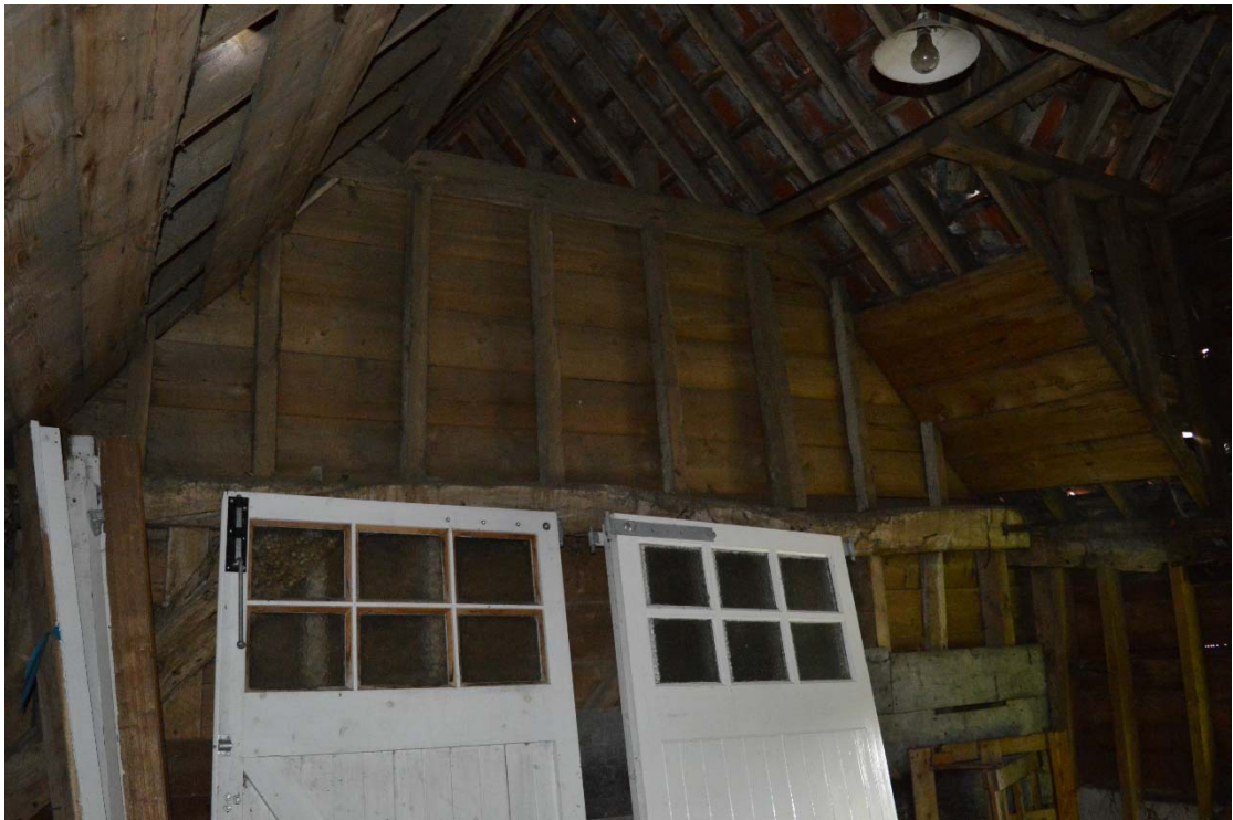
Plate 21: Interior of stable, Bay 3, looking west (HRWF_067)
