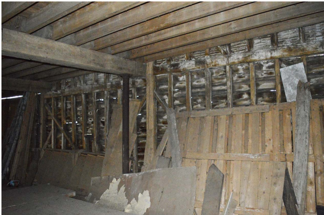
Plate10: Ground floor of barn, Bays 1 and 2, looking north-east (HRWF_031)
