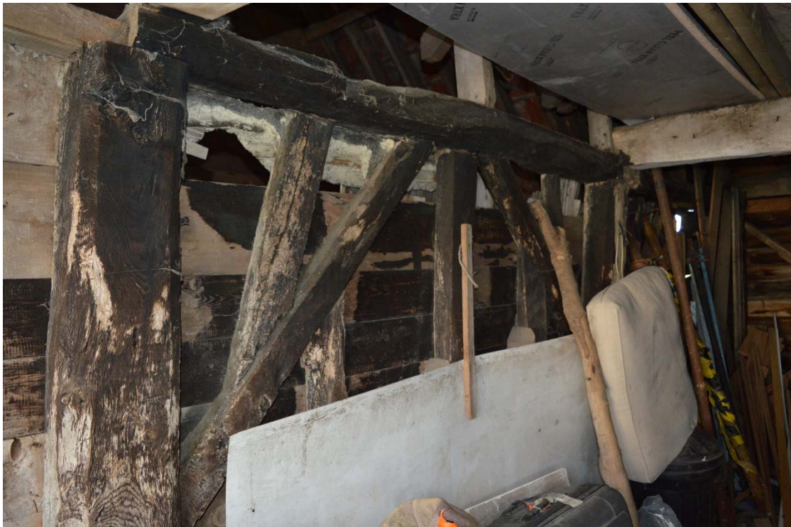
Plate 25: Interior of stable, Bay 5. Stud wall built with rough, large scantling timber, looking south-east (HRWF_073)
