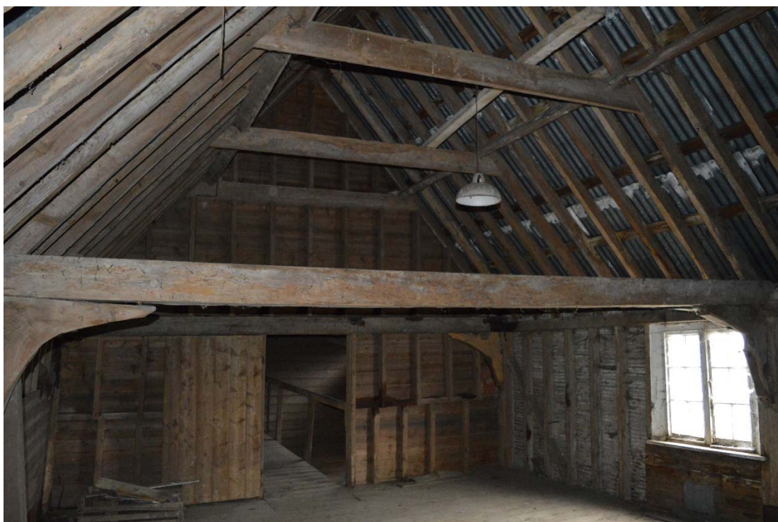
Plate 8: Barn roof structure, Bays 1 and 2, looking north (HRWF_047)
