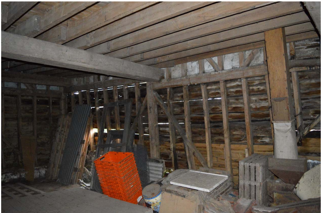
Plate 6: Interior of barn, Bays 1 and 2, looking west (HRWF_032)
