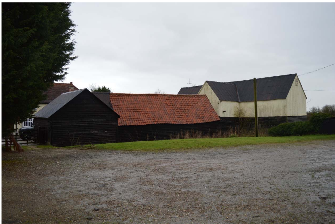
Plate 18: South elevation of stable, backing onto presumed moat (HRWF_004)
