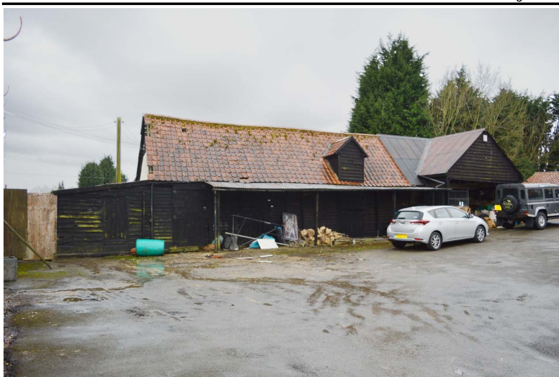
Plate 19: North elevation of stable facing into yard (HRWF_014)
