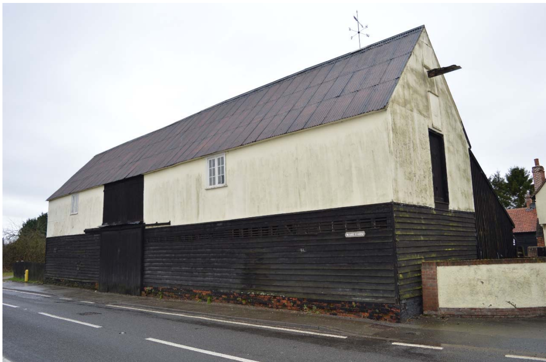
Plate 4: North and east elevations of barn (HRWF_013)
