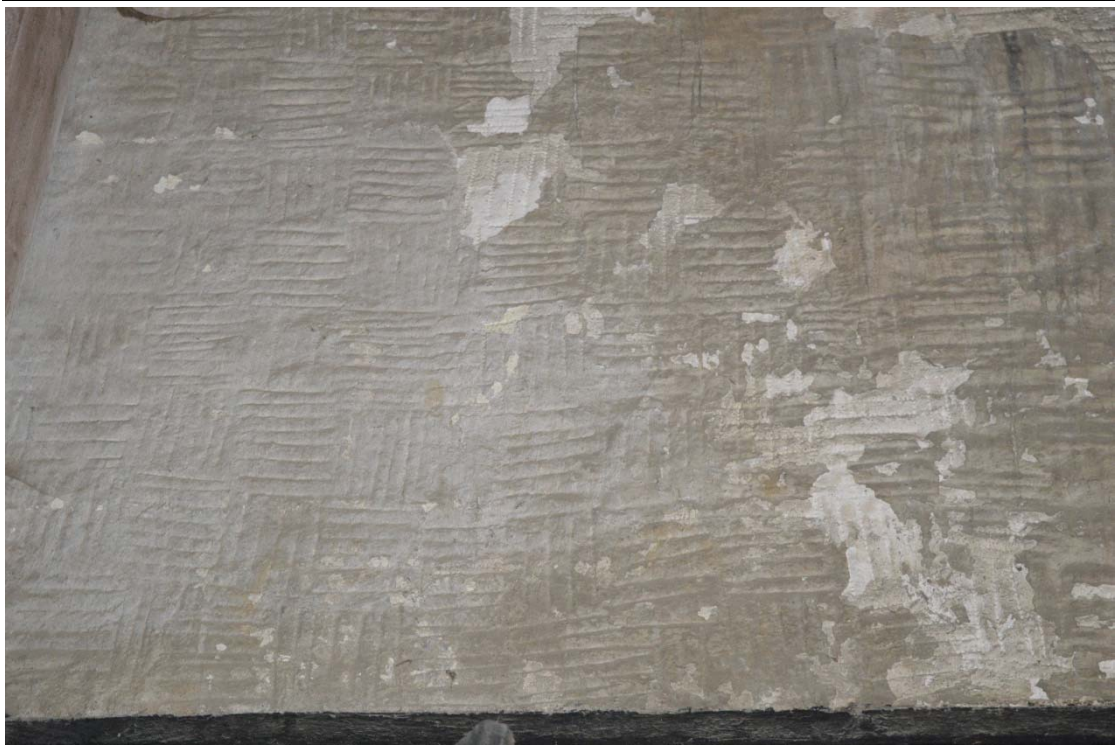
Plate 3: Decorative plaster on exterior of wagon porch wall, looking south (HRWF_020)
