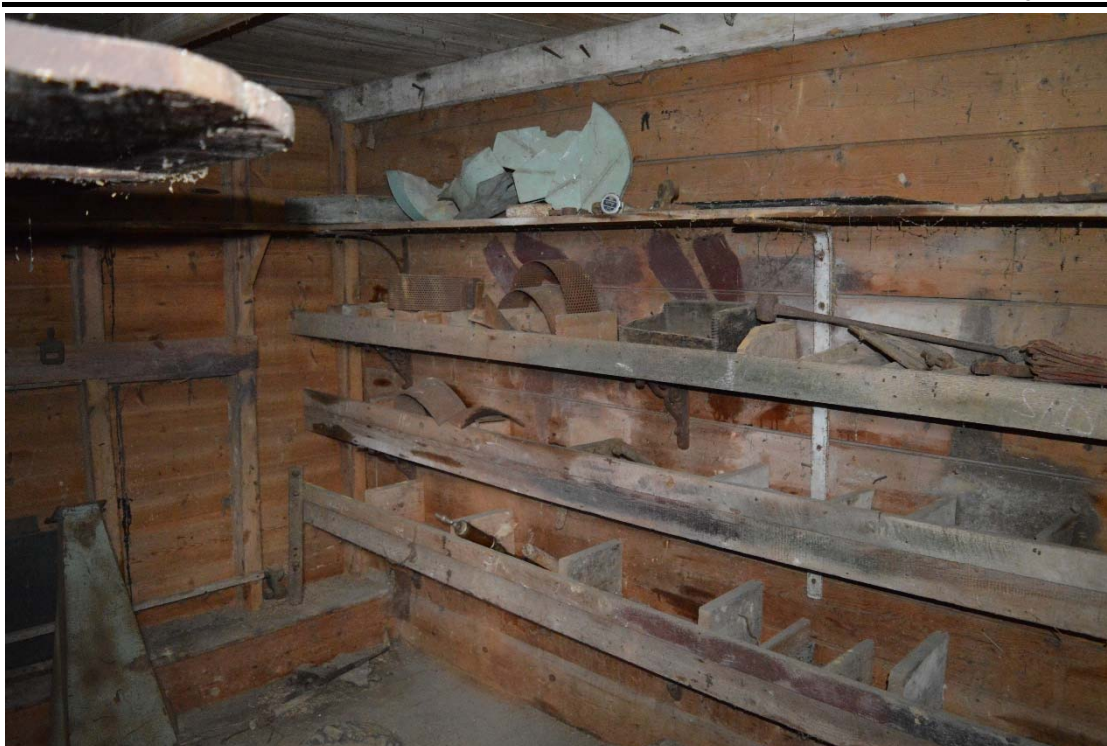
Plate 17: First floor of barn, part of Bay 6 converted into store room, looking south-west (HRWF_060)
