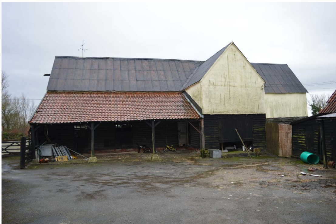
Plate 1: West elevation of barn showing midstrey and later shelter (HRWF_017)
