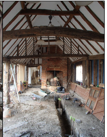
The south wing interior works, looking north
