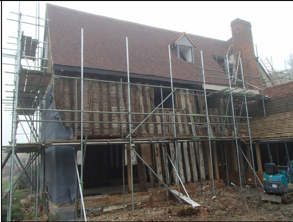
The west wing during works, looking north
