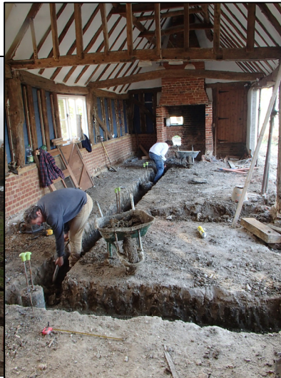
The south wing interior works, looking south
