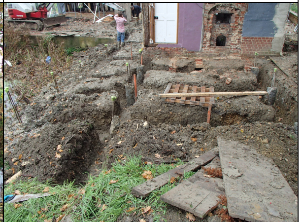
Exterior works to the south of the south wing, looking north
