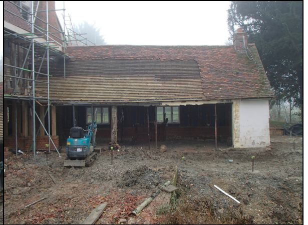
The south wing during works looking east
