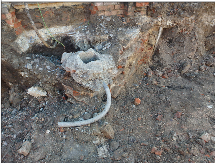
Wall 11 looking south-east
