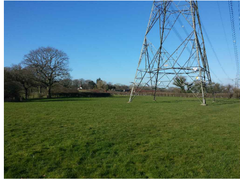
Fig. 10b westernmost enclosure showing electricity tower base
