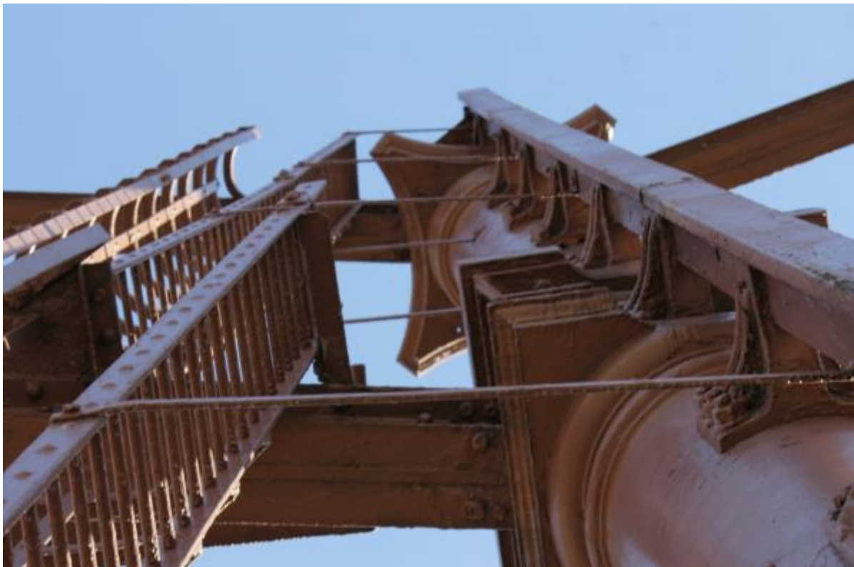
Plate 35: Ladder and guide rail detail (MRA16-0223)
