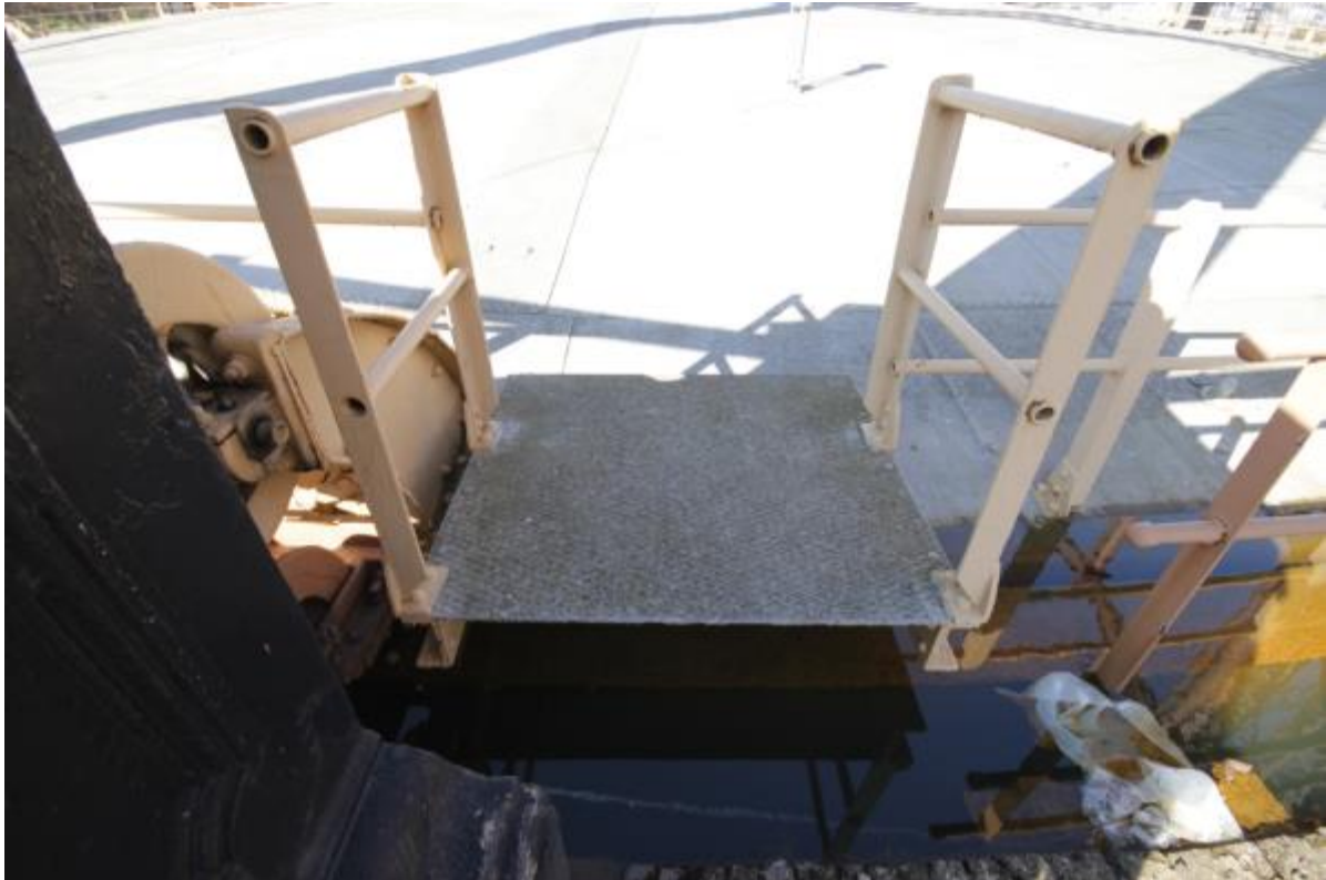
Plate 31: Bridge to the crown of Gasholder No. 2 (MRA16-0208)
