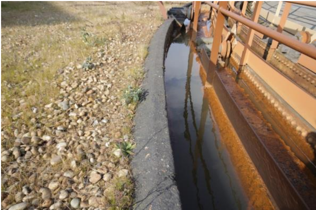
Plate 3: Concrete rim to the brick tank of Gasholder No. 1 (MRA16-0012)
