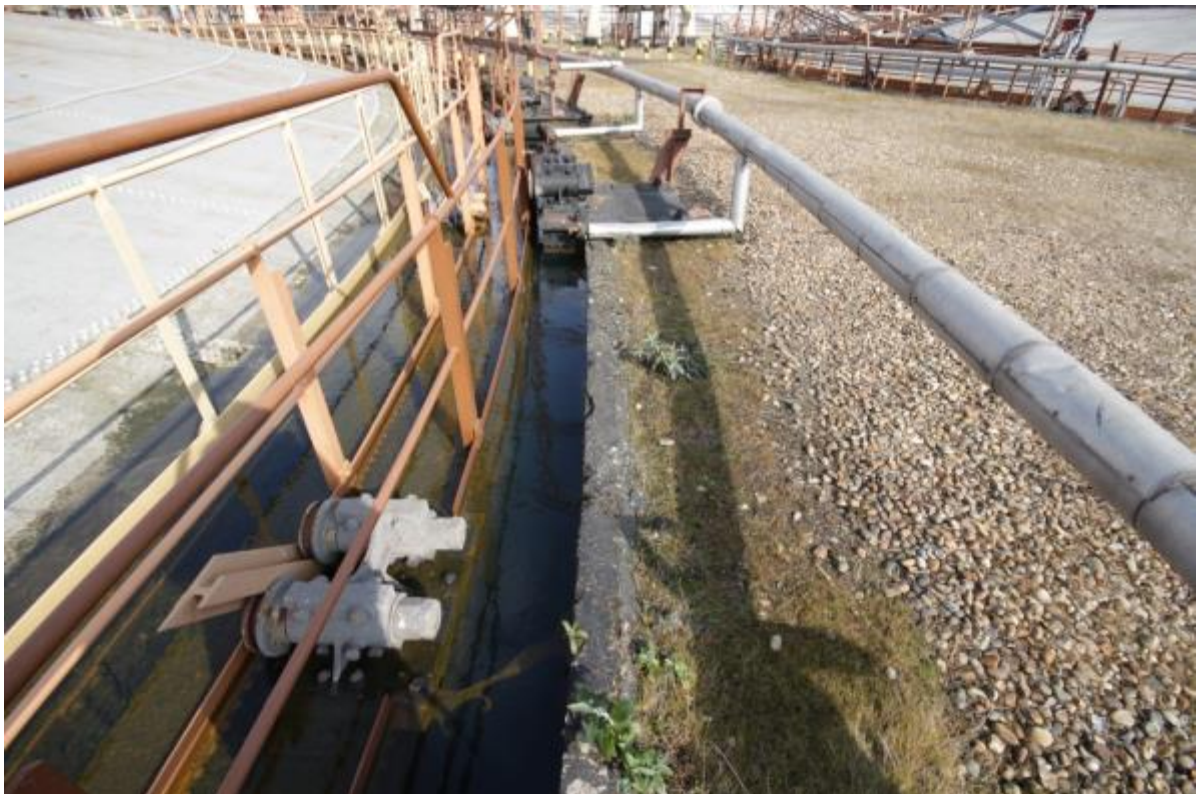
Plate 17: Concrete rim and ring main to Gasholder No. 4 (MRA16-0072)
