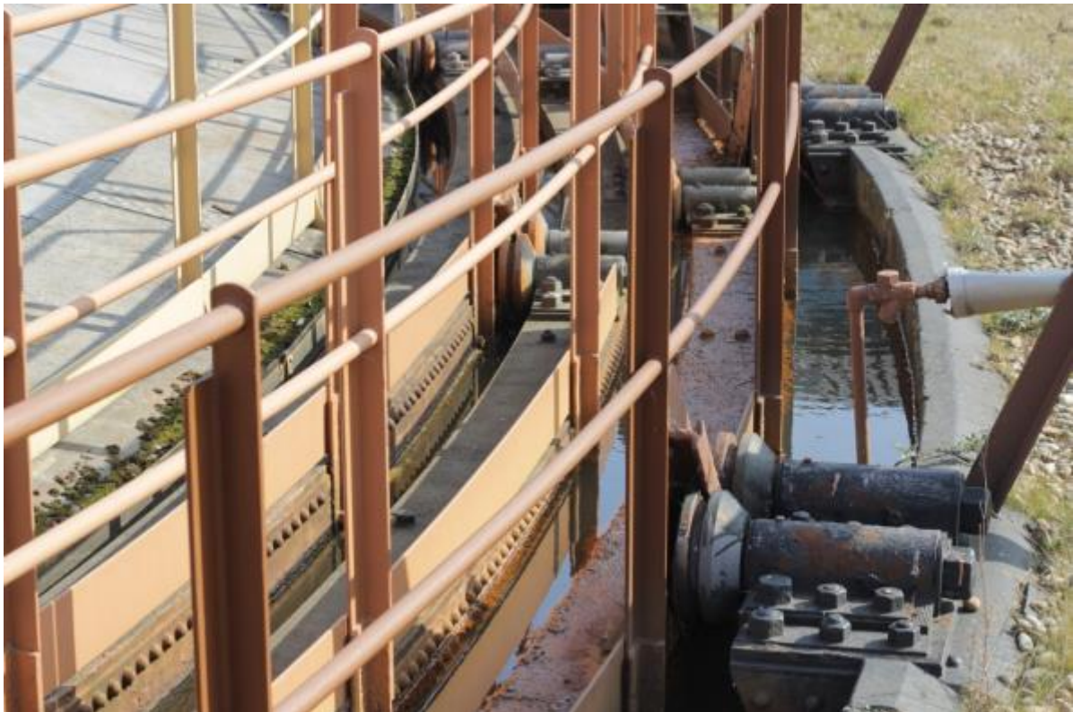
Plate 5: Lift grips and lutes on Gasholder No. 1 (MRA16-0067)
