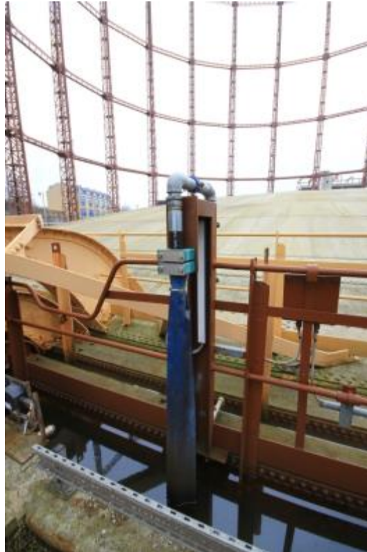
Plate 50: Hose guide, Gasholder No. 5 (MRA16-0249)
