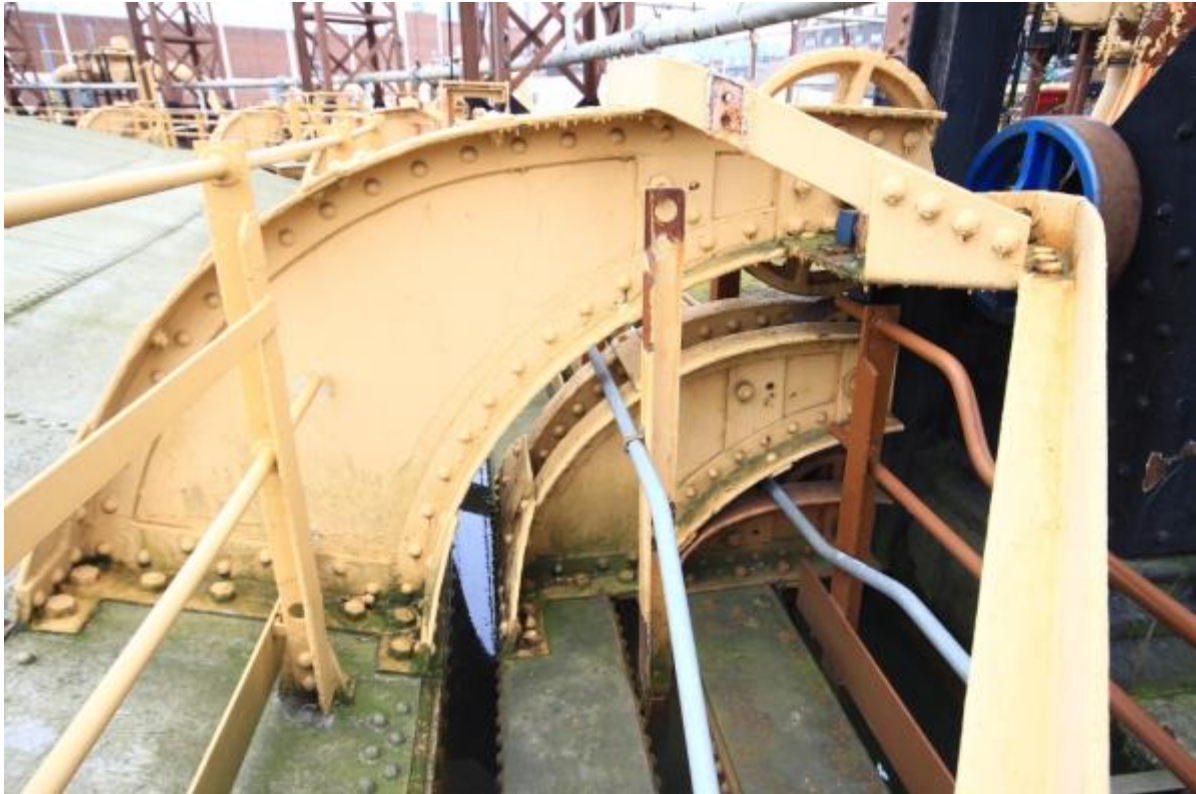
Plate 48: Guide carriages, Gasholder No. 5 (MRA16-0252)
