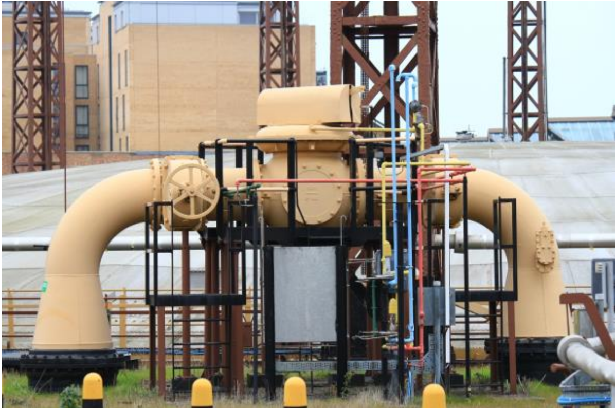
Plate 14: Volumetric governor, Gas holder No. 1 (MRA16-0351)
