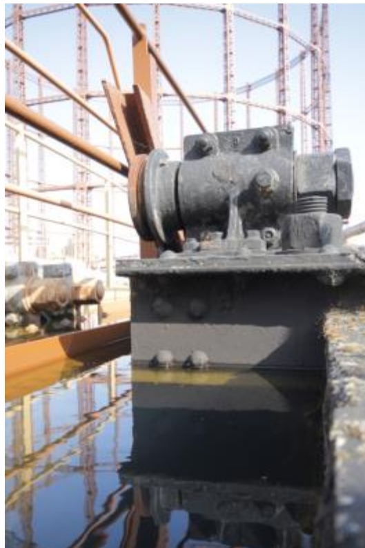
Plate 24: Outer guide carriage projecting into the lute (MRA16-0082)
