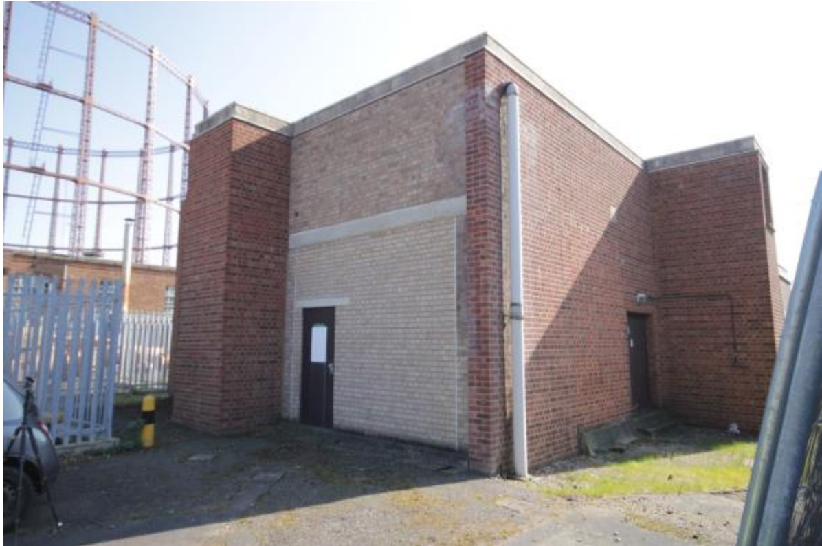
Plate 59: The Gas Pumping Plant Building (MRA16-0148)
