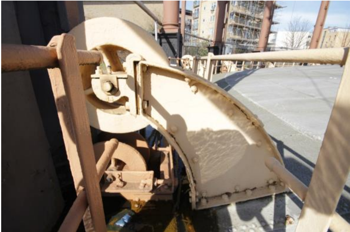
Plate 36: Guide carriages, Gasholder No. 2 (MRA16-0166)
