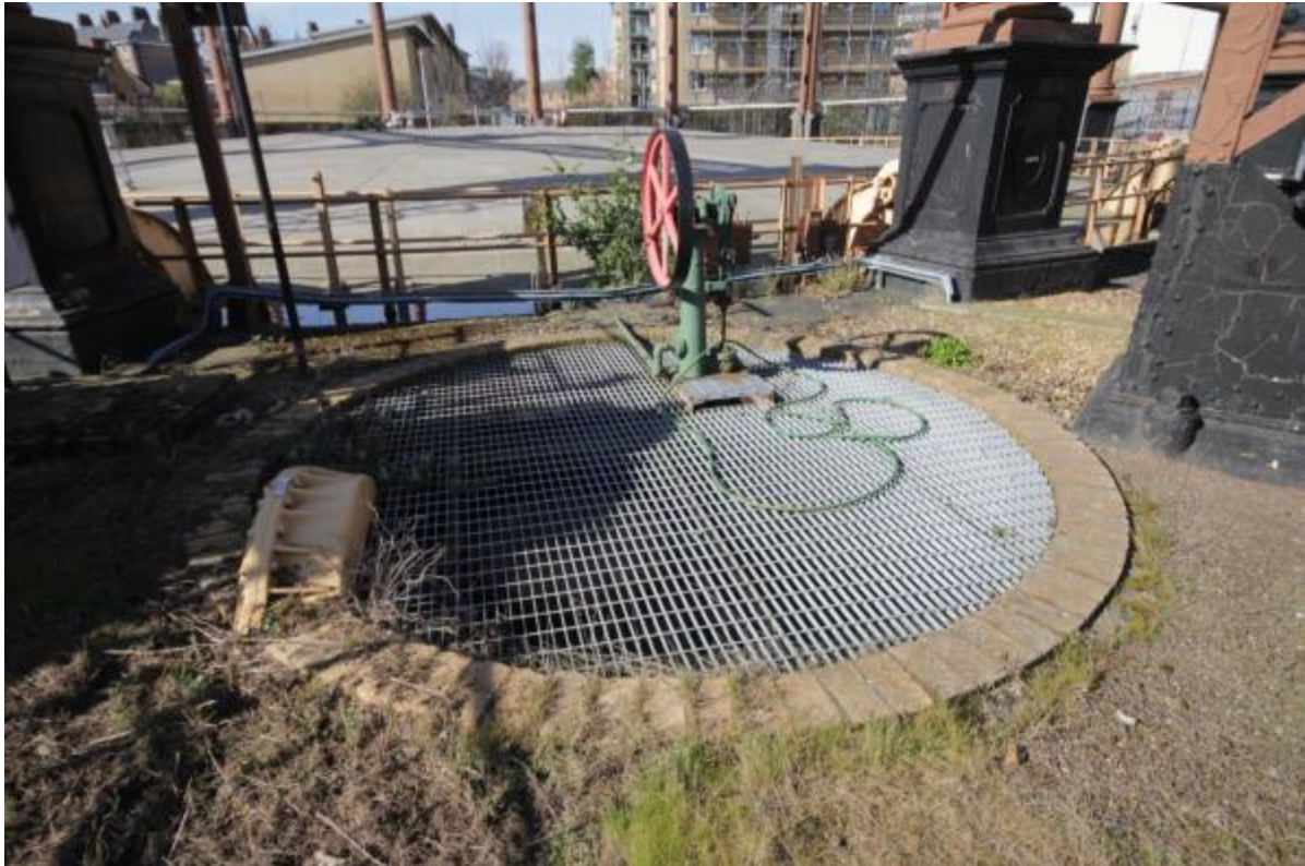
Plate 39: Siphon pit, pump, and piping, Gasholder No. 2 (MRA16-0197)
