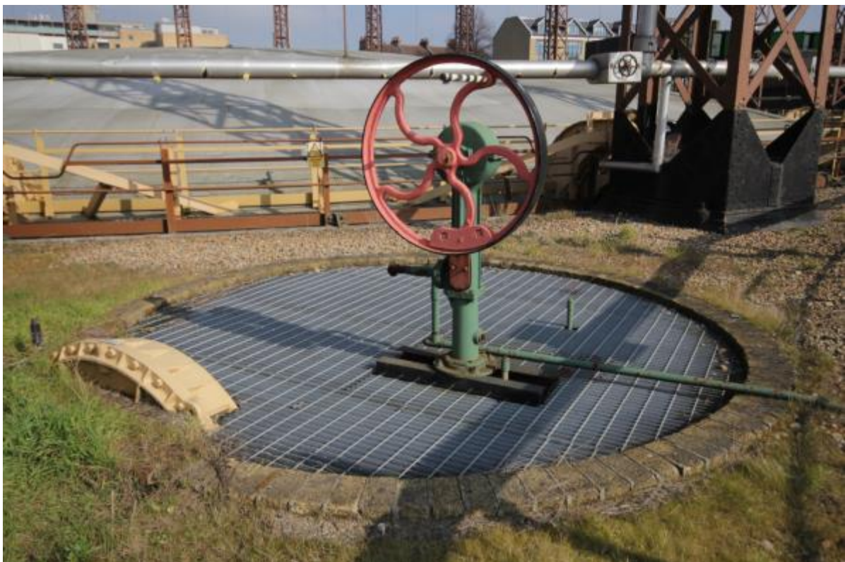
Plate 15: Siphon pit, Gas holder No. 1 (MRA16-0055)
