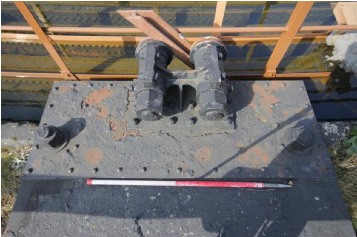
Plate 23: Guide carriage to outer lift (MRA16-0075)
