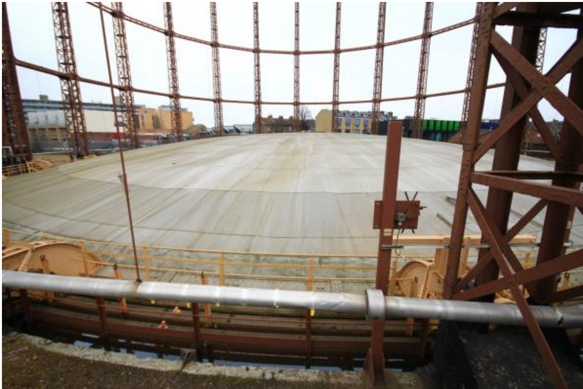
Plate 43: Crown of Gasholder No. 5 (MRA16-0385)
