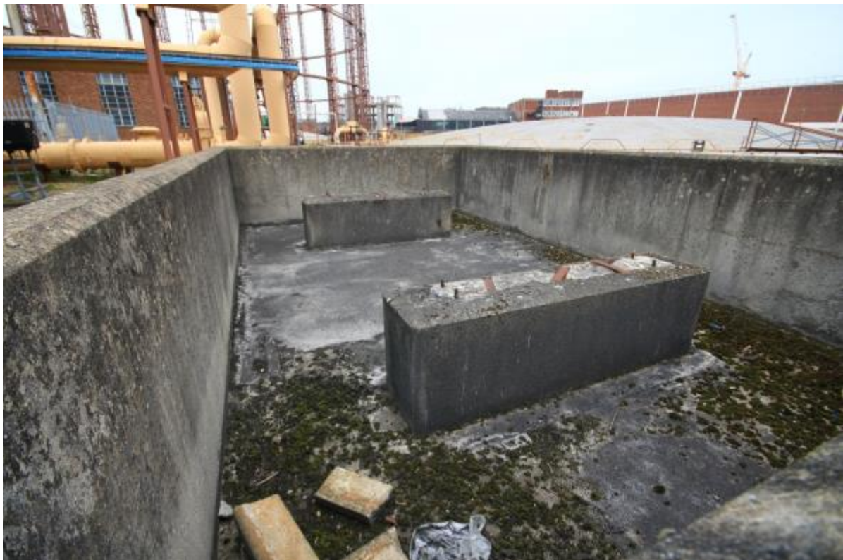
Plate 66: Former Fuel Store (MRA16-0401)
