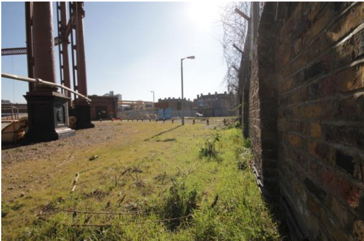
Plate 68: North compound wall (MRA16-0181)
