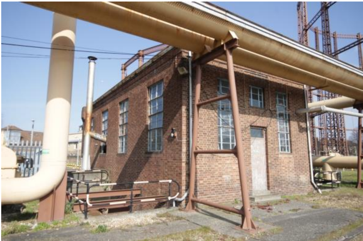
Plate 56: The Valve House (MRA16-0108)
