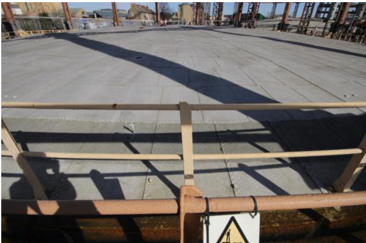
Plate 30: Crown of Gasholder No. 2 (MRA16-0162)
