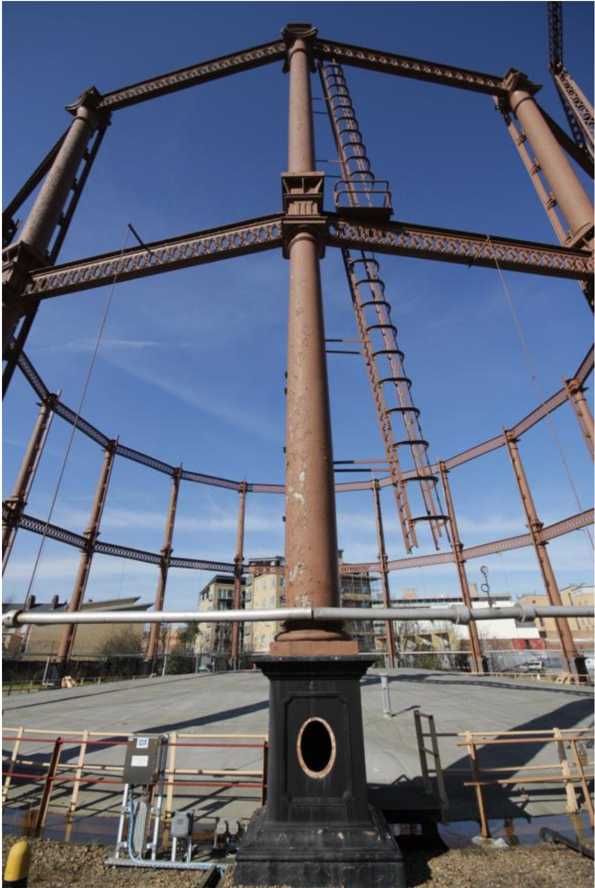
Plate 38: Ladders and column overview, Gasholder No. 2 (MRA16-0206)
