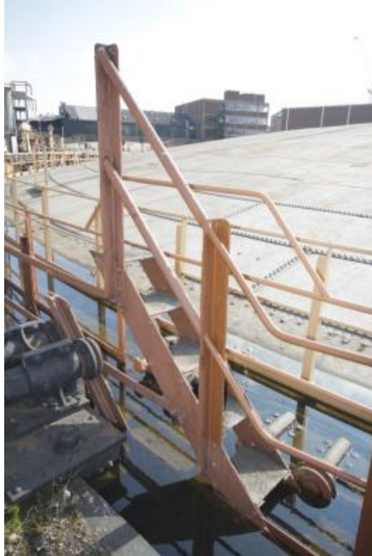
Plate 25: Lift stairs, Gasholder No. 4 (MRA16-0096)
