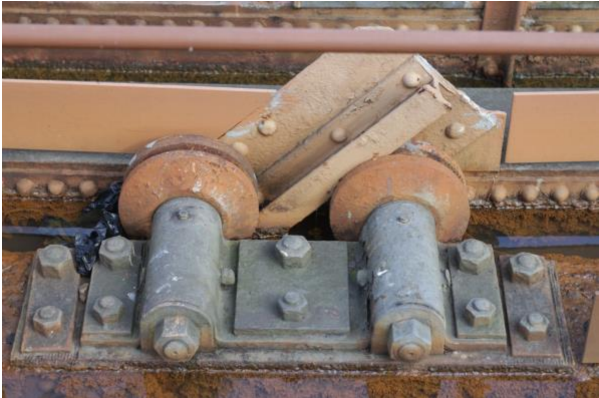
Plate 10: Guide carriage to inner lifts (MRA-0062)
