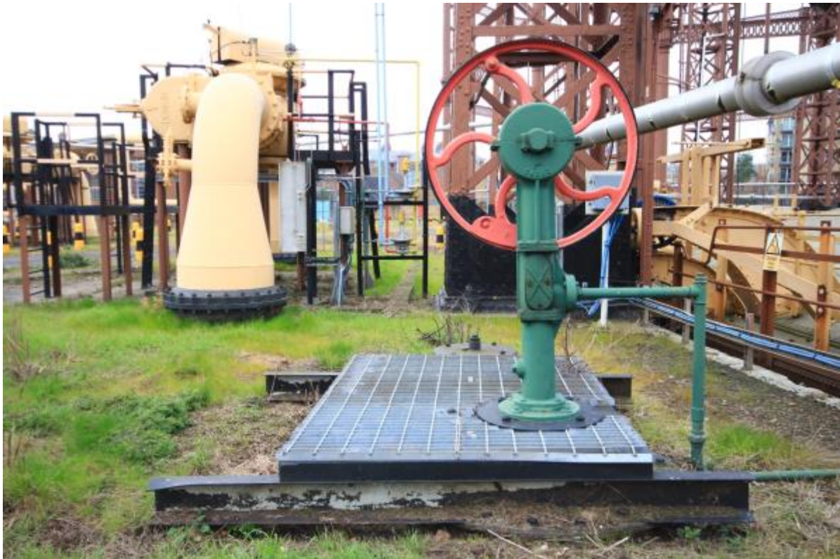
Plate 53: Siphon pit, pump, and governor beyond, Gasholder No. 5 (MRA16-0309)
