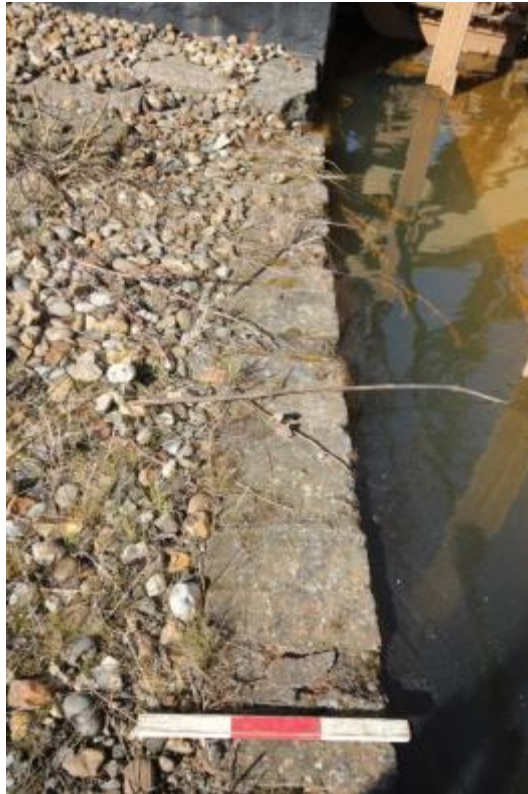
Plate 29: Brick tank to Gasholder No. 2 (MRA16-0161)
