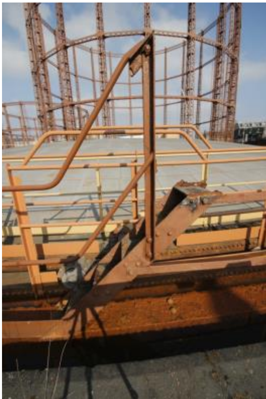
Plate 13: Remnant stair section (MRA16-0026)
