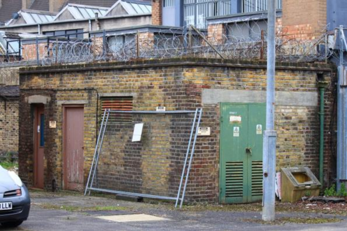
Plate 63: Electrical Substation (MRA16-0374)
