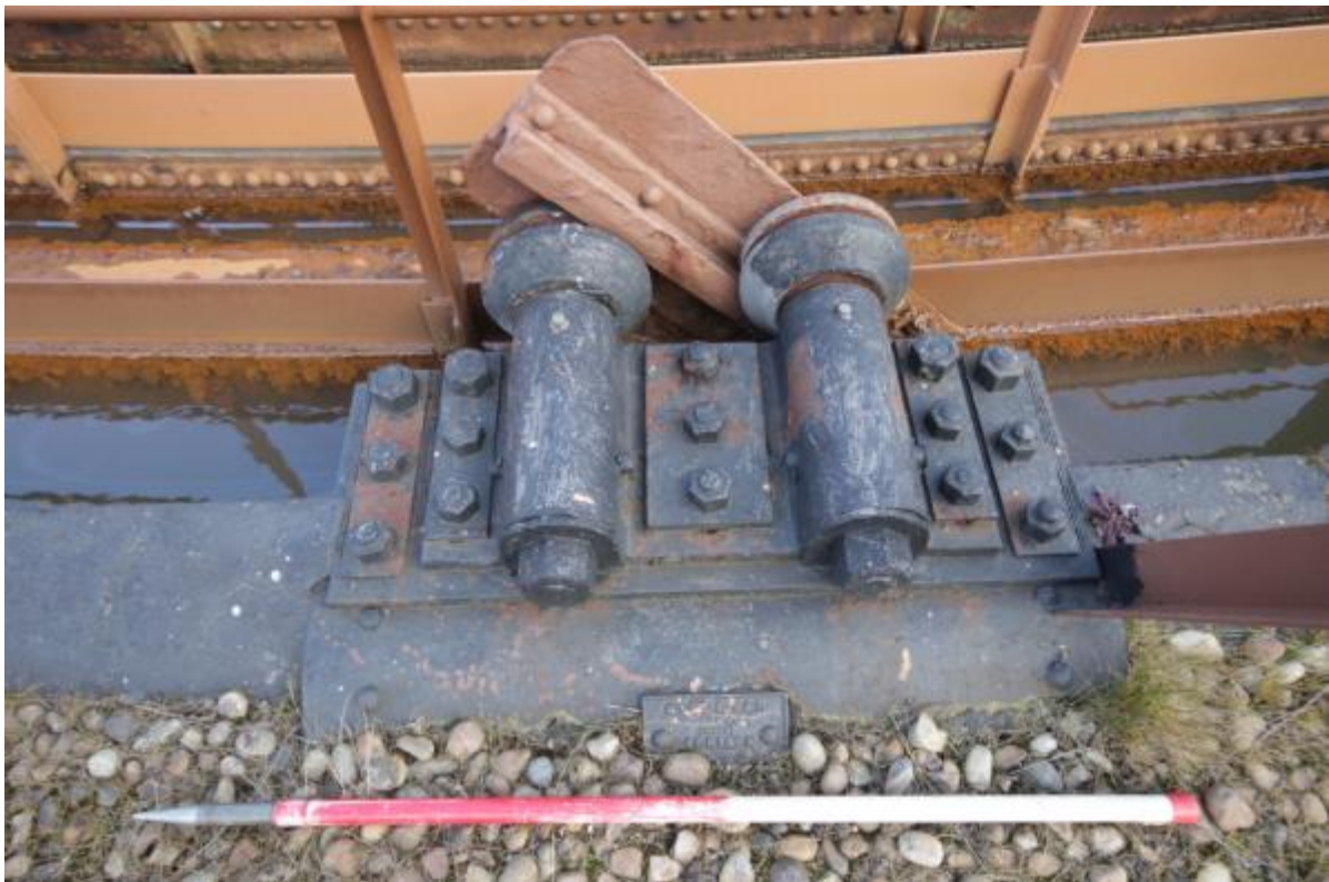
Plate 11: Guide carriage to outer lift (MRA-0061)
