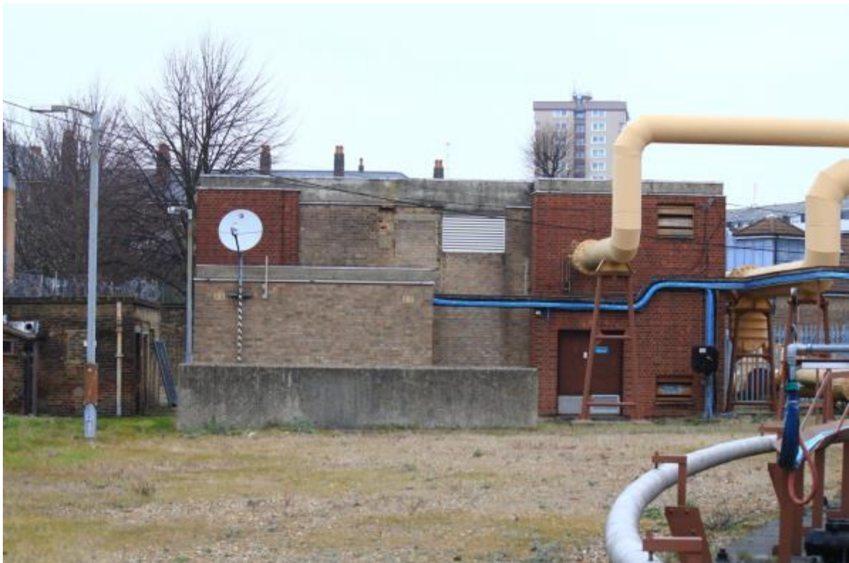
Plate 60: The Gas Pumping Plant Building (MRA16-0367)
