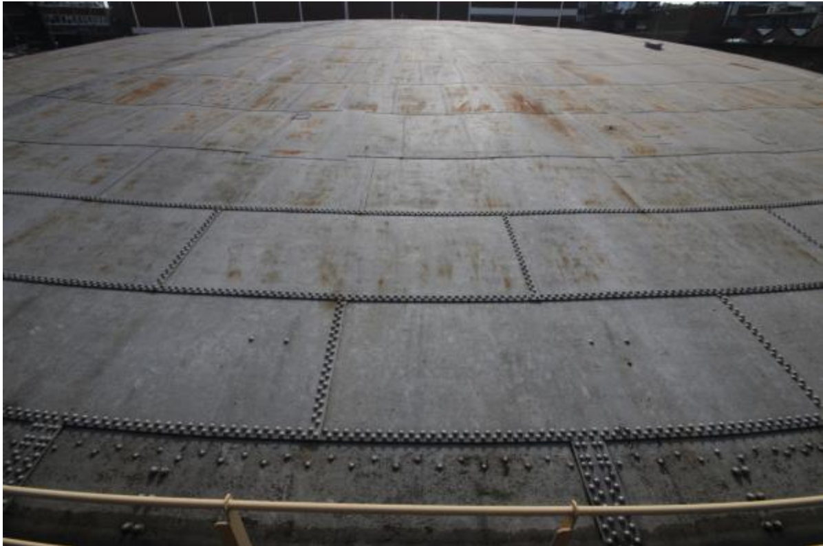
Plate 18: Crown detail, Gasholder No. 4 (MRA16-0099)
