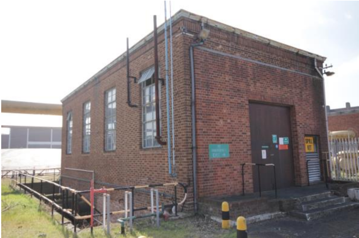
Plate 55: The Valve House (MRA16-0122)
