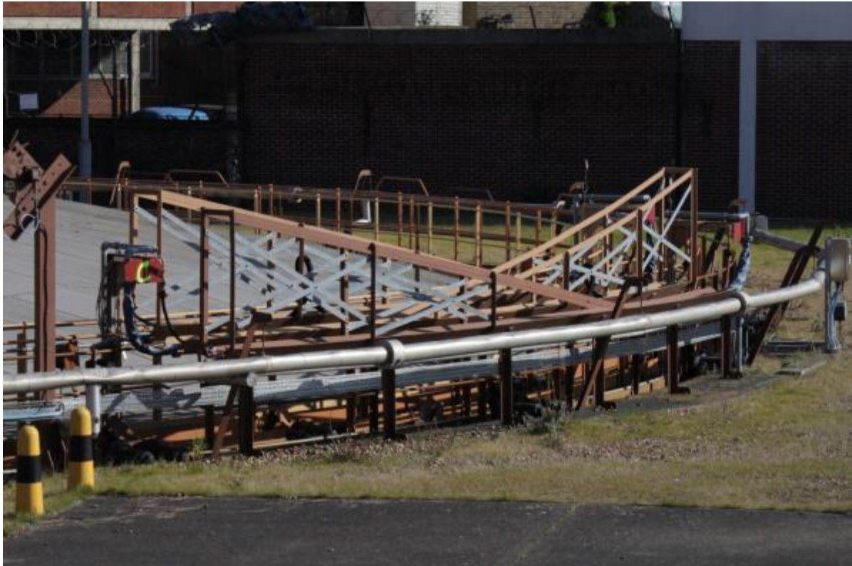
Plate 6: Hose guides (MRA16-0229)
