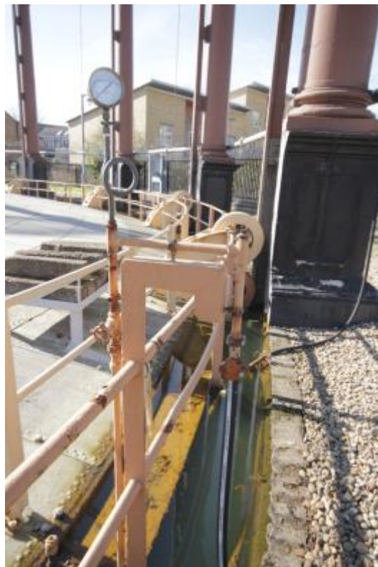
Plate 37: Hose guide, Gasholder No. 2 (MRA16-0186)
