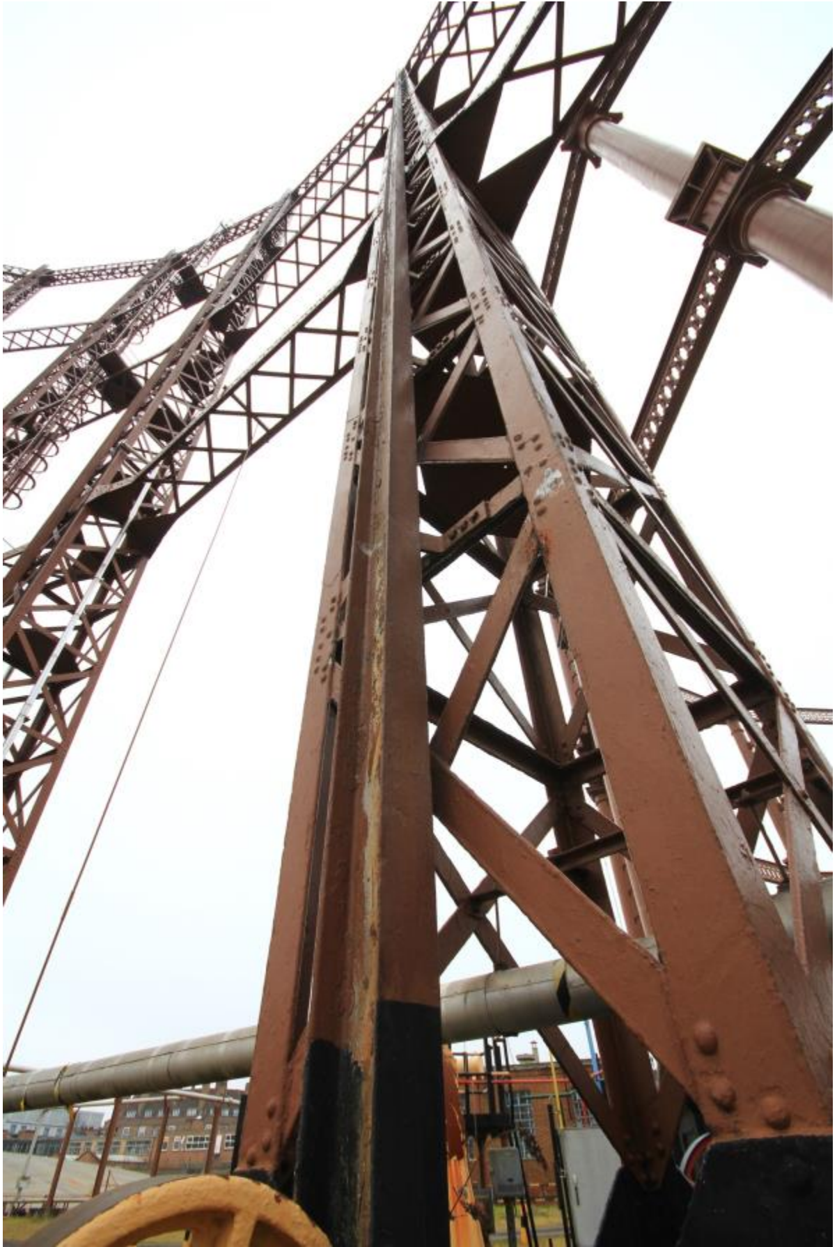
Plate 47: Guide rail, Gasholder No. 5 (MRA16-0257)
