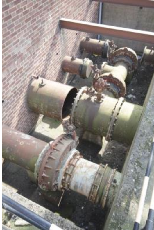
Plate 57: Pit to the west of the Valve House (MRA16-0113)
