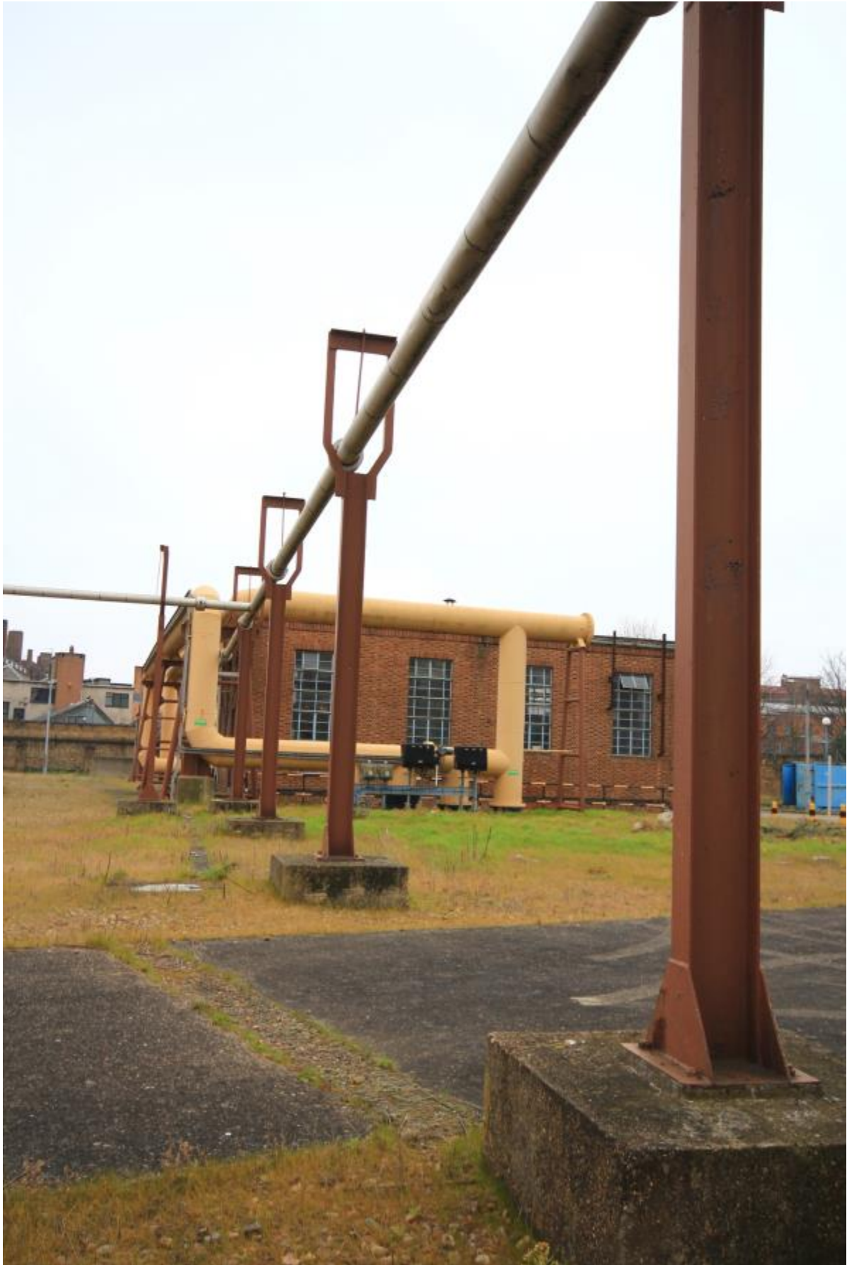
Plate 61: Piping from gasholders emerges to the east of the Valve House, while piping for the antifreeze system runs overhead (MRA16-0321)
