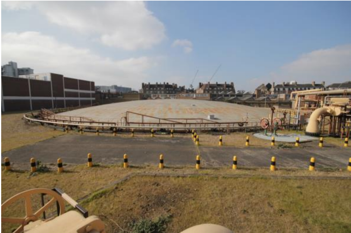
Plate 16: Gasholder No. 4 (MRA16-0057)
