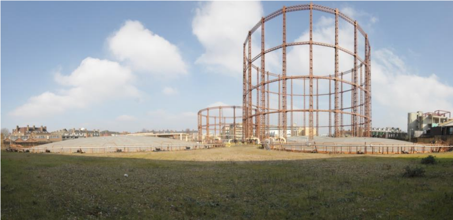
Plate 1: Overview of the site, with Gasholders No. 1 and No. 4 in the foreground, and No. 2 and No. 5 beyond (MRA16-0402)
