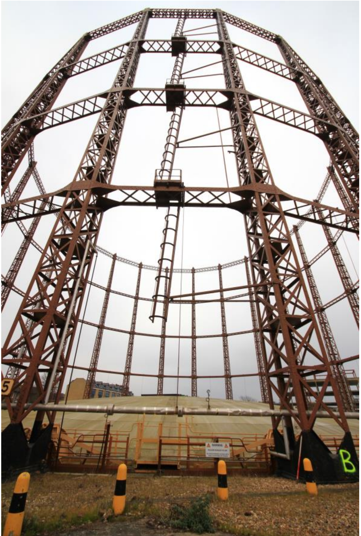
Plate 52: Ladders, Gasholder No. 5 (MRA16-0327)
