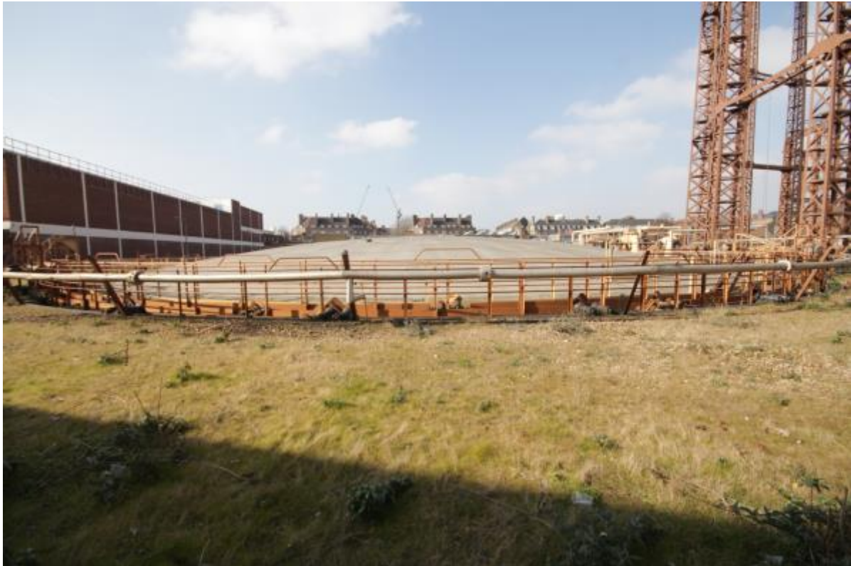
Plate 2: Gasholder No. 1 (MRA16-0031)
