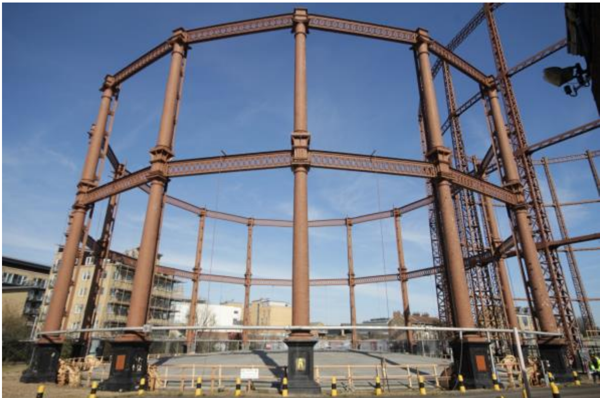
Plate 28: Gasholder No. 2 (MRA16-0154)
