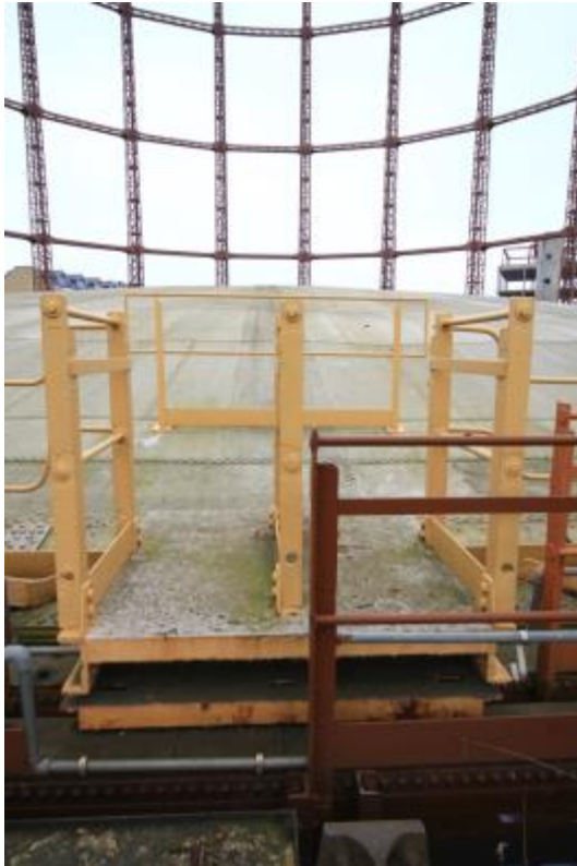
Plate 44: Crown bridge Gasholder No. 5 (MRA16-0322)
