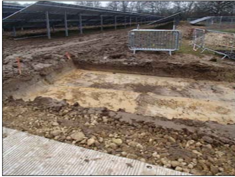
Fig. 3a West facing photograph of transformer foundation trench
