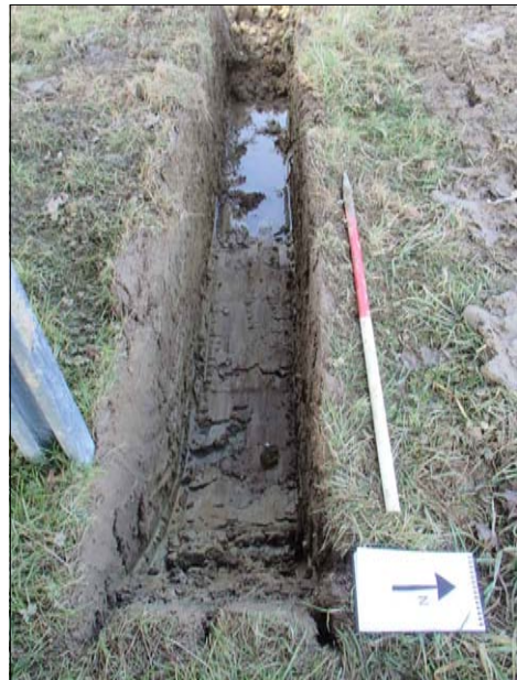
Fig. 3d west facing photo of Earthing cable trench 65
