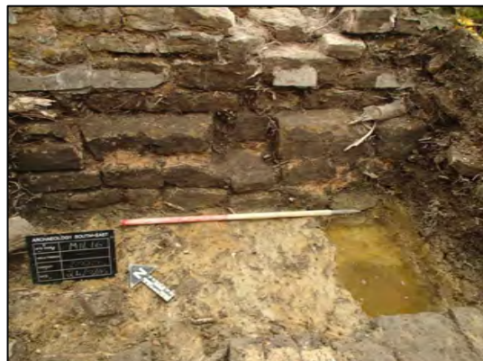
Foundation structure 3005 looking north-east
