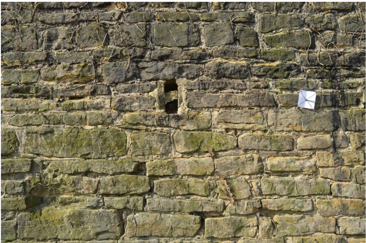
Plate 4: Detail of the stonework and the lime mortar composition, Elevation 7 (6948_0023)
