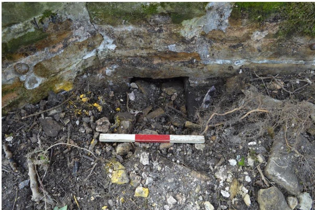
Plate 19: Detail of the opening within the south-west corner of the mill, possible drainage channel or ventilation shaft, Elevation 2 (6948_0036)
