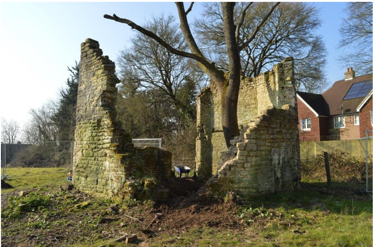
Plate 10: Location of former doorway to the loading bay at first floor level, Elevation 5 (6948_0016)
