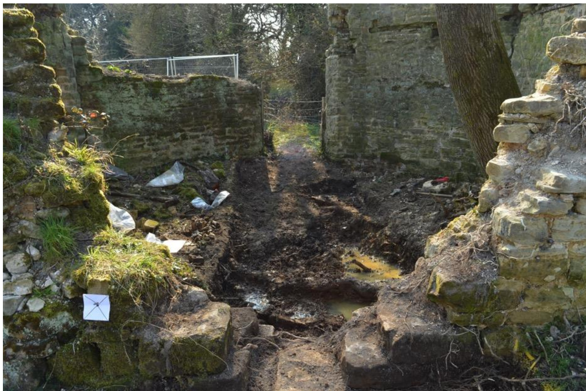
Plate 15: General layout of the mill's interior, facing south (6948_0066)
