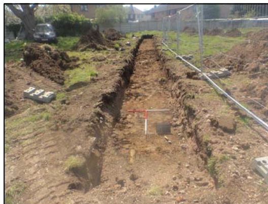
Trench 4 looking southwest
