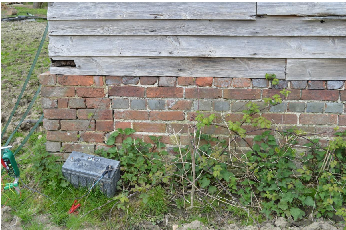
Plate 14: Brick plinth wall and straight joint at south-east corner of barn, looking west (11)
