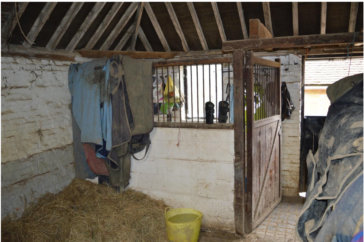
Plate 22: Interior of stable, looking east (22)
