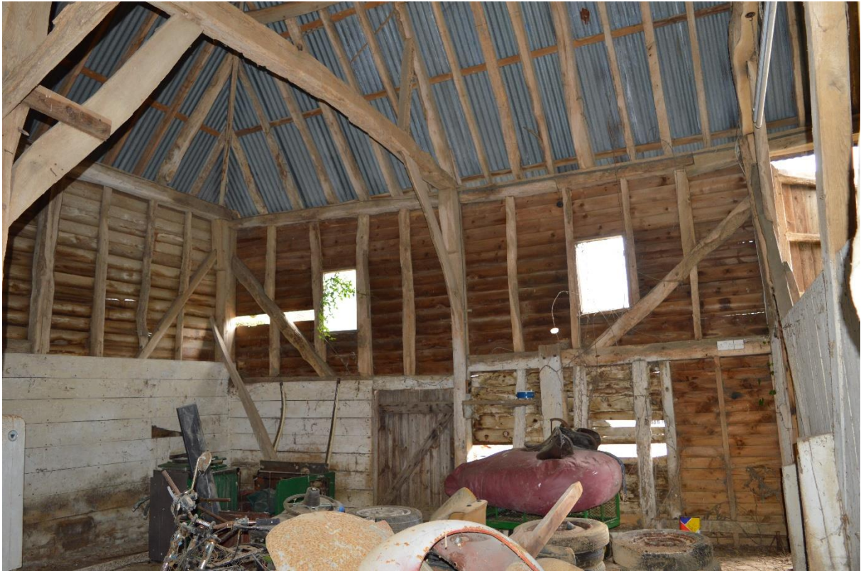
Plate 13: Interior of cow house, looking north (61)
