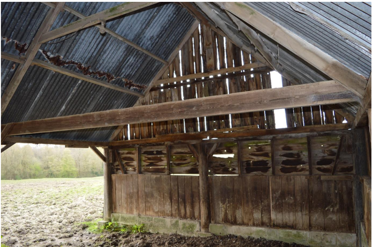
Plate 16: Interior of cattle shelter, looking south-east (14)
