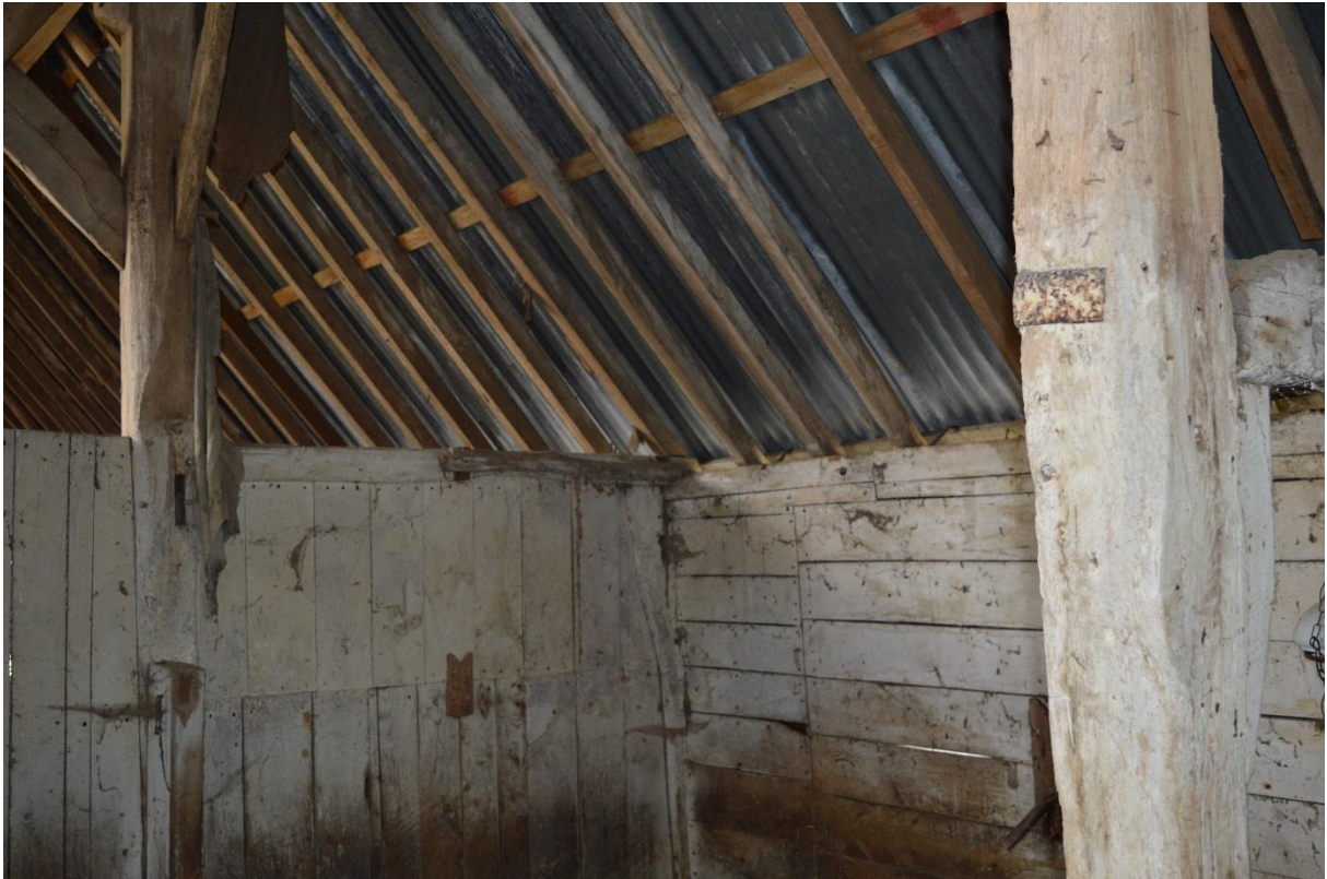
Plate 7: Empty mortice on arcade post of Truss 4, looking south-east (64)
