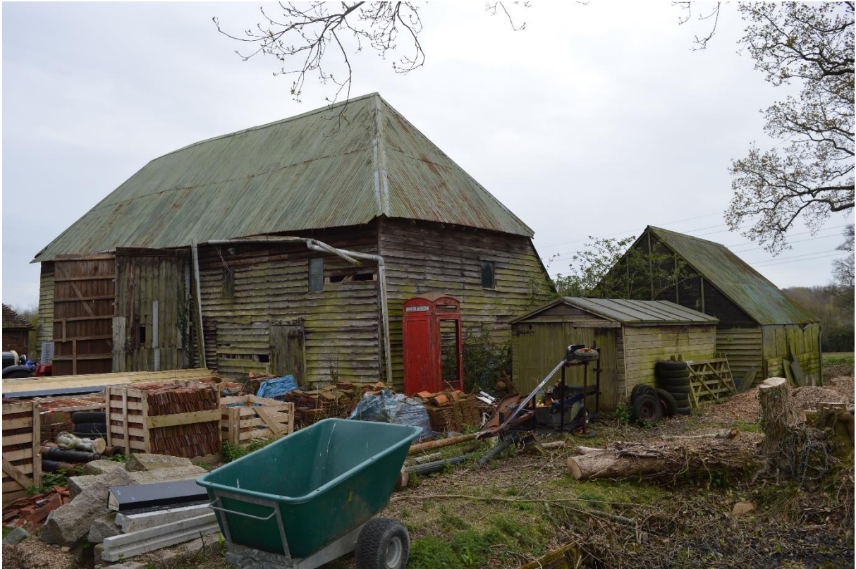
Plate 1: The barn, looking south-east (4)
