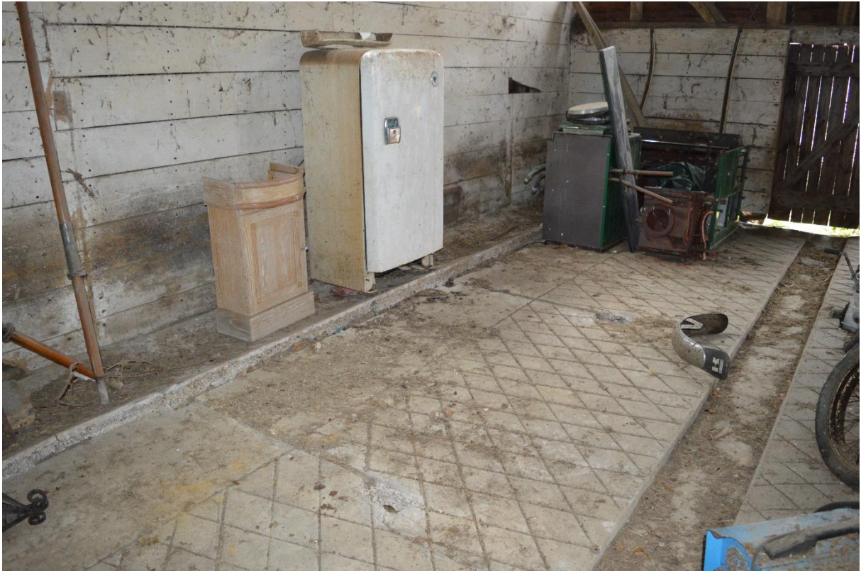
Plate 15: Concrete floor in cow house, looking north-west (77)
