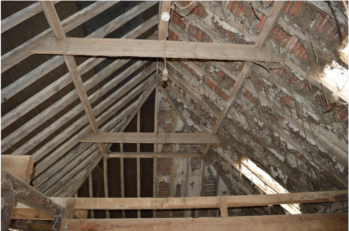
Plate 21: Stable roof, looking south (23)
