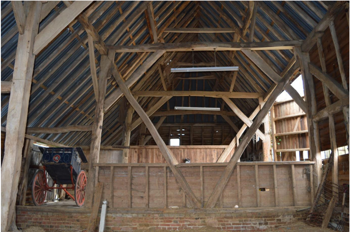
Plate 3: Interior of barn, looking west (47)
