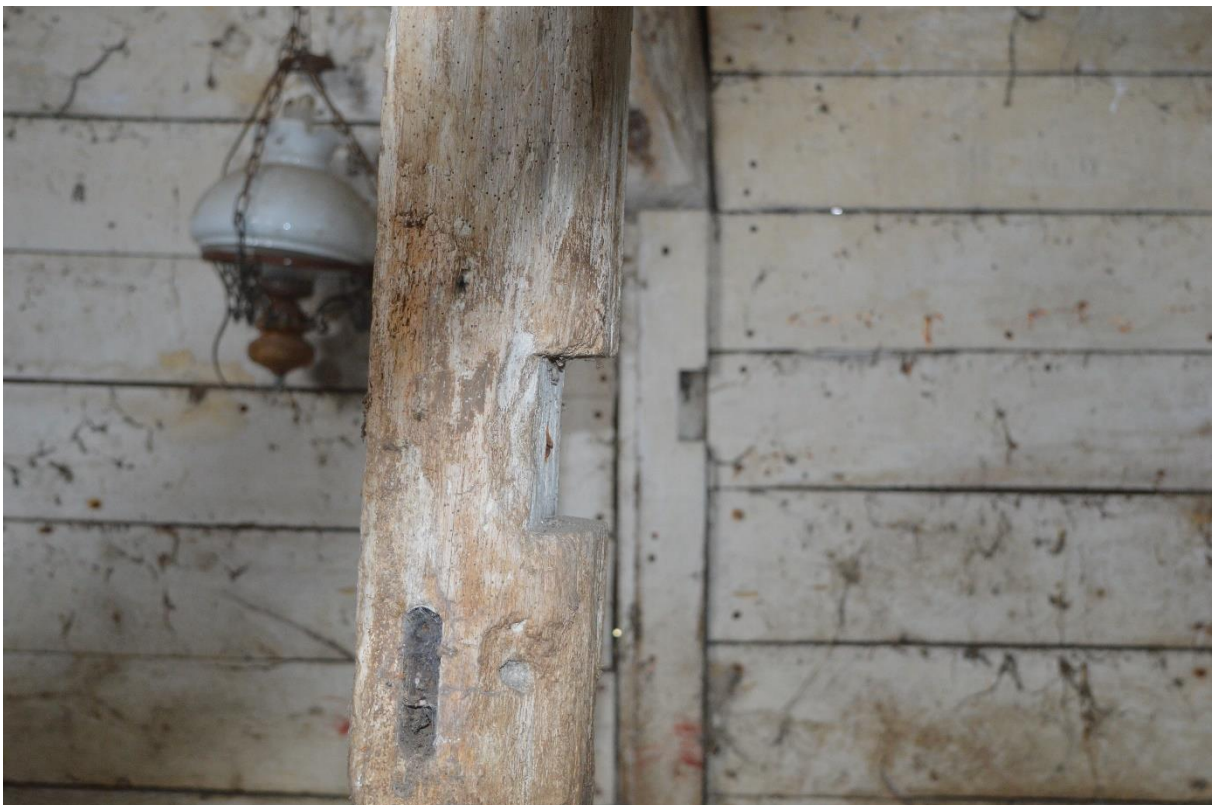
Plate 12: Empty mortices for inserted partition at Truss 5, looking south (73)
