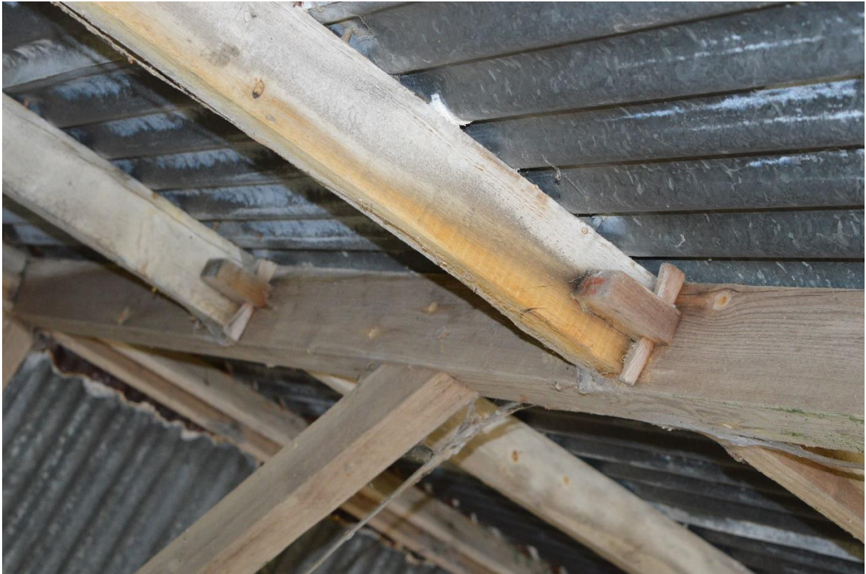
Plate 17: Cattle shelter purlins jointed to rafter with through tenon and key (85)
