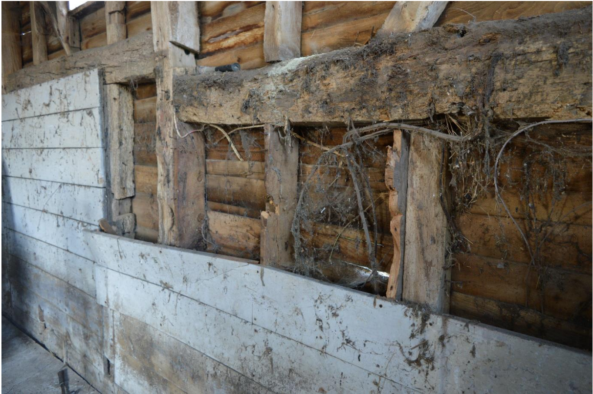
Plate 23: Elm boarding and underlying studwork, looking south-west (100)
