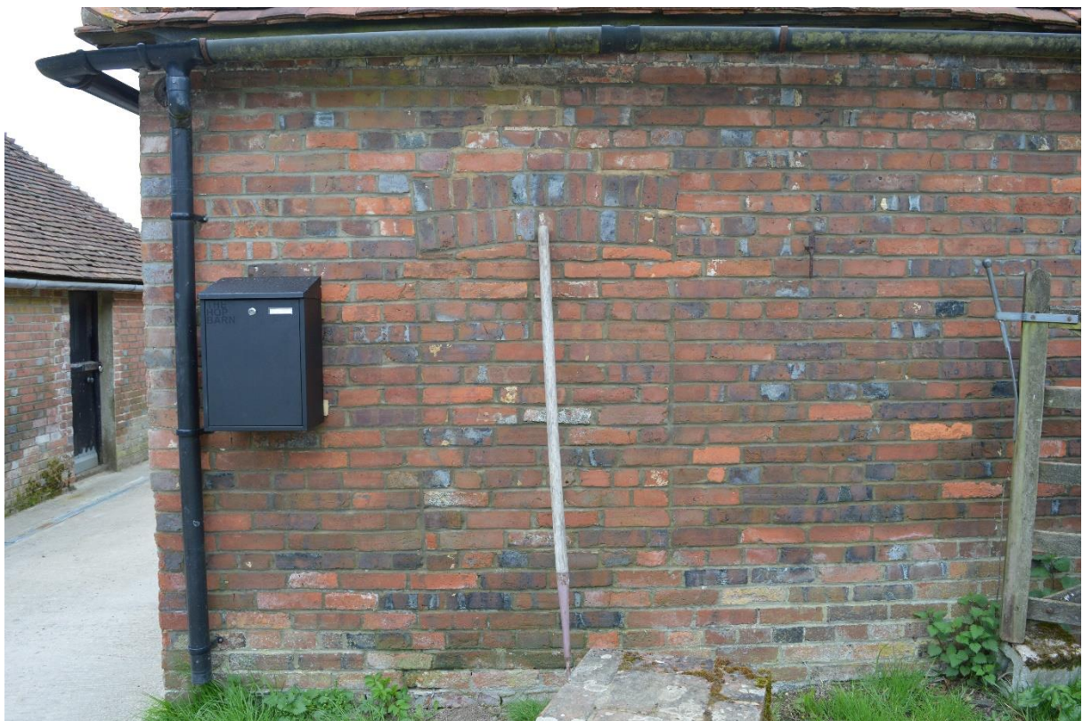
Plate 20: Blocked opening on north elevation of stable (20)
