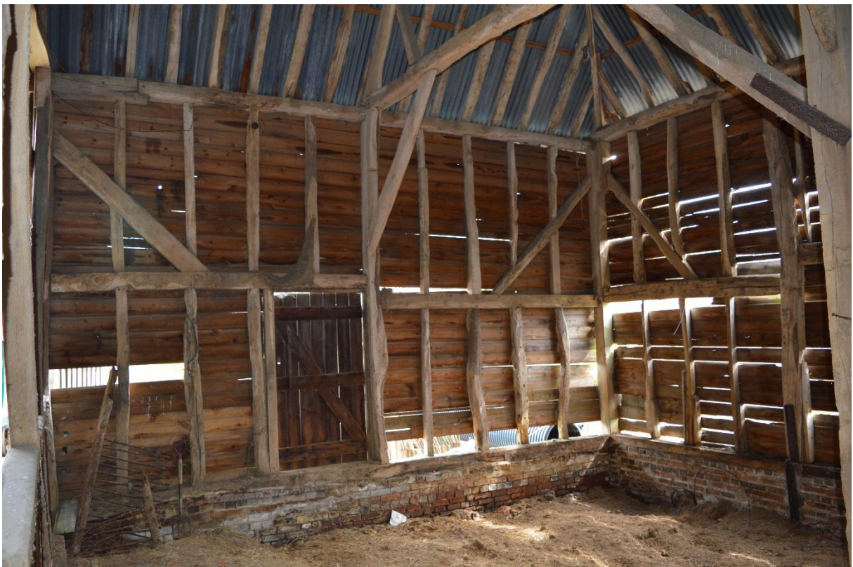
Plate 4: Interior of barn, looking north-east (41)
