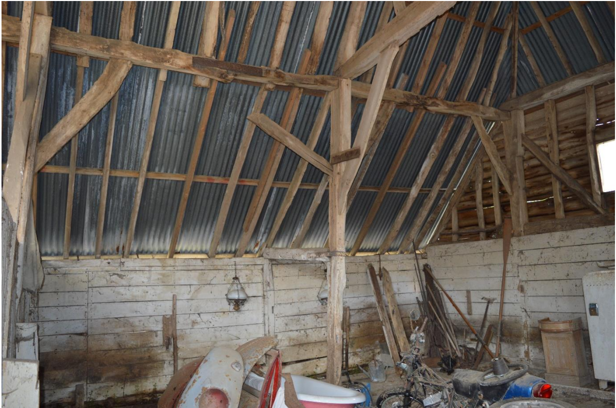
Plate 11: Boarded walls in converted cow house, looking south (56)
