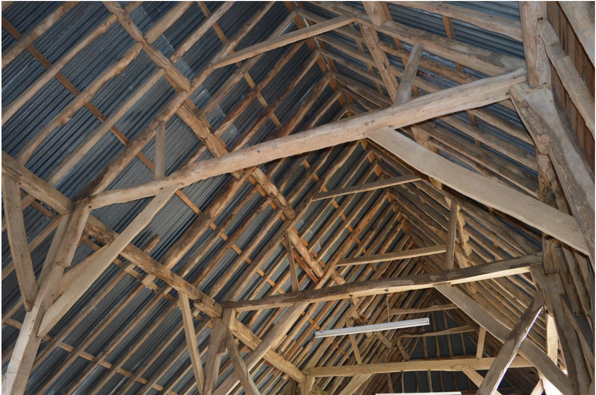
Plate 5: Barn roof, looking west (51)
