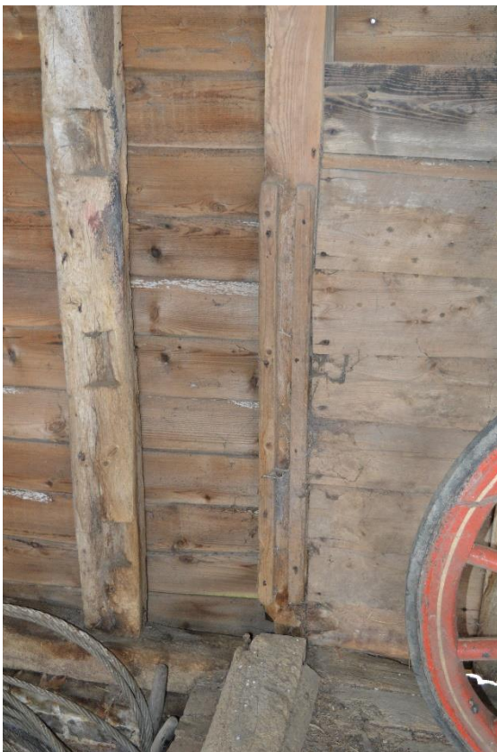
Plate 10: Groove for removable partition at Truss 3, looking south (40)
