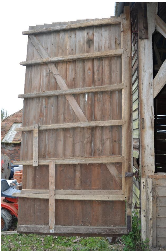
Plate 8: Midstrey door on north side of barn, looking east (33)
