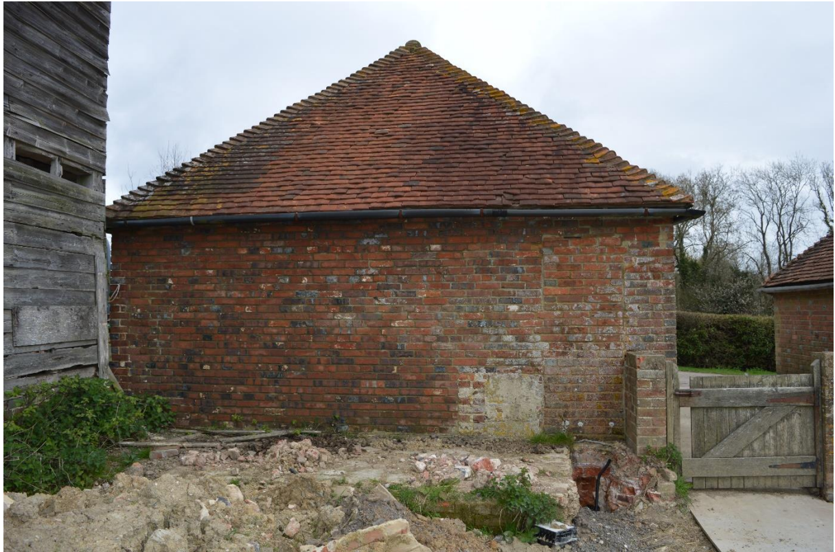
Plate 19: South elevation of stable with remains of lean-to and blocked openings (10)
