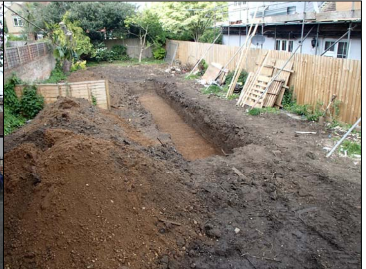
The trench within the site, looking north
