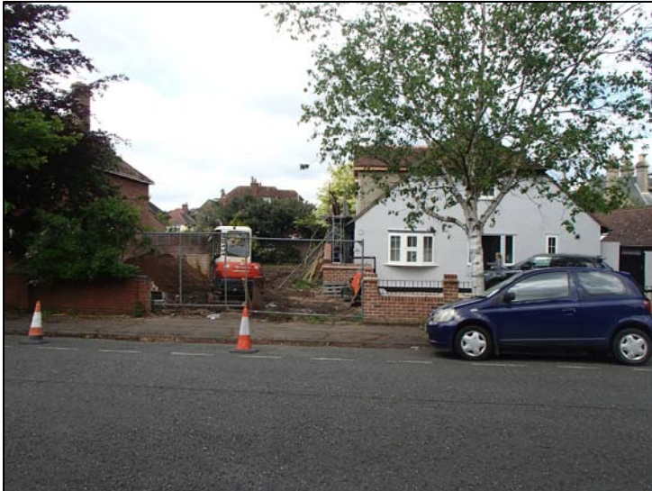
The site from Cambridge Road, looking north-west
