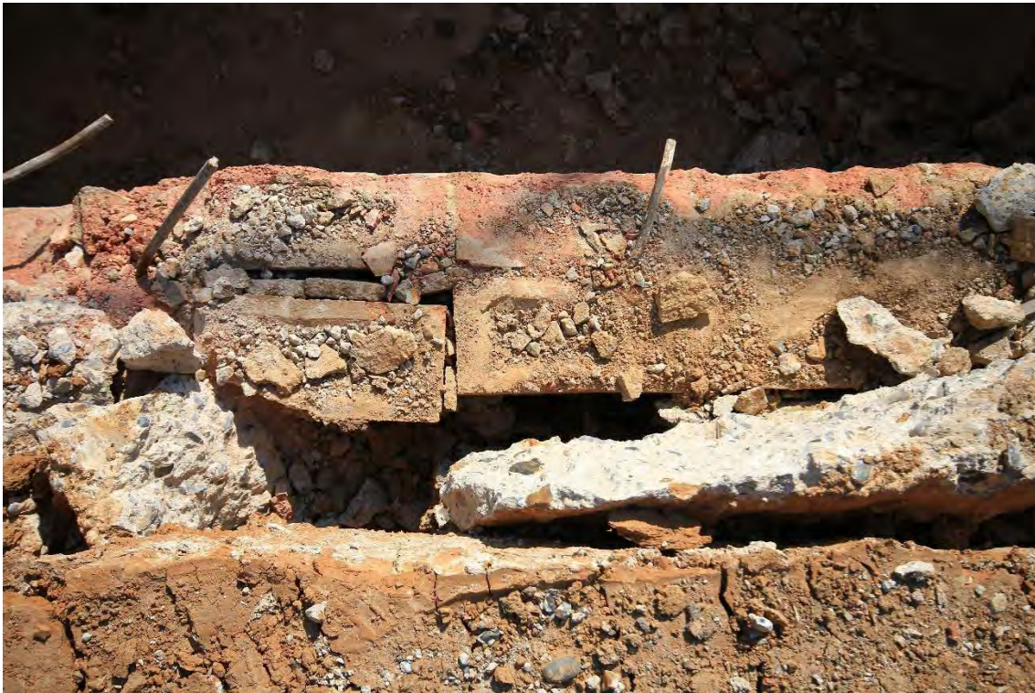
Plate 13: Shelter 4, western wall of the west gallery, note: combined brick and concrete construction, facing east (down) (7)
