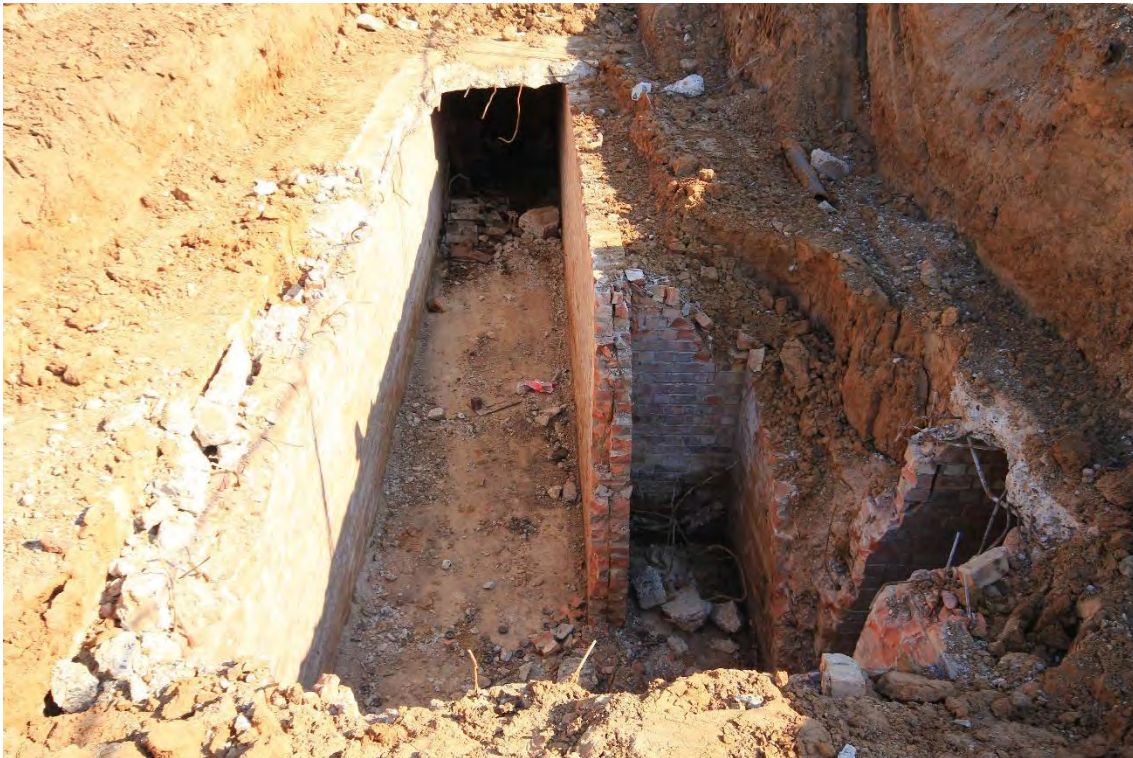
Plate 11: Shelter 4, west gallery viewed from ground level, facing north (9)
