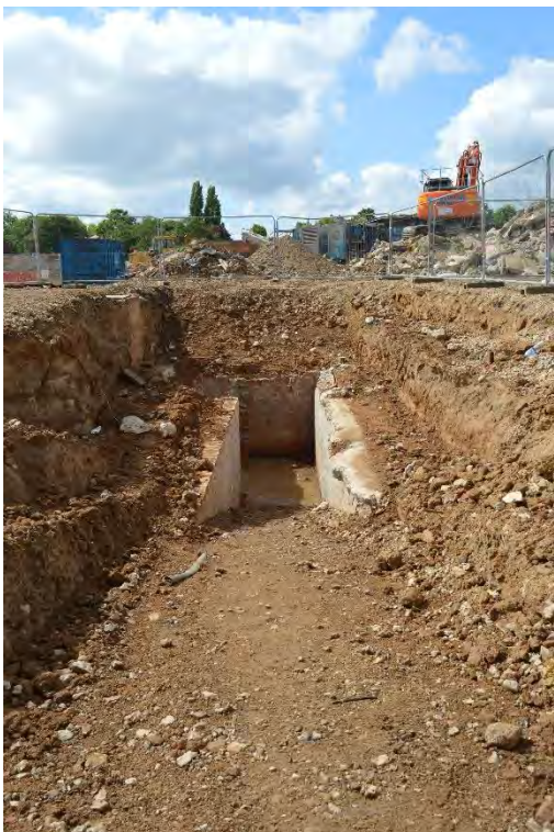
Plate 2: Shelter 4, west gallery following asbestos removal works, facing south (41)
