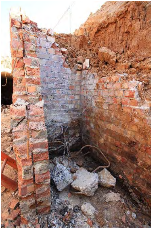
Plate 27: Shelter 4, view of the south-west chemical closet, facing north-east (32)
