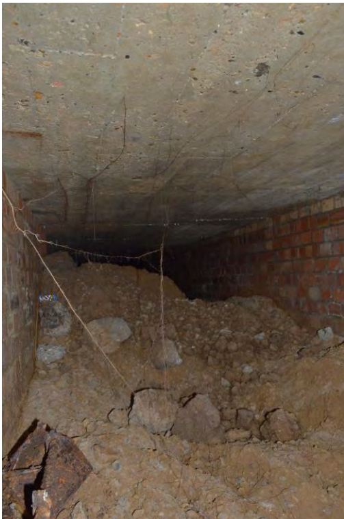
Plate 4: Shelter 4, east gallery, facing north (74)
