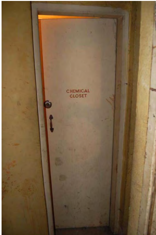
Plate 33: Shelter 1, example of a lightweight timber board door used to separate a chemical closet within Shelter 1 from the passage (FAU 2008, 41)
