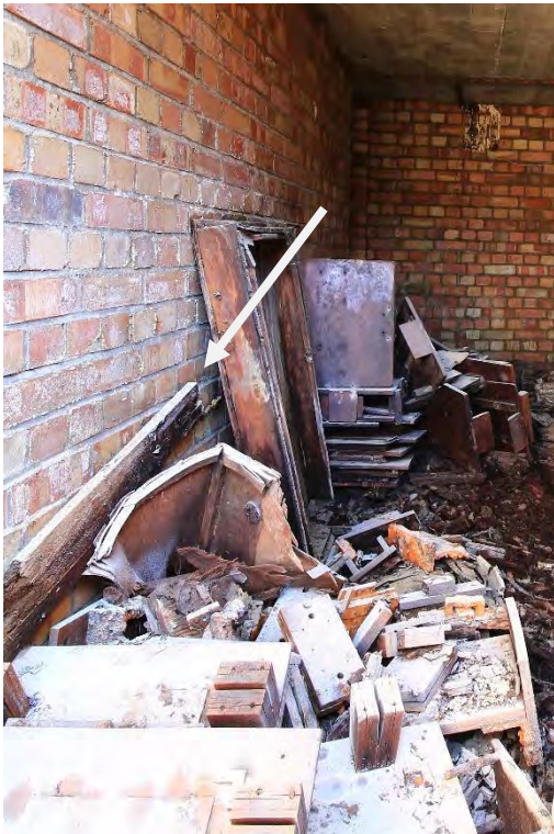
Plate 17: Shelter 4, retained wall-mounted timber seating within the west gallery, facing north (27)
