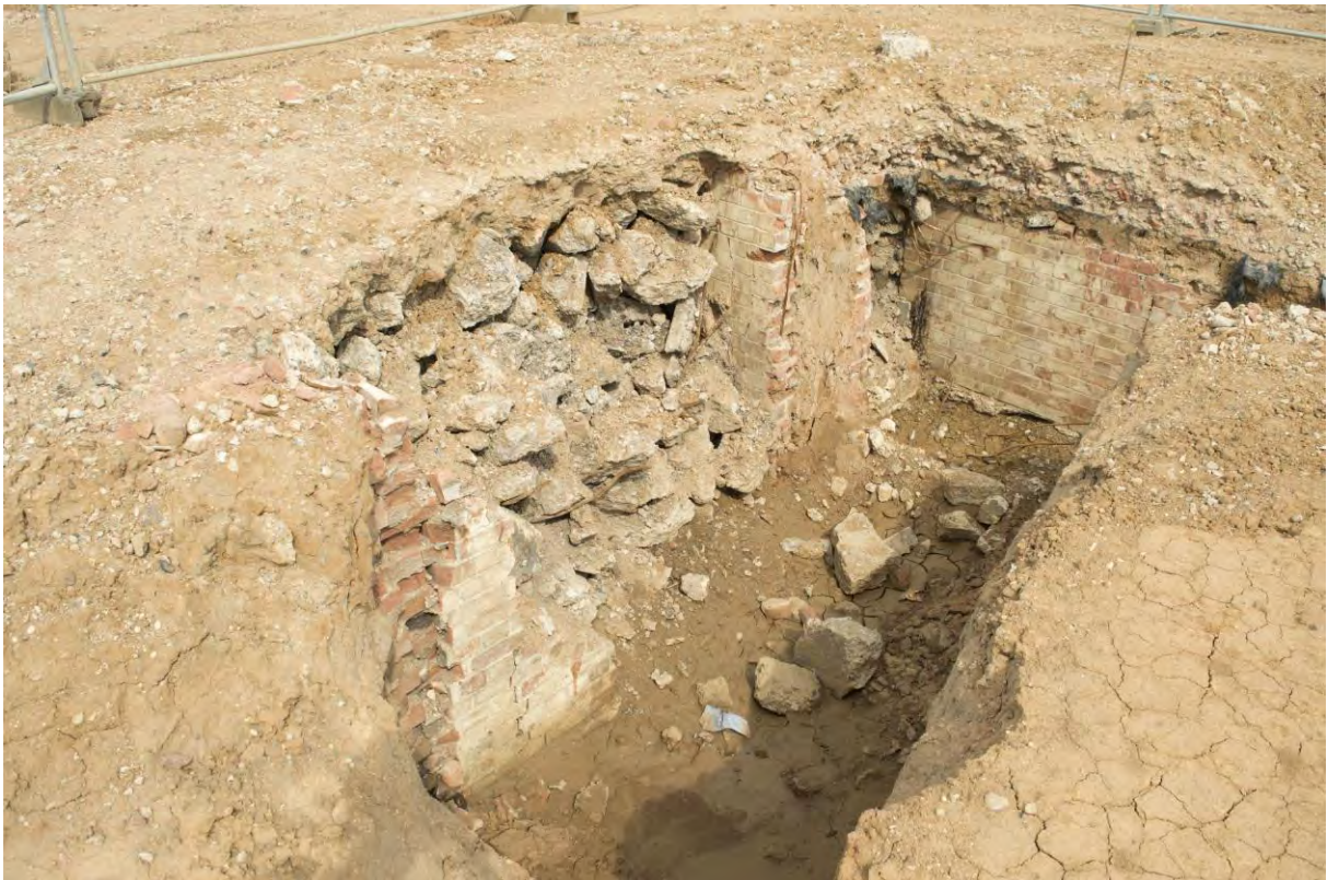
Plate 22: Shelter 4, exposed baffle section of east gallery (the main part of the gallery is backfilled with rubble). Vertical scar in brickwork to the left is from chemical closet wall. Facing north-west (137)
