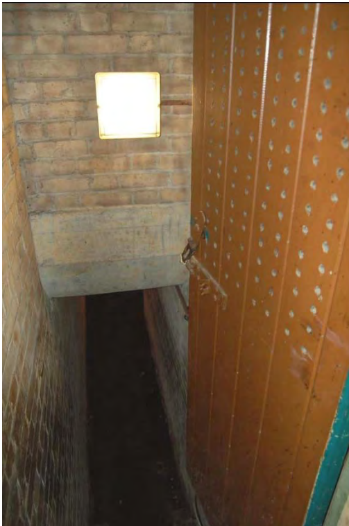
Plate 35: Shelter 3, typical appearance of the ventilated entrance doorway that served Shelter 3 (FAU 2008, 51)
