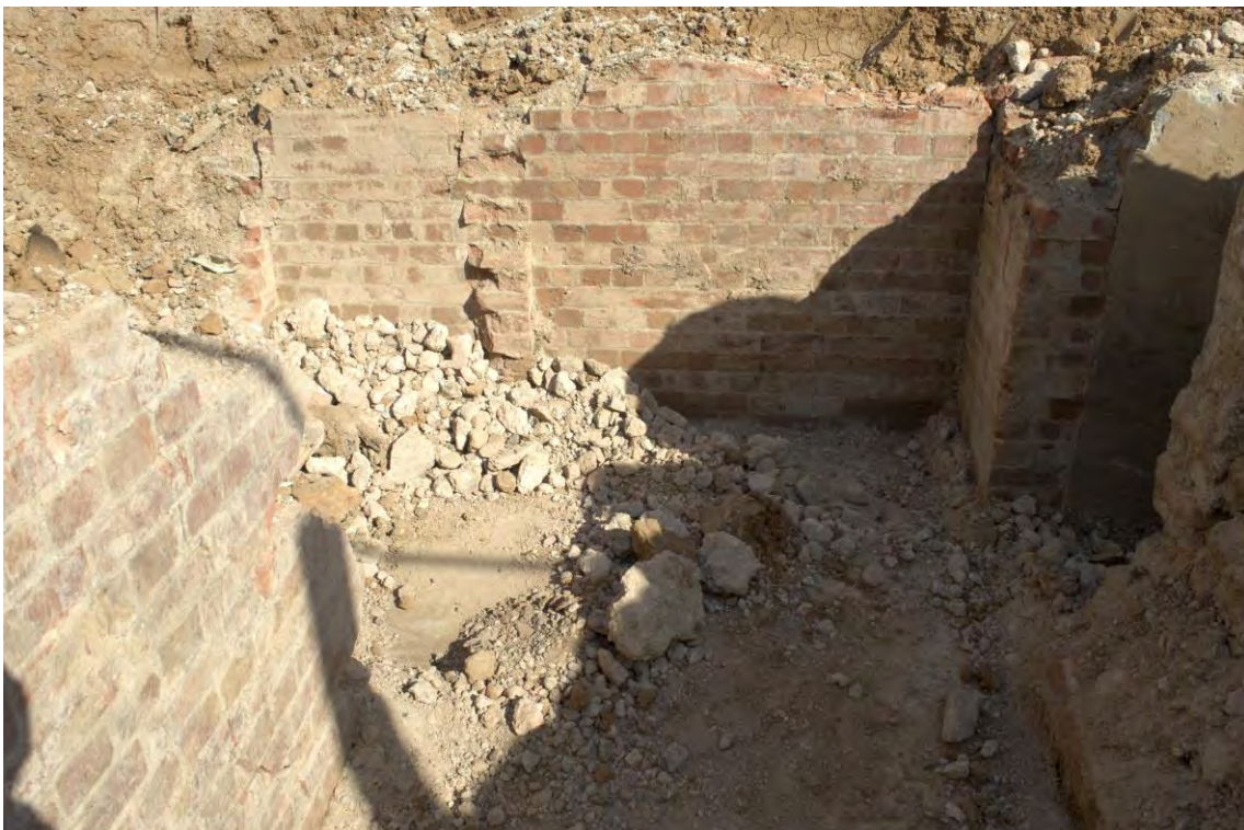
Plate 52: Shelter 5, north end of west corridor with scarring to the wall for a brick partition for chemical/water closet, facing north (87)
