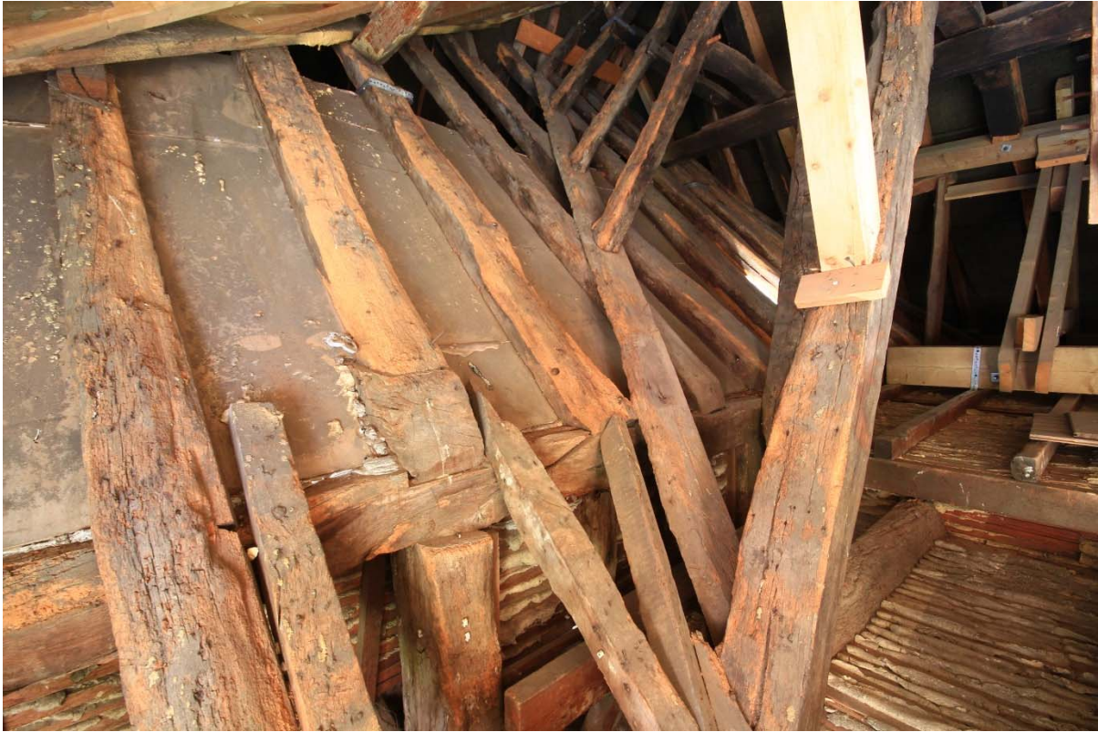
Plate 1: Easily visible intersection of the hall range and crosswing. Note the Trait de Jupiter scarf joint, looking south-west (TRE16-0248)
