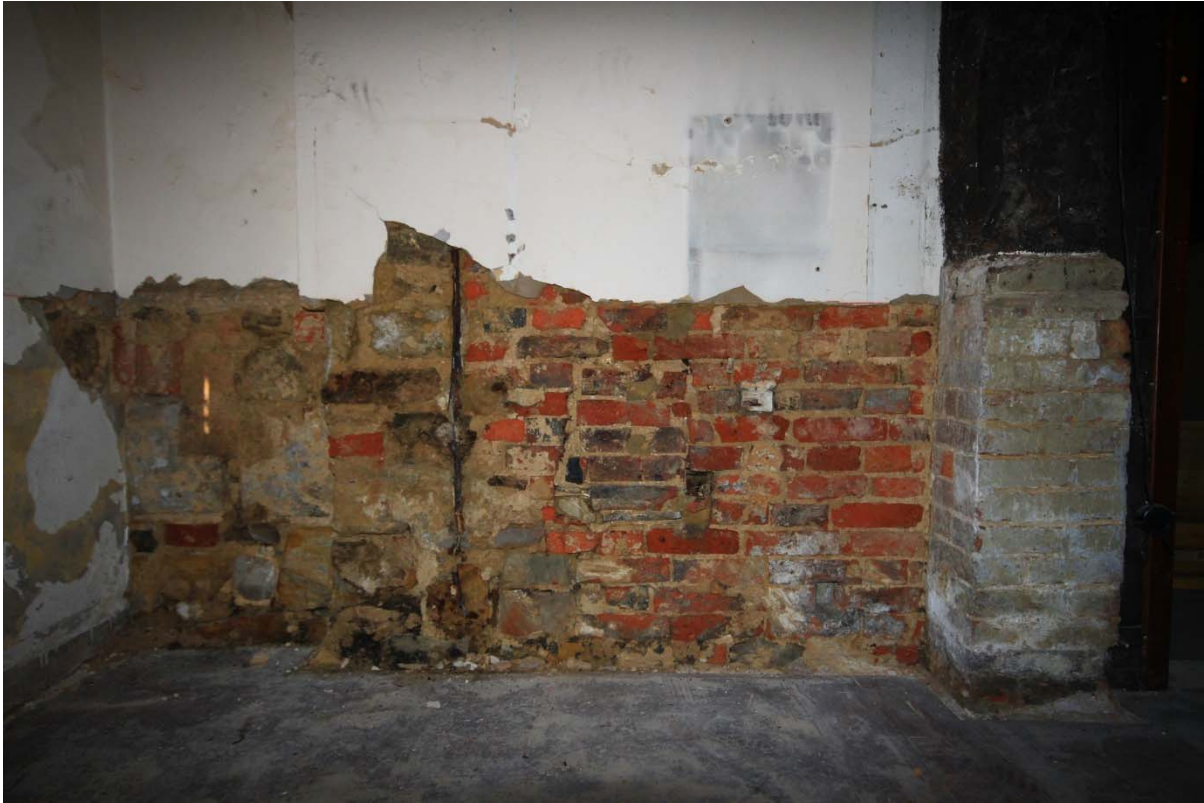
Plate 3: Exposed fabric of west wall of the 18 th -century extension to the south-east of the crossing. The brickwork corresponds with the chimney stack, looking west (TRE16-0284)
