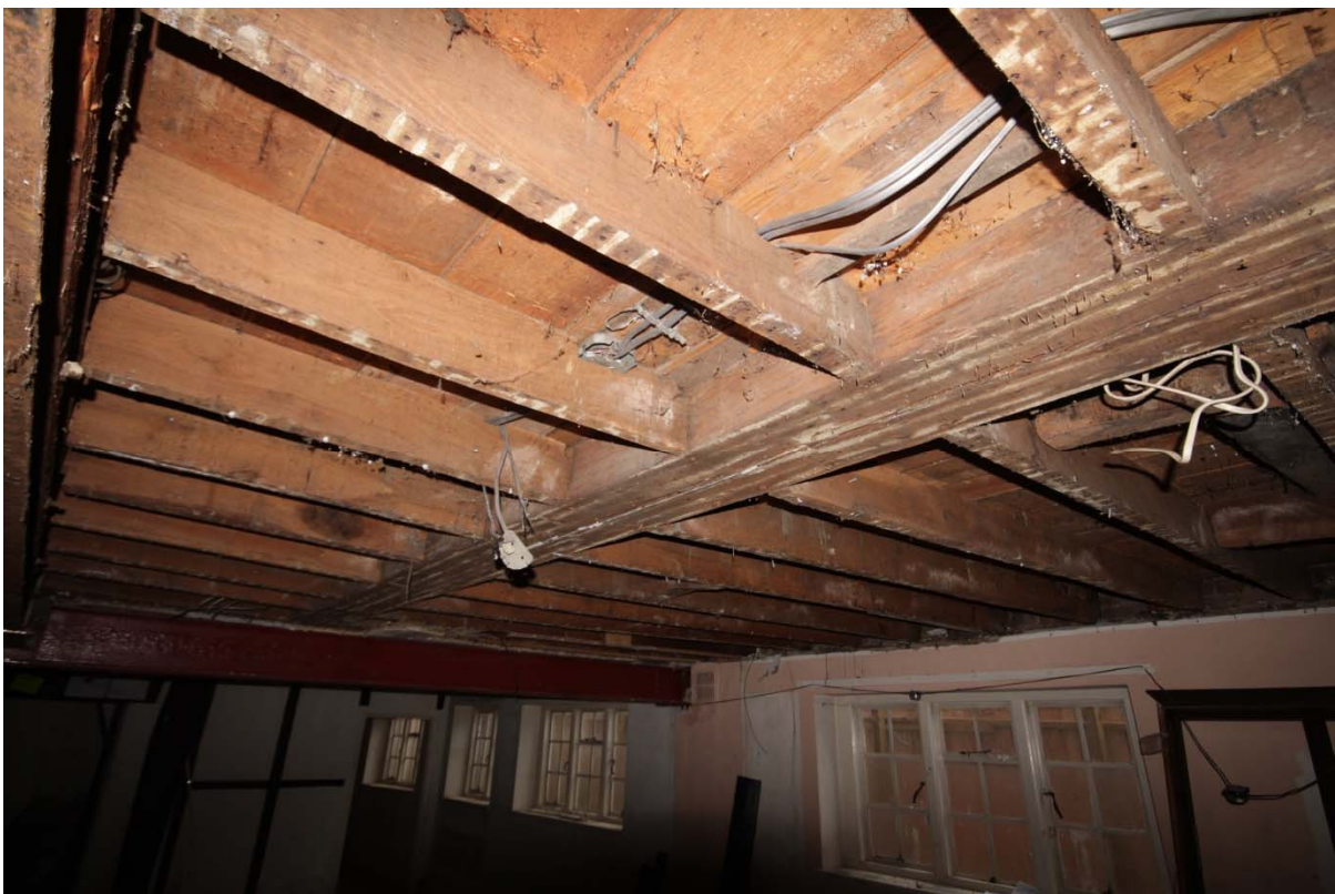
Plate 4: Exposed inserted floor to the hall range, looking south-west (TRE16-0188)
