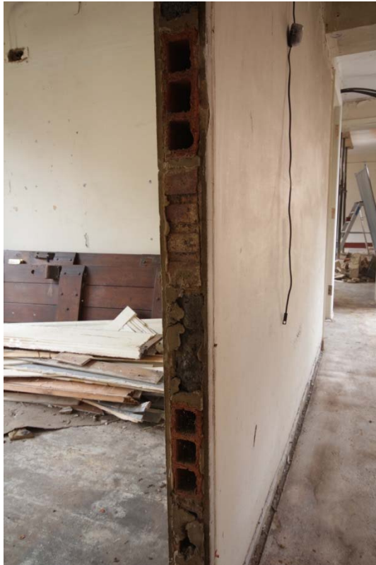
Plate 9: Exposed modern fabric of ground-floor dividing walls, looking north (TRE16-0200)
