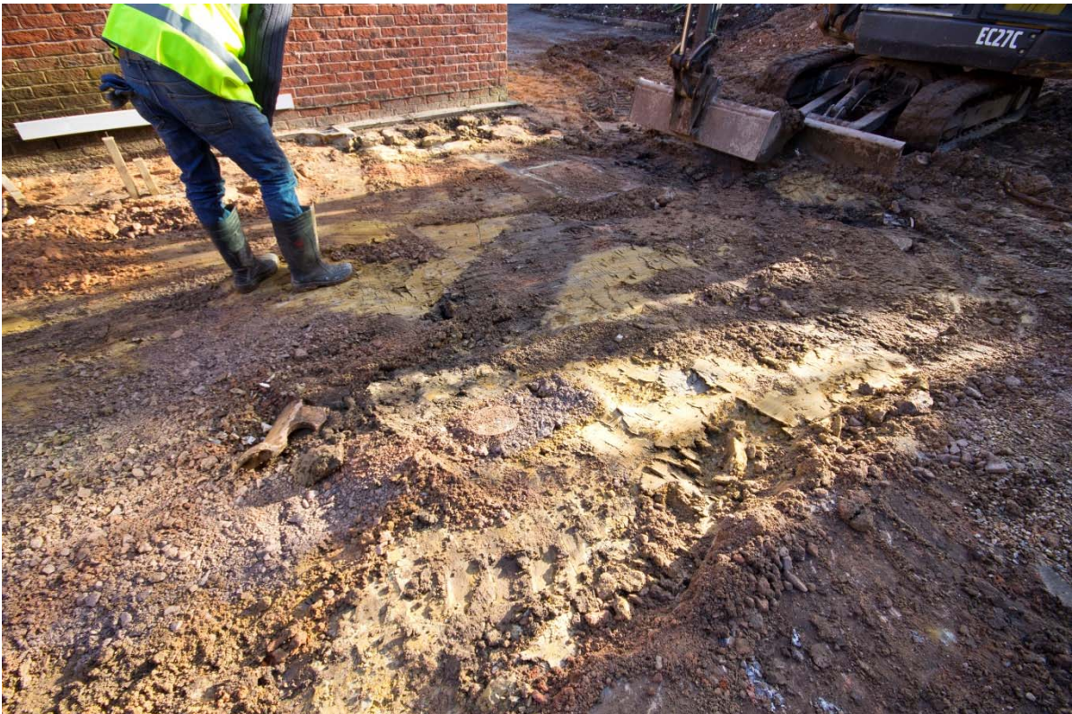
Plate 16: Modern drains cut through the underlying natural, facing south-east (TRE16-0024)
