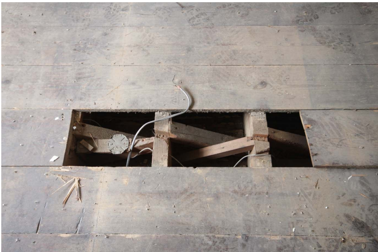
Plate 12: Exposed cross-bracing within the floor of the 1839-74 extension, looking north (TRE16-0214)
