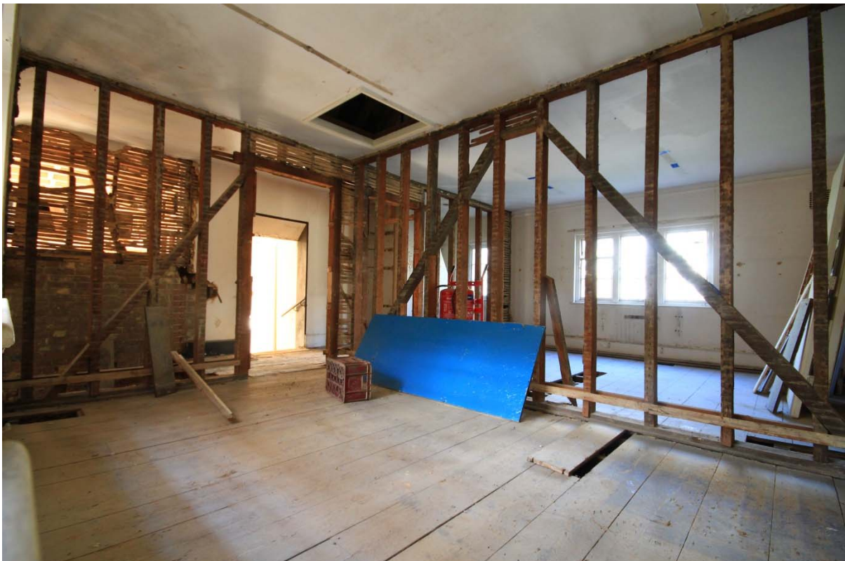
Plate 10: Overview of the revealed studwork on the first floor of the 1839-74 extension, looking southwest (TRE16-0254)
