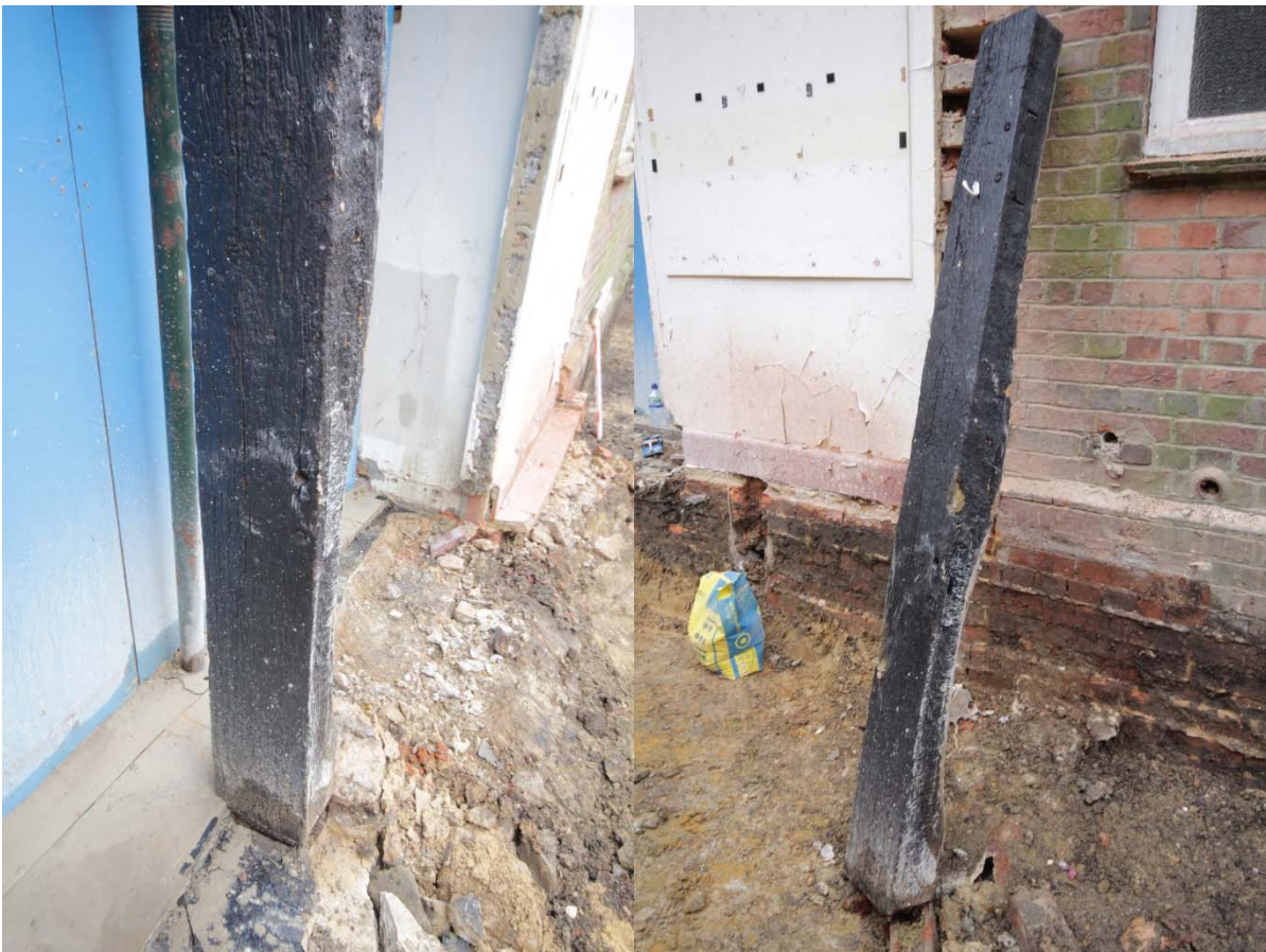
Plate 8: reused timber stanchion in situ and following removal. Notice the peg-holes and mortices (TRE16-0079 and TRE16-0109)
