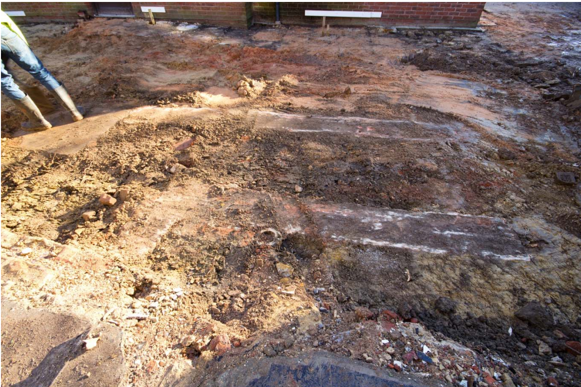
Plate 18: Brick bases to removed 20 th -century ramp, with slab (left) atop well, facing east (TRE16-0003)
