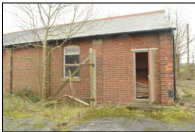
SGA15-0106 Building 27. Facing south
