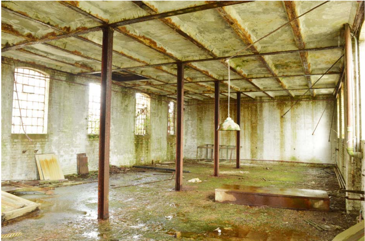
Plate 7 – The saddlery & harness store (Building 22), ground floor, looking north (SGA15-061)
