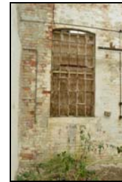
SGA15-0081 Building 25, interior. Facing south
