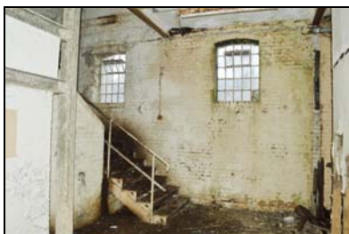
SGA15-0178 Building 28, interior, ground floor. Facing south
