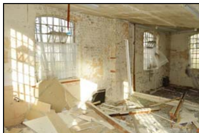
SGA15-0001 Building 29, mobilisation store, interior. Facing north-west
