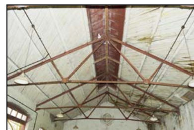
SGA15-0090 Building 26, interior. Facing north-west
