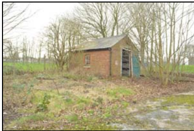
SGA15-0128 Building 30. Facing south-west
