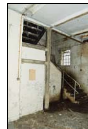
SGA15-0177 Building 28, interior, ground floor. Facing south-east
