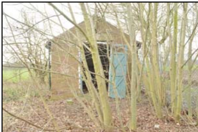
SGA15-0130 Building 30. Facing south
