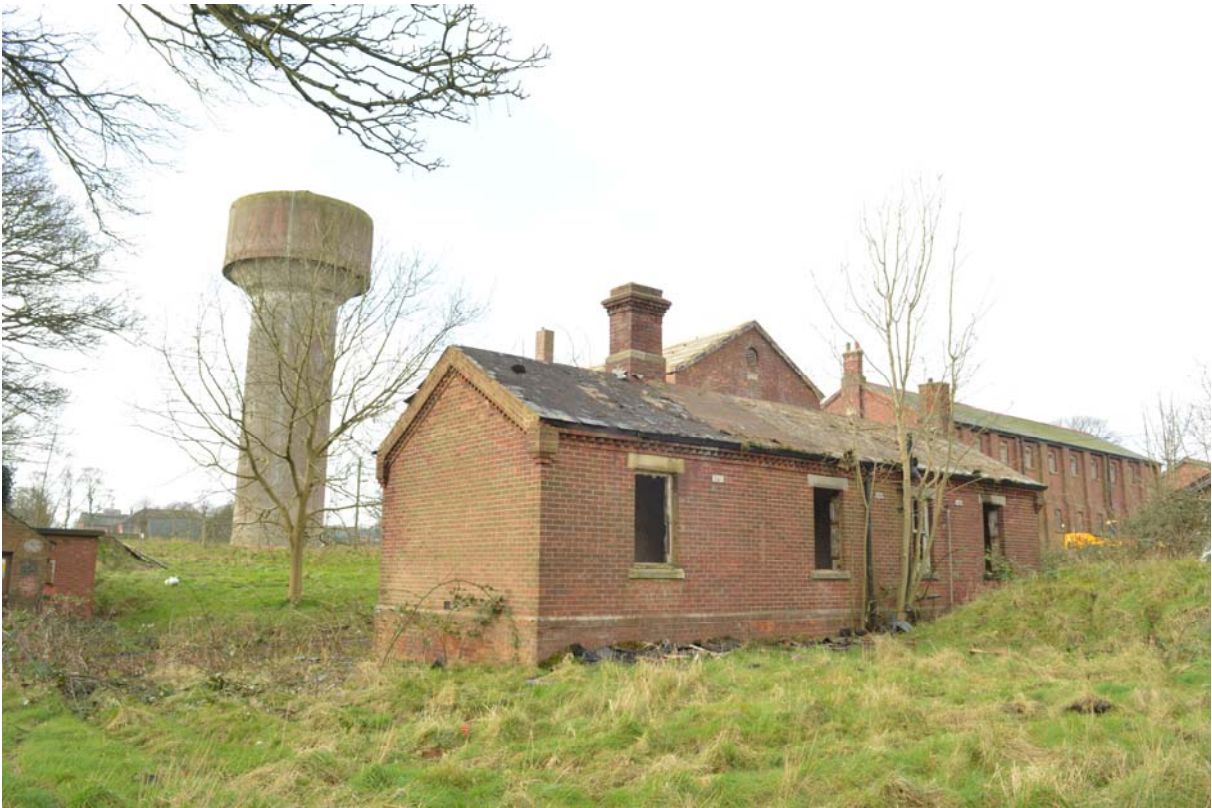
Plate 1 – General view of the site from the entrance gate, south-west (SGA15-010)
