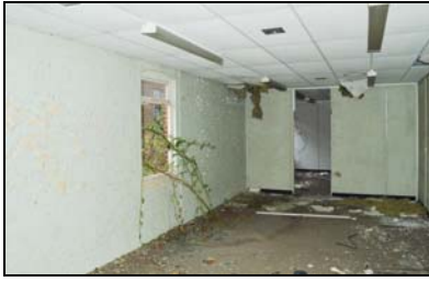
SGA15-0166 Building 27, interior. Facing south-east
