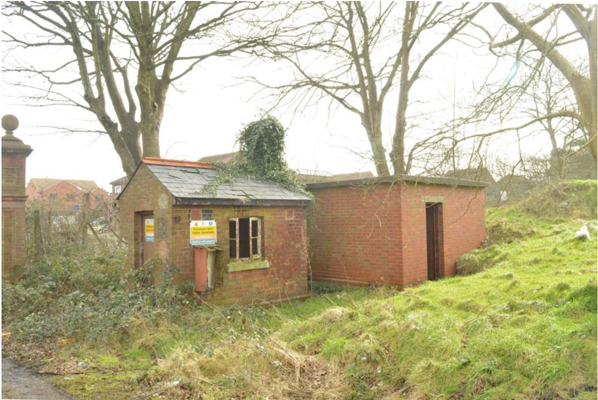
Plate 9 – The sentry hut (Building 23), looking south-east (SGA15-068)
