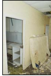
SGA15-0167 Building 27, interior. Facing north-east
