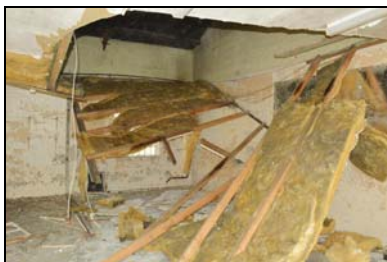
SGA15-0002 Building 29, mobilisation store, interior. Facing north-east
