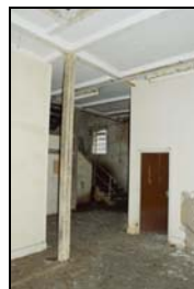
SGA15-0176 Building 28, interior, ground floor. Facing south-east
