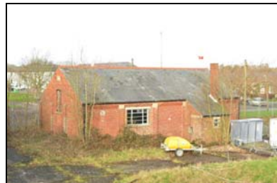
SGA15-0039 Building 32, packing case store. Facing north-west
