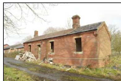
SGA15-0009 Building 24, office. Facing north-west
