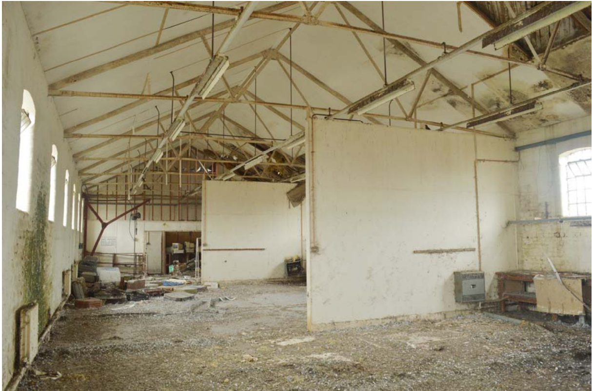
Plate 21 – Equipment store (Building 28), first floor, looking east (SGA15-196)
