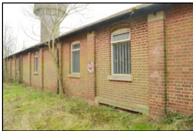
SGA15-0107 Building 27. Facing south-east
