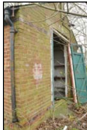
SGA15-0131 Building 30. Facing south-west
