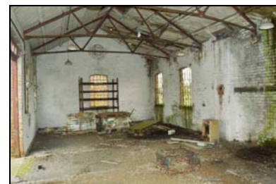
SGA15-0087 Building 26, interior. Facing south-east
