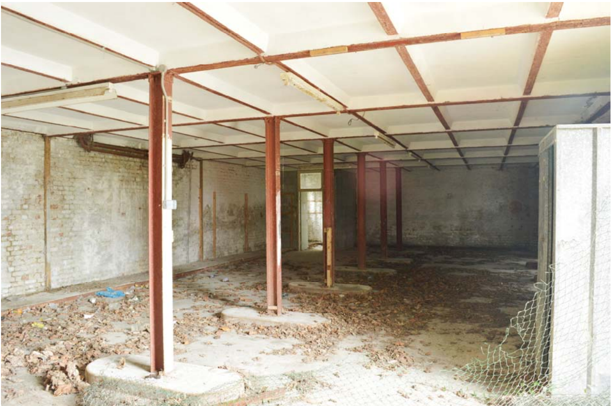
Plate 30 – Equipment store (Building 31), ground floor, looking west (SGA15-201)
