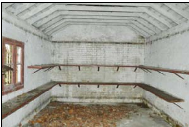
SGA15-0133 Building 30, interior. Facing south
