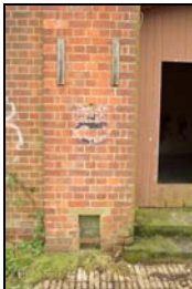
SGA15-0127 Building 28. Facing south
