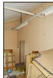
SGA15-0114 Building 27, interior. Facing south-east
