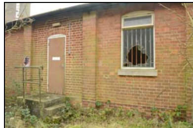
SGA15-0111 Building 27. Facing south-east
