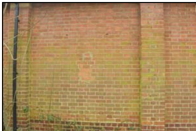
SGA15-0110 Building 27. Facing south
