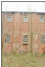
SGA15-0115 Building 28. Facing north
