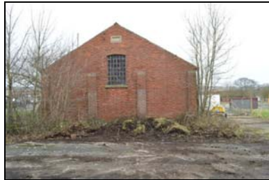
SGA15-0146 Building 32. Facing north
