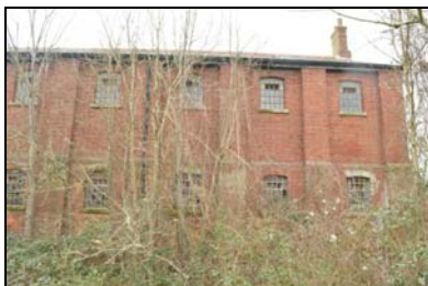
SGA15-0118 Building 28. Facing north
