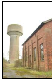
SGA15-0077 Building 25 and water tower. Facing south-east
