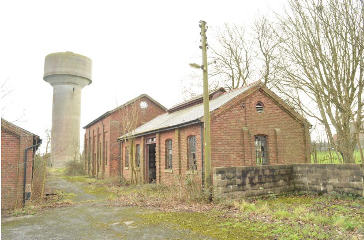
Plate 14 – Carpenters' shop (Building 26), looking south-east (SGA15-083)
