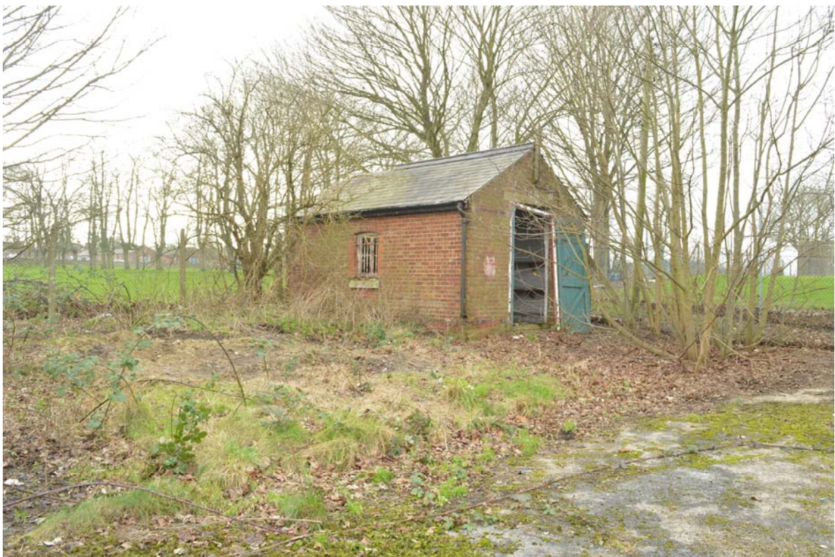
Plate 26 – Paint store (Building 30), looking south-west (SGA15-128)
