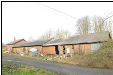
SGA15-0037 Building 29. Facing north-west
