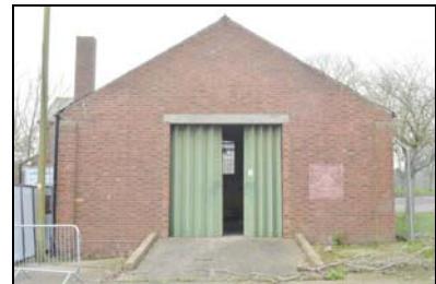
SGA15-0150 Building 32. Facing south
