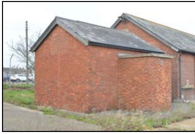
SGA15-0152 Building 33. Facing north-west
