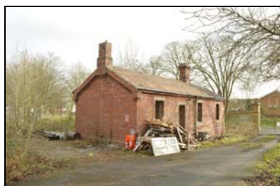
SGA15-0007 Building 24, office. Facing north-east
