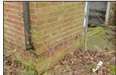
SGA15-0132 Building 30. Facing south-west
