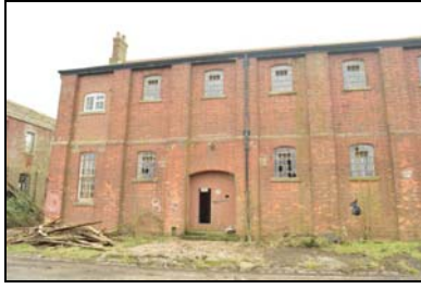
SGA15-0122 Building 28. Facing south
