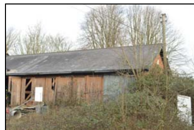
SGA15-0015 Building 29, water cart shed. Facing north
