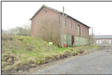
SGA15-0142 Building 31. Facing south-west
