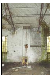
SGA15-0088 Building 26, interior. Facing south
