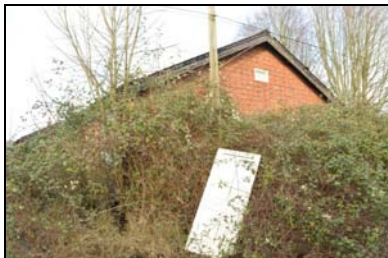
SGA15-0038 Building 29, water cart shed. Facing north-west
