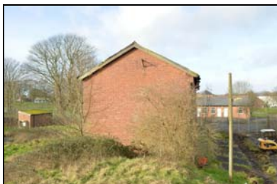
SGA15-0043 Building 31. Facing west
