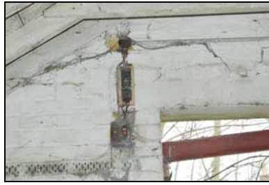
SGA15-0137 Building 30, interior. Facing north
