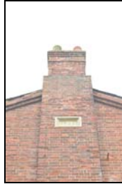
SGA15-0125 Building 28. Facing west
