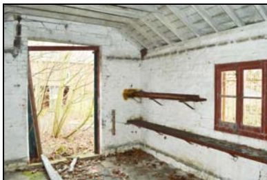
SGA15-0134 Building 30, interior. Facing north-east
