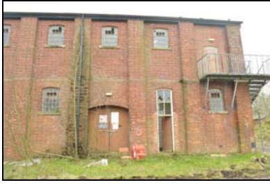
SGA15-0121 Building 28. Facing south
