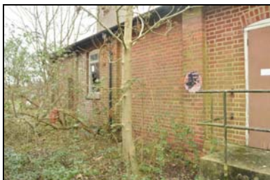
SGA15-0112 Building 27. Facing south-east
