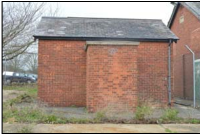
SGA15-0151 Building 33. Facing west
