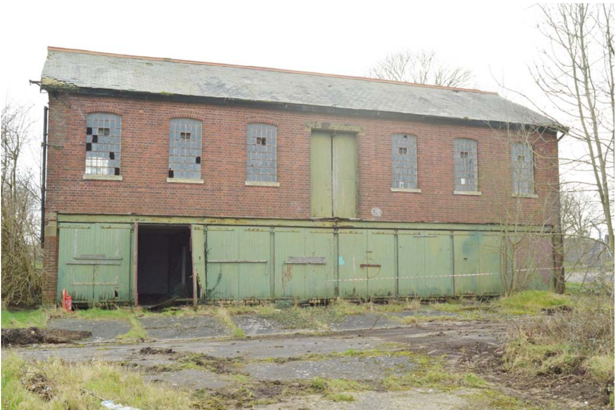
Plate 28 – Equipment store (Building 31), north elevation (SGA15-143)
