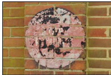
SGA15-0108 Building 27. Facing south
