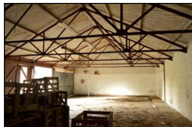
SGA15-0045 Building 29, water cart shed, interior. Facing west
