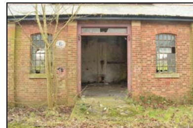
SGA15-0084 Building 26. Facing south
