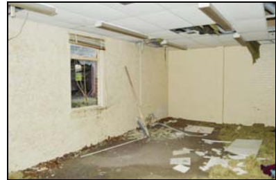
SGA15-0162 Building 27, interior. Facing south-west
