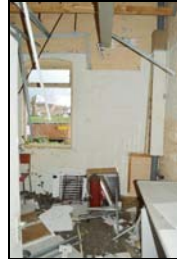
SGA15-0170 Building 27, interior. Facing north
