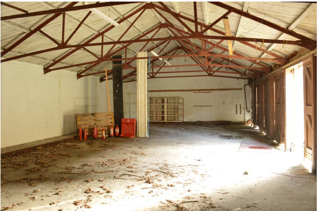
Plate 24 – Mobilisation wagon shed (Building 29), interior, looking east (SGA15-026)
