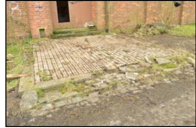
SGA15-0126 Building 28. Facing south-west
