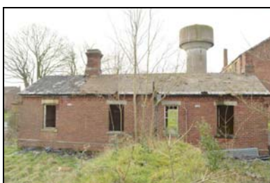
SGA15-0011 Building 24, office. Facing south
