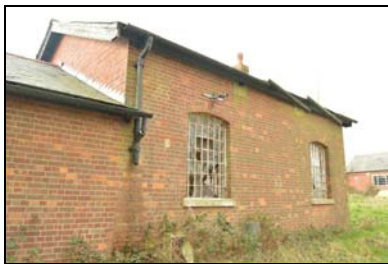
SGA15-0032 Building 29, mobilisation store. Facing south-west
