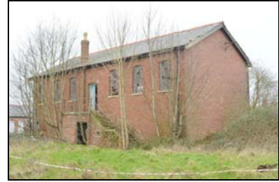
SGA15-0141 Building 31. Facing north-west
