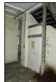
SGA15-0180 Building 28, interior, ground floor. Facing north-east
