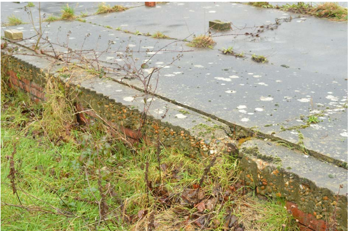
Plate 38 – Nissen Hut platform, showing impression of corrugated iron cladding (SGA15-220)
