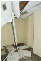
SGA15-0172 Building 27, interior. Facing north-east
