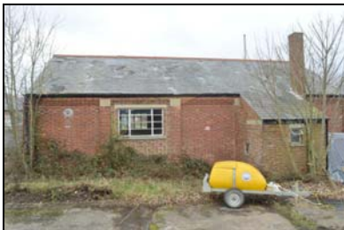
SGA15-0148 Building 32. Facing west
