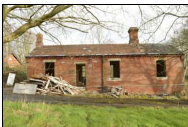
SGA15-0008 Building 24, office. Facing north
