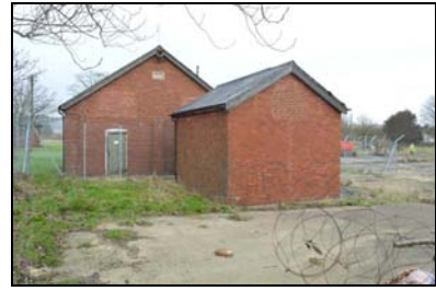
SGA15-0153 Buildings 33 & 34. Facing north
