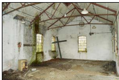
SGA15-0086 Building 26, interior. Facing north-west
