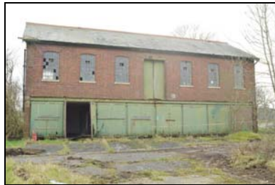
SGA15-0143 Building 31. Facing south
