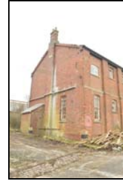
SGA15-0123 Building 28. Facing south-west
