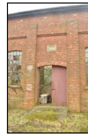
SGA15-0078 Building 25. Facing south
