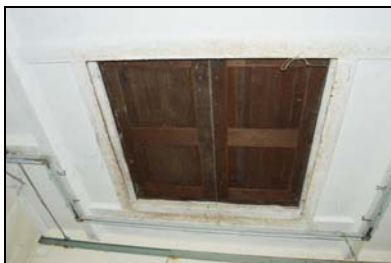
SGA15-0175 Building 28, interior, trapdoor. Facing north
