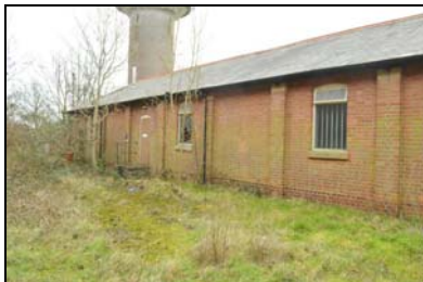
SGA15-0109 Building 27. Facing south-east
