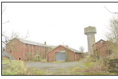
SGA15-0113 Buildings 26, 27, 28 & water tower. Facing east
