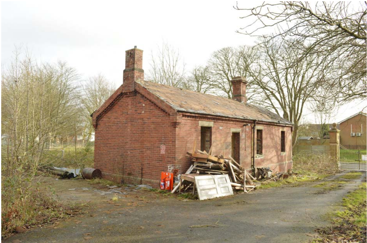
Plate 11 – Ordnance office (Building 24), looking north-east (SGA15-007)
