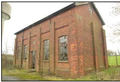
SGA15-0076 Building 25. Facing south-east
