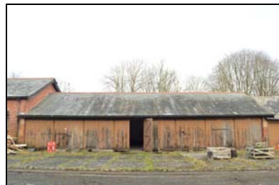
SGA15-0036 Building 29, wagon shed. Facing north
