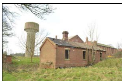
SGA15-0010 Building 24, office. Facing south-west
