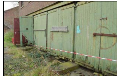
SGA15-0144 Building 31. Facing south-east
