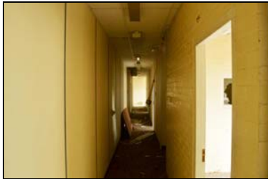
SGA15-0161 Building 27, interior. Facing west
