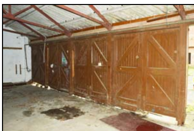
SGA15-0005 Building 29, wagon shed, interior. Facing south-east
