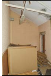
SGA15-0155 Building 27, interior. Facing west
