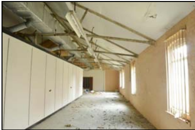
SGA15-0160 Building 27, interior. Facing west
