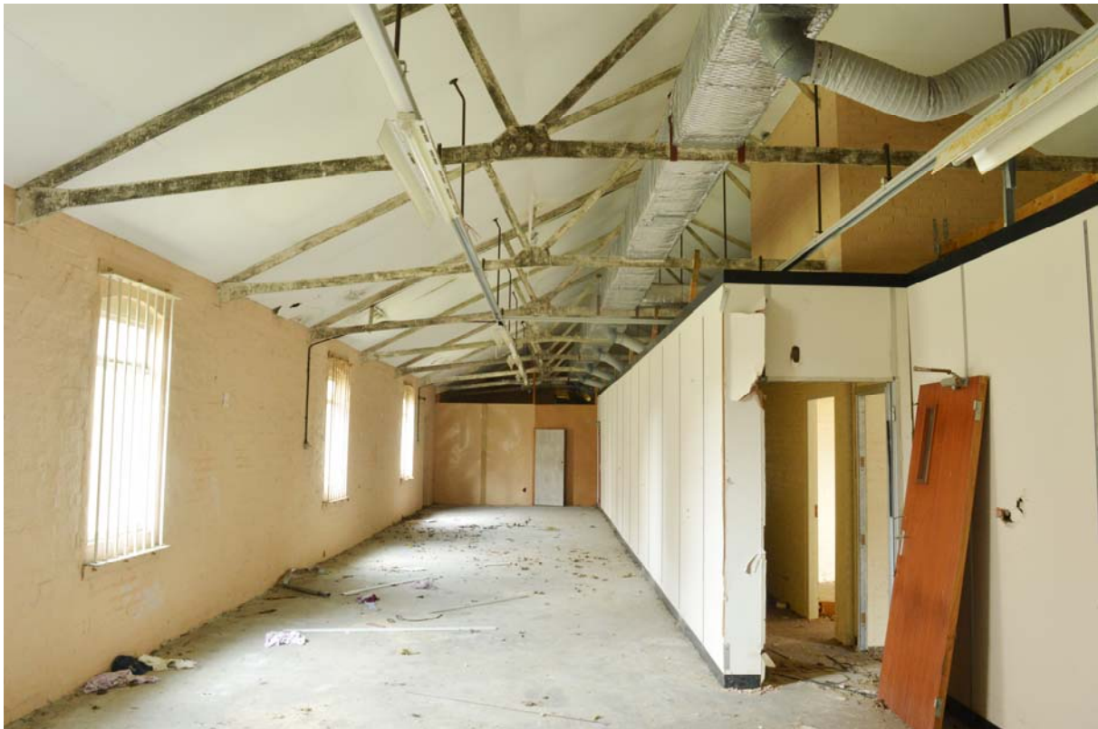
Plate 17 – Receiving shed (Building 27), interior, looking east (SGA15-159)
