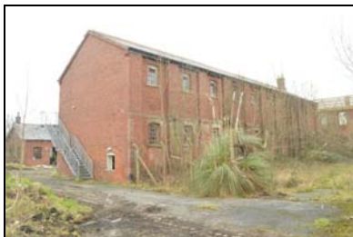
SGA15-0116 Building 28. Facing north-east
