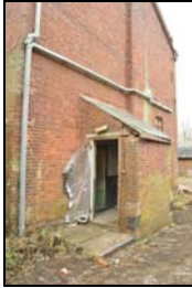
SGA15-0124 Building 28. Facing north-west
