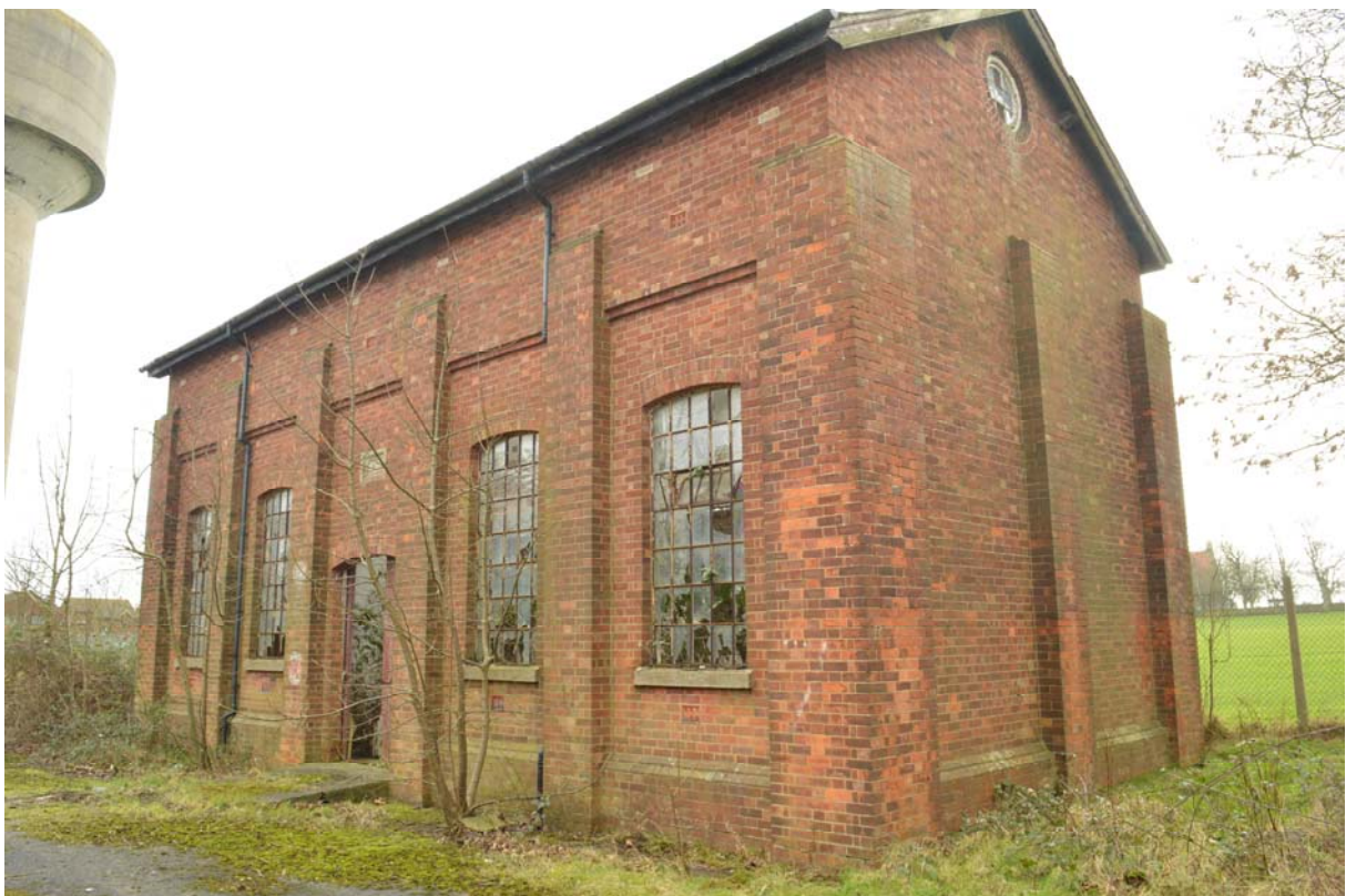
Plate 12 – Tent repairing shed (Building 25), looking south-east (SGA15-076)
