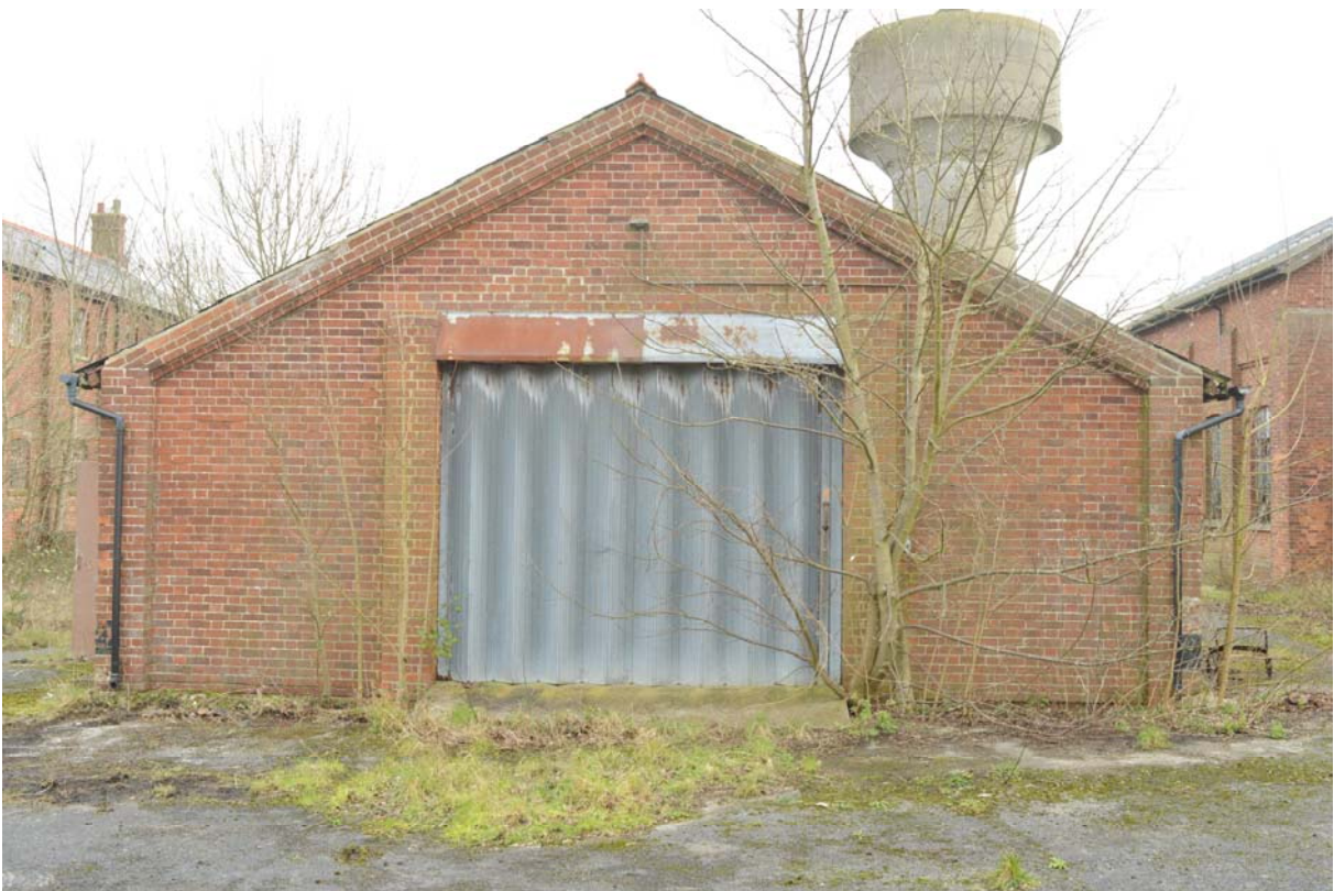
Plate 34 – Packing case store (Building 32), north elevation (SGA15-095)
