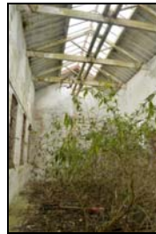
SGA15-0080 Building 25, interior. Facing west
