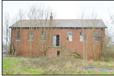
SGA15-0140 Building 31. Facing north
