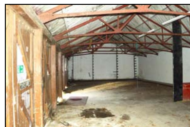
SGA15-0006 Building 29, wagon shed, interior. Facing west
