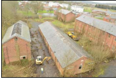
SGA15-0227 General view of site. Facing north-west
