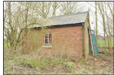
SGA15-0129 Building 30. Facing west
