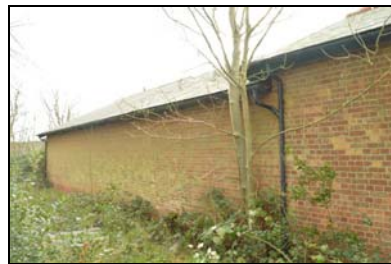
SGA15-0033 Building 29. Facing south-east
