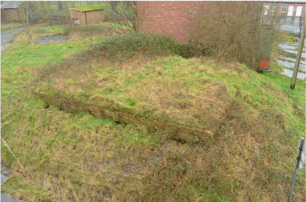
Plate 42 – Water tank to west of receiving store (Building 27), looking west (SGA15-200)
