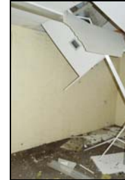
SGA15-0171 Building 27, interior. Facing north-east
