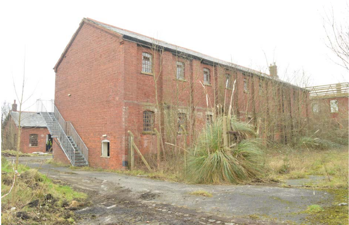
Plate 19 – Equipment store (Building 28), south and west elevations (SGA15-116)
