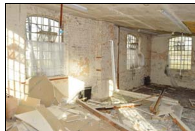
SGA15-0003 Building 29, mobilisation store, interior. Facing north-west
