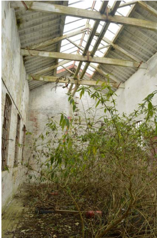
Plate 13 – Tent repairing shed (Building 25), interior, looking west (SGA15-080)
