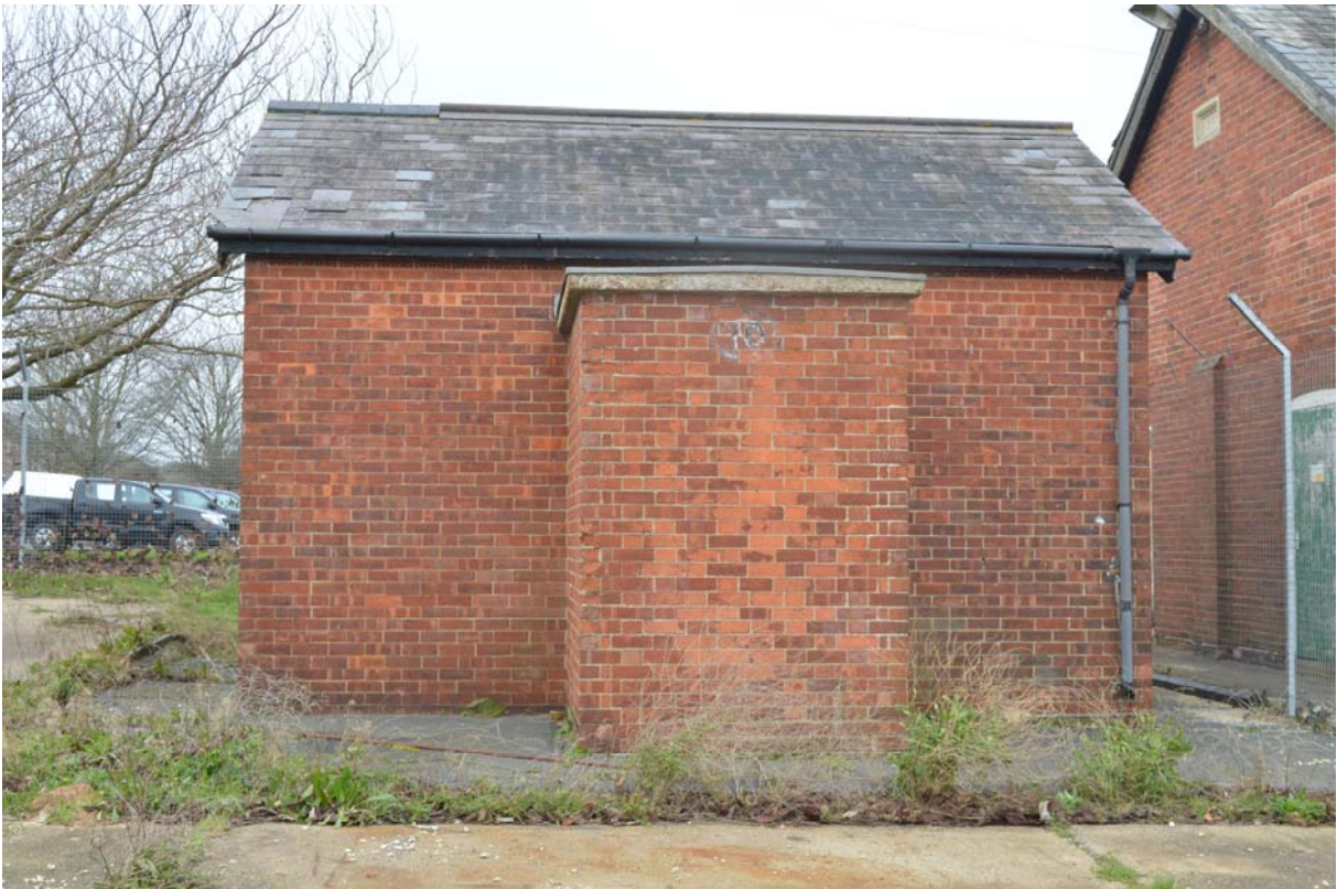
Plate 36 – Store (Building 33), looking west (SGA15-151)
