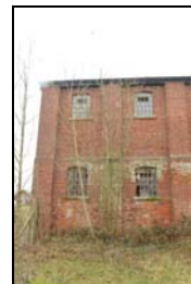
SGA15-0117 Building 28. Facing north
