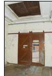
SGA15-0174 Building 28, interior, ground floor. Facing north
