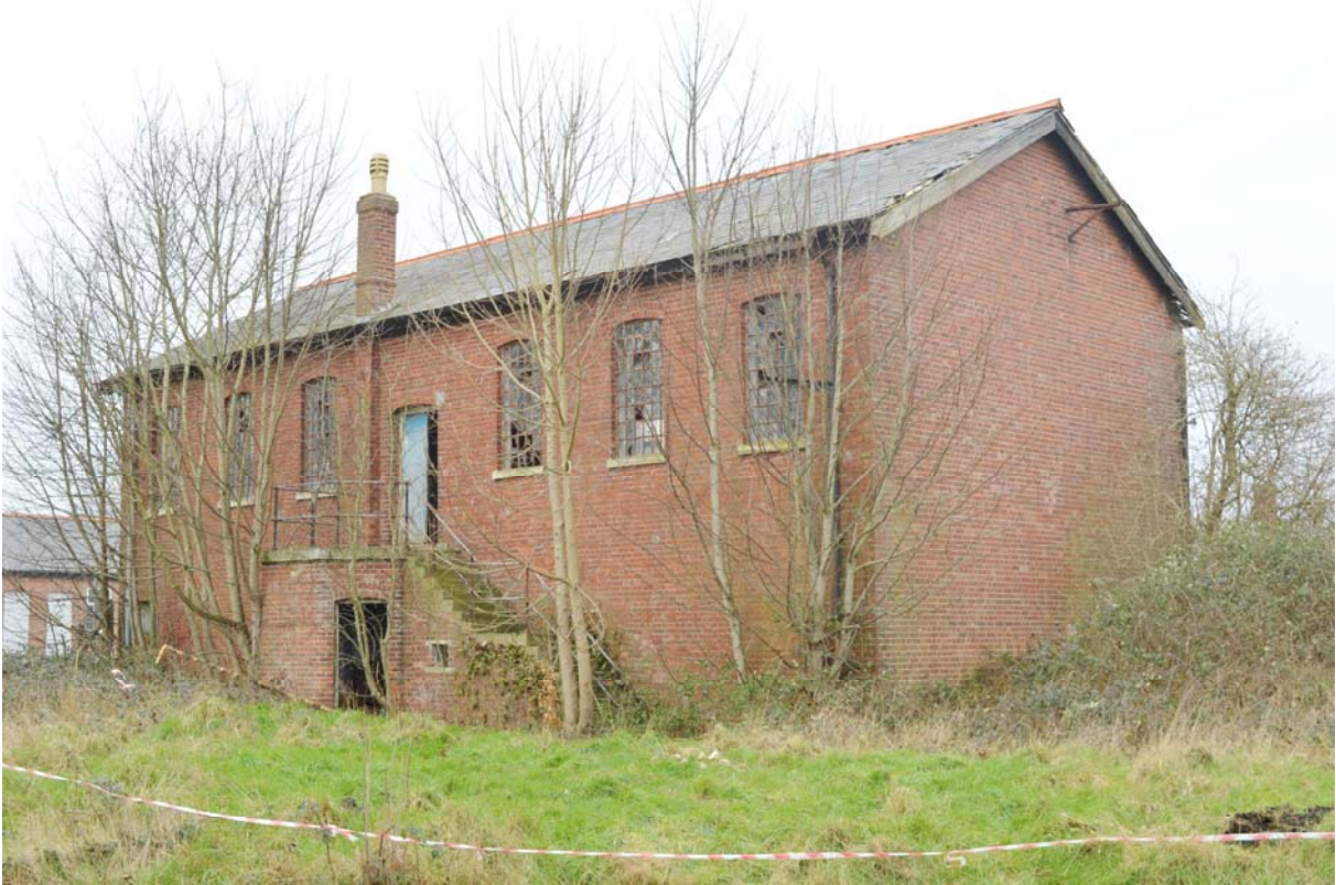
Plate 29 – Equipment store (Building 31), south and east elevations (SGA15-141)
