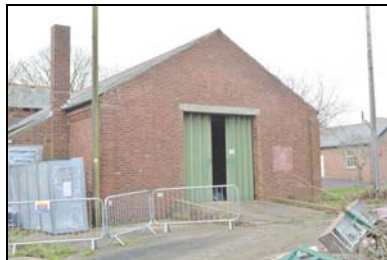
SGA15-0149 Building 32. Facing south-west
