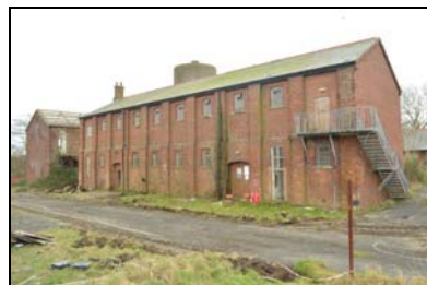
SGA15-0120 Building 28. Facing south-east
