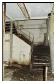
SGA15-0179 Building 28, interior, ground floor. Facing east
