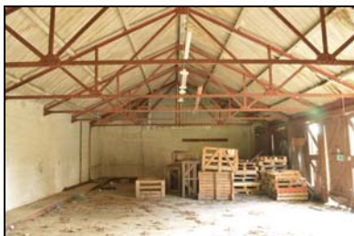
SGA15-0044 Building 29, water cart shed, interior. Facing east
