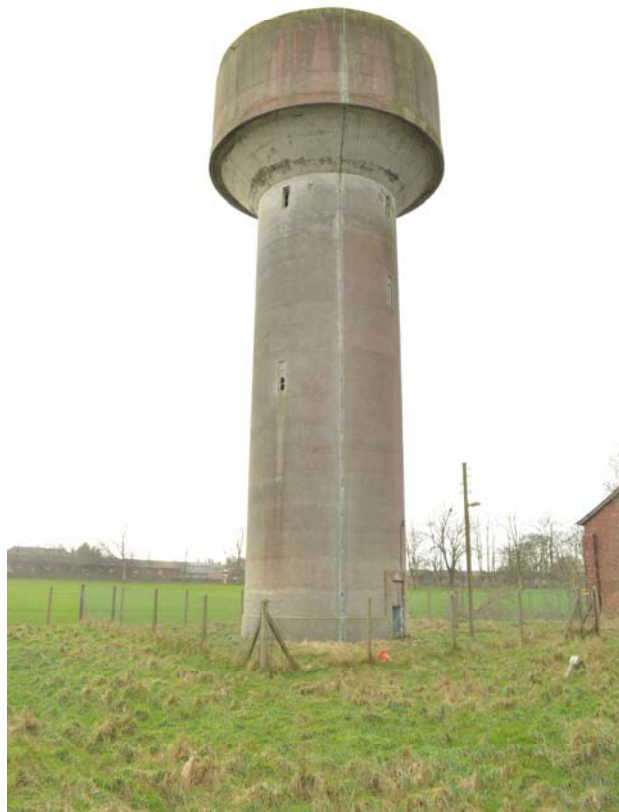
Plate 4 – The water tower (Building 21), looking south-west (SGA15-052)
