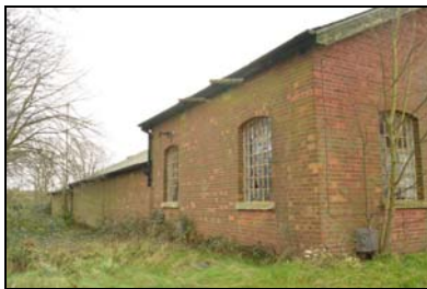
SGA15-0031 Building 29. Facing south-east
