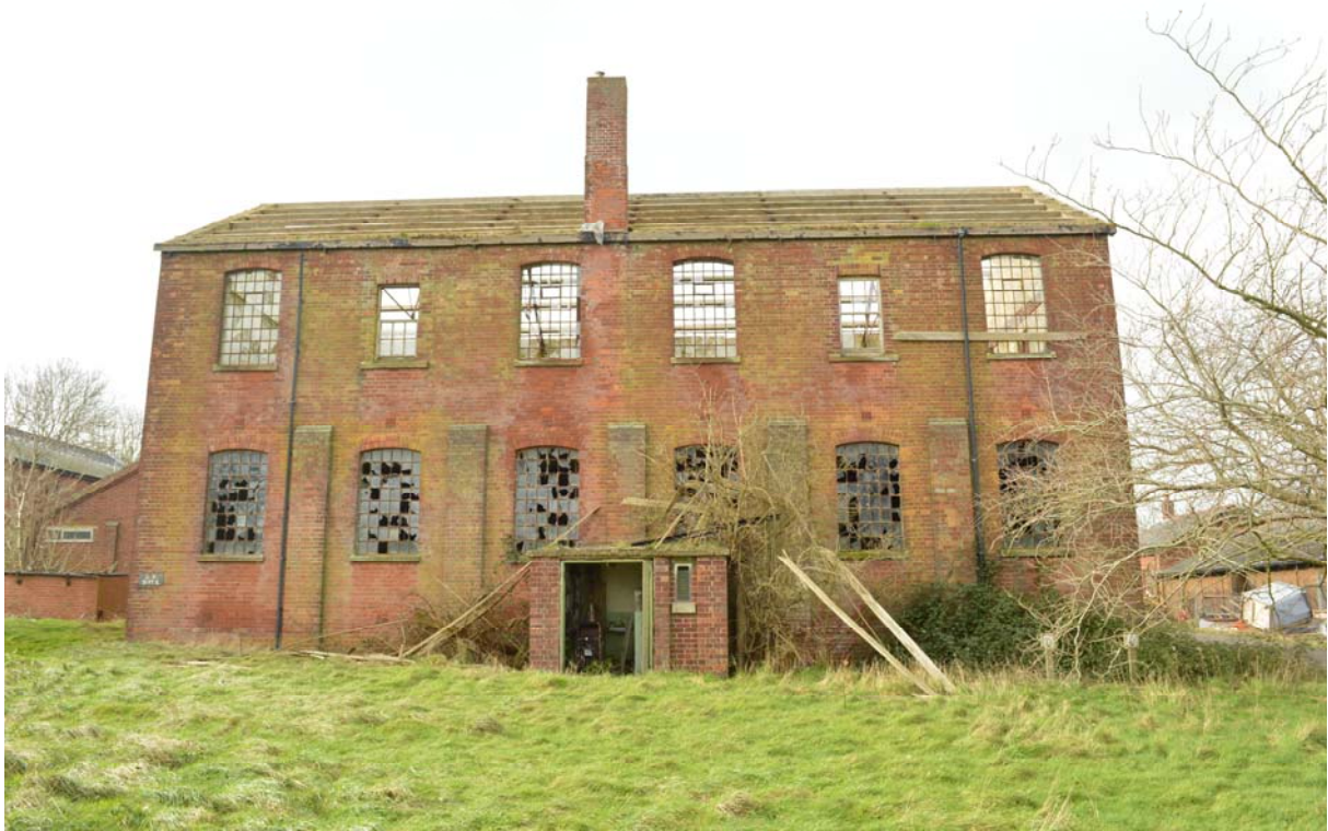
Plate 5 – The saddlery & harness store (Building 22), east elevation (SGA15-058)
