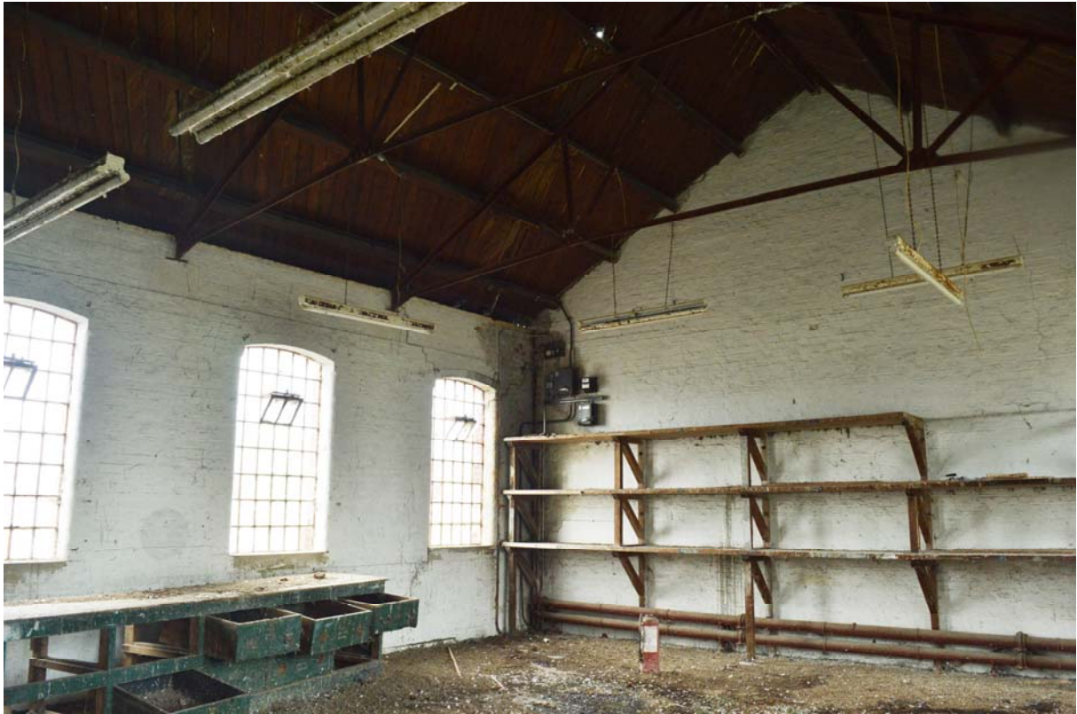
Plate 31 – Equipment store (Building 31), first floor, looking north-east (SGA15-205)
