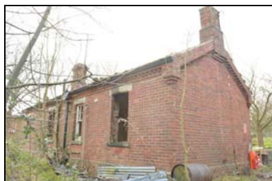
SGA15-0013 Building 24, office. Facing south-east
