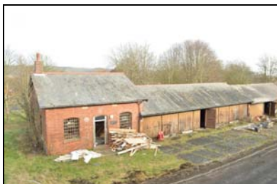
SGA15-0040 Building 29. Facing north-east
