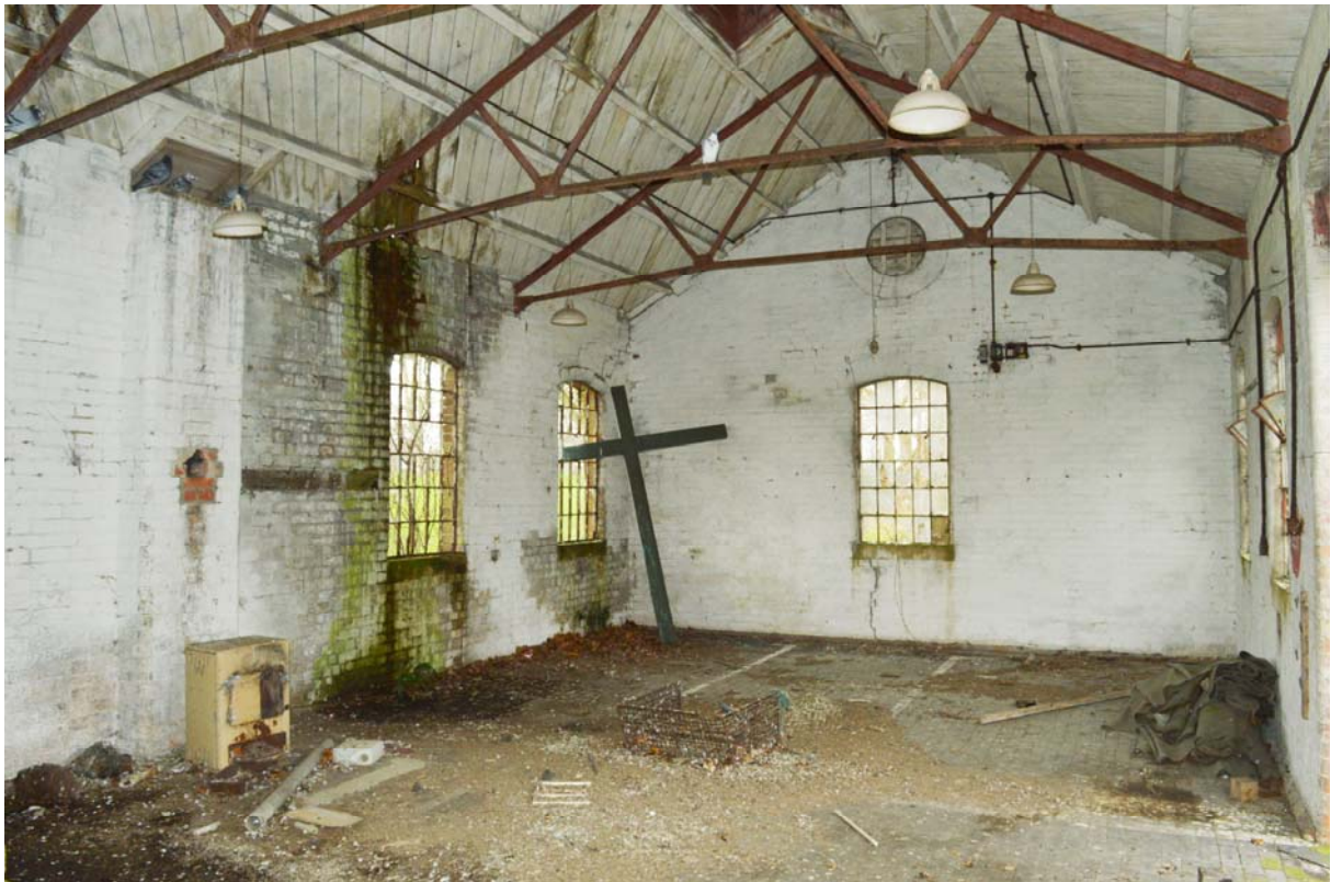
Plate 15 – Carpenters' shop (Building 26), interior, looking west (SGA15-086)
