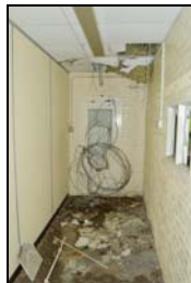
SGA15-0164 Building 27, interior. Facing south
