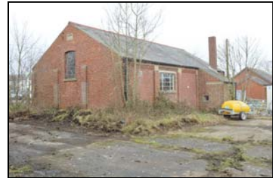
SGA15-0147 Building 32. Facing north-west
