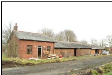
SGA15-0034 Building 29. Facing north-east
