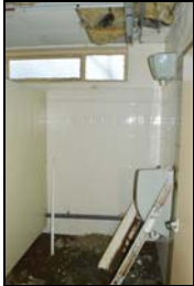
SGA15-0169 Building 27, interior. Facing north
