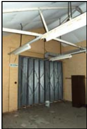
SGA15-0157 Building 27, interior. Facing west
