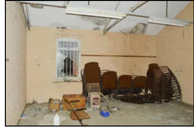
SGA15-0156 Building 27, interior. Facing south
