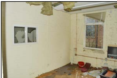
SGA15-0163 Building 27, interior. Facing south-east
