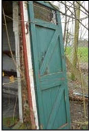
SGA15-0139 Building 30, door. Facing west
