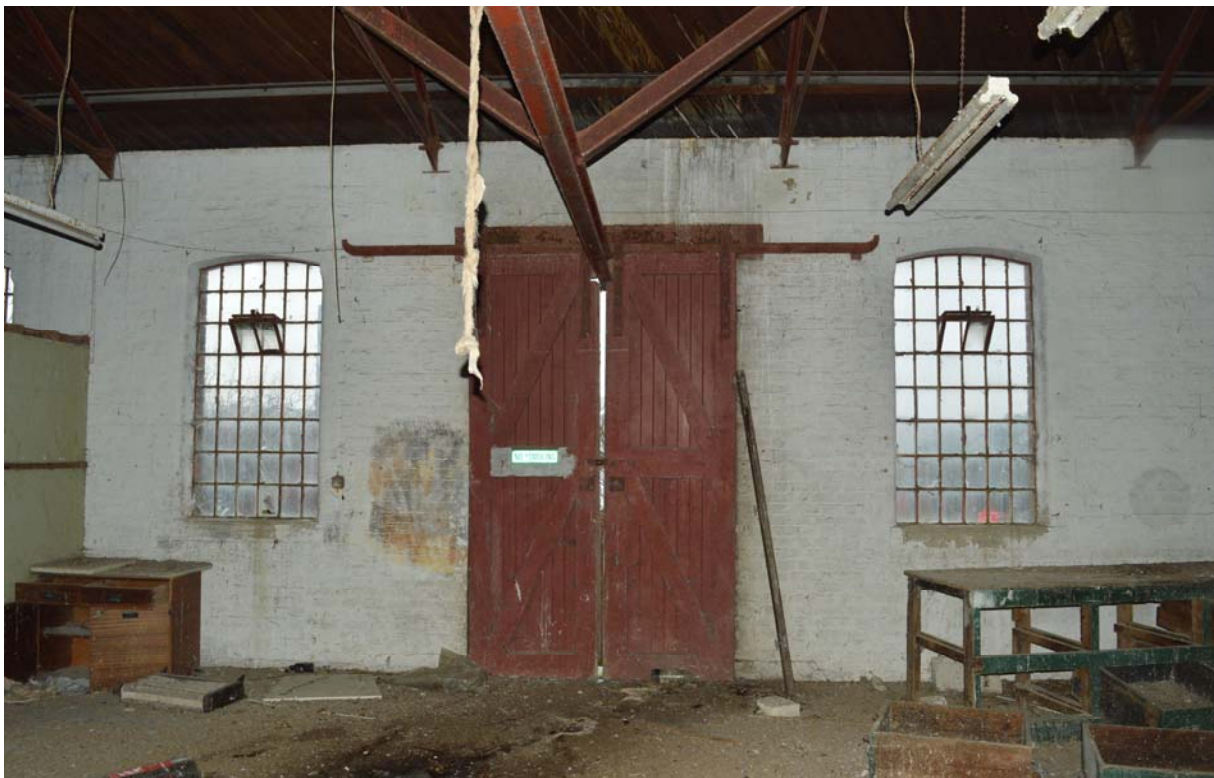
Plate 32 – Equipment store (Building 31), first floor, goods crane and doorway, looking north (SGA15-208)
