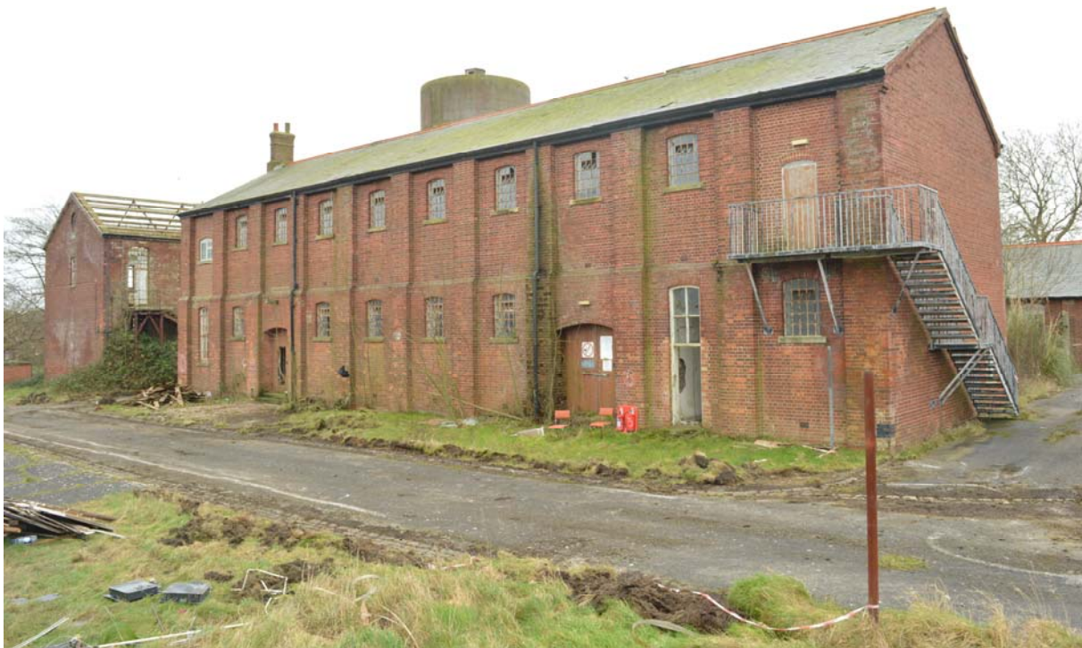
Plate 18 – Equipment store (Building 28), north elevation (SGA15-120)
