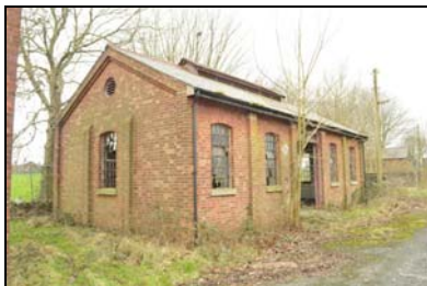
SGA15-0082 Building 26. Facing south-west
