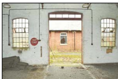
SGA15-0089 Building 26, interior. Facing north
