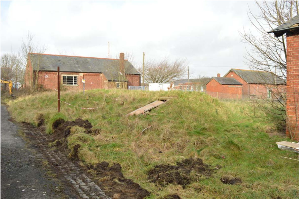
Plate 41 – Air raid shelter to west of mobilisation store (Building 29), looking north-west (SGA15-047)
