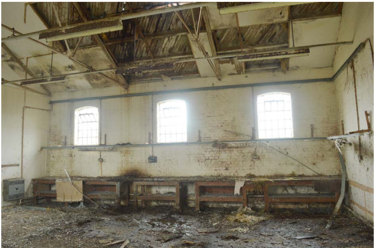
Plate 22 – Equipment store (Building 28), first floor, looking south (SGA15-197)
