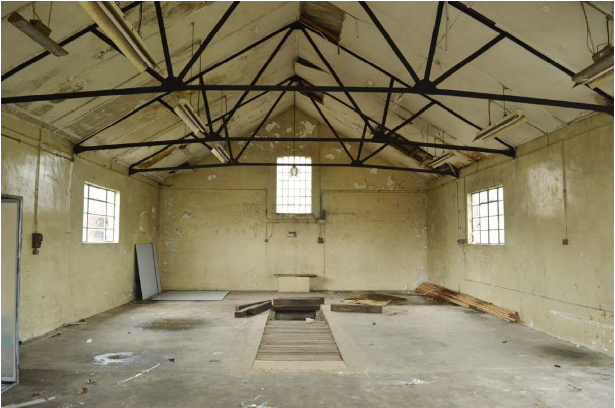
Plate 35 – Packing case store (Building 32), interior, looking south (SGA15-214)
