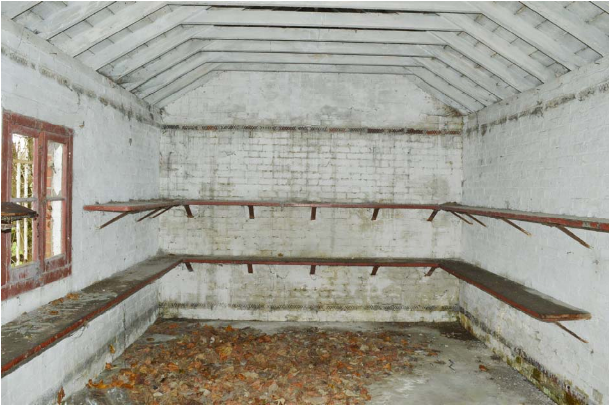
Plate 27 – Paint store (Building 30), interior, looking south (SGA15-133)
