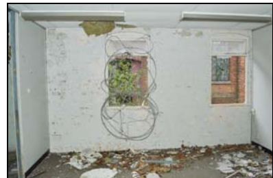
SGA15-0165 Building 27, interior. Facing south
