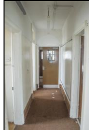
SGA15-0278 Building 18, ground floor, corridor. Facing east
