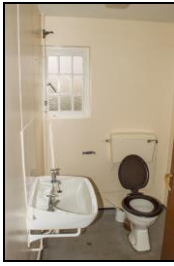
SGA15-0274 Building 17, WC. Facing east
