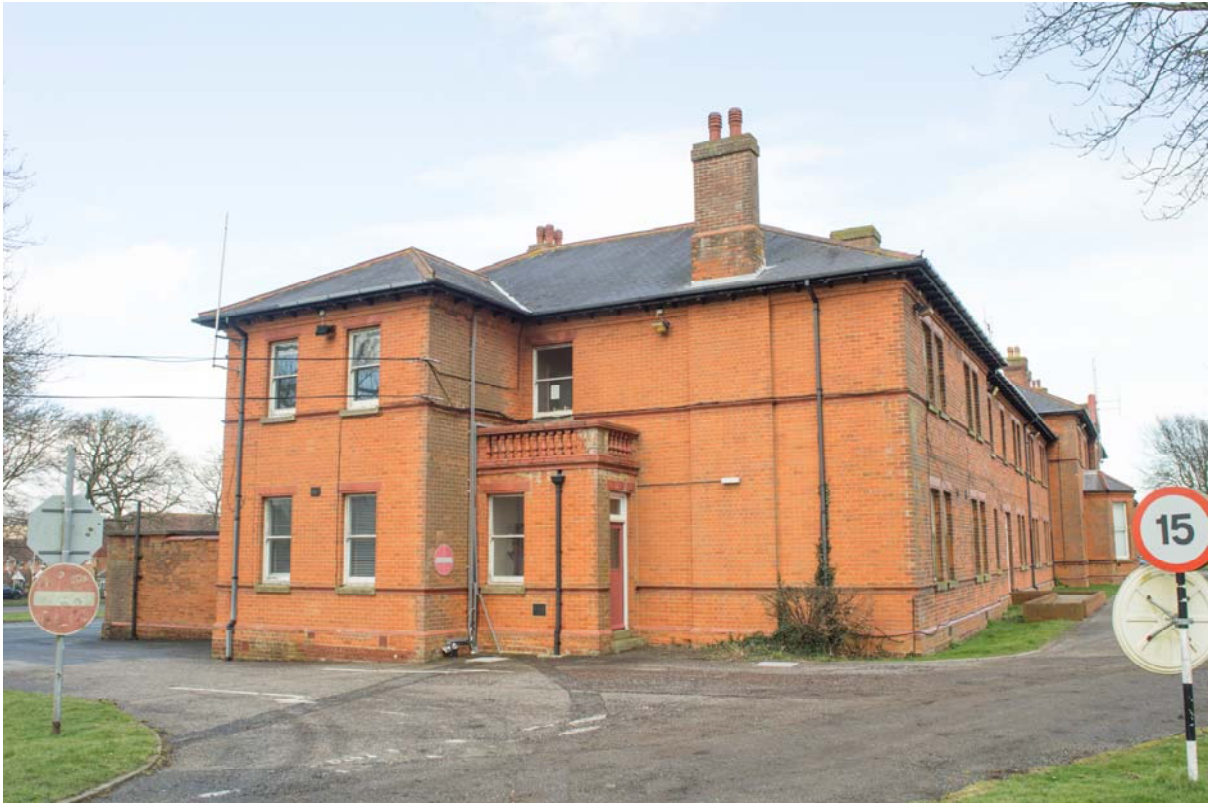
Plate 54 – Building 20: field officers' quarters at western end of building. View looking east (SGA15-414)
