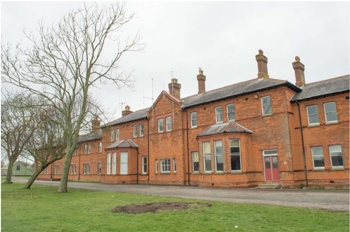
Plate 46 – Building 20: officers' mess, front elevation showing location of former main entrance. View looking north-west (SGA15-385)
