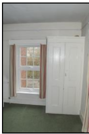
SGA15-0604 Building 19, W side, first floor, N bedroom. Facing west
