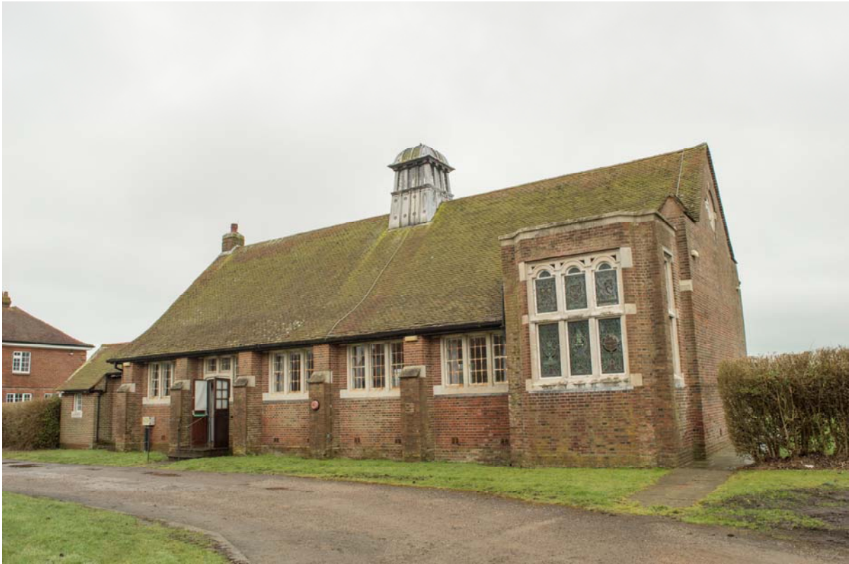
Plate 13 – Building 17: Sir John Moore Library, exterior view looking south-east (SGA15-311)
