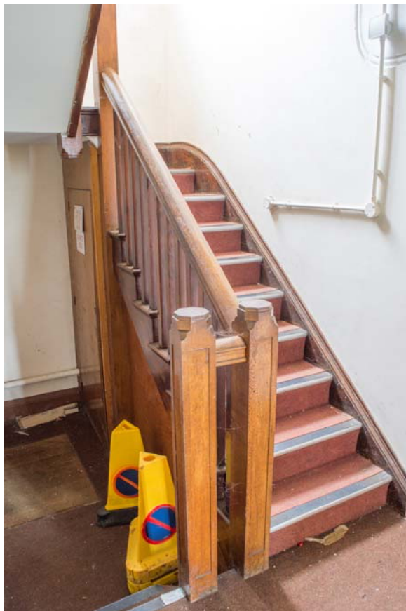
Plate 32 – Building 18: general view of stair, looking north-east (SGA15-281)
