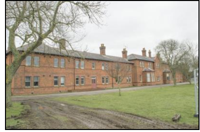
SGA15-0381 Building 20, exterior. Facing north-east
