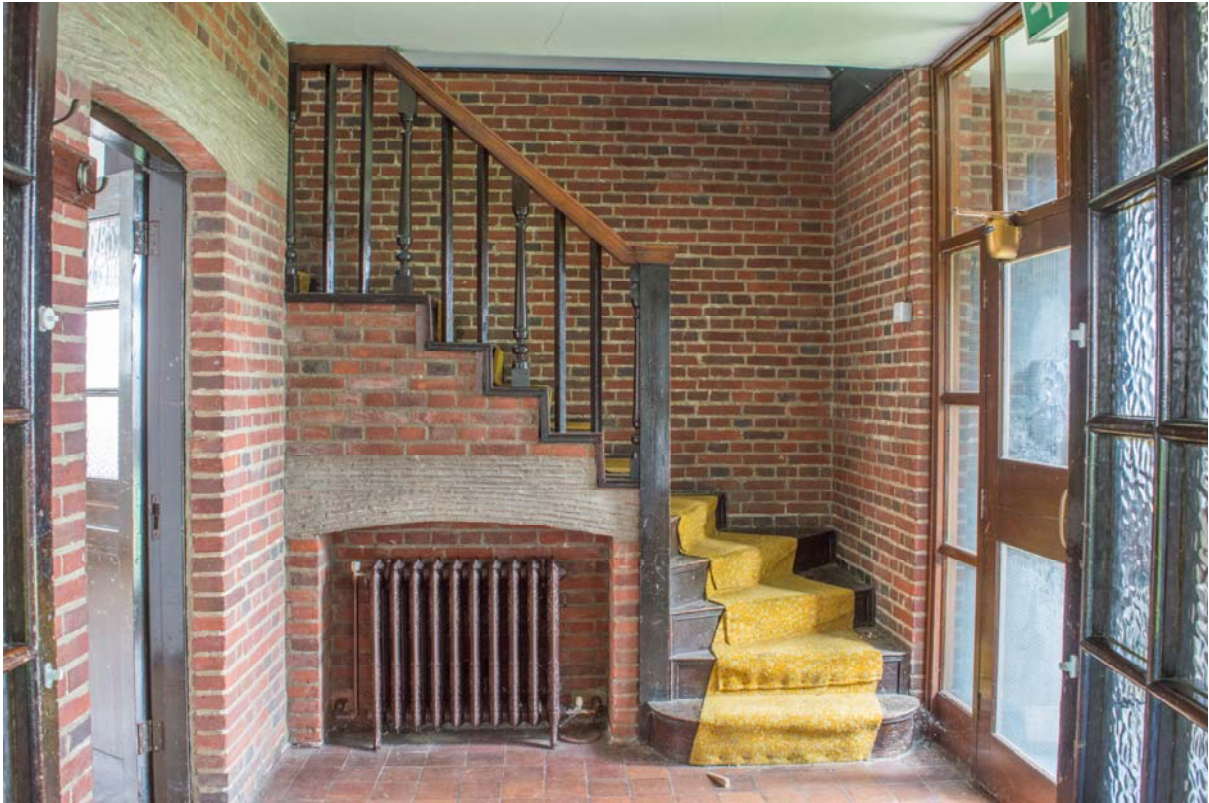
Plate 19 – Building 17: Sir John Moore Library, view of the vestibule looking east towards the stair (SGA15-264)
