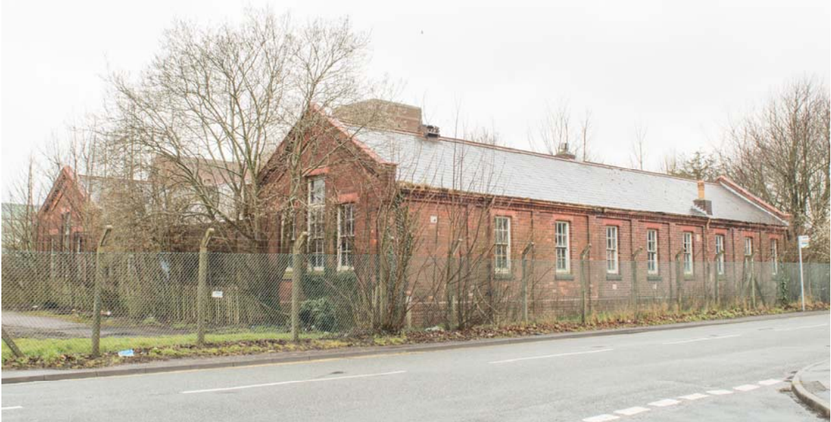
Plate 7 – Building 15: exterior of the adults' school, looking south-west (SGA15-612)
