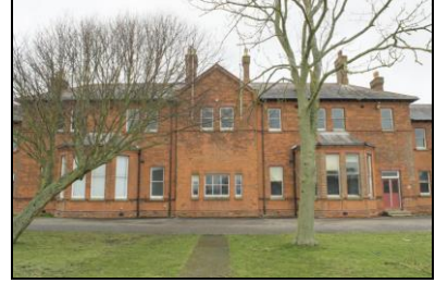
SGA15-0384 Building 20, exterior. Facing north
