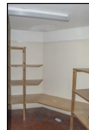
SGA15-0609 Building 19, W side, first floor, W extension. Facing west
