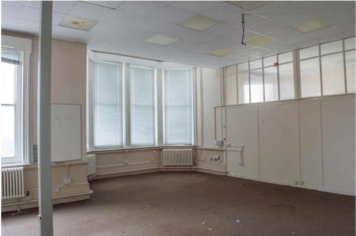
Plate 66 – Building 20: ground floor, mess room. View looking south-west (SGA15-462)
