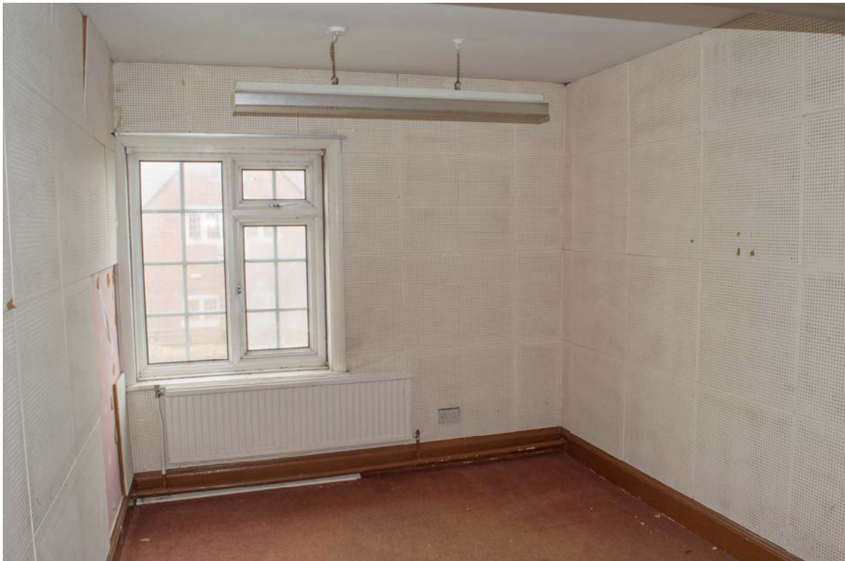
Plate 34 – Building 18: first floor, interrogation room at the western end of the building. View looking west (SGA15-291)
