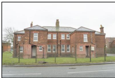
SGA15-0611 Building 19, exterior. Facing south
