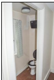
SGA15-0610 Building 19, W side, first floor, W extension. Facing east
