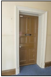
SGA15-0454 Building 20, ground floor, billiard room entrance. Facing north
