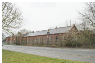
SGA15-0613 Building 15, exterior. Facing south-east
