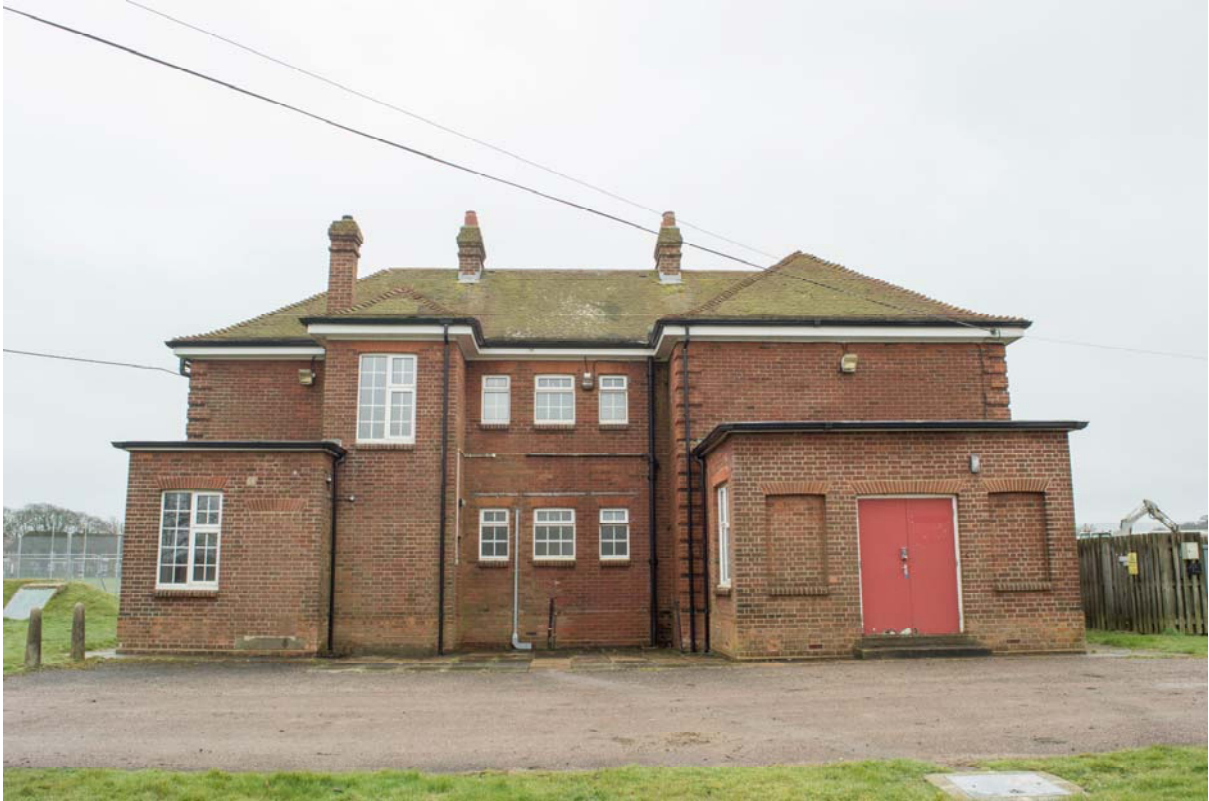
Plate 27 – Building 18: Police Station, general view looking south (SGA15-325)
