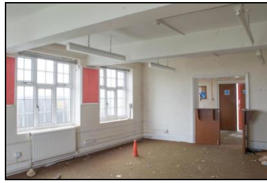
SGA15-0275 Building 18, ground floor, main room. Facing north-west
