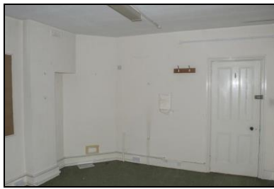
SGA15-0605 Building 19, W side, first floor, N bedroom. Facing south
