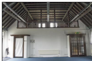
SGA15-0243 Building 17, hall, balcony. Facing east
