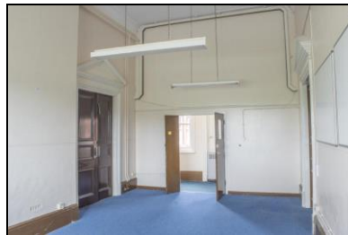
SGA15-0461 Building 20, ground floor, former lobby. Facing north
