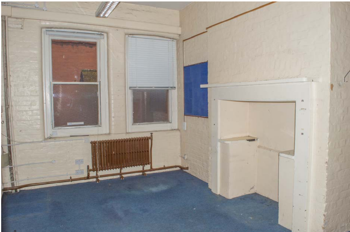
Plate 59 – Building 20: commander's quarters, ground floor, kitchen. View looking north-west (SGA15-420)
