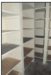
SGA15-0466 Building 20, ground floor, service expense. Facing south-west
