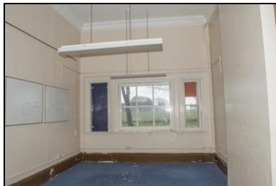
SGA15-0460 Building 20, ground floor, former lobby. Facing south
