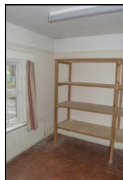
SGA15-0608 Building 19, W side, first floor, W extension. Facing west
