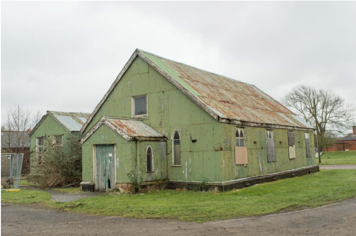
Plate 9 – Building 16: iron church, general view looking north-east (SGA15-335)
