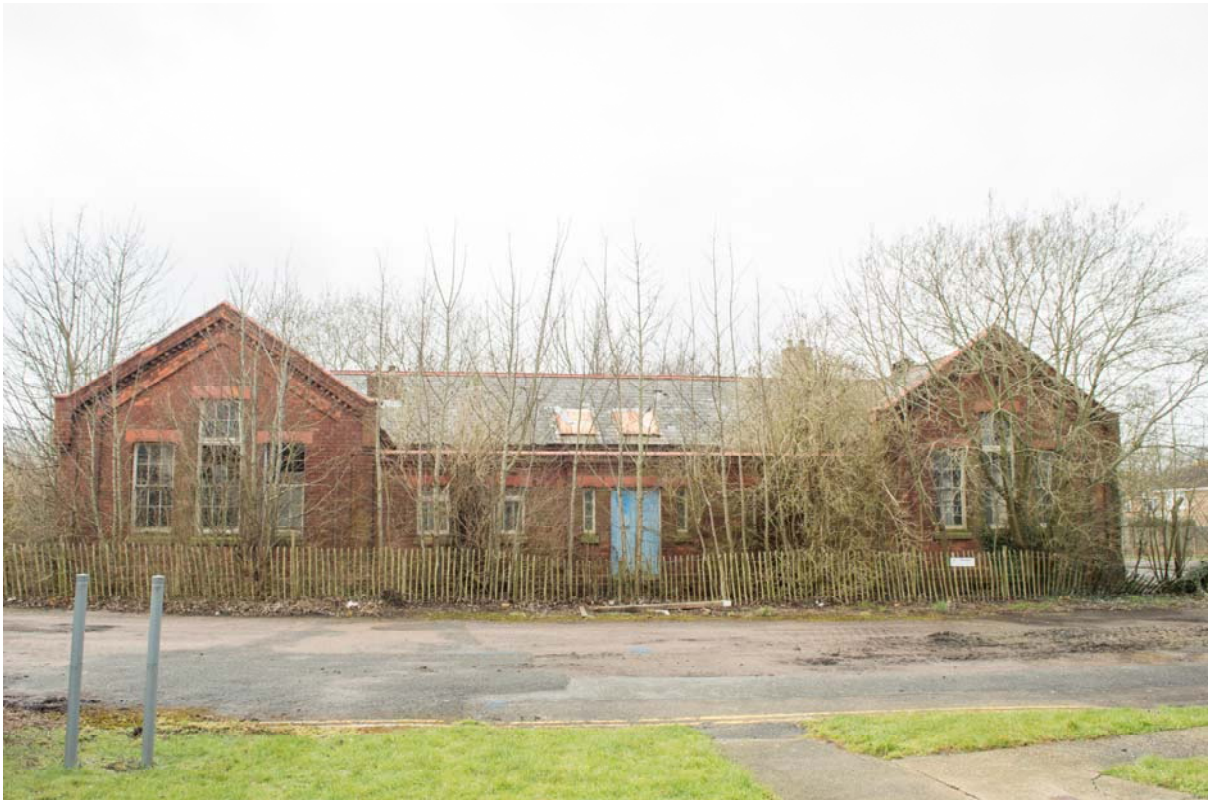
Plate 6 – Building 15: front elevation of the adults' school, looking west (SGA15-349)
