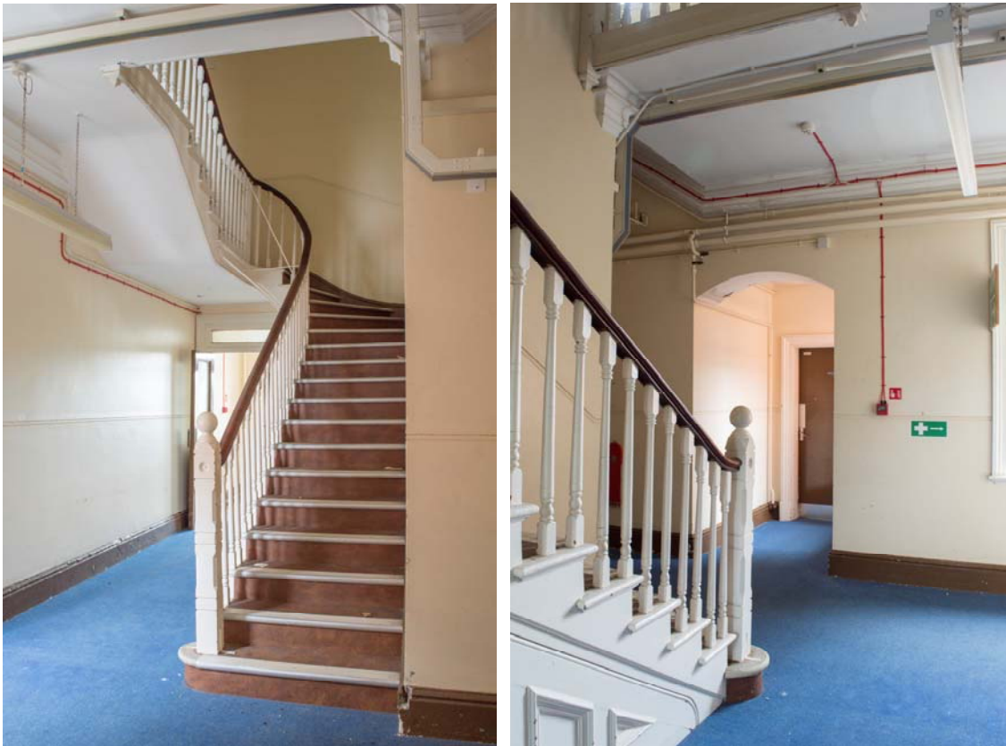
Plate 67 – Building 20: ground floor, views of main stair (SGA15-462)
