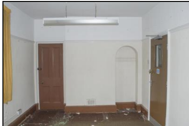
SGA15-0280 Building 18, ground floor, SE room. Facing west
