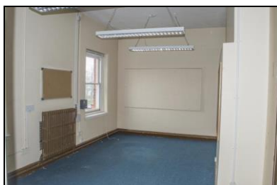
SGA15-0541 Building 20, first floor, field officers' servants room. Facing east
