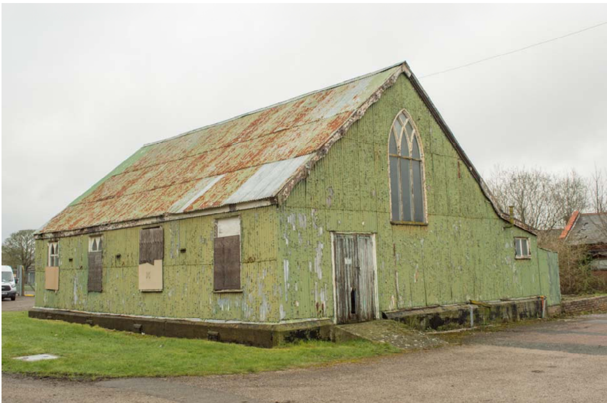
Plate 10 – Building 16: iron church, general view looking north-west (SGA15-333)
