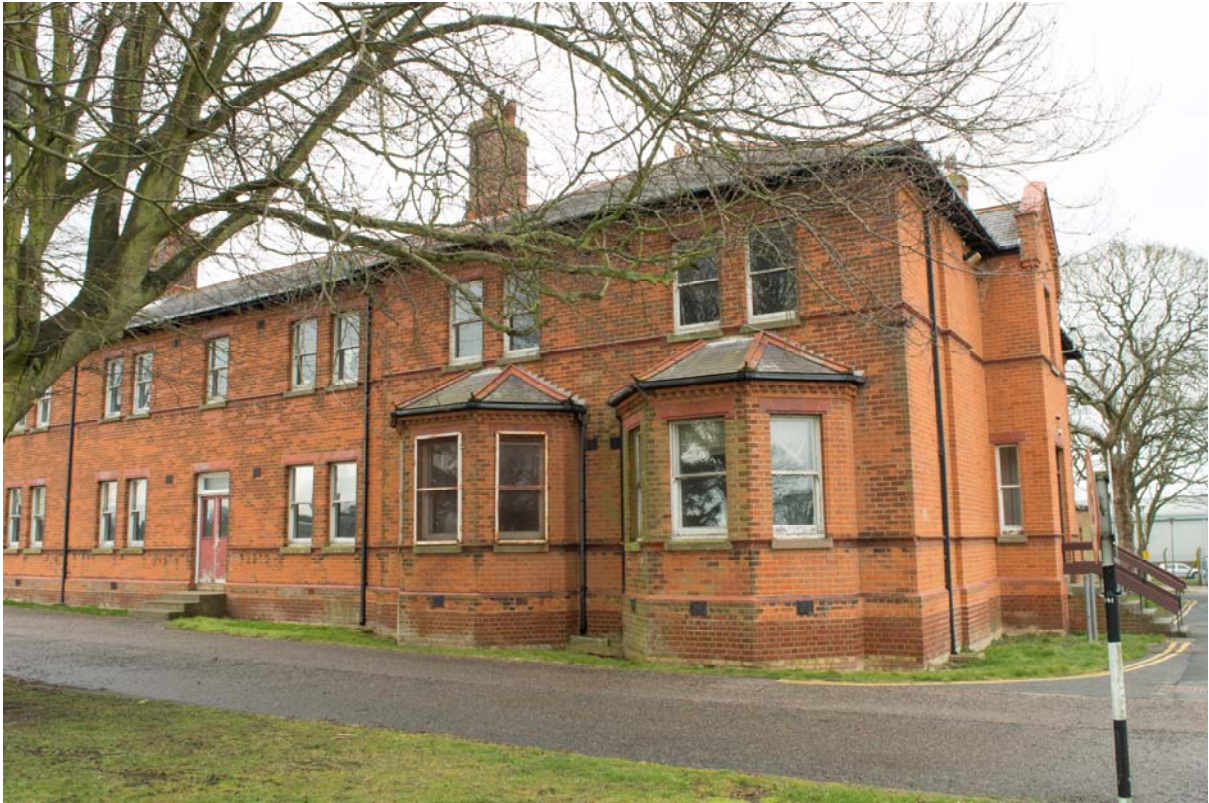
Plate 47 – Building 20: front elevation of commander's residence at eastern end of building, looking north (SGA15-387)
