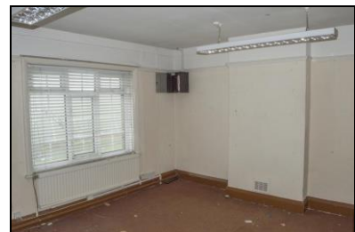
SGA15-0288 Building 18, first floor, S room. Facing north-east
