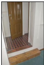
SGA15-0532 Building 20, first floor, field officers' WC. Facing north
