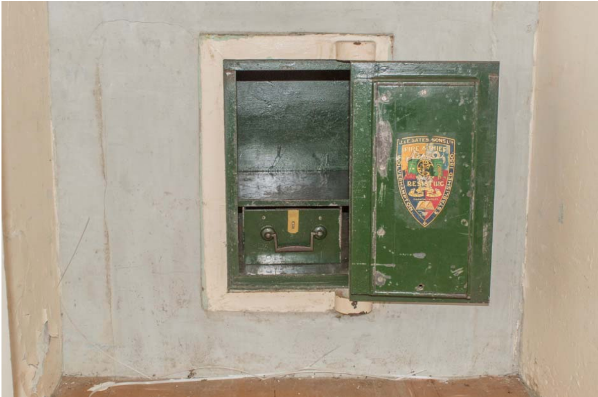
Plate 41 – Building 19: western house, ground floor, safe within former pantry (SGA15-554)
