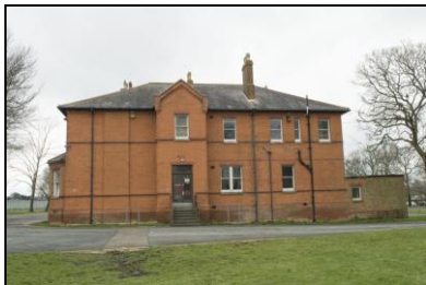
SGA15-0388 Building 20, exterior. Facing west
