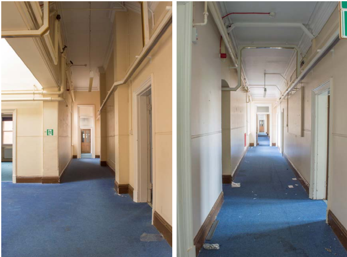
Plate 55 – Building 20: ground level, views along the main corridor (SGA15-465 & 484)
