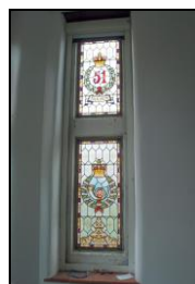
SGA15-0242 Building 17, hall, window detail. Facing west
