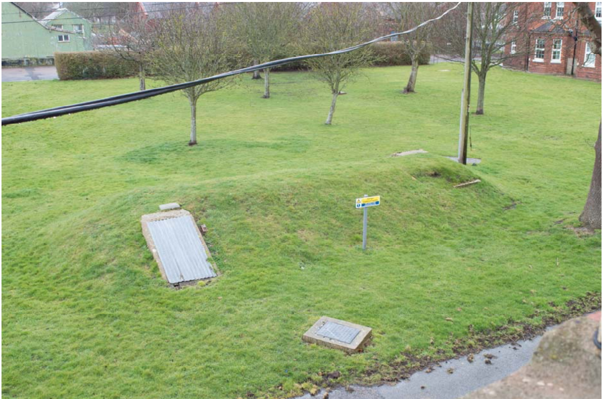
Plate 86 – Detail of air raid shelter to the west of Building 20. View looking north-west (SGA15-538)
