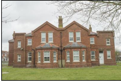
SGA15-0379 Building 19, exterior. Facing north
