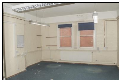
SGA15-0467 Building 20, ground floor, pantry. Facing east
