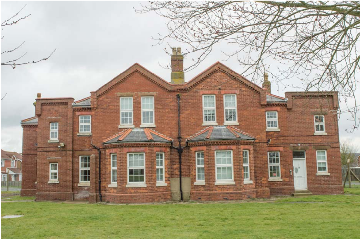
Plate 35 – Building 19: front elevation, looking north (SGA15-379)
