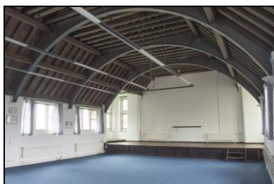
SGA15-0230 Building 17, hall. Facing west
