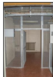
SGA15-0540 Building 20, first floor, field officers' servants room. Facing east
