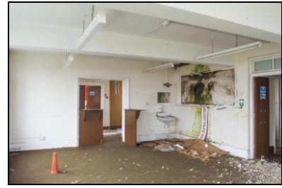
SGA15-0276 Building 18, ground floor, main room. Facing north
