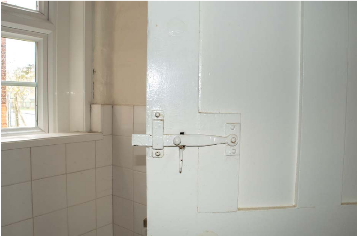
Plate 39 – Building 19: eastern house, ground floor, archaic latch within original kitchen (SGA15-572)
