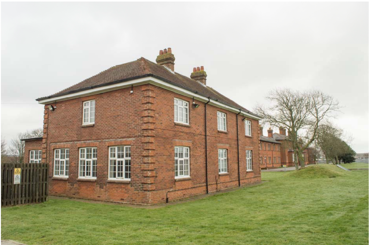
Plate 28 – Building 18: Police Station, general view looking north-east towards the officers' mess (SGA15-327)
