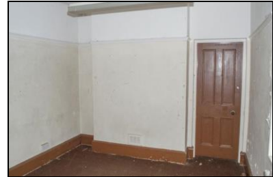
SGA15-0279 Building 18, ground floor, S room. Facing east
