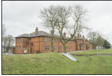
SGA15-0380 Air raid shelter Building 20, exterior. Facing north-east
