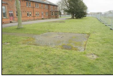
SGA15-0383 Building 20, exterior, flagpole base. Facing north-east
