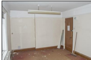
SGA15-0284 Building 18, first floor, SE room. Facing west
