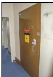
SGA15-0539 Building 20, first floor, field officers' service corridor. Facing north
