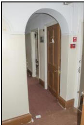
SGA15-0283 Building 18, first floor, landing. Facing west
