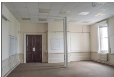
SGA15-0463 Building 20, ground floor, mess room. Facing east
