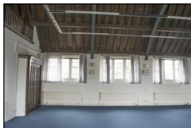
SGA15-0235 Building 17, hall. Facing south
