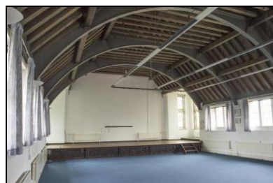
SGA15-0231 Building 17, hall. Facing west
