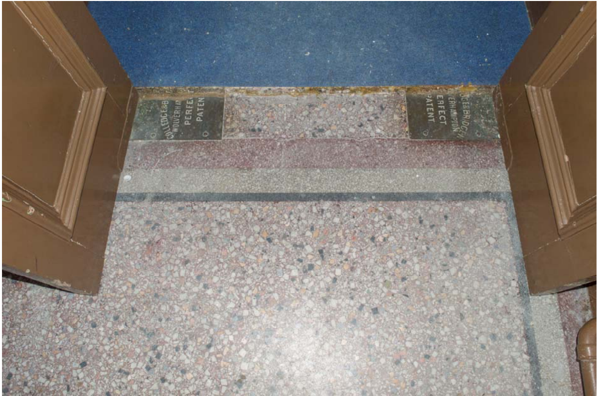
Plate 68 – Building 20: ground floor, original terrazzo floor to main stairwell (SGA15-450)
