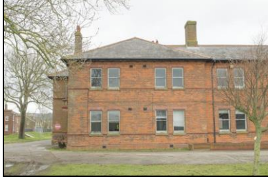
SGA15-0382 Building 20, exterior. Facing north
