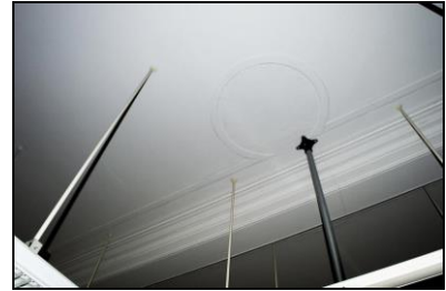
SGA15-0459 Building 20, ground floor, ante room, ceiling. Facing
