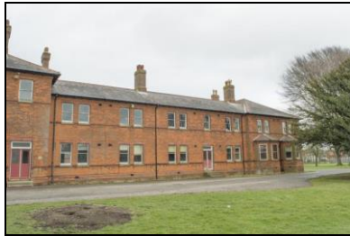
SGA15-0386 Building 20, exterior. Facing north
