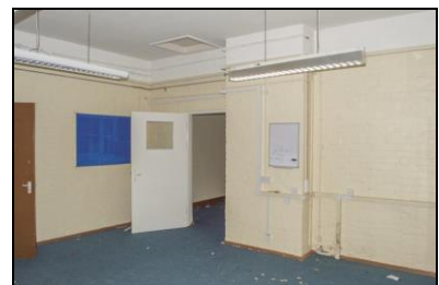
SGA15-0468 Building 20, ground floor, pantry. Facing north-west
