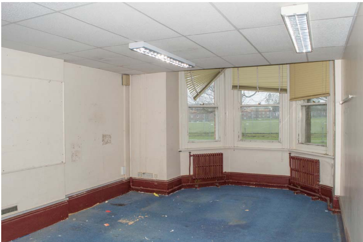
Plate 57 – Building 20: commander's quarters, ground floor living room. View looking south (SGA15-428)
