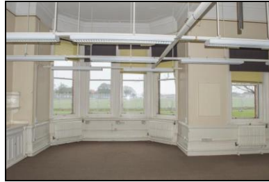
SGA15-0458 Building 20, ground floor, ante room. Facing south
