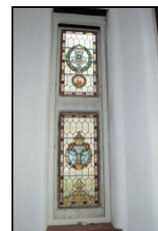
SGA15-0240 Building 17, hall, window detail. Facing west
