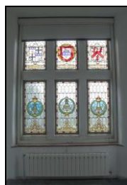
SGA15-0241 Building 17, hall, window detail. Facing south
