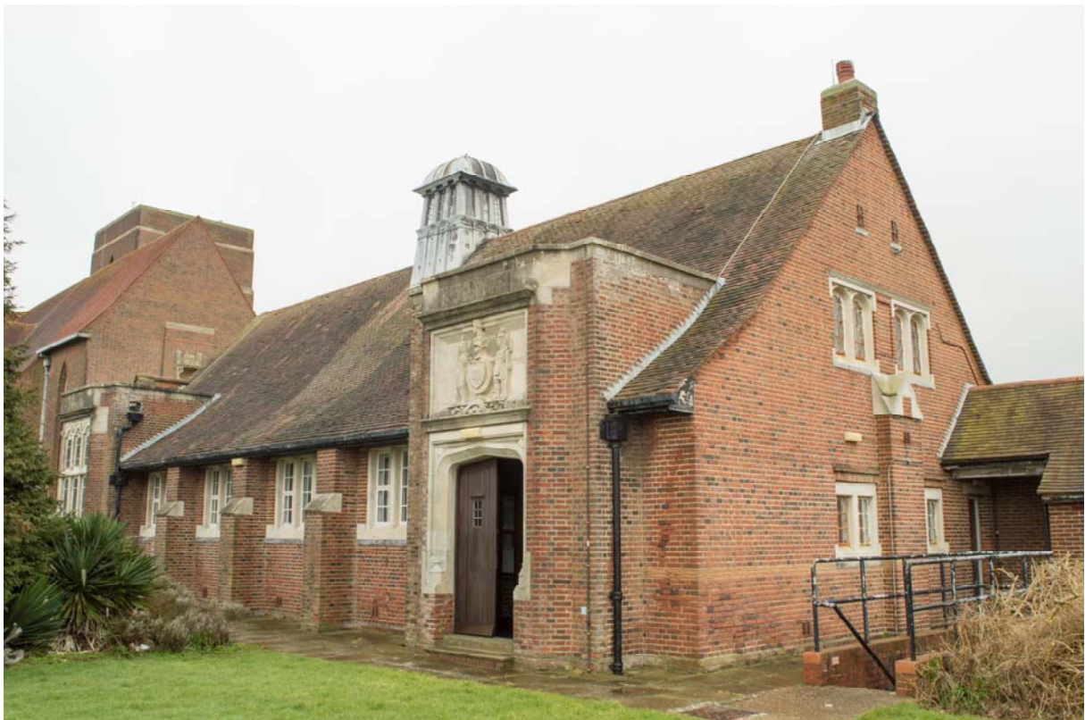
Plate 12 – Building 17: Sir John Moore Library, exterior view looking north-west (SGA15-296)
