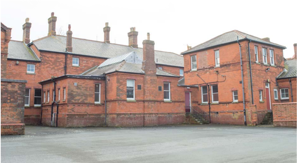
Plate 51 – Building 20: officers' mess, main service wing with billiard room to the left of the image and mess man's accommodation to the right. View looking south-west (SGA15-399)
