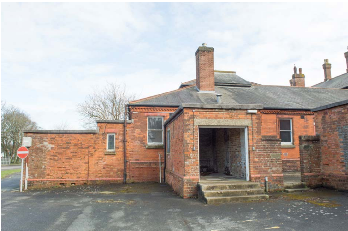
Plate 50 – Building 20: officers' mess, main kitchen with plain stack and former coal store in foreground. View looking east (SGA15-405)
