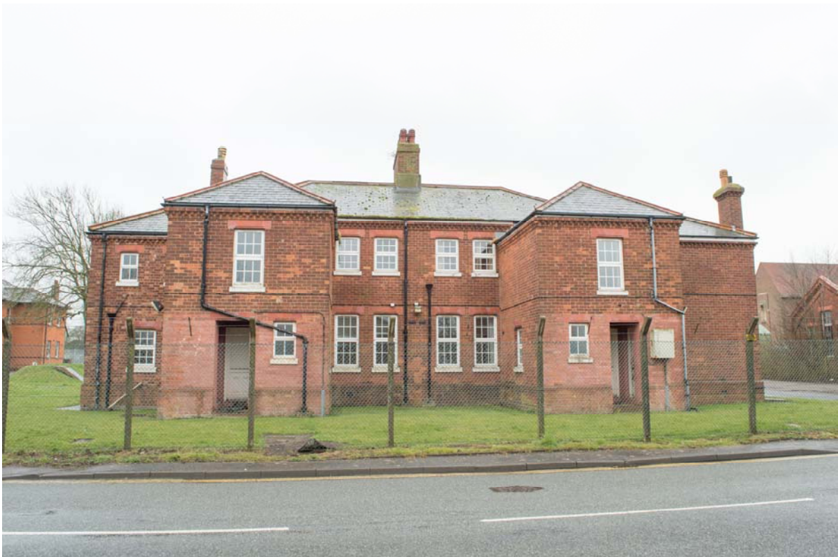
Plate 36 – Building 19: rear elevation, looking south (SGA15-611)
