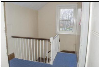
SGA15-0530 Building 20, first floor, service stair. Facing north
