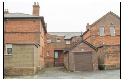
SGA15-0393 Building 20, exterior. Facing south
