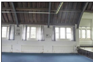
SGA15-0236 Building 17, hall. Facing south
