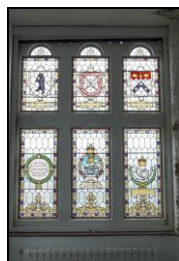
SGA15-0239 Building 17, hall, window detail. Facing north
