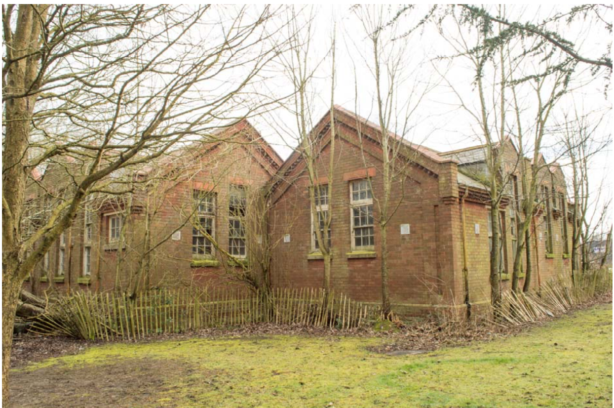
Plate 4 – Building 15: general view of the infants' school, looking south-east (SGA15-364)
