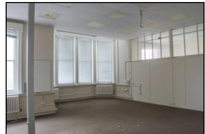
SGA15-0462 Building 20, ground floor, mess room. Facing south-west
