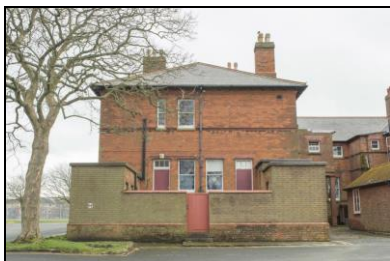
SGA15-0391 Building 20, exterior. Facing south
