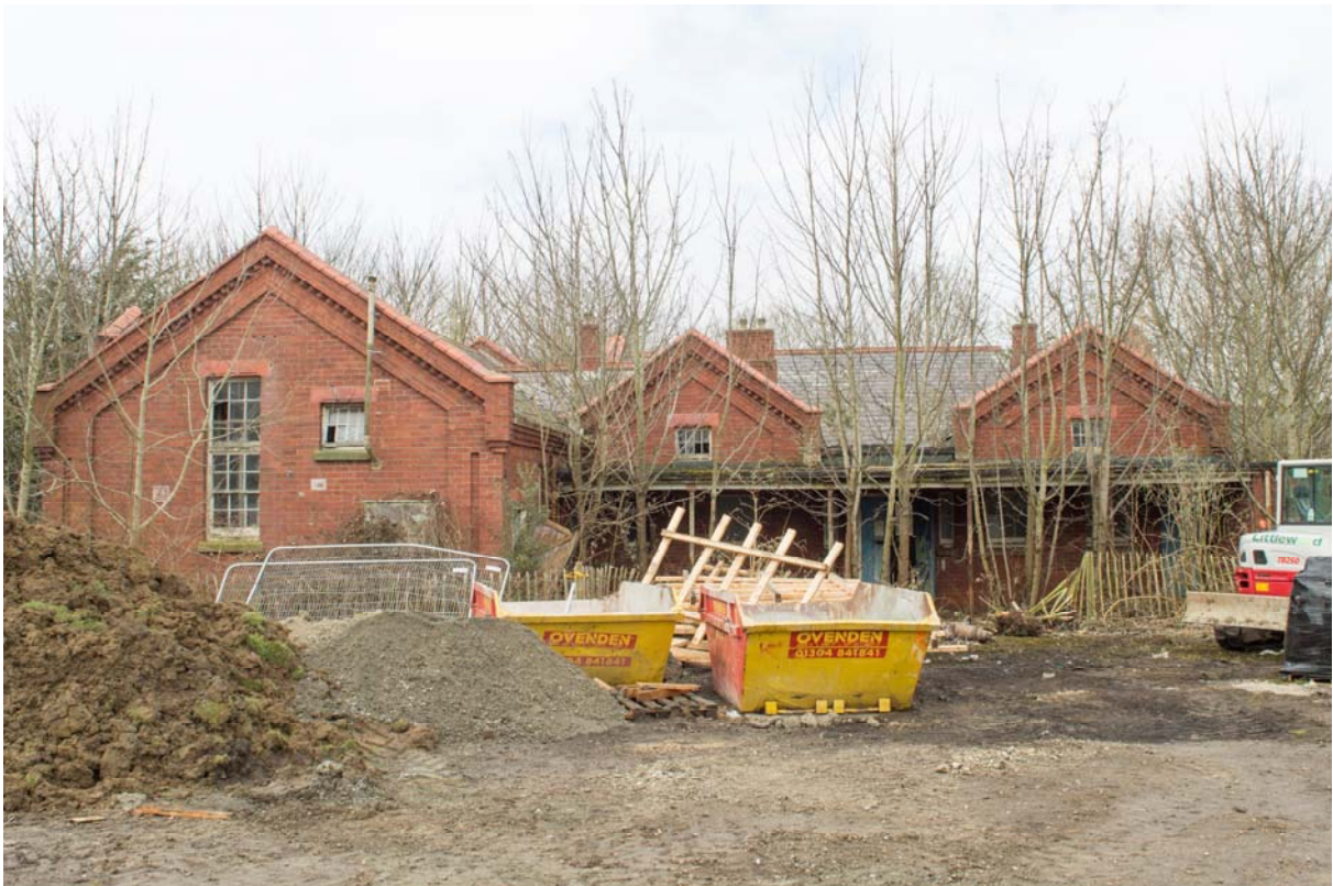
Plate 3 – Building 15: general view of the infants' school, looking north (SGA15-357)
