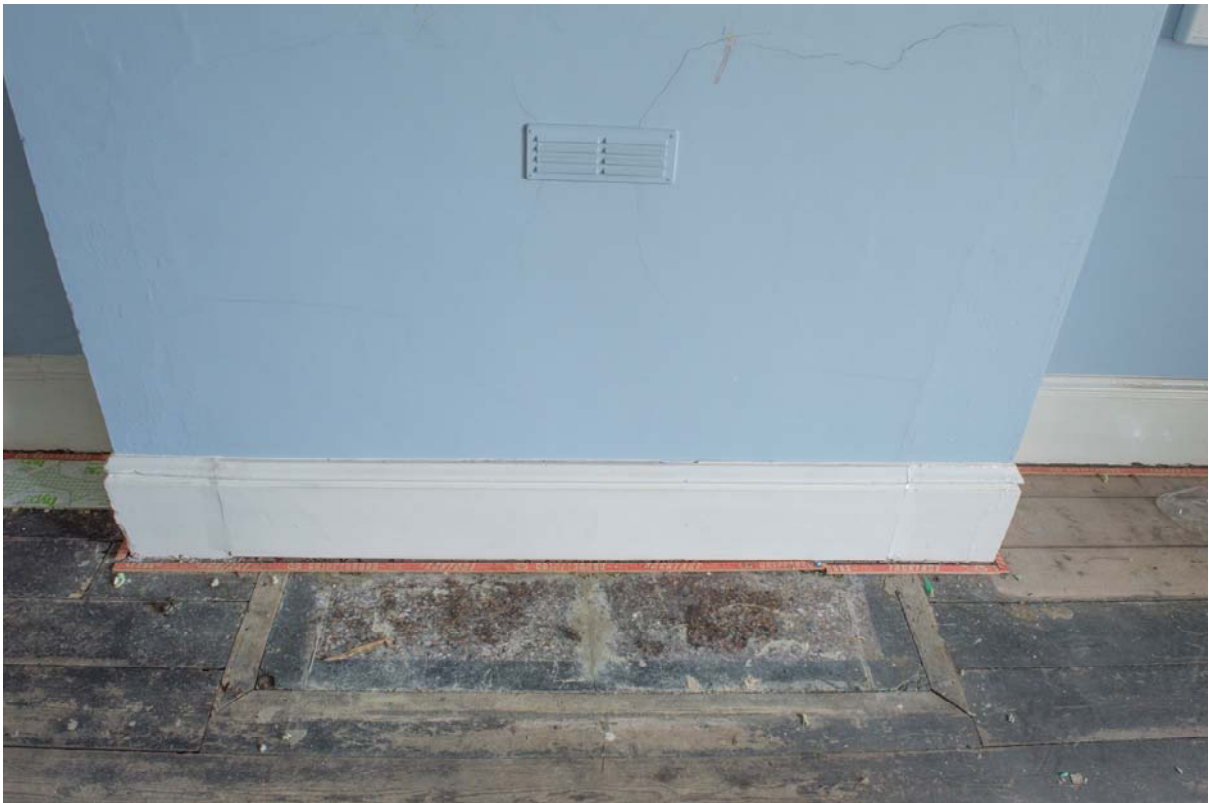
Plate 80 – Building 20: first floor, terrazzo hearthstone to officer's room (SGA15-524)
