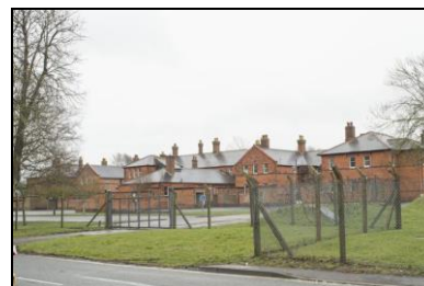
SGA15-0615 Building 20, exterior. Facing south-east
