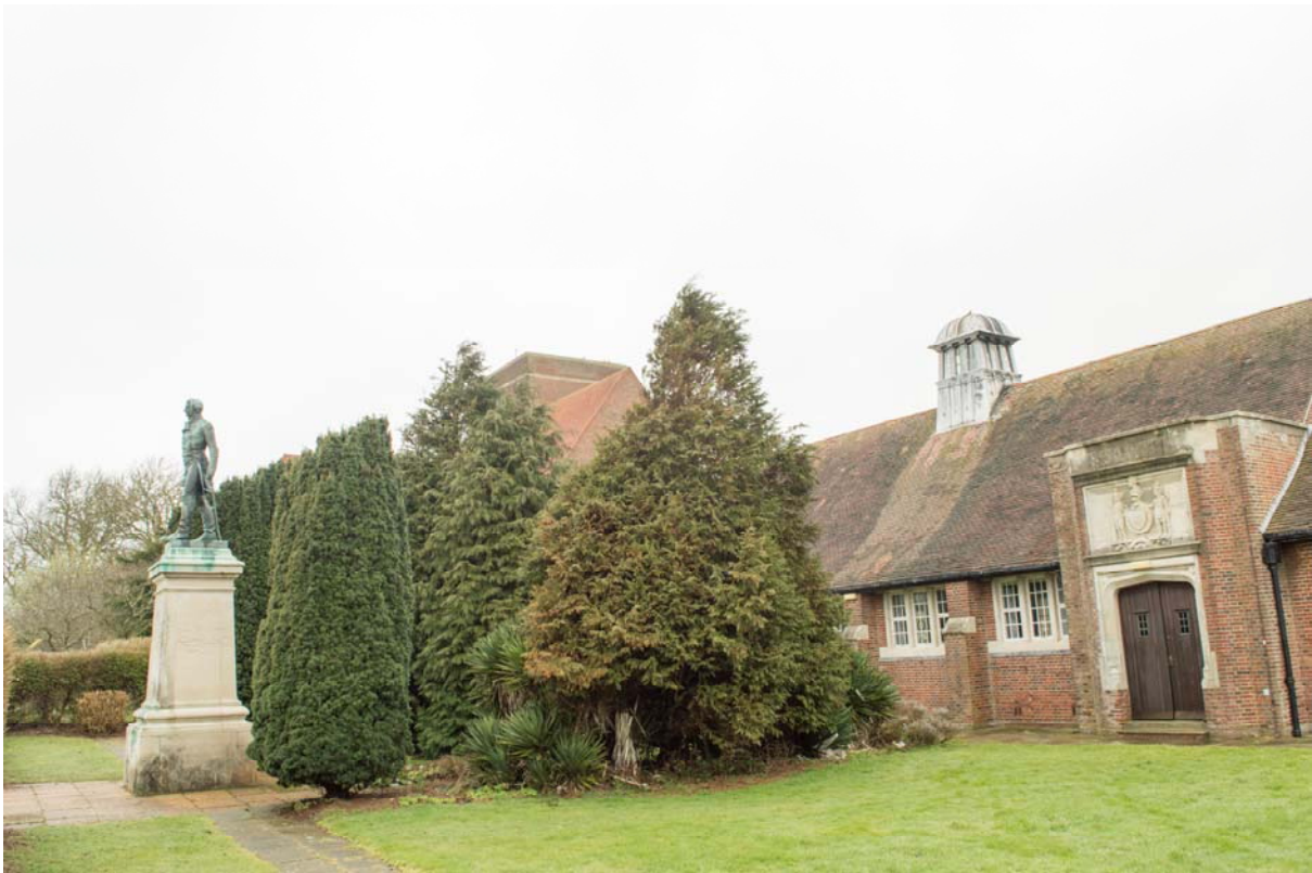
Plate 17 – Building 17: Sir John Moore Library, showing the statue to the front of the building. View looking north-west (SGA15-316)
