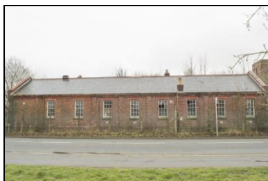
SGA15-0614 Building 15, exterior. Facing south
