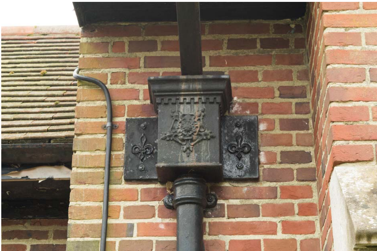
Plate 16 – Building 17: Sir John Moore Library, detail of hopper (SGA15-314)
