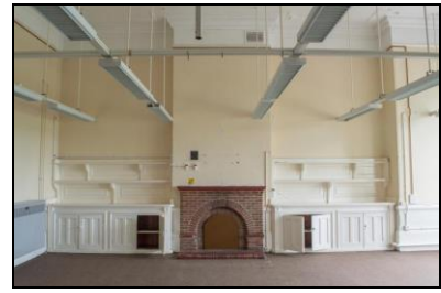
SGA15-0456 Building 20, ground floor, ante room. Facing east
