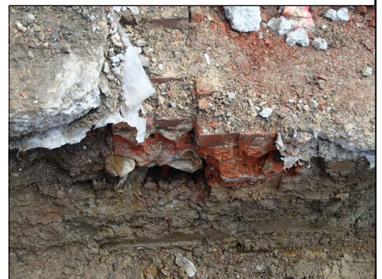
Wall footings 009 and 010
