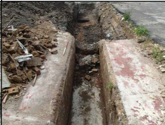
Trench 2, looking west
