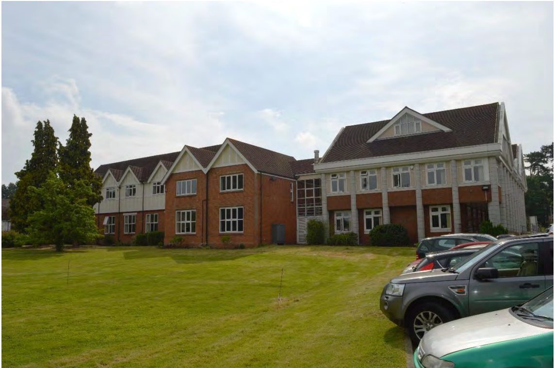
North-west elevation of the main college building, facing east (2)
