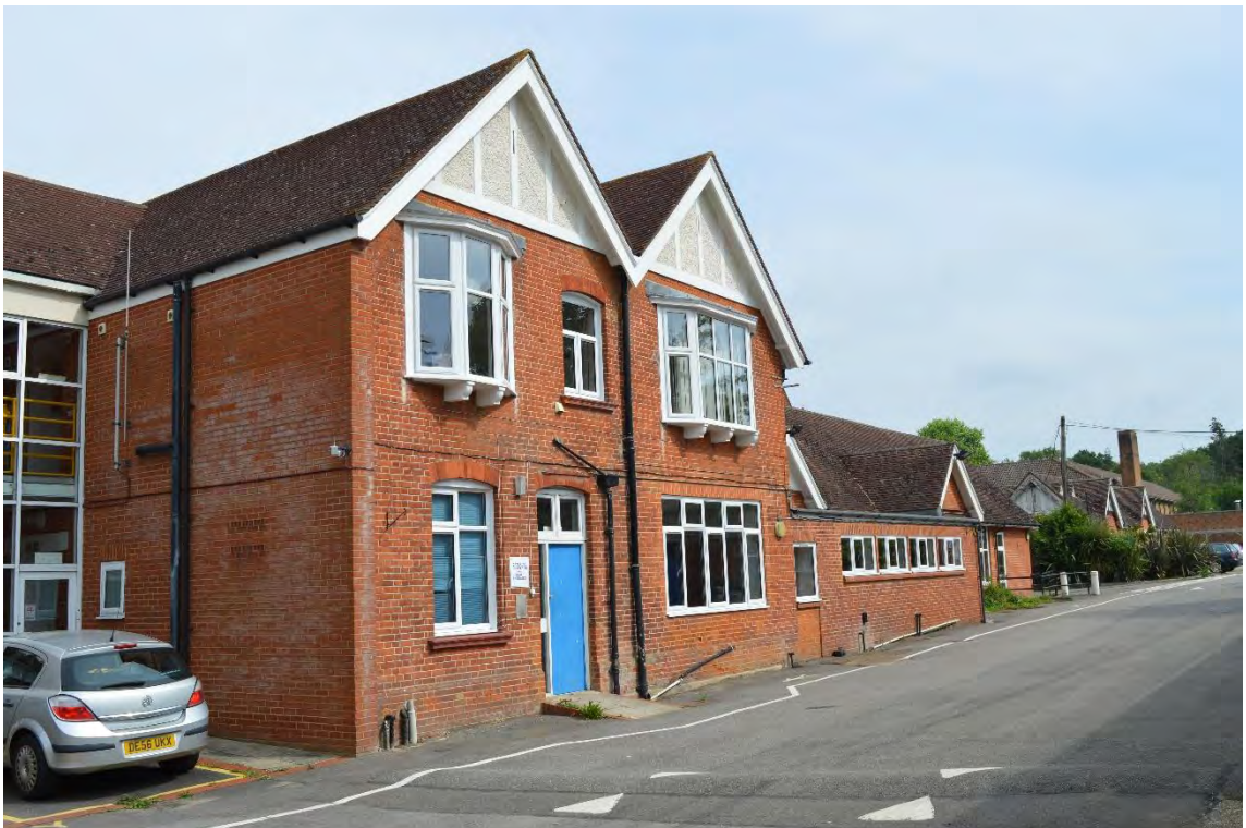
South-east elevation of the main college building, facing north (11)
