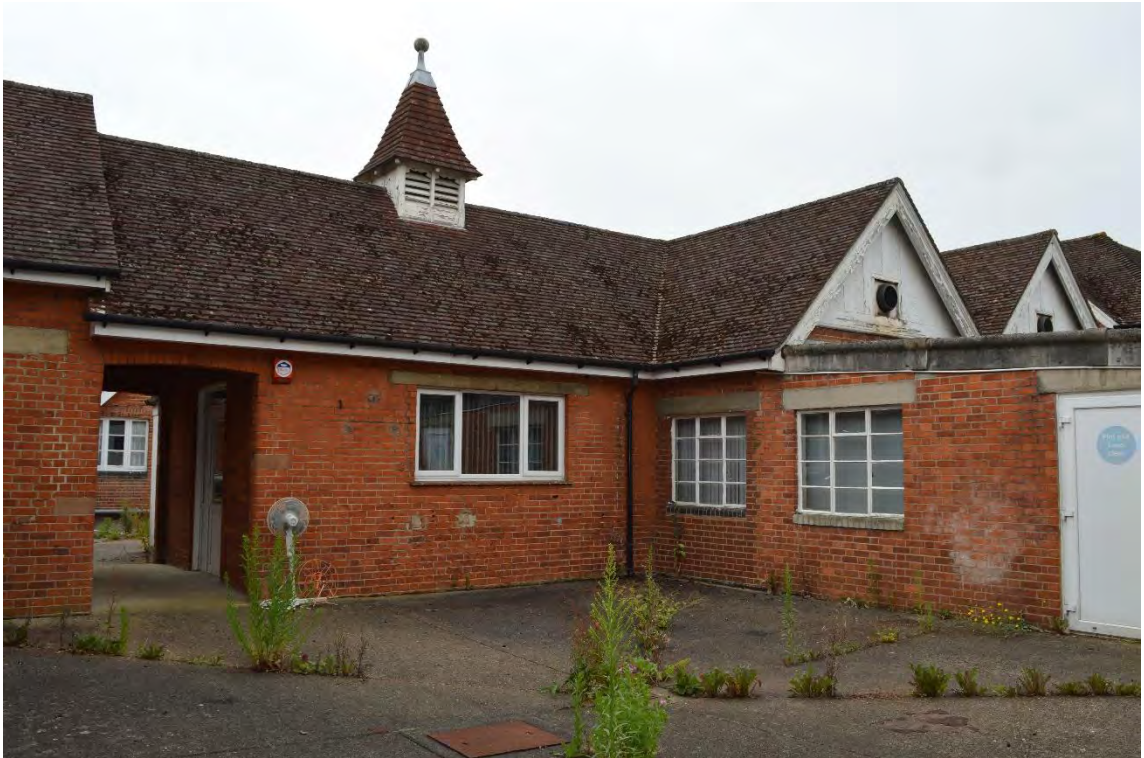
View of the north-west elevation of the central projection of the rear block, facing south (28)
