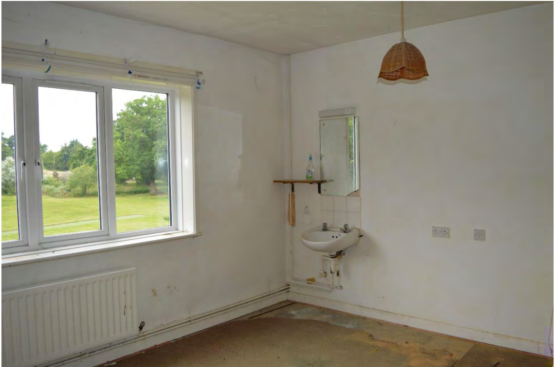
View of the disused accommodation at first floor level within the main college building's north-west range, facing north (55)
