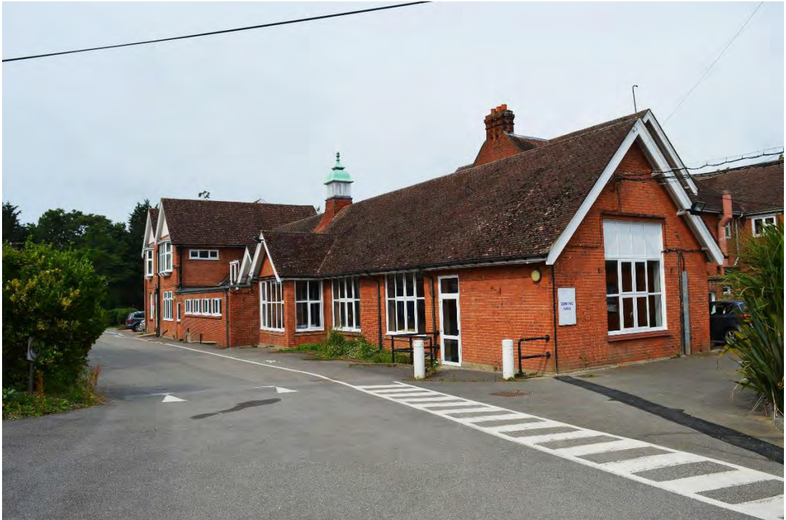
South-east elevation of the main college building, facing west (9)
