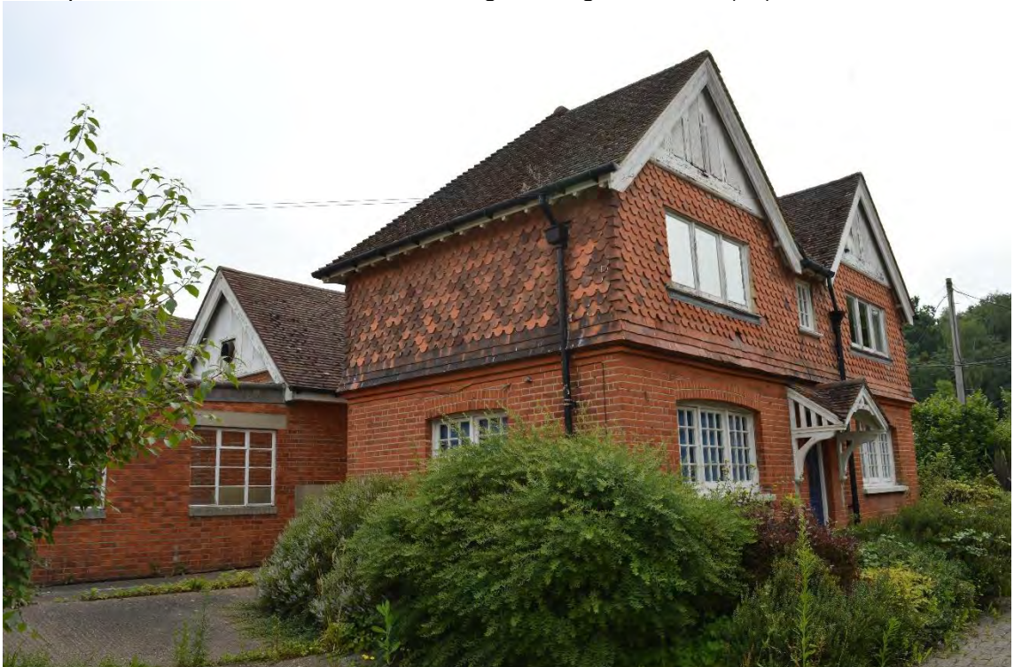
North-west elevation of the cottage, facing east (24)
