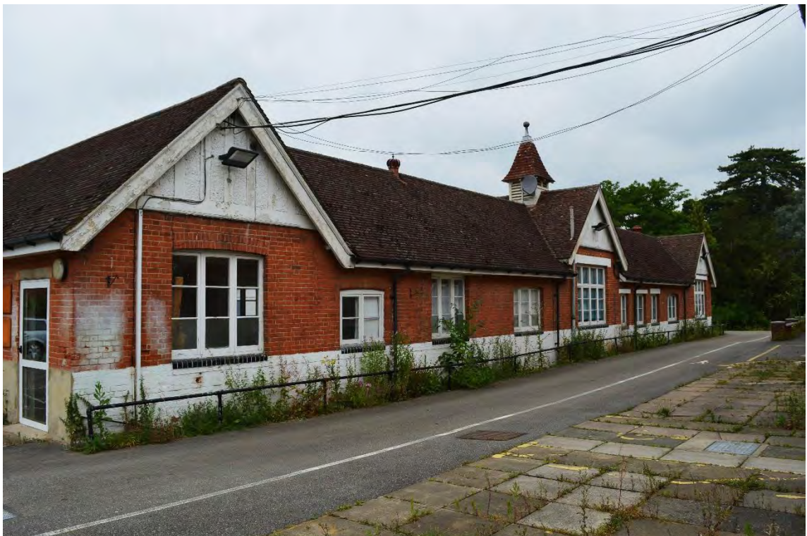
North-east elevation of the rear range, facing north-west (43)
