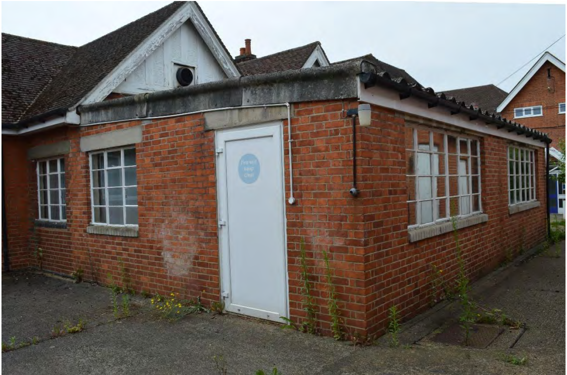
Plate 27: North-west yard and extension, facing south-west (27)
