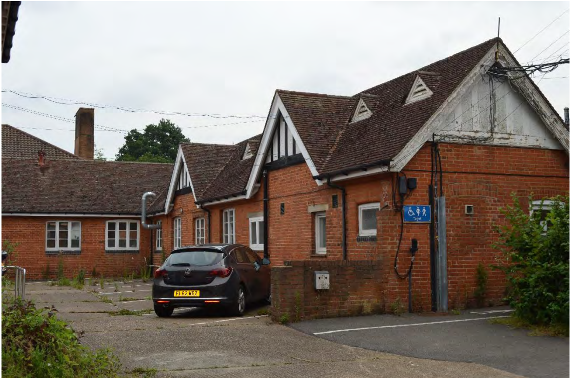
View of the south-east courtyard, facing north-east (36)
