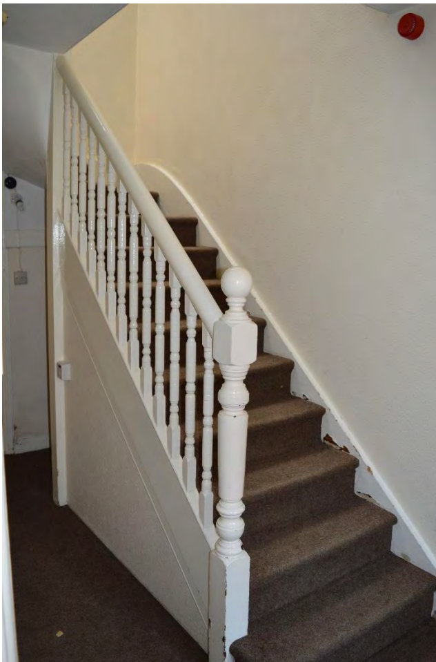
The central staircase within the cottage, facing north-east (68)
