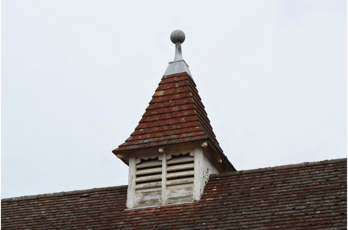
Detail of the lantern found upon the central projection of the rear block, facing north-west (34)
