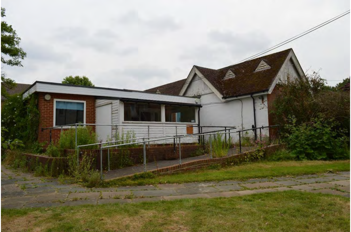
South-west end of the rear block's north-west range, facing north-east (48)
