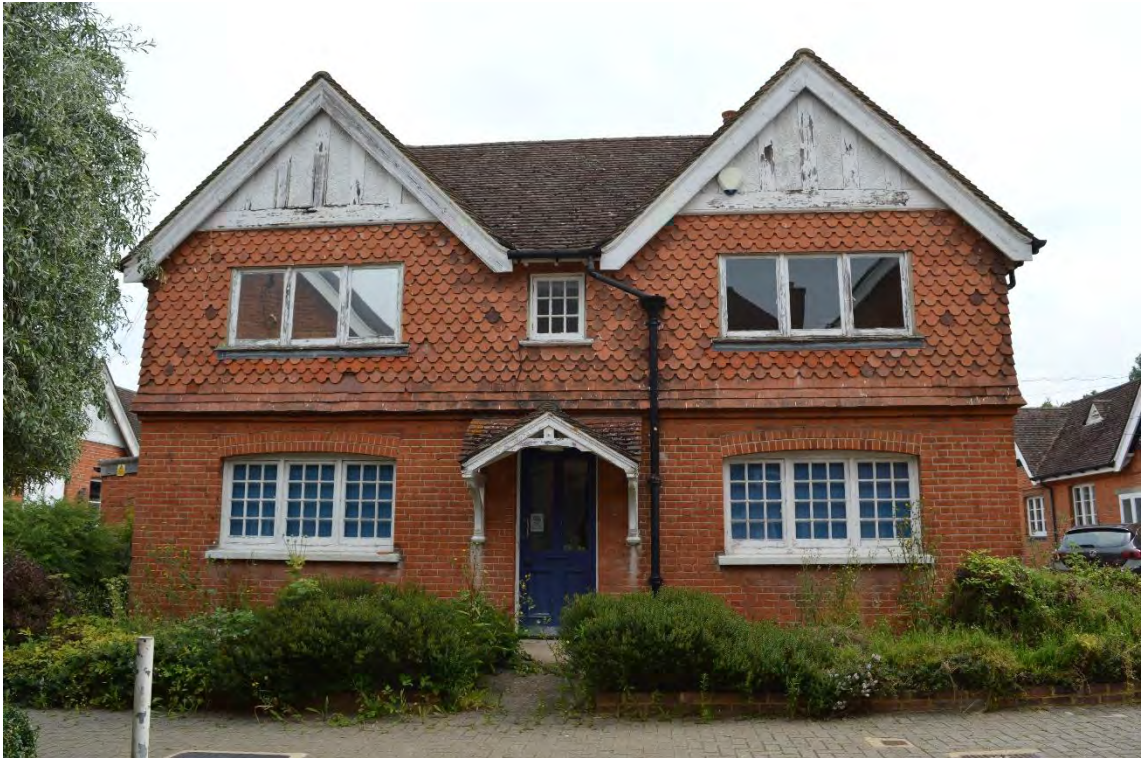
Principal south-west elevation of the cottage, facing north-east (20)
