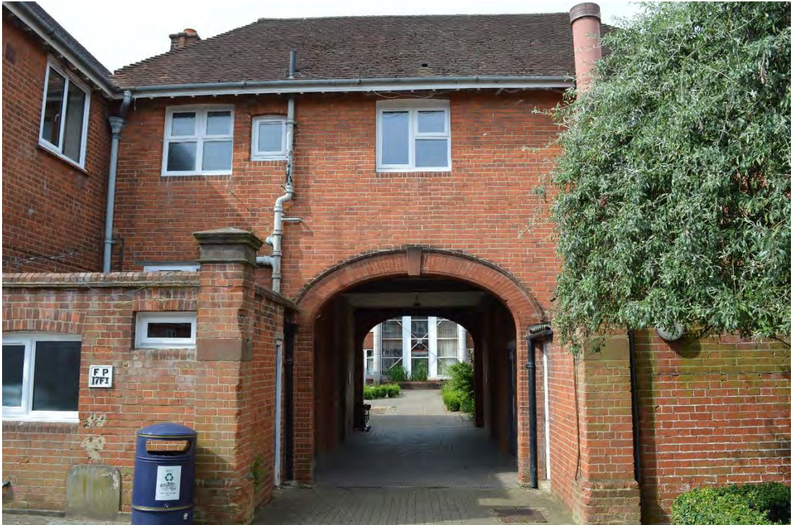
Central range and passageway within the rear block, facing south-west (5)
