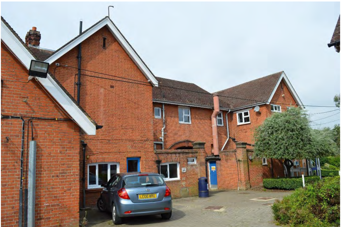
Rear block, facing west (7)
