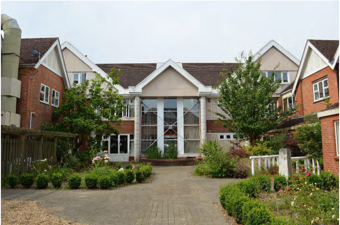
View of the internal courtyard within the main college building, facing south-west towards the modern entrance building (17)
