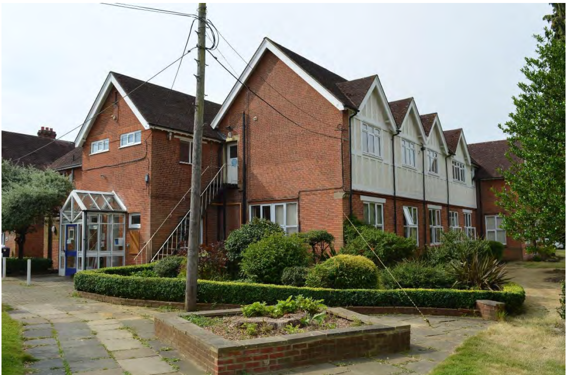
Northern corner of the main college building, facing south (3)
