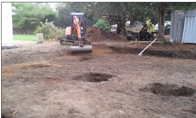
F. View over site following ground reduction (looking south-east)
