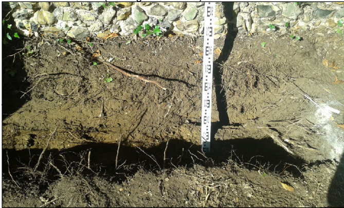
E. Section of footing trench by the garden wall
