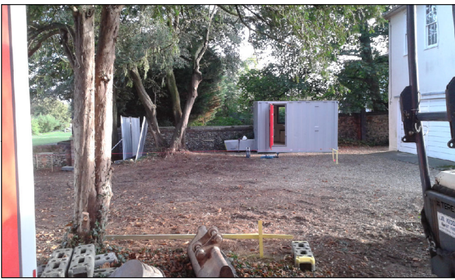
A. Pre excavation view of the site (looking north)
