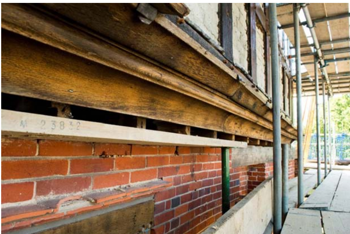
Plate 30: Jetty soffit on west elevation (#BCA16-0088)
