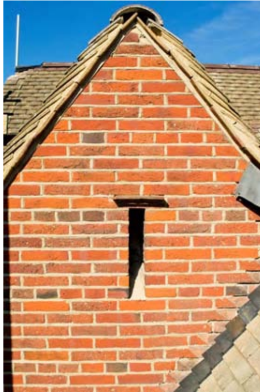
Plate 19: Set-back gable on east elevation, east wing (#BCA16-0133)
