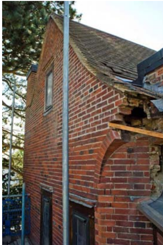
Plate 16: Arch on second floor (#BCA16-0153)
