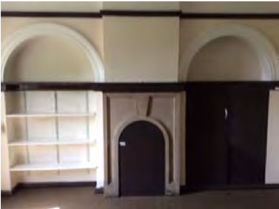
Plate 52: Fireplace and arched alcoves in former east-wing bedroom (photo provided by London Square) (#BCA16-0243)
