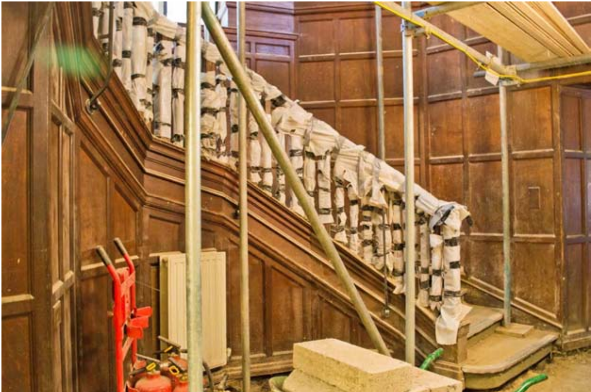
Plate 45: The Main Staircase (#BCA16-0176)
