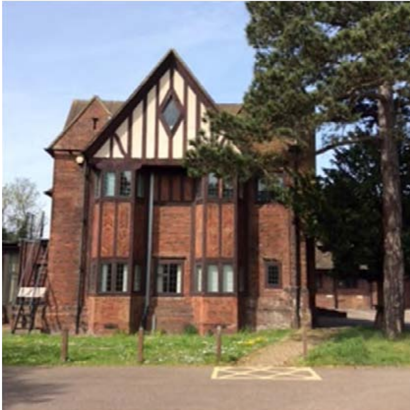
Plate 17: East elevation of the east wing (photo provided by London Square) (#BCA16-0235)
