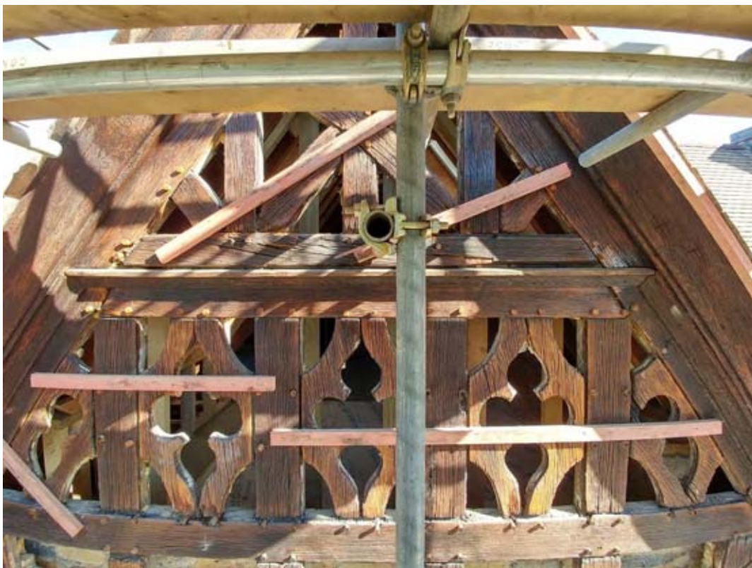
Plate 22: Central south gable detail (#BCA16-0018)
