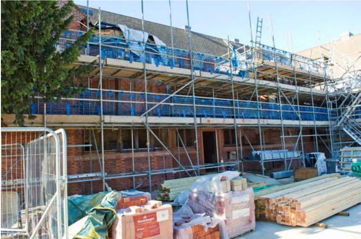
Plate 13: North elevation, east wing (#BCA16-0022)
