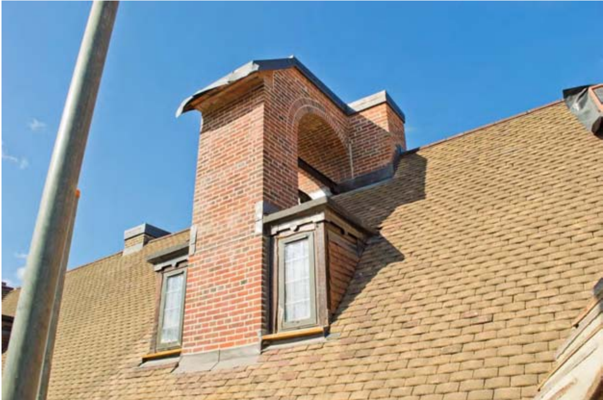
Plate 39: Flying buttress chimney (#BCA16-0147)
