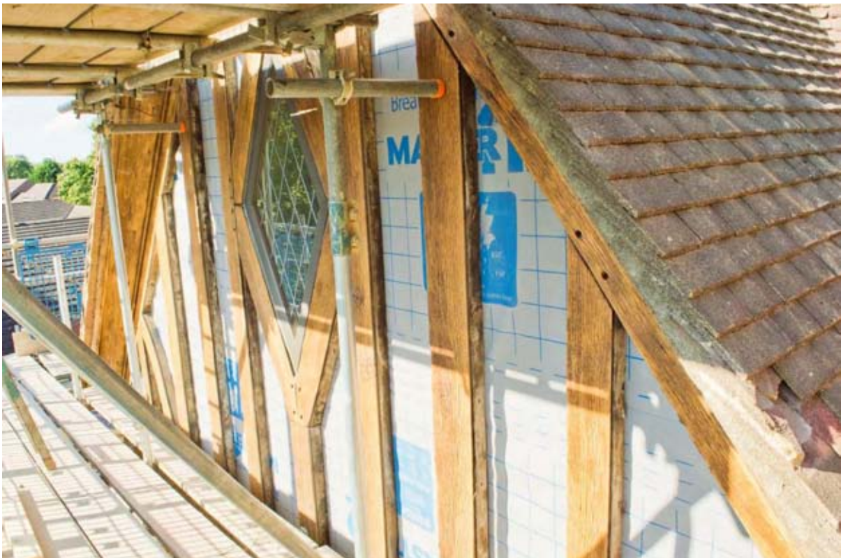
Plate 18: Half-timbering in gable of east elevation of east wing (#BCA16-0129)
