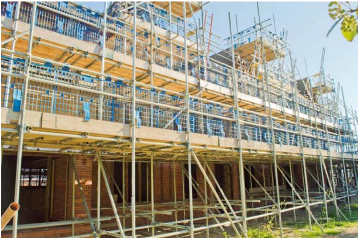
Plate 20: South elevation of Bassets House (#BCA16-0057)
