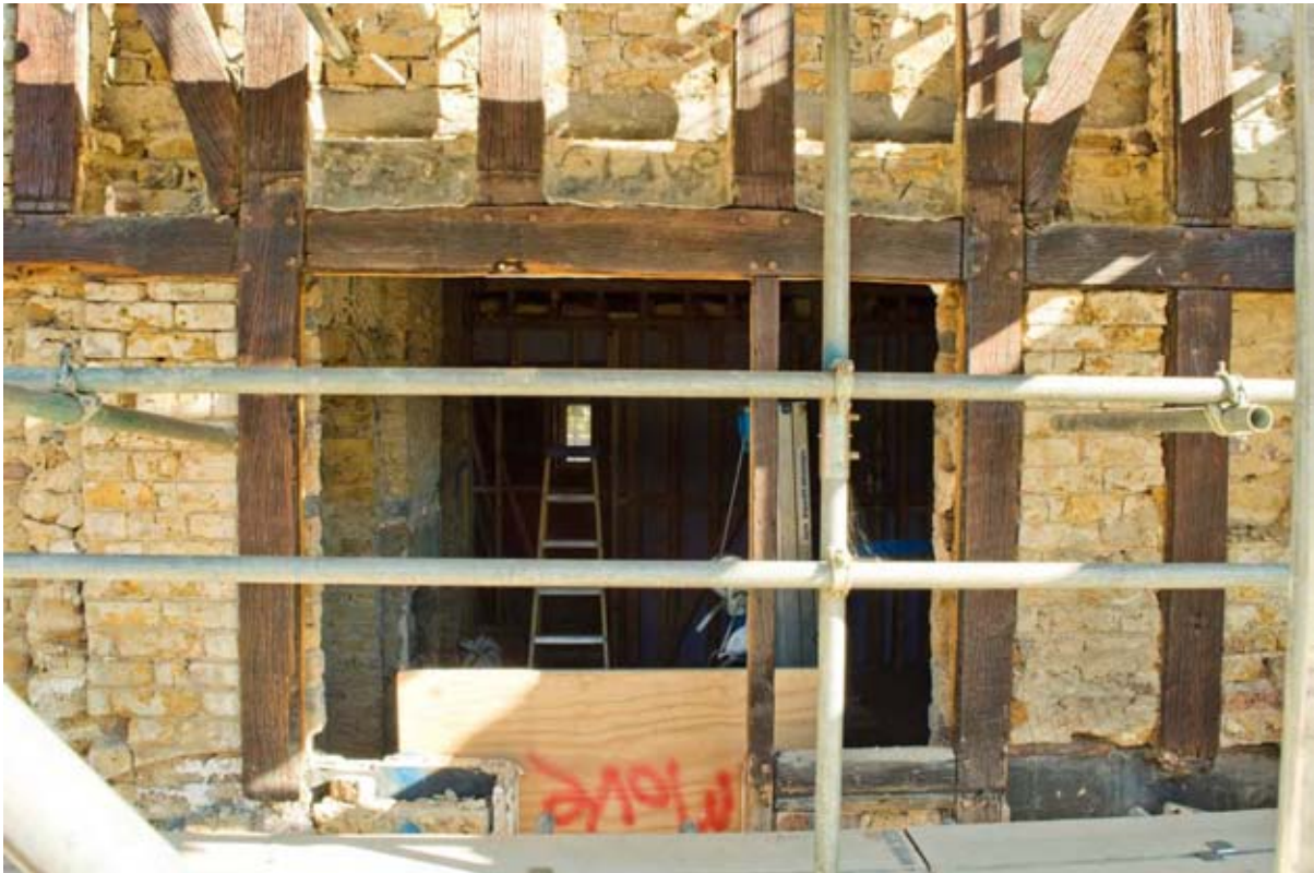
Plate 3: Buff brick exposed behind formerly rendered panels (#BCA16-0114)
