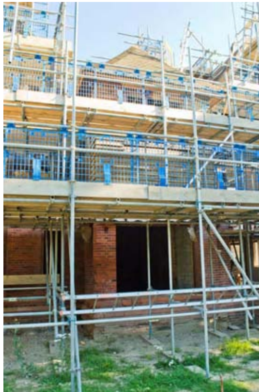
Plate 26: Hipped roof section of the south elevation (#BCA16-0059)
