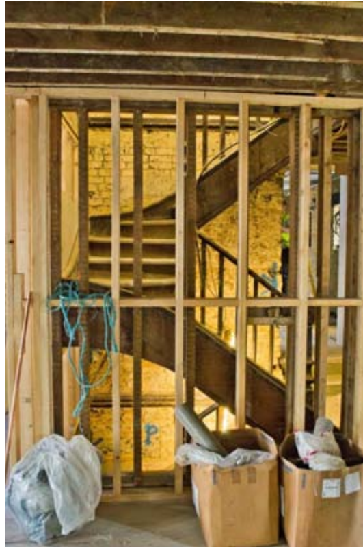
Plate 61: Servant's Stair, exposed beyond stripped back stud walls (#BCA16-0200)
