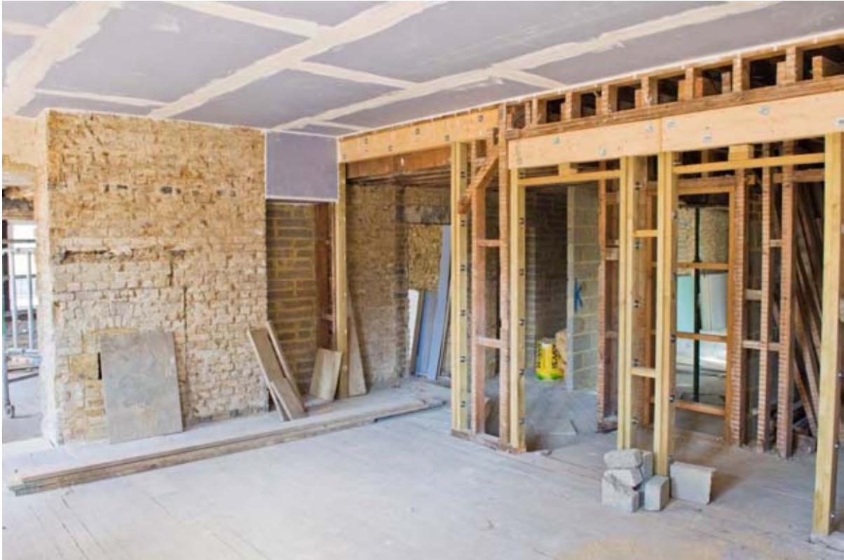
Plate 55: Former east-wing bedroom, west of the hall (#BCA16-0192)
