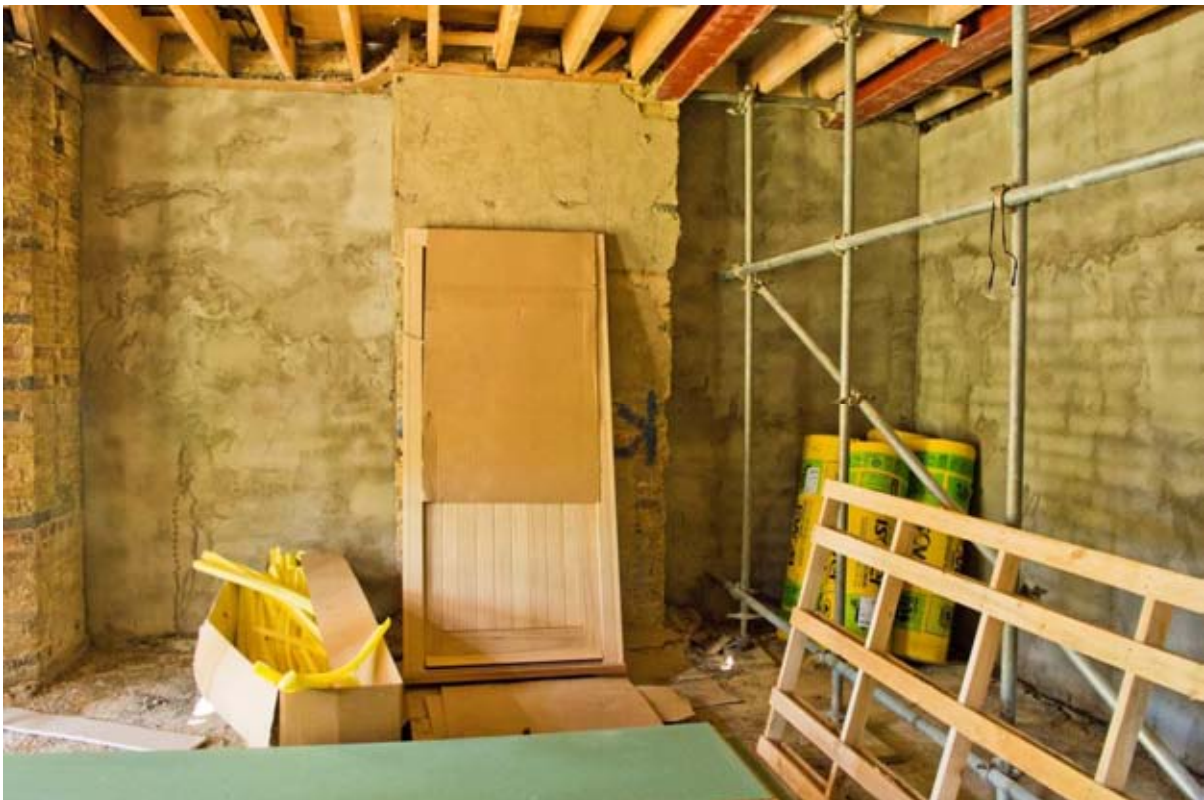
Plate 46: Former Hall – note inserted floor above (#BCA16-0163)
