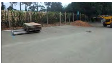
BCA16-0244 General Trench 1. Facing north-east
