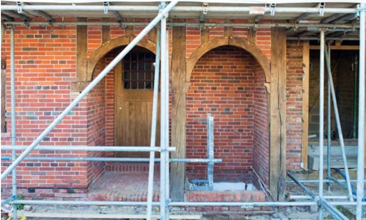
Plate 34: Oak arches to service hatch and doorway (#BCA16-0043)
