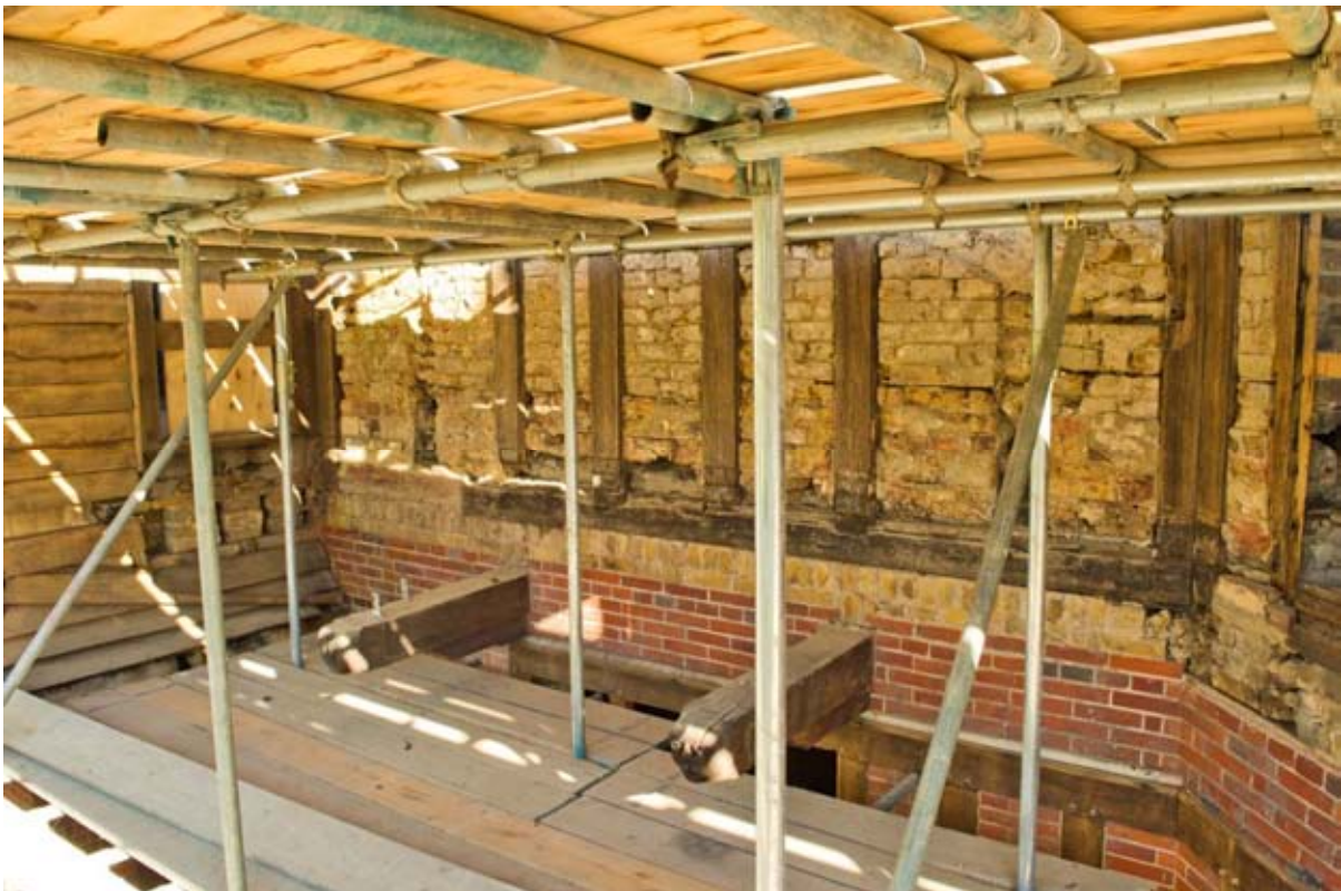
Plate 24: Oak beams with grotesques, former balcony supports. (#BCA16-0075)
