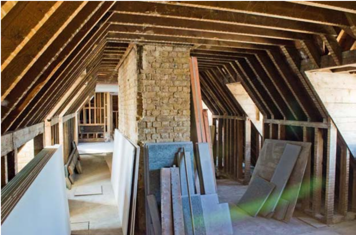
Plate 60: Overview of second floor level of north wing (#BCA16-0215)
