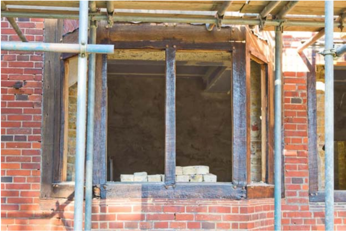
Plate 1: Window detail, east elevation, east wing (#BCA16-0020)
