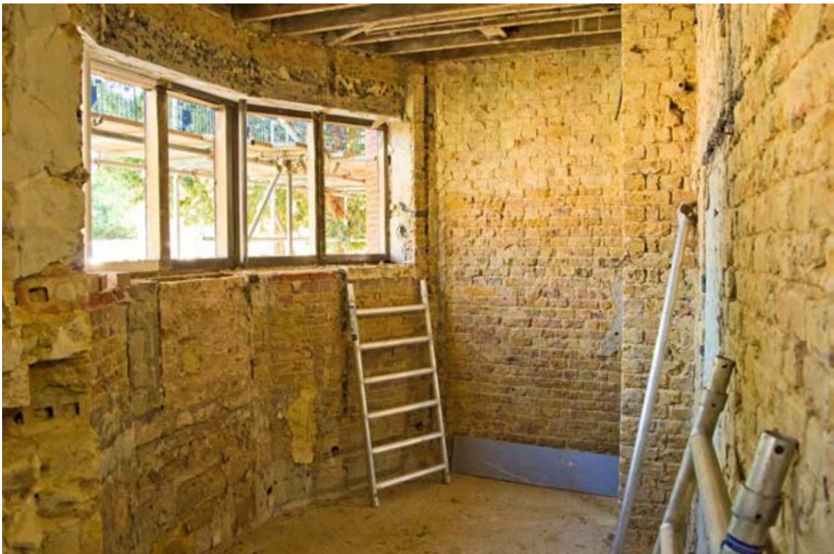
Plate 40: Former toilet (#BCA16-0166)
