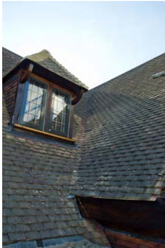
Plate 12: Valley and ridge tiles on roof (#BCA16-0104)
