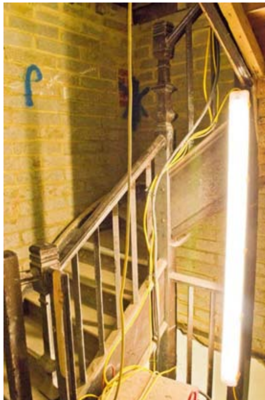
Plate 62: Servant's Stair (#BCA16-0210)
