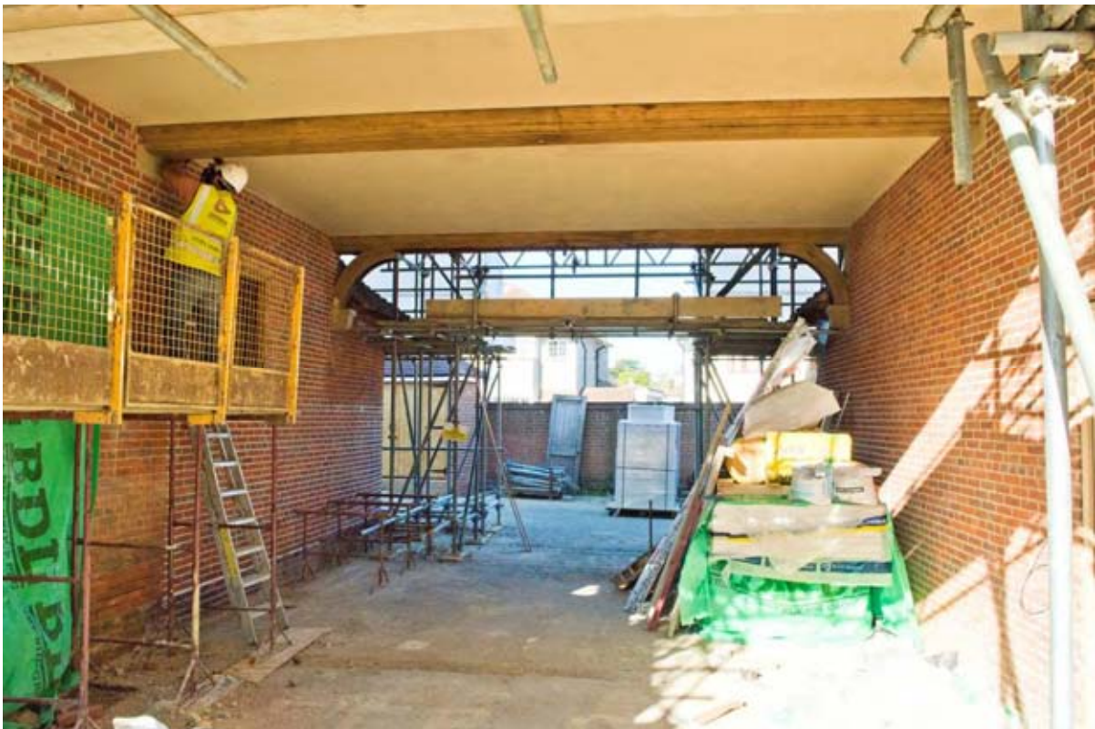
Plate 32: Overview of the covered drive (#BCA16-0031)
