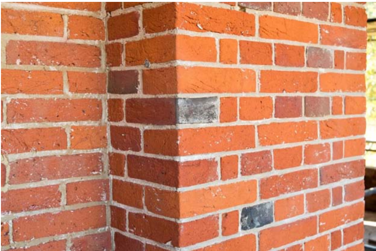
Plate 2: Detail of brickwork showing signs of clamp firing (#BCA16-0052)
