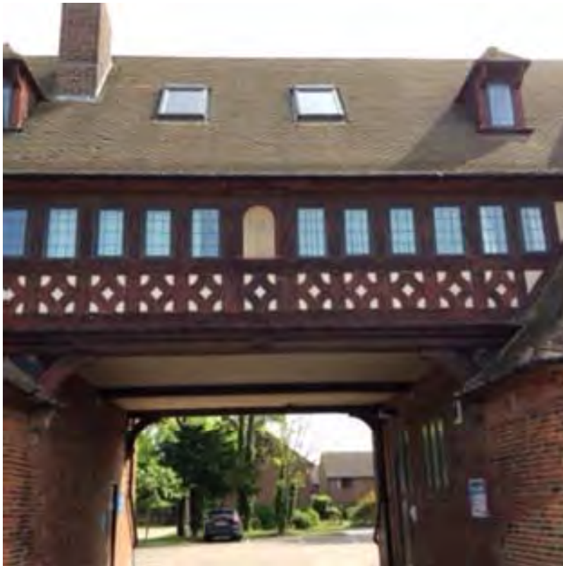
Plate 31: West elevation of the gantry (photo provided by London Square) (#BCA16-0237)
