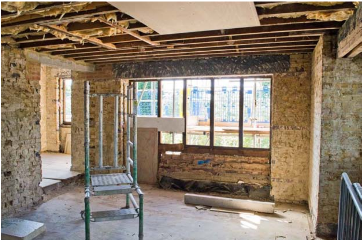
Plate 56: Former western-most east-wing bedroom (#BCA16-0195)
