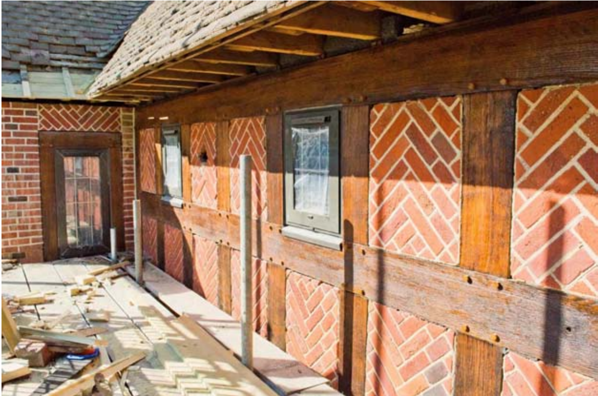
Plate 11: Timber soffit to eaves (#BCA16-0148)
