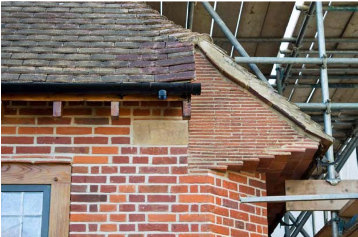
Plate 10: Tiled soffit to eaves (#BCA16-0040)
