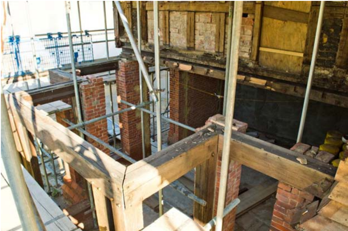
Plate 7: Oak timber structural members (#BCA16-0080)
