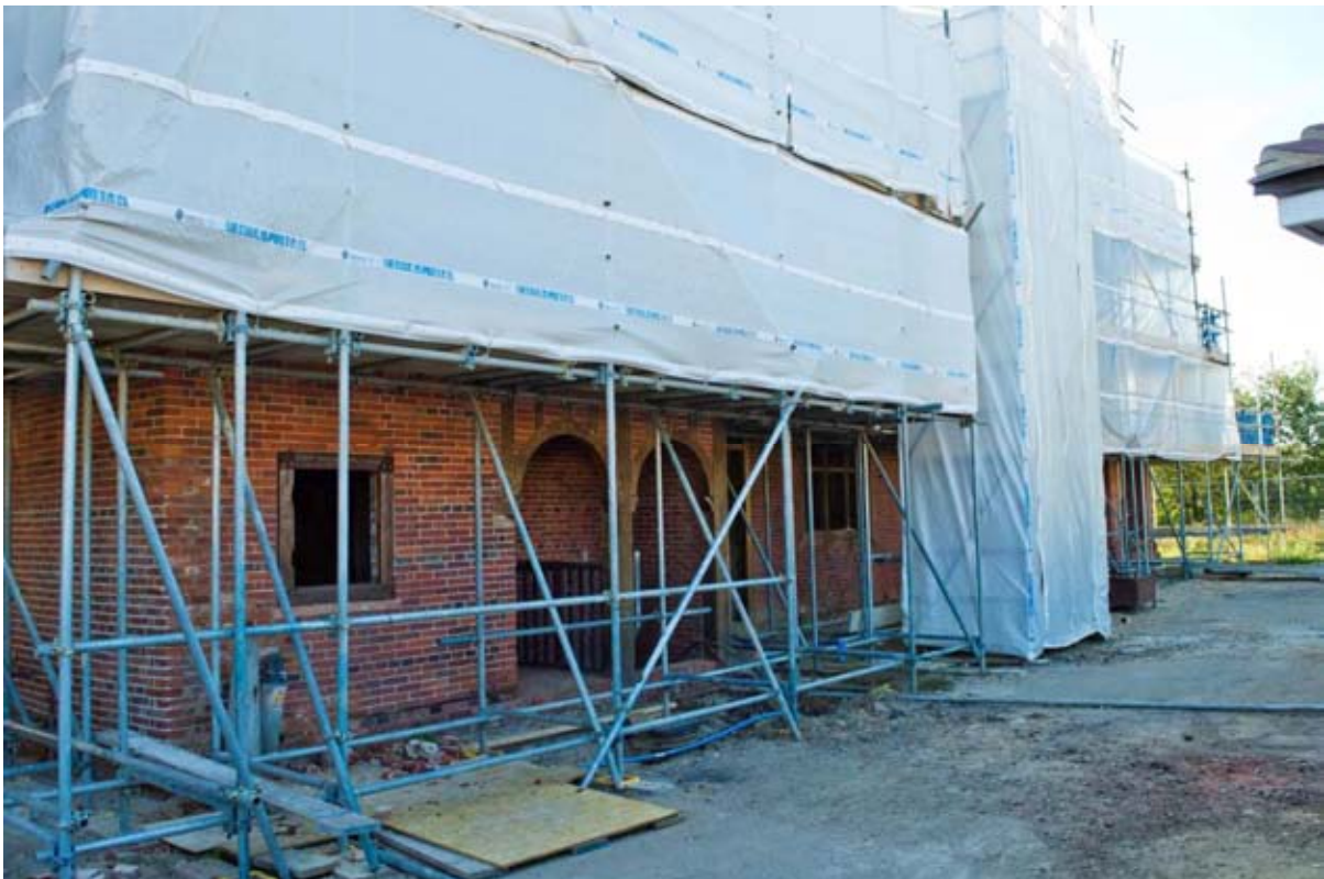
Plate 28: West elevation, south of the covered driveway (#BCA16-0037)
