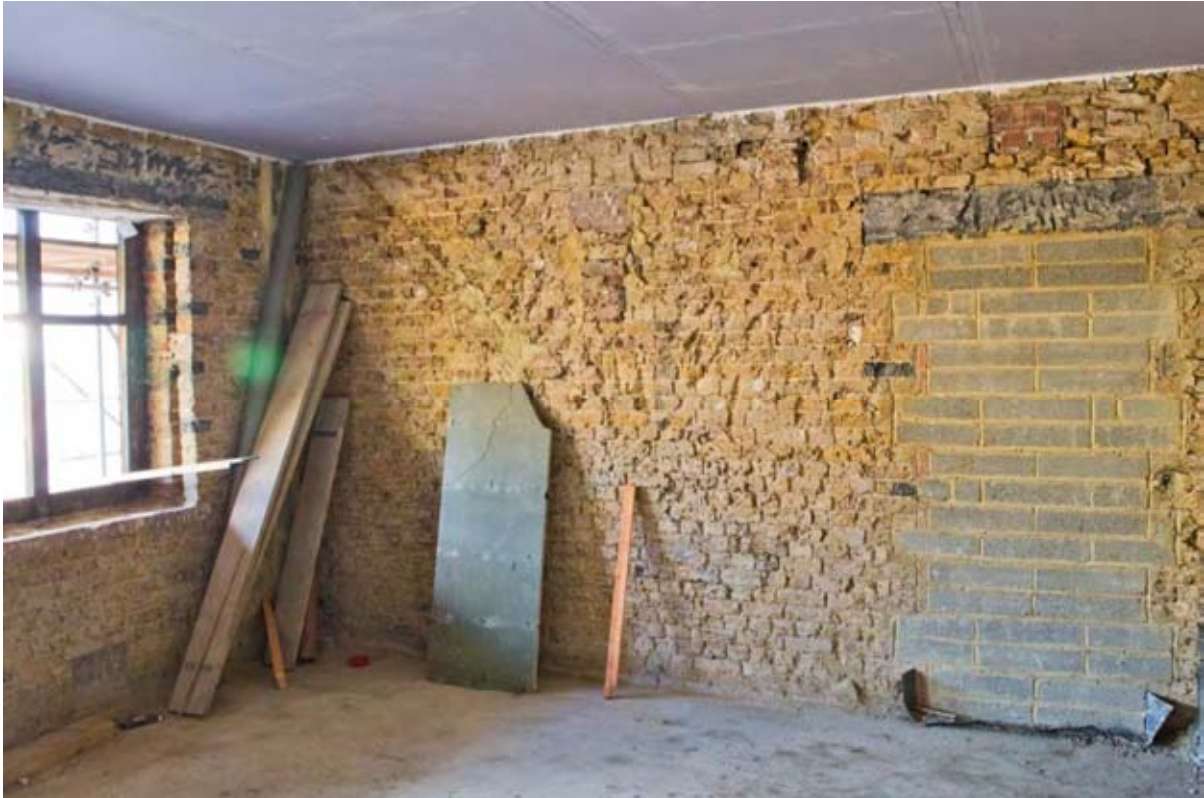
Plate 57: A typical north wing ground-floor room (#BCA16-0184)
