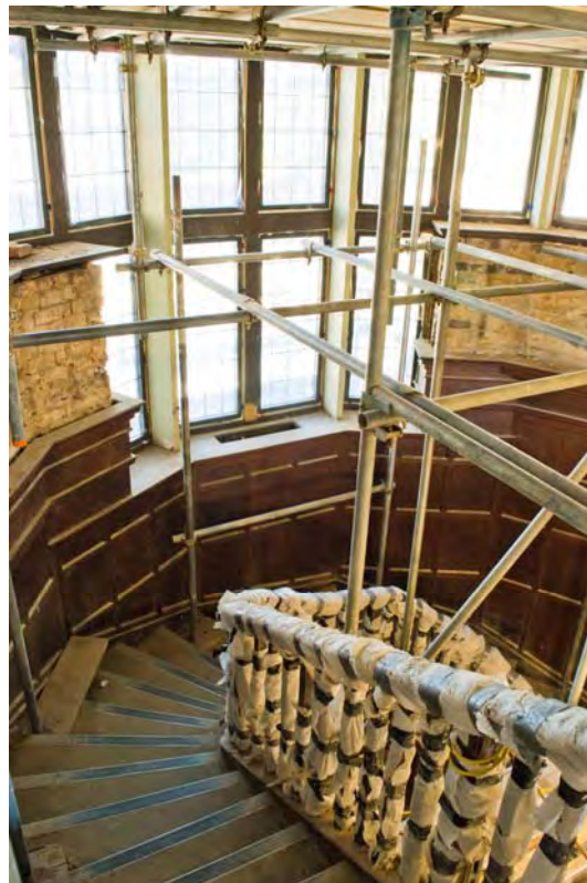
Plate 48: Overview of the Main Staircase from the first-floor landing (#BCA16-0191)
