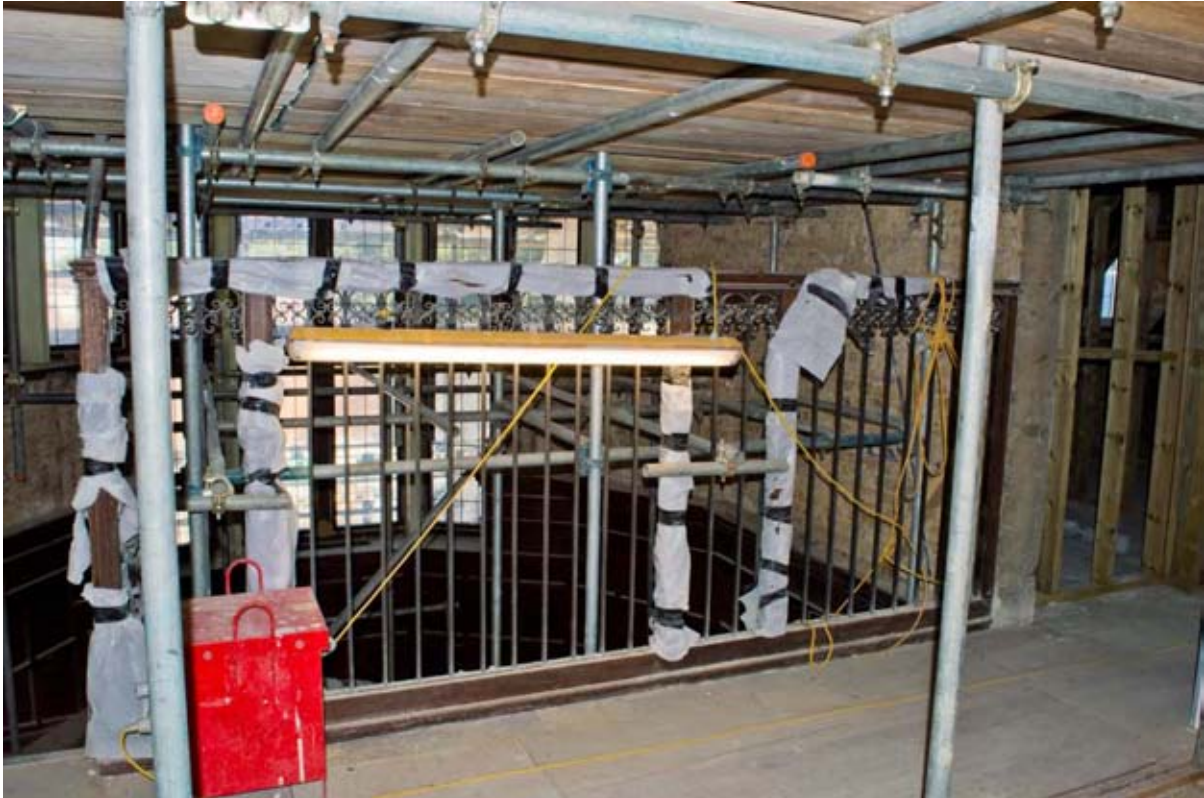
Plate 49: Extant landing railing (#BCA16-0223)
