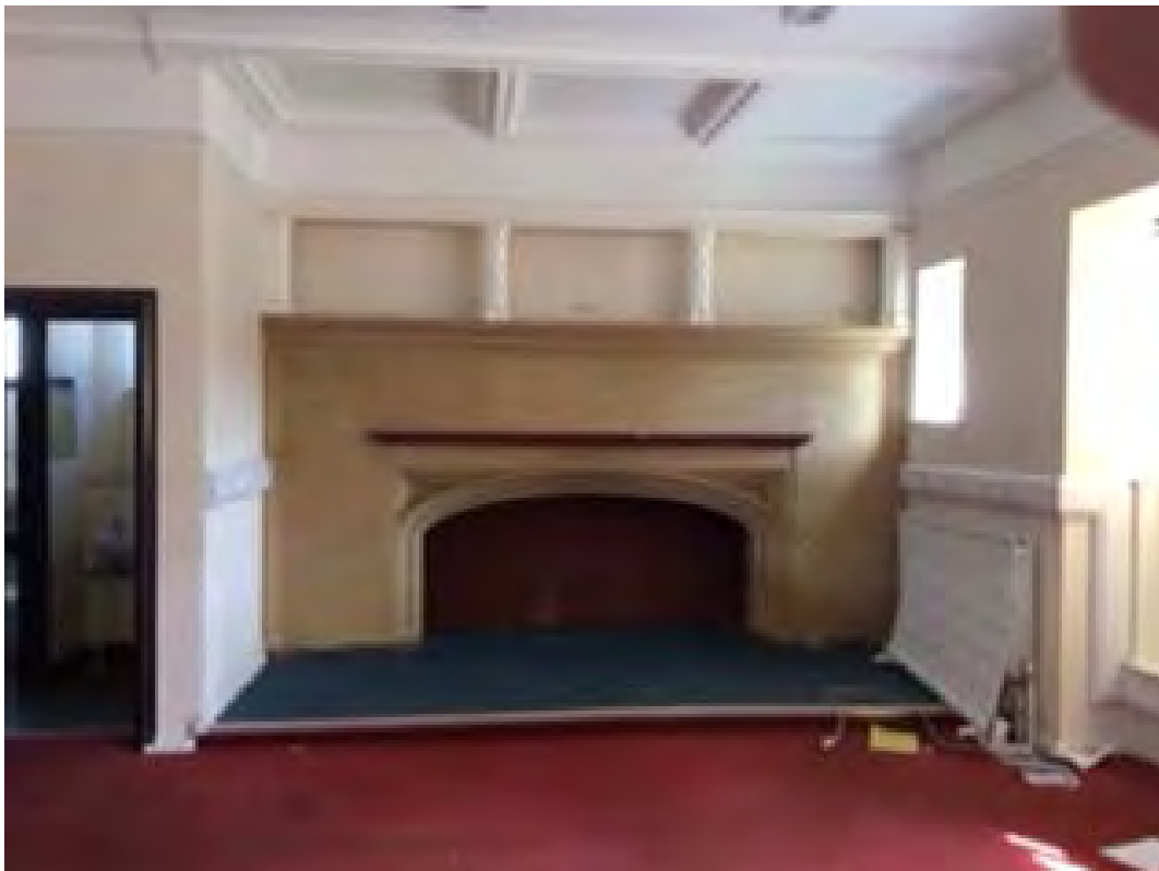
Plate 42: Former Billiard Room (photo provided by London Square) (#BCA16-0239)
