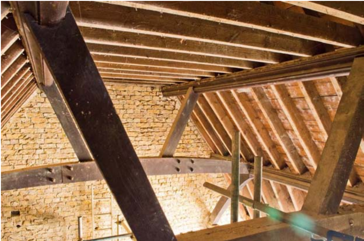
Plate 50: Composite trusses above former hall (#BCA16-0219)
