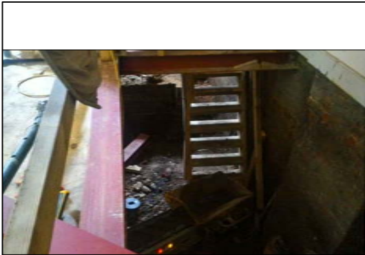
View east into the basement
