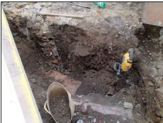
Made ground deposits
