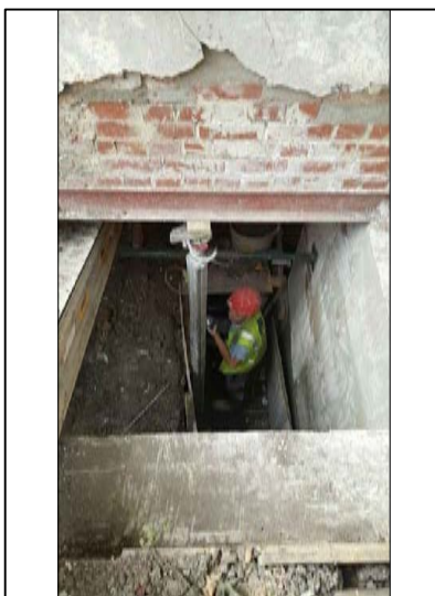
View south into the basement
