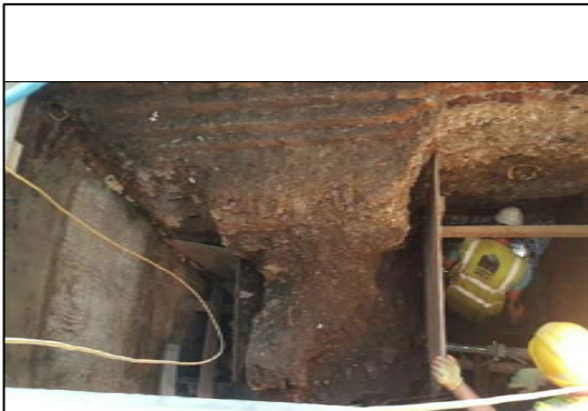
View east into the basement
