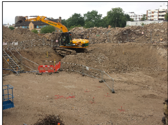
View south-west into block F
