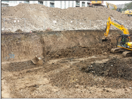
View north-west into block F
