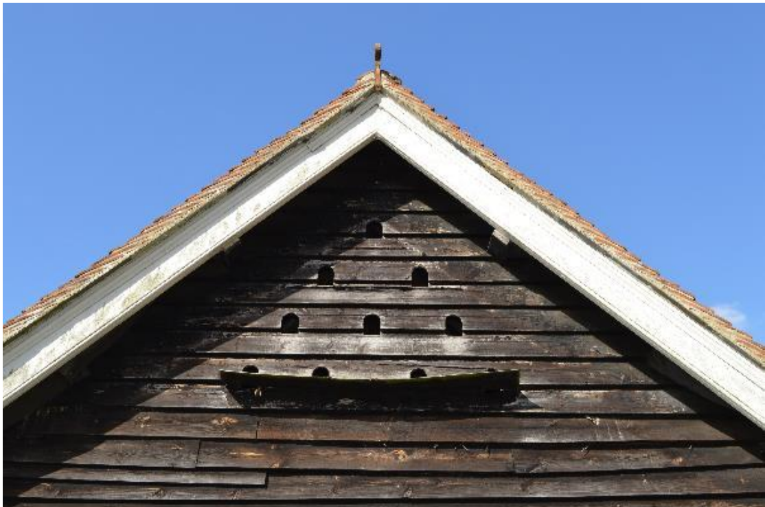
Plate 22 Dovecote arched openings within the south elevation of the wagon porch, facing north (41)
