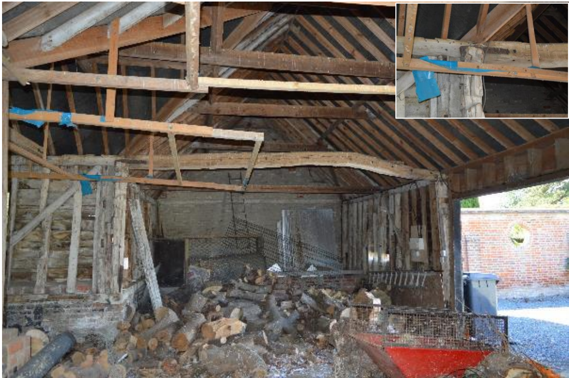
Plate 10 Tie beam construction with iron strap and staples, facing west (36 & 12)
