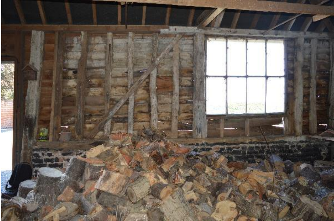
Plate 19 North side of Bays 2 and 3 showing replacement wall plate, facing north-east (26)
