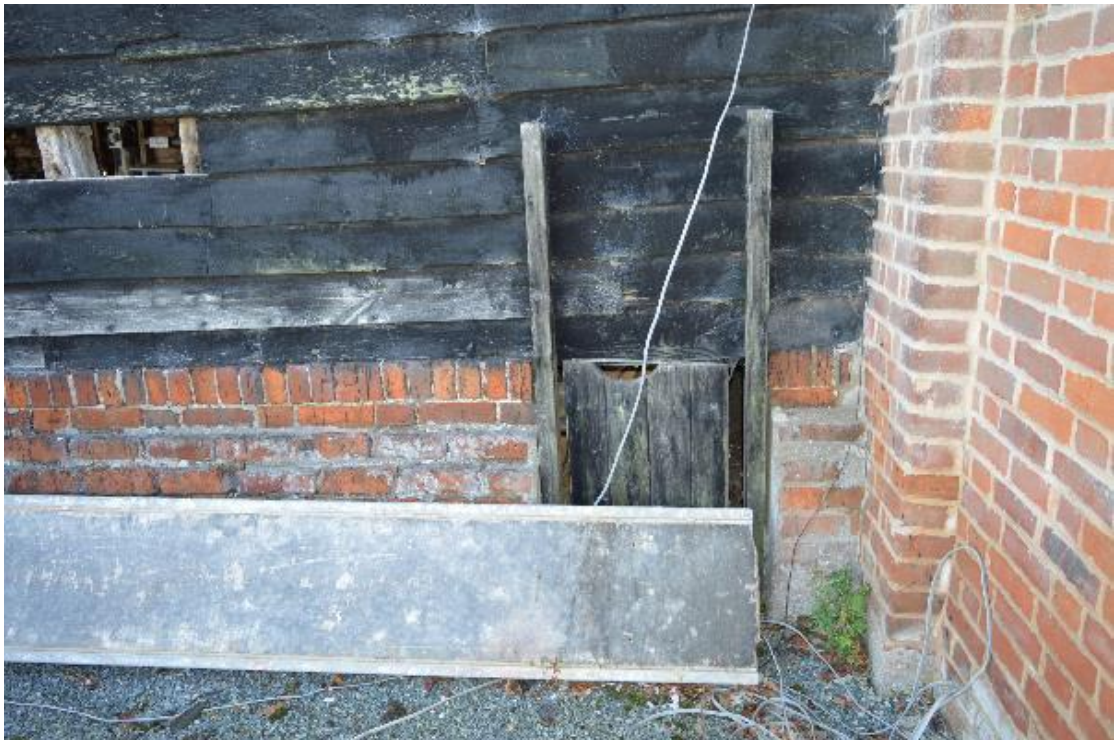
Plate 24 Inserted opening into dog pen within the barn's western end, north elevation, facing south (23)
