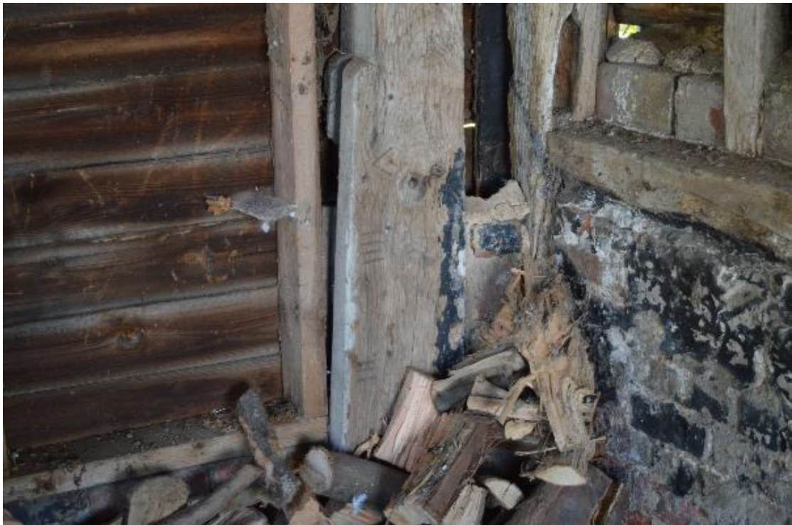
Plate 20 Detail of carpentry marks upon the western jamb to southern doorway, note the integral groove detailing for leap boards, facing south-west (18)
