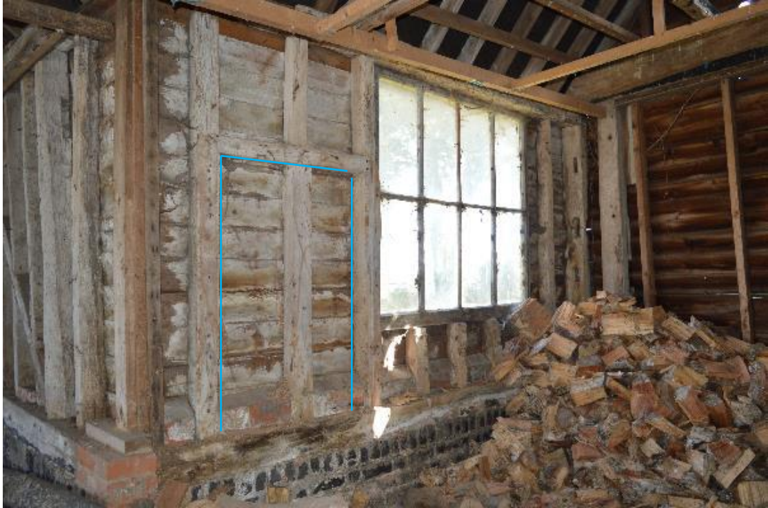
Plate 15 Former opening within the eastern wall of the wagon porch, facing east (15)
