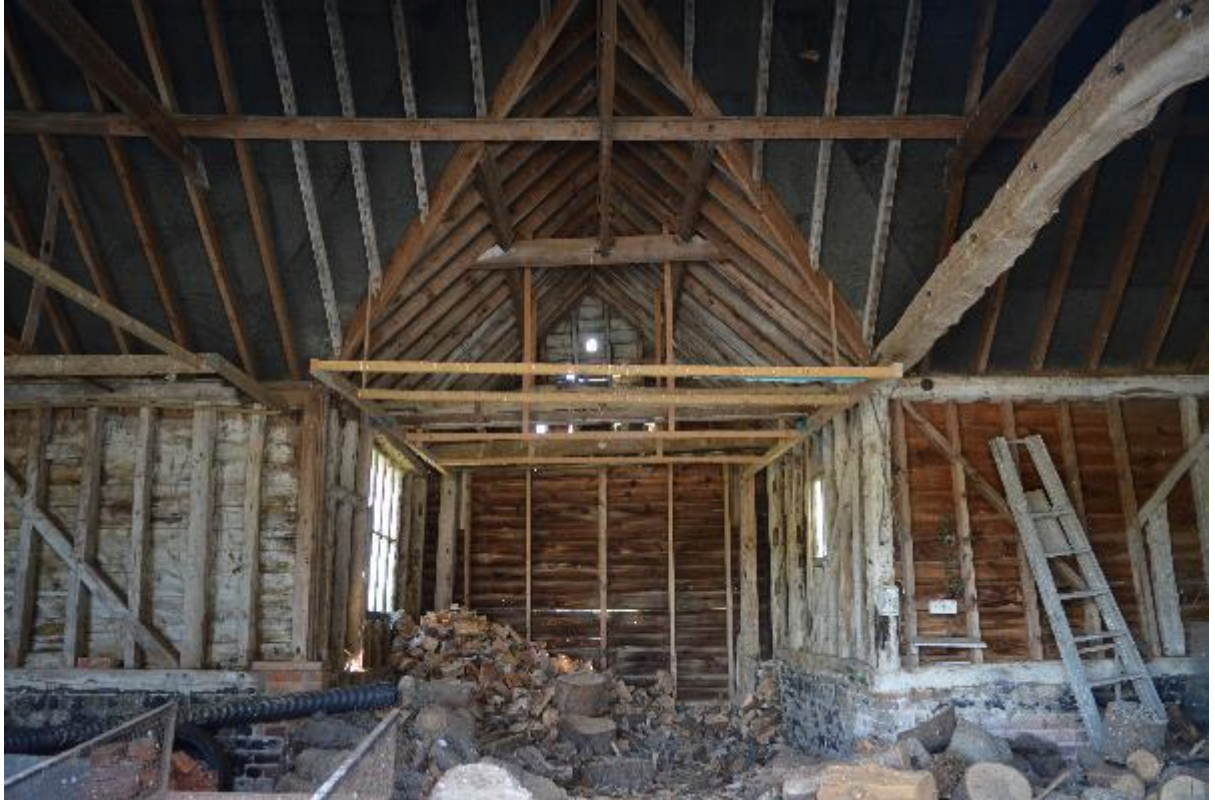
Plate 11 Tie beam construction within southern waggon porch and midstrey bay, facing south (8)
