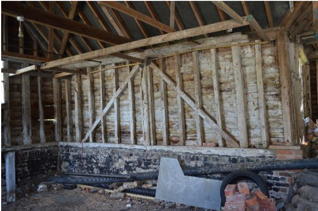
Plate 14 General wall frame construction, southern side of Bays 1 & 2) facing south-east (11)
