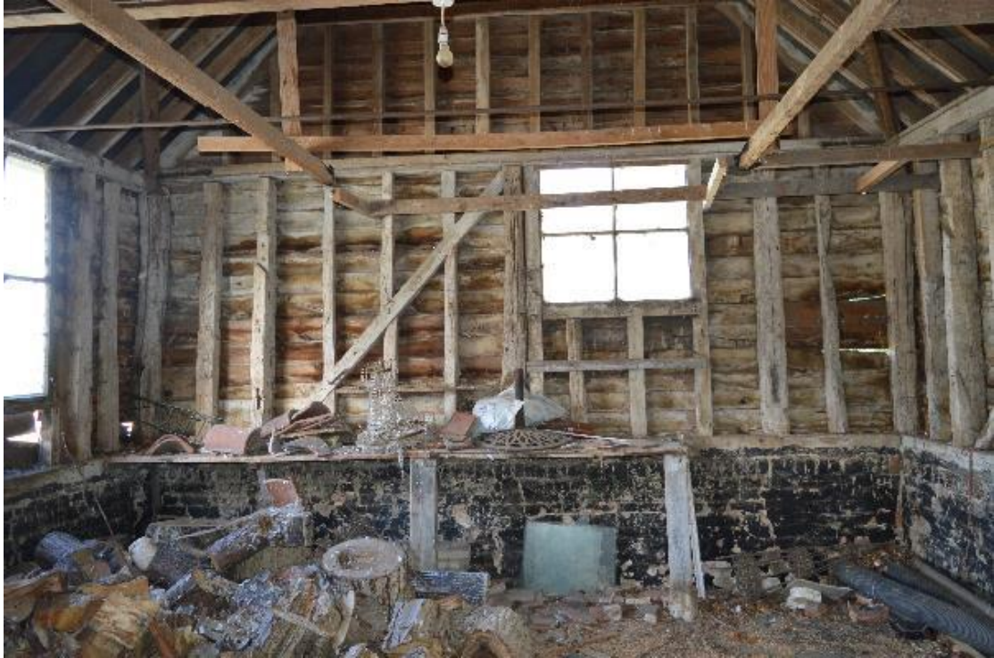
Plate 13 General wall frame construction, east wall of Bay 1, facing east (28)
