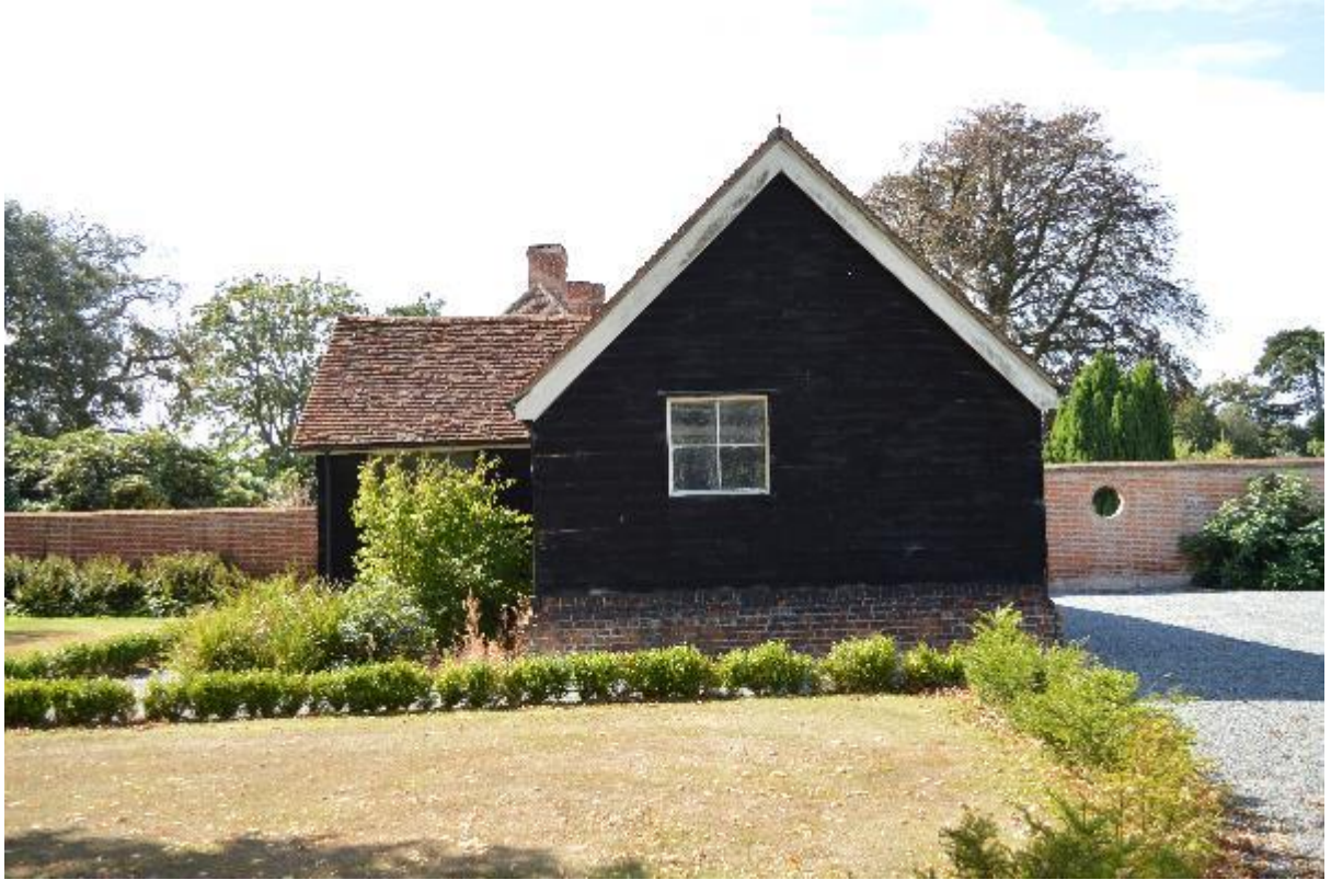
Plate 5 View of the external east elevation, facing west (3)
