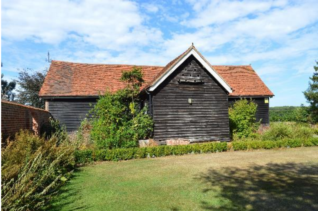
Plate 7 View of the external south elevation, facing north (1)
