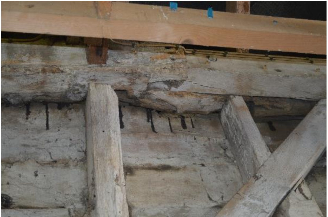
Plate 16 Face-halved and bladed scarf joint, west wall of wagon porch, facing west (14)
