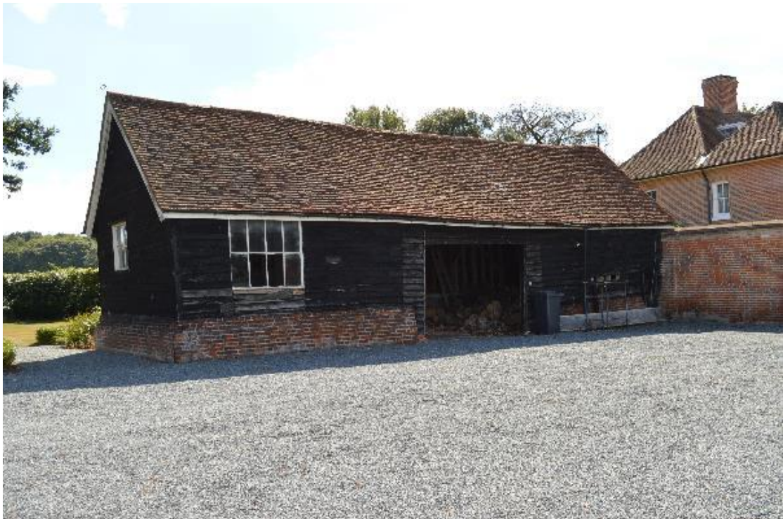
Plate 4 View of the external north elevation, facing south-west (4)
