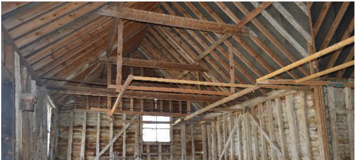
Plate 12 Common rafter roof construction, facing east (6)
