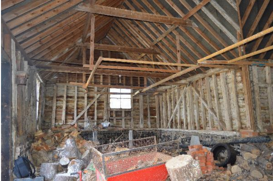
Plate 9 General view of the barn's interior, facing south-east (6)
