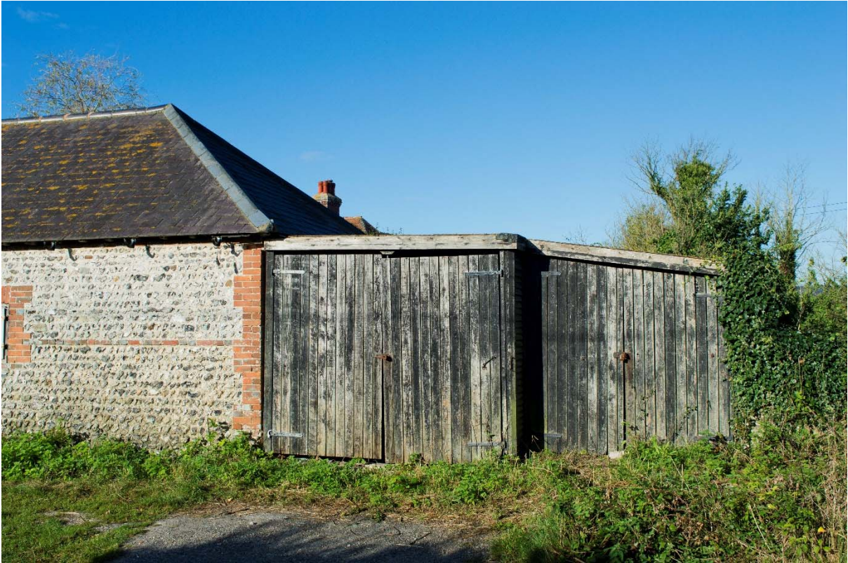
Plate 15: East elevation of northern shelter (5)
