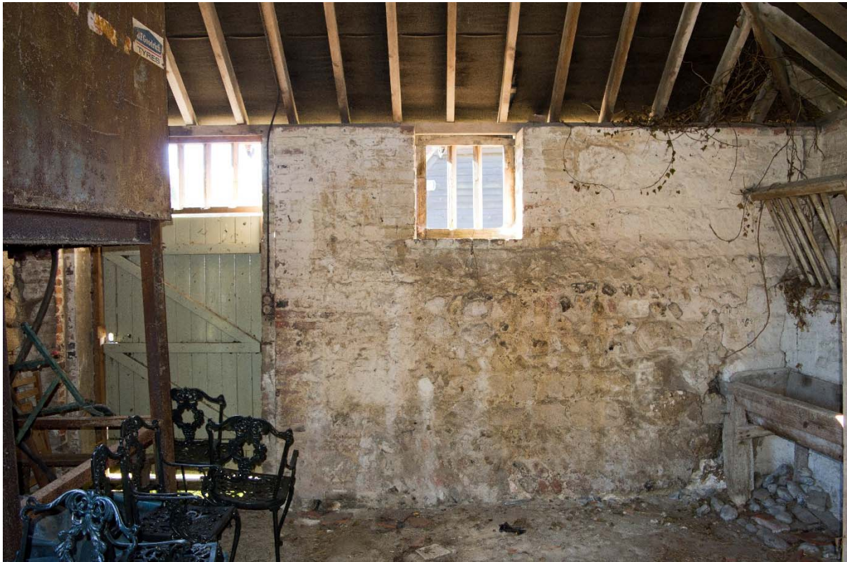
Plate 9: Walling material of the earlier structure surviving beneath the window within the south wall of the present building (28)
