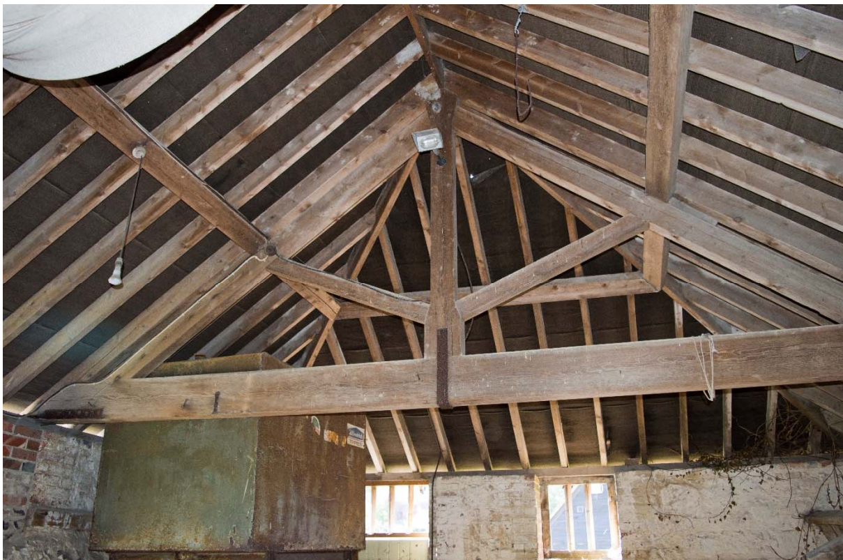
Plate 10: View of the roof, looking south (56)
