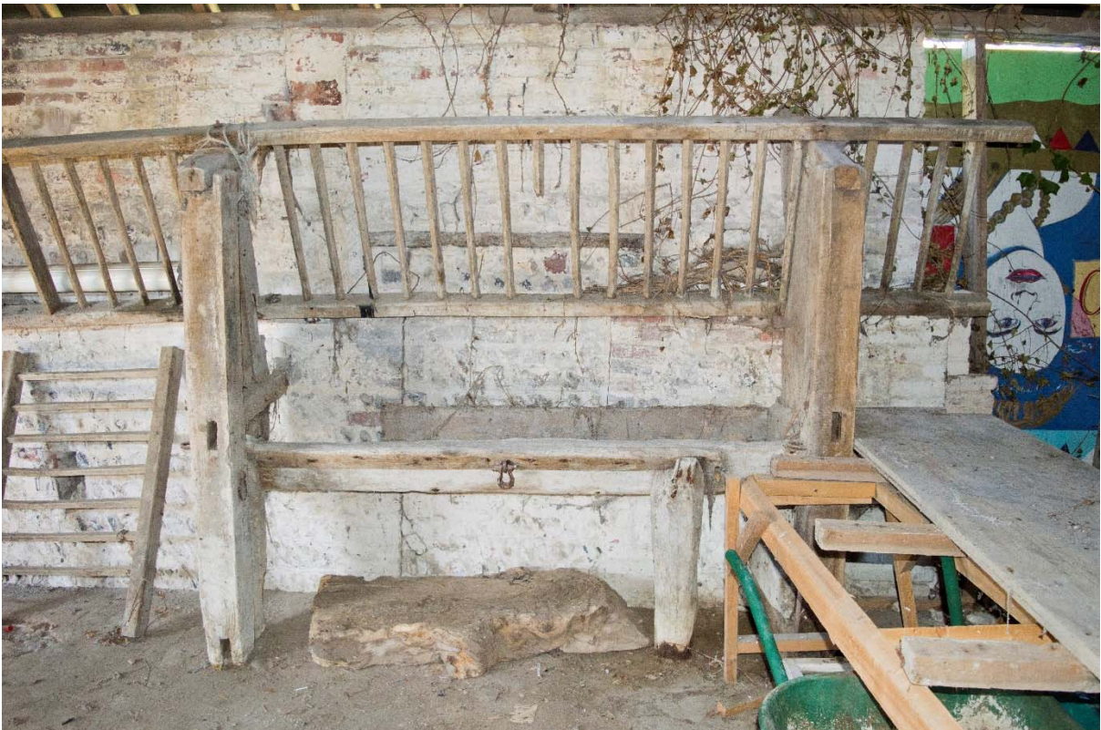
Plate 12: Detail of trough and hay-rack towards north end of the building. Note the blocked opening behind (51)
