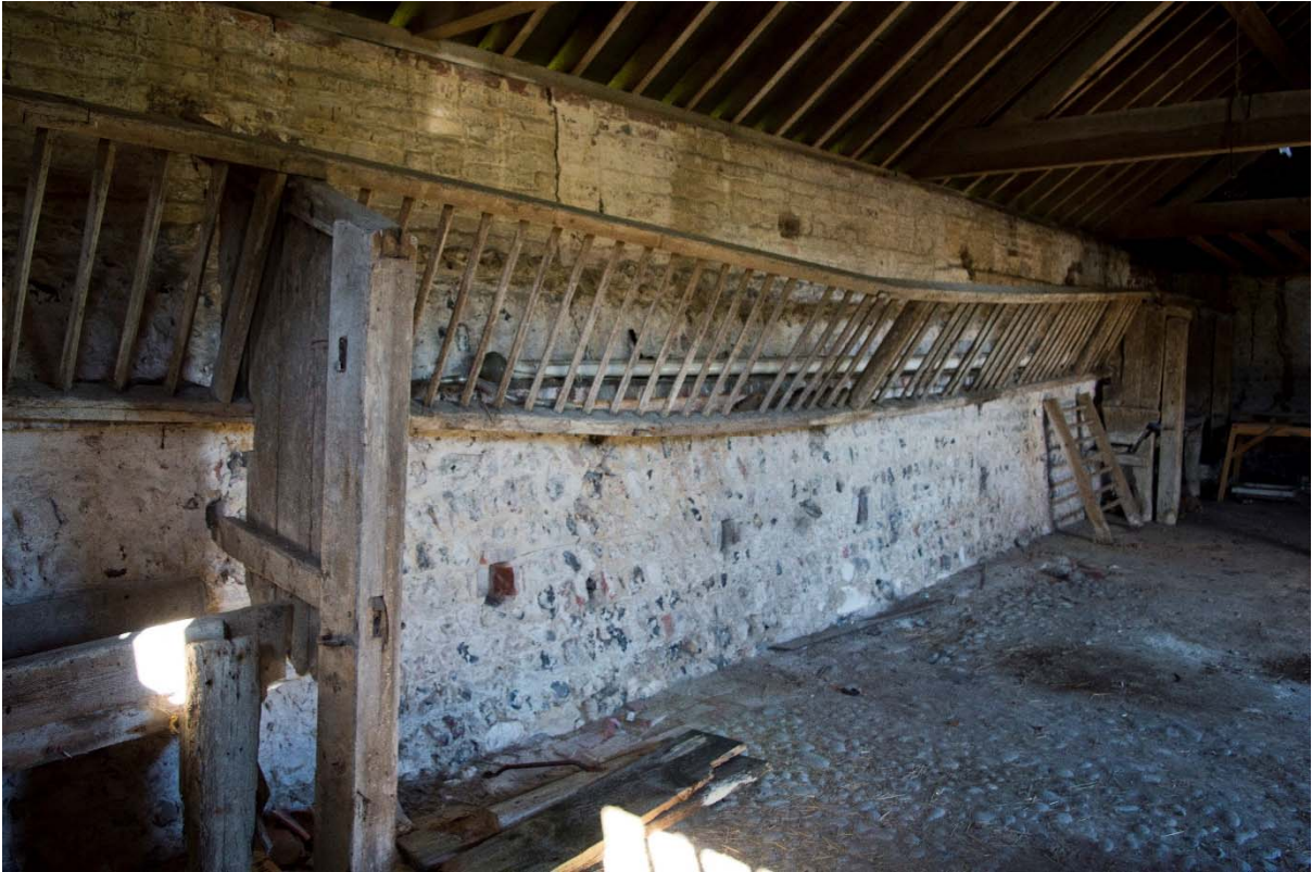
Plate 11: Hay-rack along the west side of the building. Note truncated stall-partition (44)
