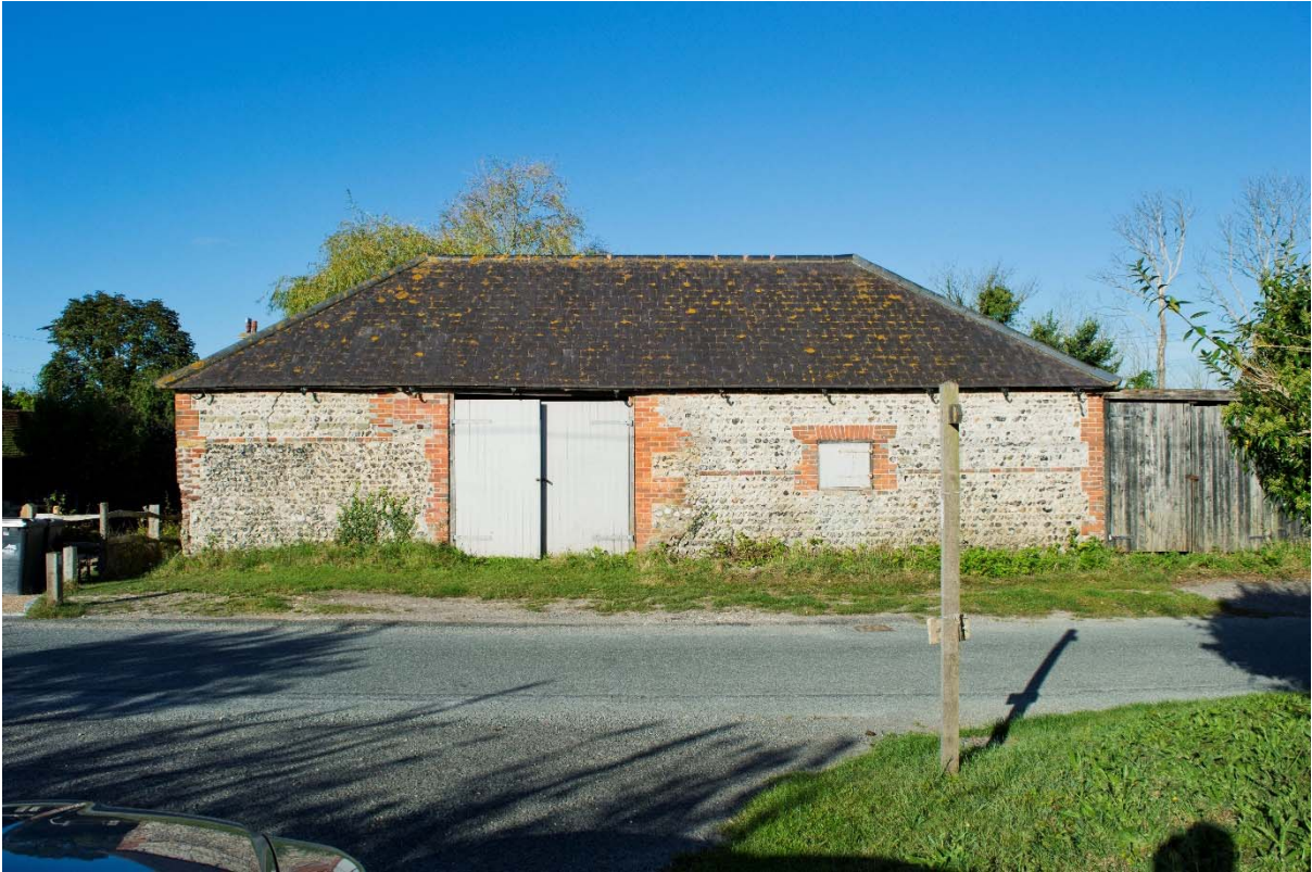
Plate 1: East elevation of the building (1)
