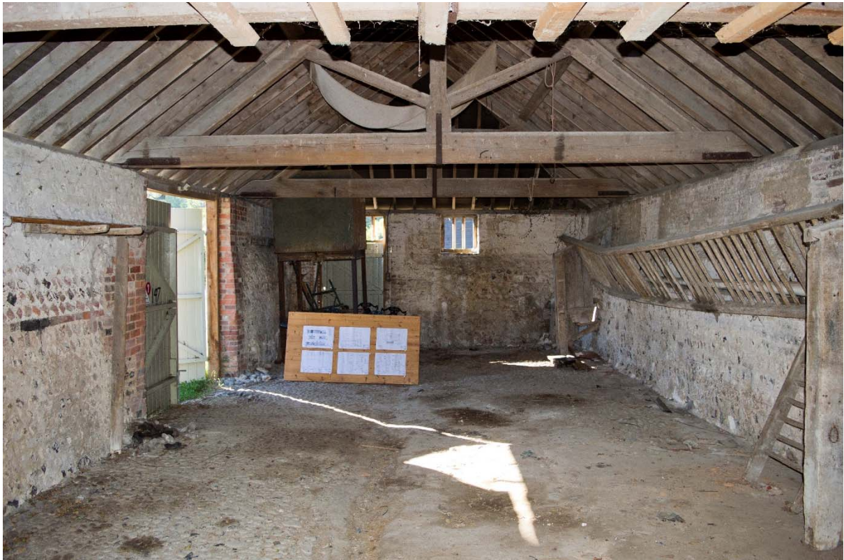
Plate 7: Interior of the building, looking south (26)
