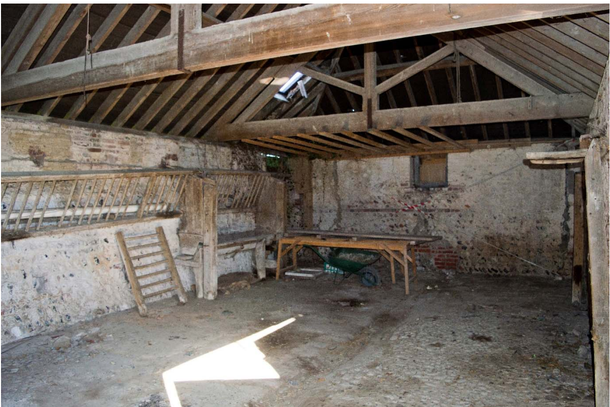
Plate 6: Interior of the building, looking north-west (24)
