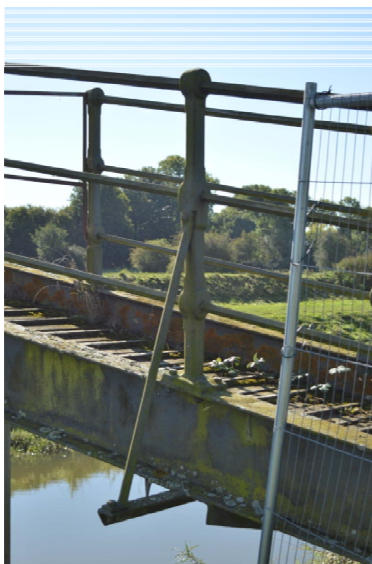
Plate 13: Bollard in original handrail, supported by angle-iron bracing (#EFO16-0056)
