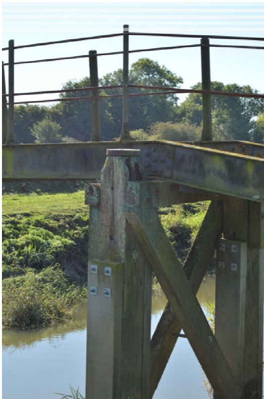
Plate 9: Timber pile finial and tie-beam detail (#EFO16-0055)
