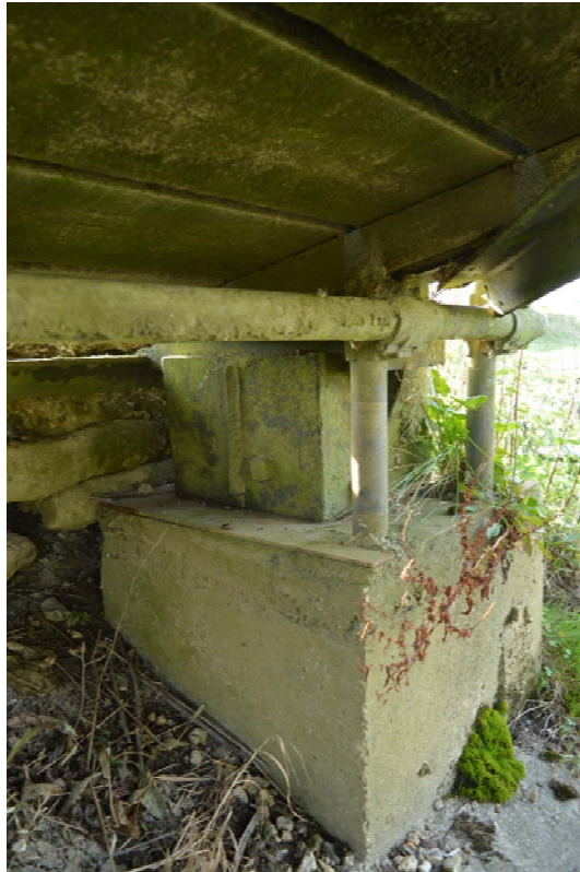
Plate 6: Concrete pier, box stanchion and inserted scaffold (#EFO16-0041)
