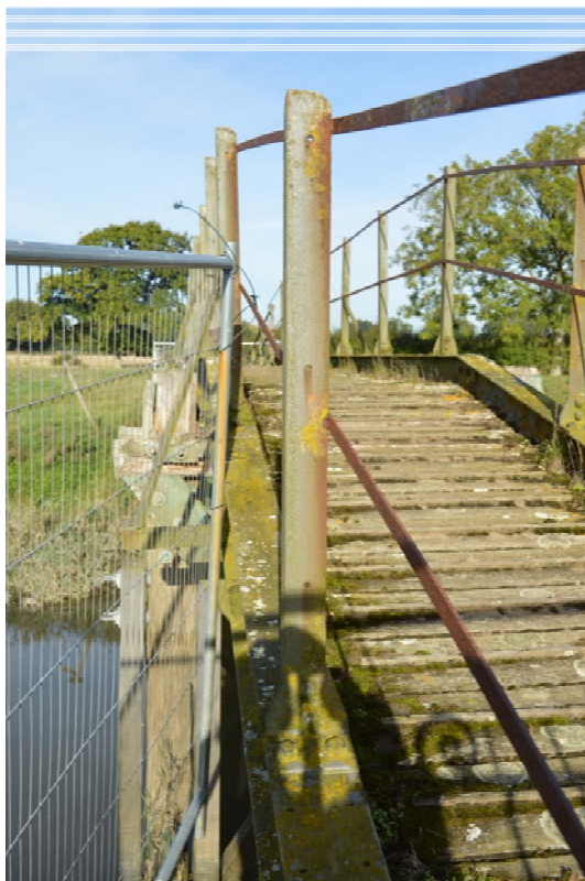
Plate 14: Replacement angle-iron and flat iron handrail (#EFO16-0042)
