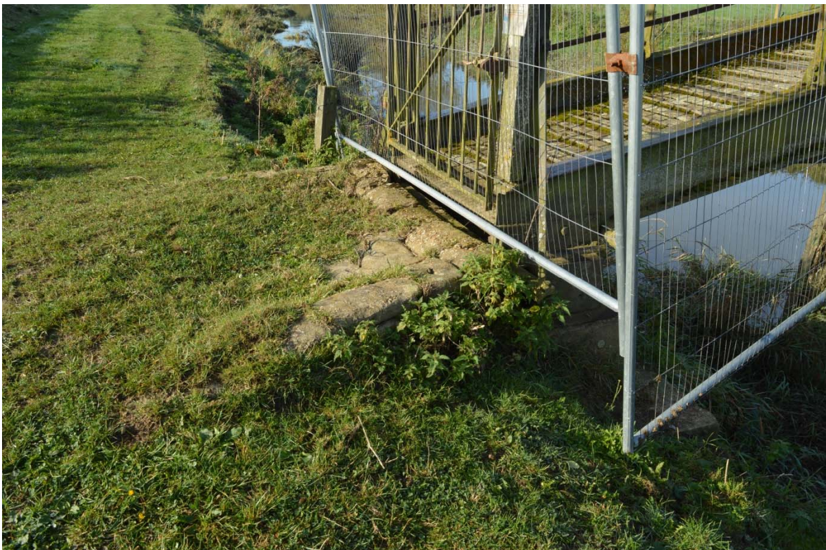
Plate 7: Concreted sandbag ramp to east side of the bridge (#EFO16-0032)
