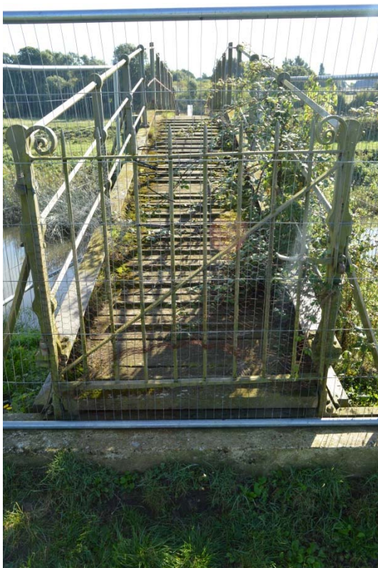
Plate 15: West gate to the bridge (#EFO16-0068)
