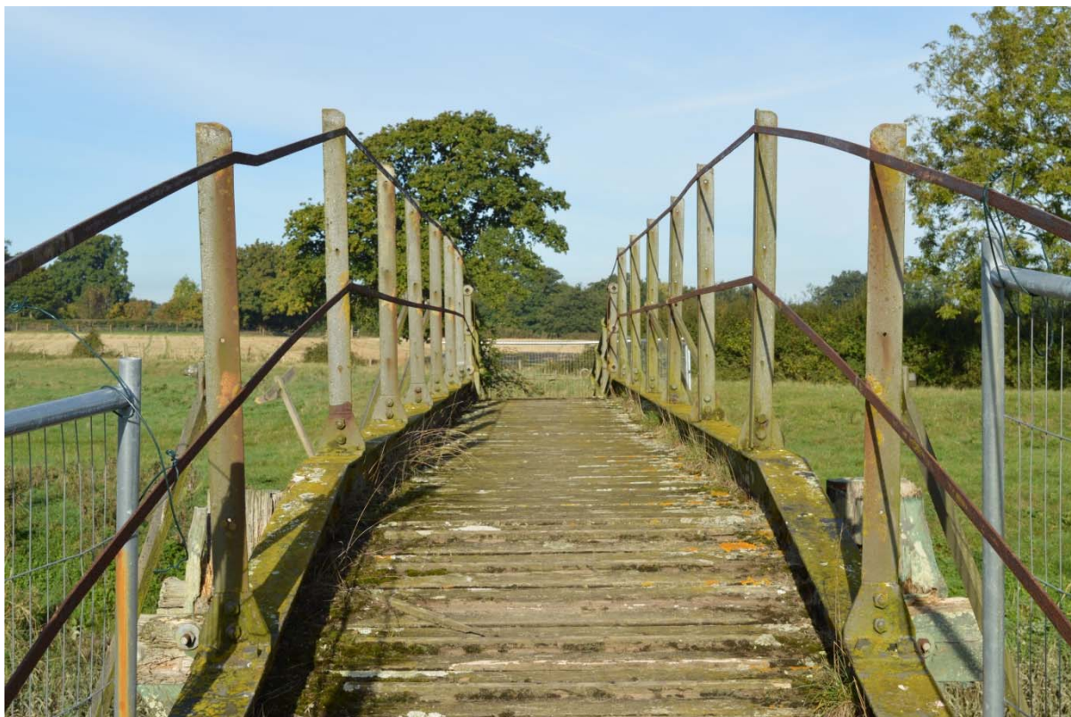
Plate 11: View west along the bridge deck (#EFO16-0044)
