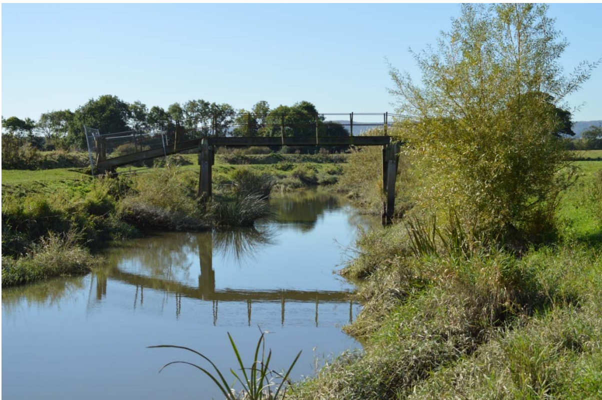
Plate 3: North elevation of the bridge (#EFO16-0054)
