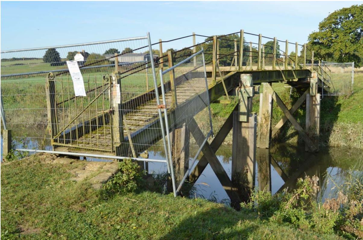
Plate 5: Oblique view of the north elevation of the bridge (#EFO16-0030)
