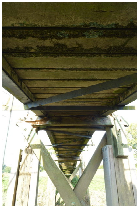
Plate 10: Soffit of the bridge (#EFO16-0038)
