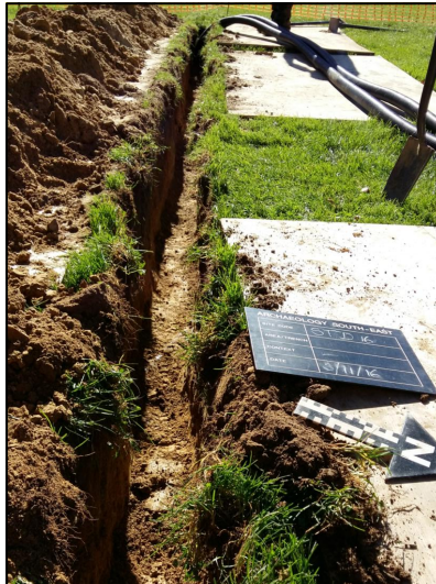
View of trench excavation through Goose Green
