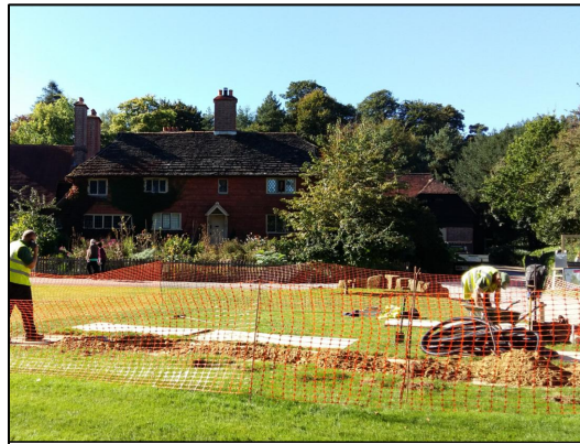
View of works with Standen House in background
