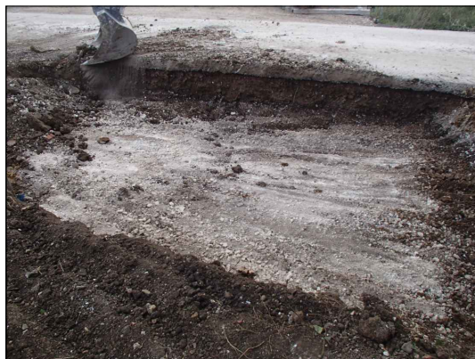
Western area looking south
