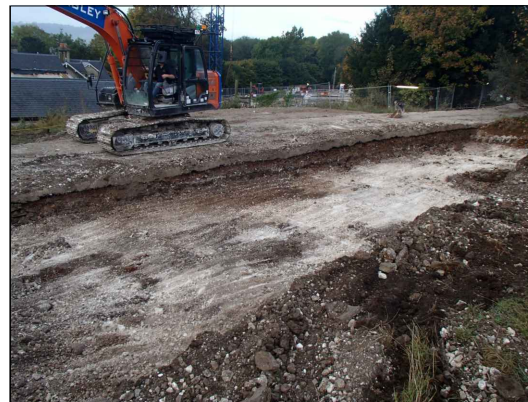
Western area looking south
