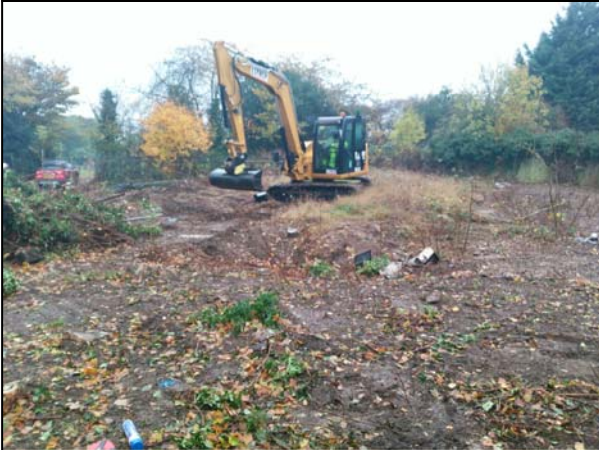
General view of the site
