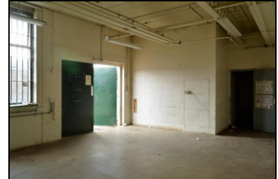
HOB16-0786 Building 23, original range, arms trainer store
