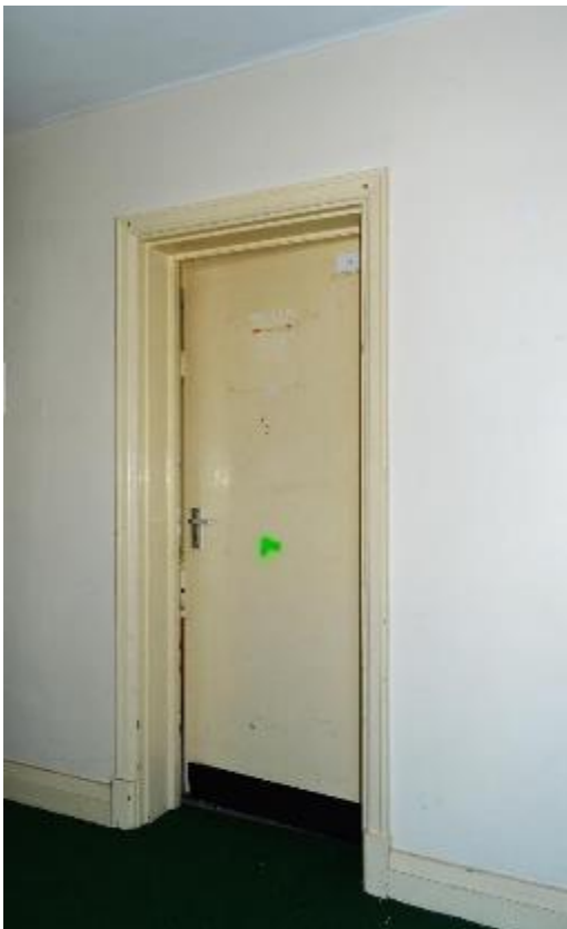
Plate 10: Building 1, original range, first floor (75)
