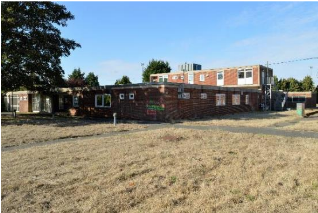
Plate 32: Building 3, south-east elevation (228)
