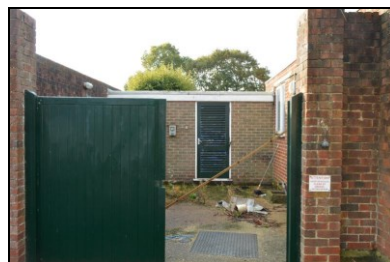
HOB16-0012 Building 1, western courtyard
