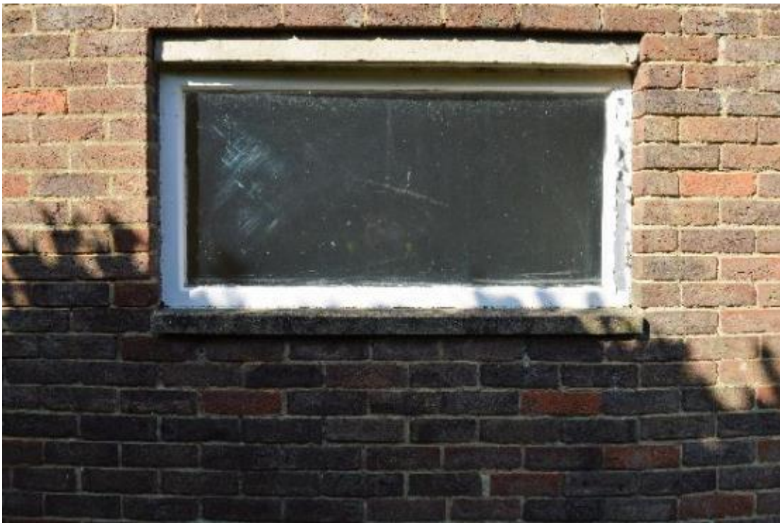
Plate 46: Building 5, typical window arrangement (293)
