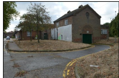
HOB16-0429 Building 18, north-east corner
