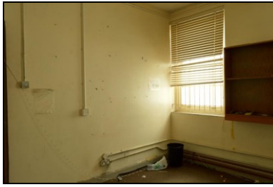
HOB16-0526 Building 12, east wing, ground floor
