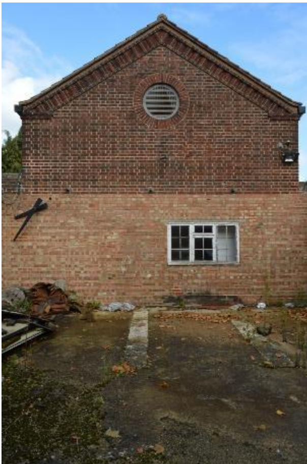
Plate 154: Building 18, south elevation (435)
