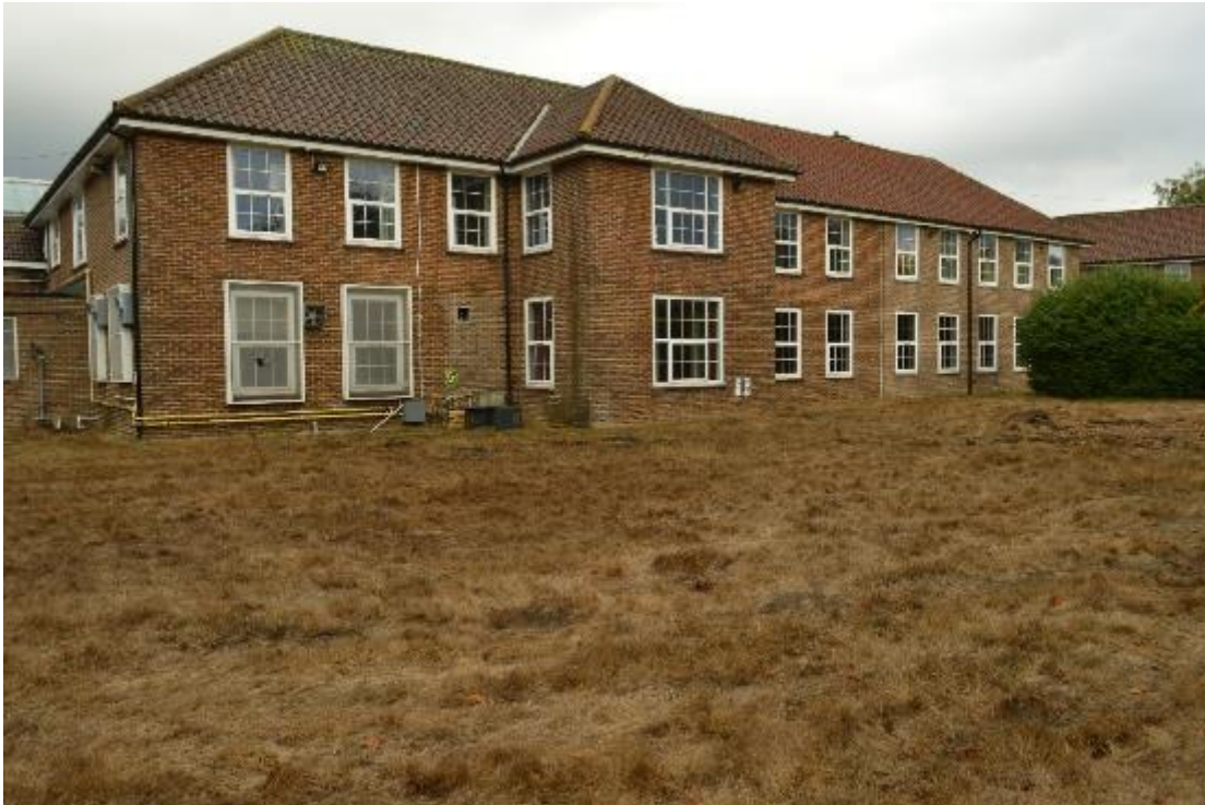
Plate 109: Building 14, south elevation (578)
