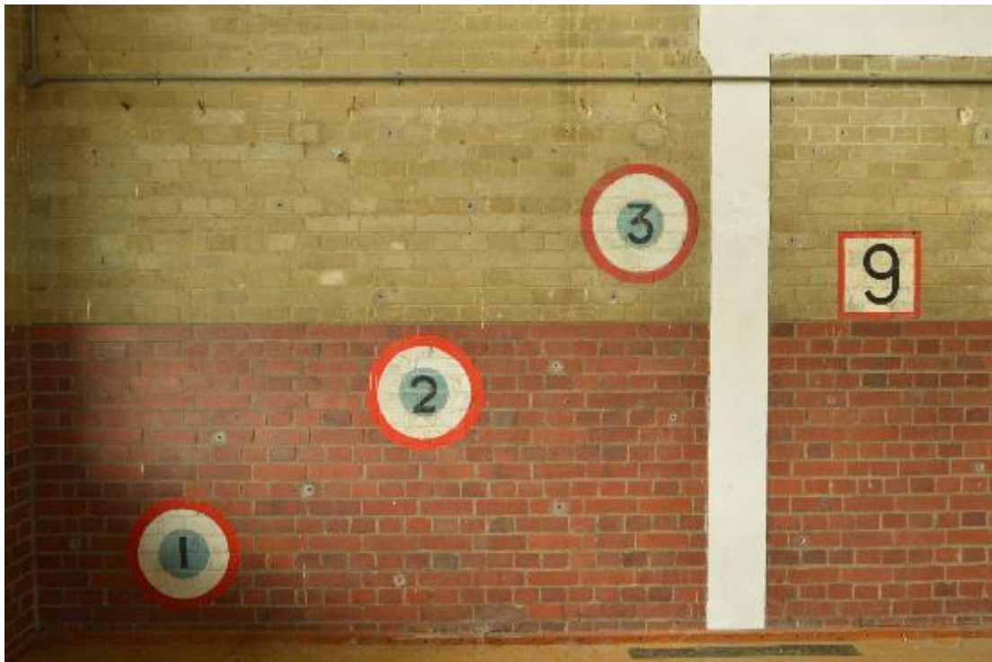
Plate 144: Building 17, south range, ground floor, gym wall finishing (680)
