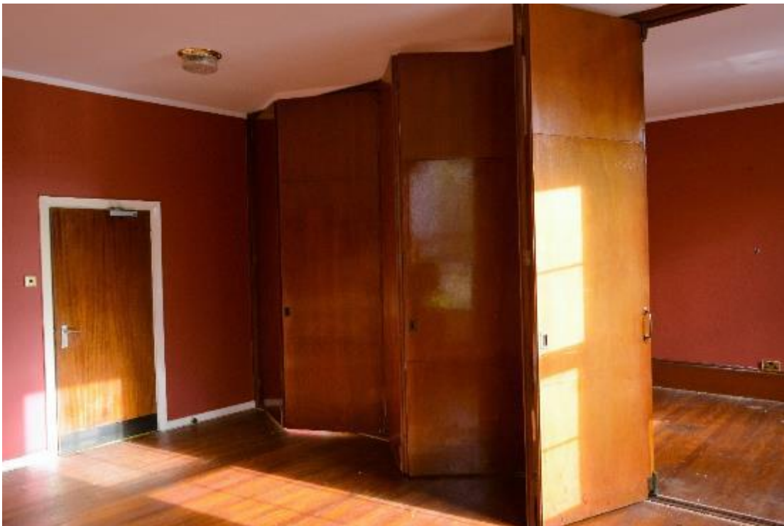
Plate 114: Building 14, original range, ground floor, dining room, pine shutters (590)
