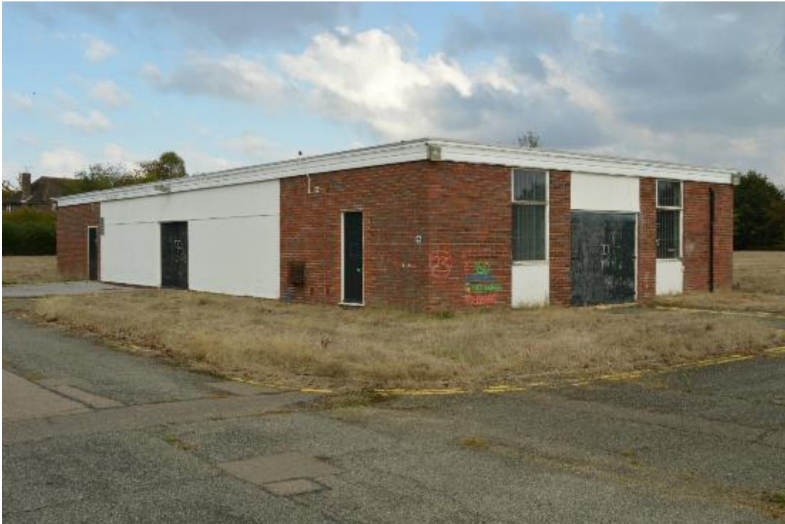
Plate 185: Building 23, south-west corner (772)
