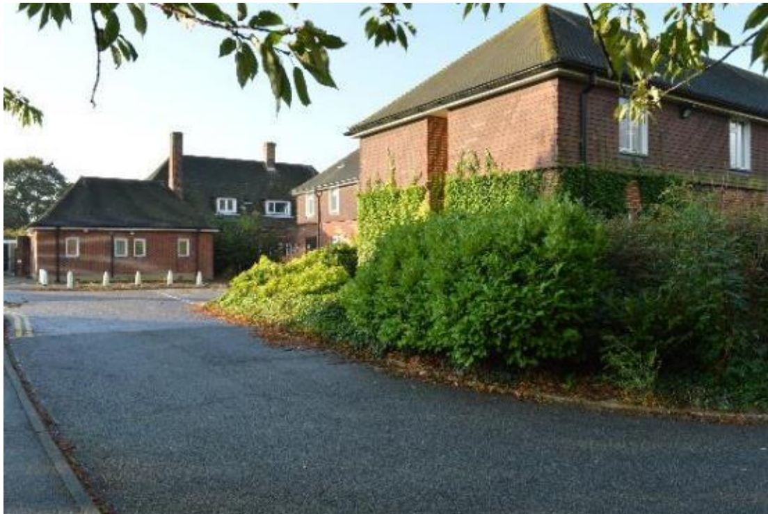
Plate 1: Building 1, east elevation (3)
