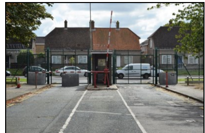
HOB16-0219 Building 2A, north elevation
