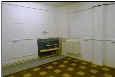
HOB16-0218 Building 2, west extension
