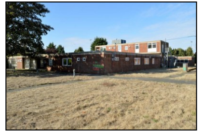
HOB16-0228 Building 3, south-east elevation
