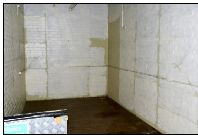
HOB16-0776 Building 23, original range
