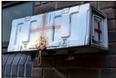
HOB16-0863 Building 25, south elevation passage, first aid box
