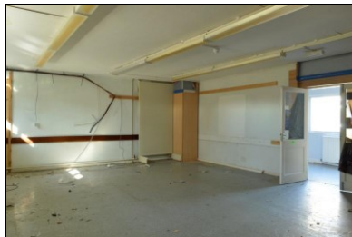
HOB16-0236 Building 3, ground floor
