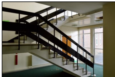
HOB16-0581 Building 14, east extension, ground floor
