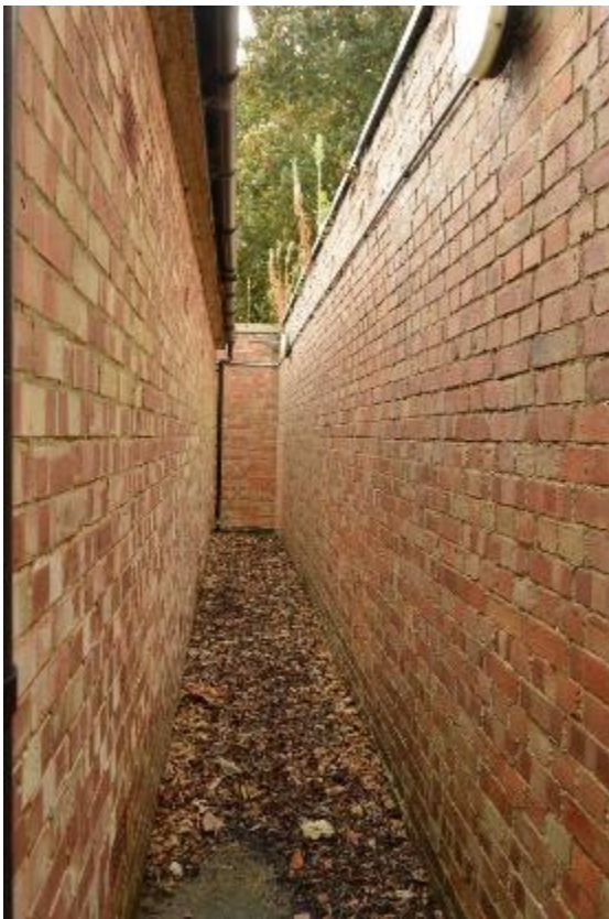
Plate 56: Building 6, north internal passage (319)
