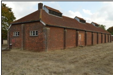
HOB16-0760 Building 22, south-west corner
