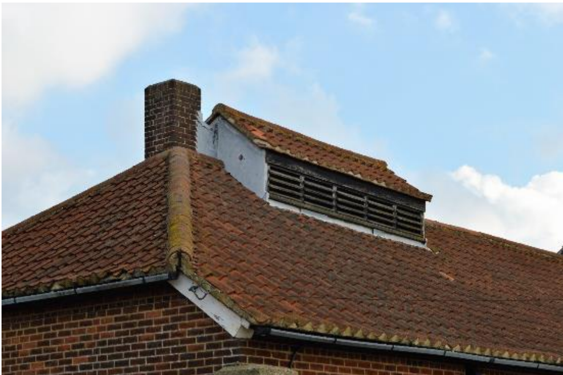
Plate 176: Building 22, south-west corner, roof vent and chimney detail (761)
