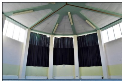
HOB16-0298 Building 5, band practice room
