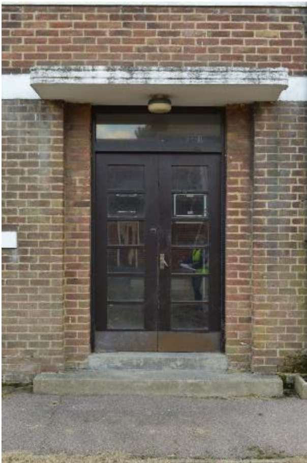
Plate 132: Building 17, north elevation, principal entrance (661)
