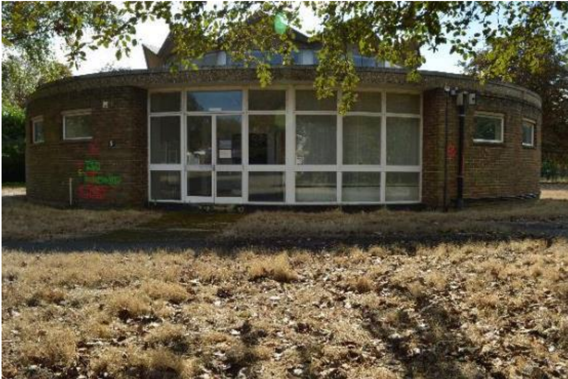
Plate 45: Building 5, north side (292)
