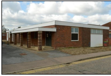
HOB16-0331 Building 8, south-east elevation
