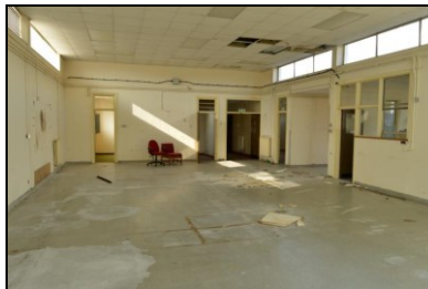
HOB16-0641 Building 15, sports hall
