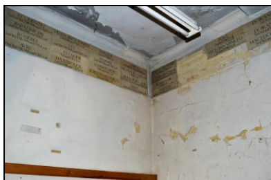
HOB16-0203 Building 2, west extension
