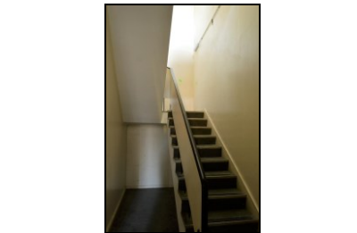
HOB16-0252 Building 3, north range
