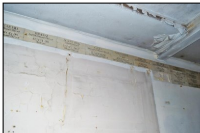
HOB16-0206 Building 2, west extension
