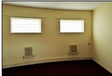
HOB16-0305 Building 5, instrument store
