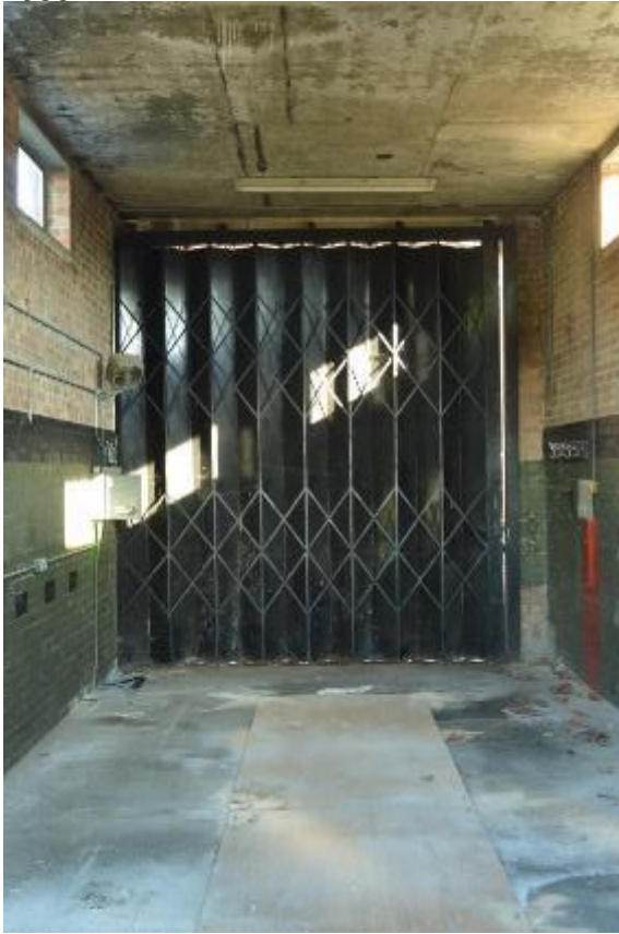
Plate 61: Building 7, north room, vehicle maintenance (329)
