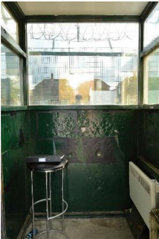
Plate 30: Building 2A, interior (2243)
