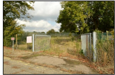
HOB16-0909 Access road at the northern end of the site providing access to Building 24
