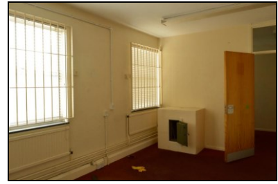
HOB16-0753 Building 21, north-east range, ground floor
