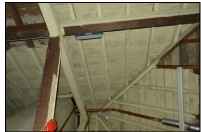
HOB16-0624 Building 14, original range, roof
