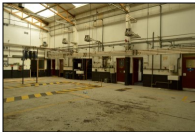
HOB16-0796 Building 24, west range, garage
