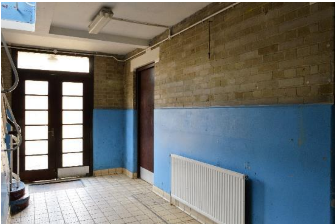
Plate 138: Building 17, north range, ground floor, lobby (664)
