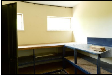
HOB16-0304 Building 5, instrument store
