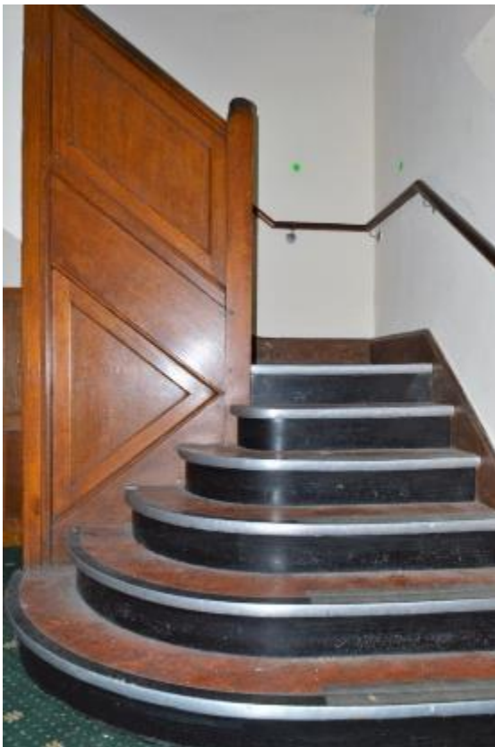
Plate 8: Building 1, original range, ground floor, staircase (41)
