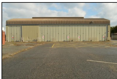
HOB16-0794 Building 24, west range, west elevation
