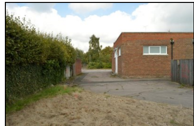
HOB16-0891 View of the west elevation of Building 2
