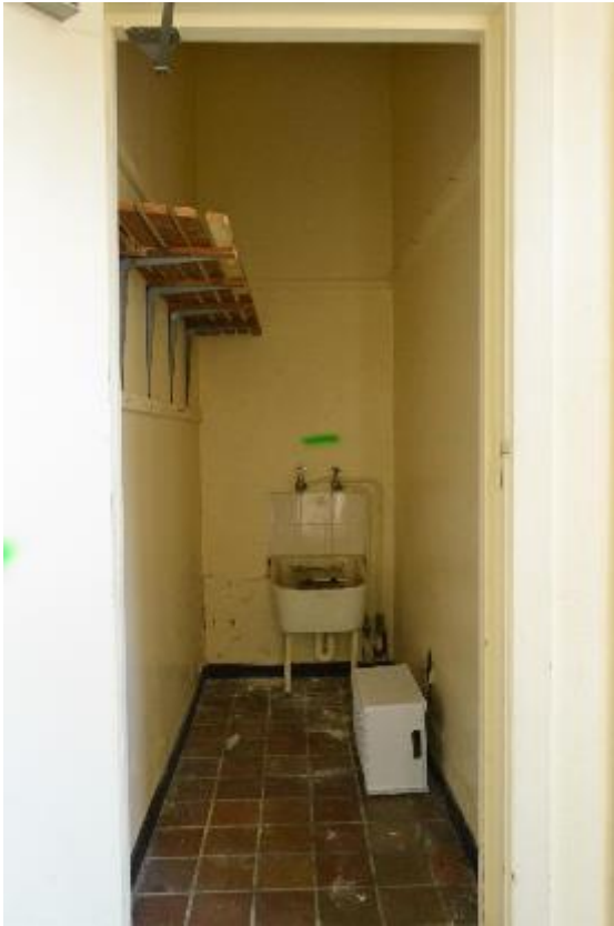
Plate 7: Building 1, original range, ground floor, kitchen store (46)
