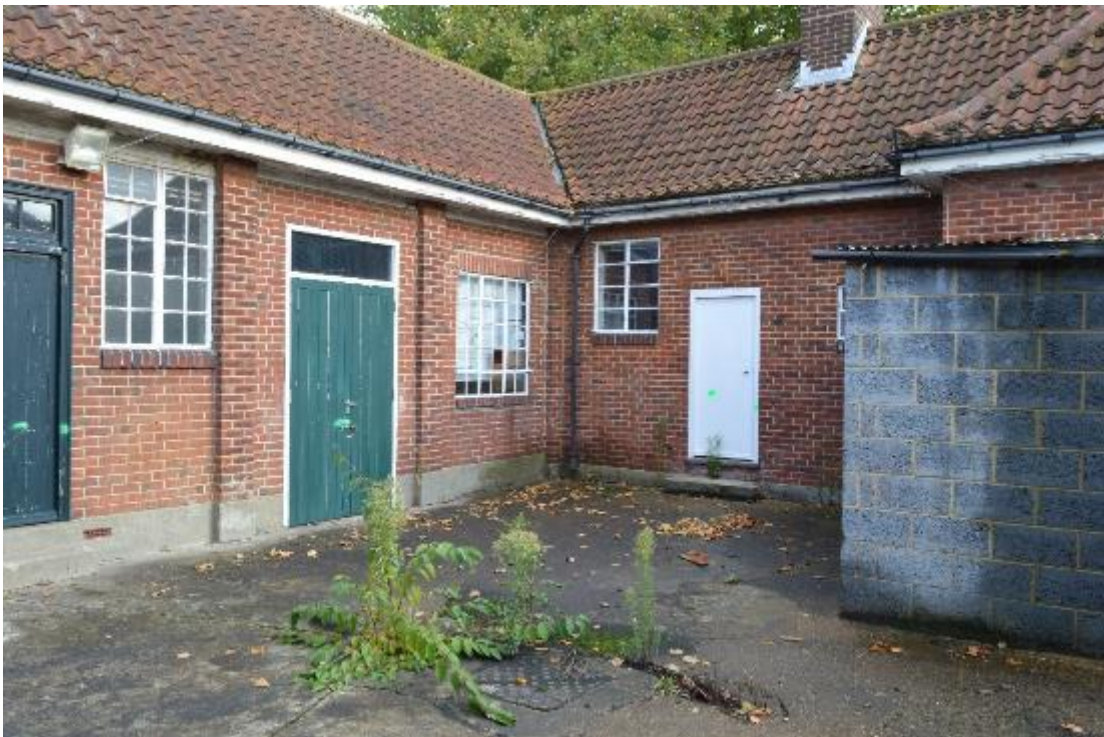
Plate 88: Building 11, internal courtyard (439)
