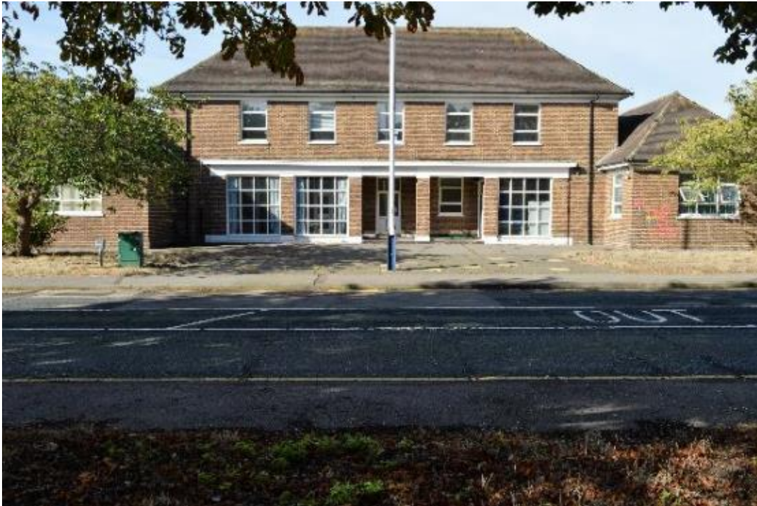
Plate 15: Building 2, east extension (108)
