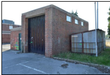
HOB16-0323 Building 7, north-east corner
