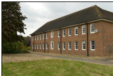
HOB16-0464 Building 12, south-east corner
