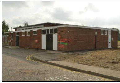
HOB16-0632 Building 15, north-west corner
