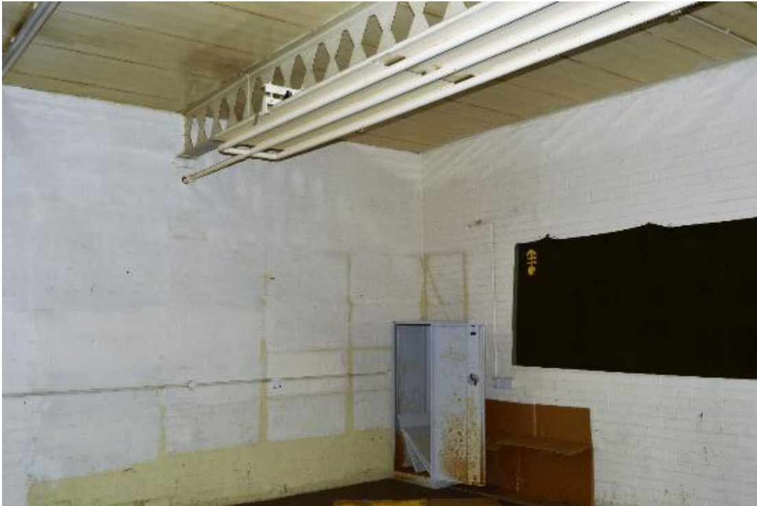
Plate 187: Building 23, original range, north coy (775)
