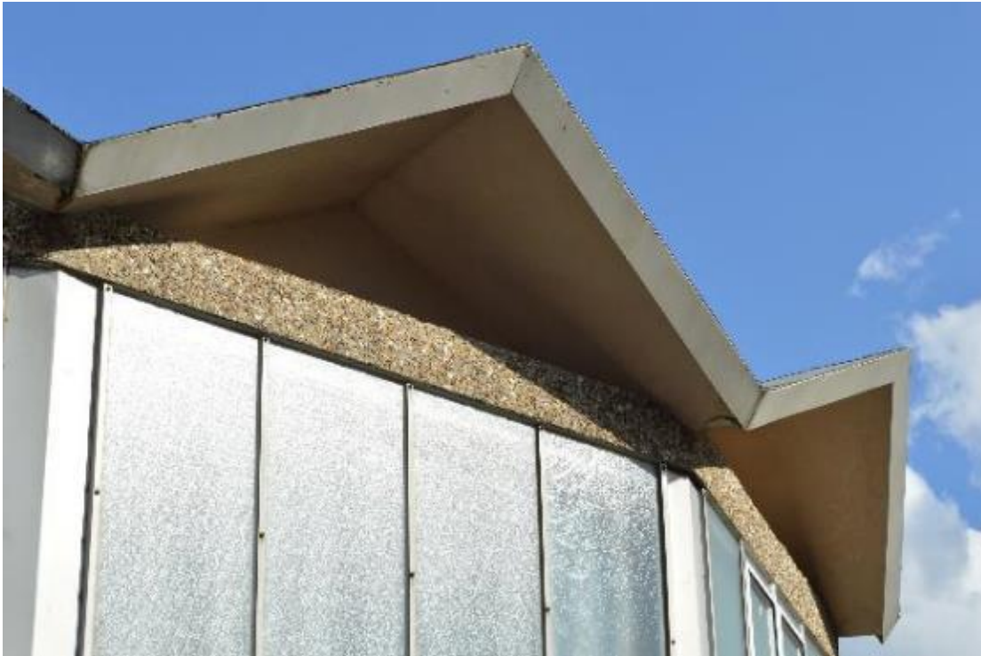
Plate 47: Building 5, roof and upper window arrangement (294)
