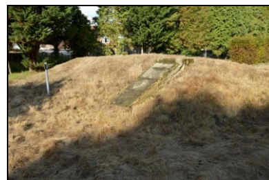
HOB16-0879 Bunker 1, south-east corner
