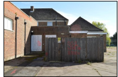
HOB16-0114 Building 2, west elevation
