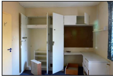
HOB16-0095 Building 1, interior, north range
