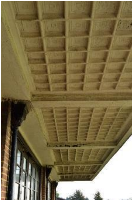
Plate 134: Building 17, south elevation, veranda detailing (659)
