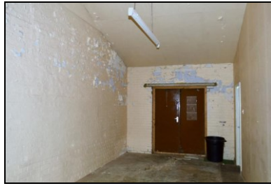
HOB16-0767 Building 22, east room
