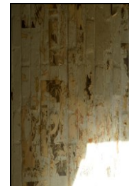
HOB16-0420 Building 10, armoury, north wall newspaper clippings
