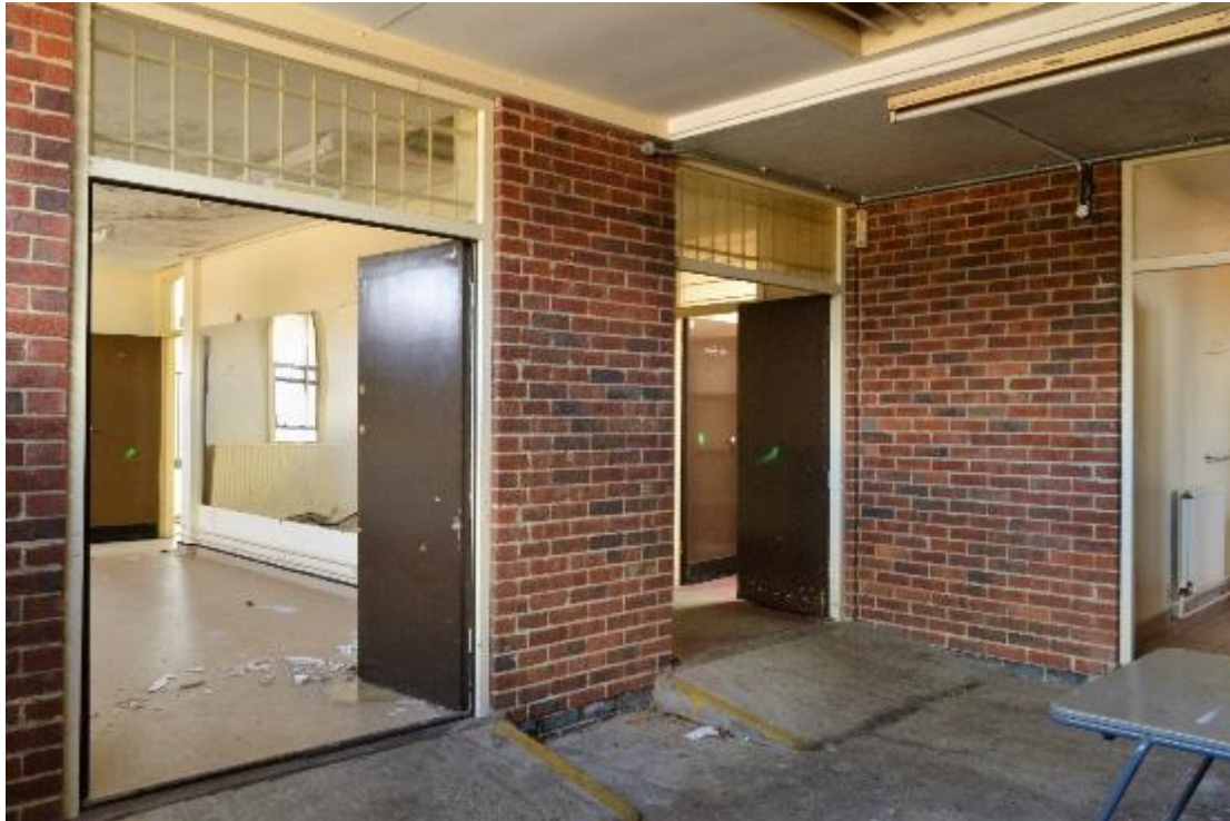
Plate 127: Building 15, covered yard (645)
