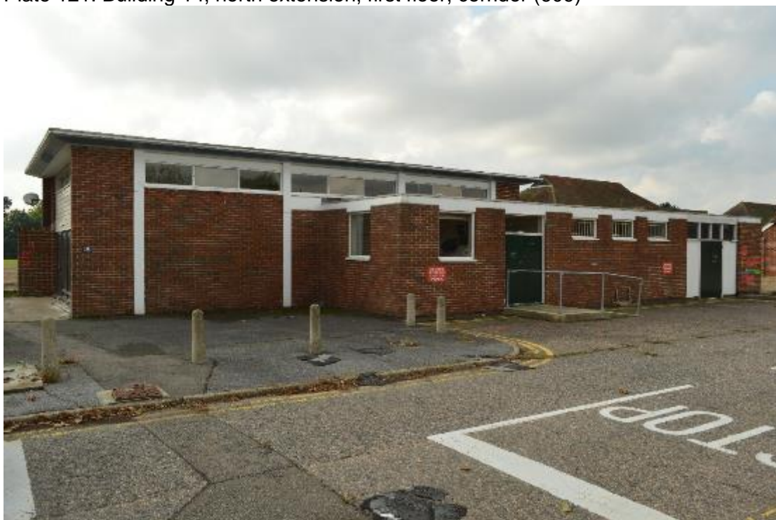
Plate 122: Building 15, north elevation (633)
