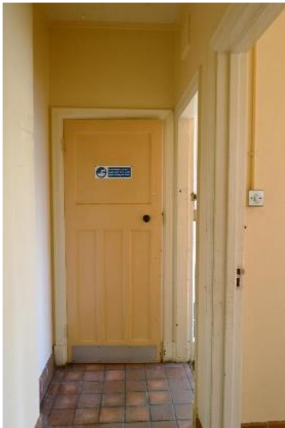
Plate 6: Building 1, original range, ground floor, original door (54)
