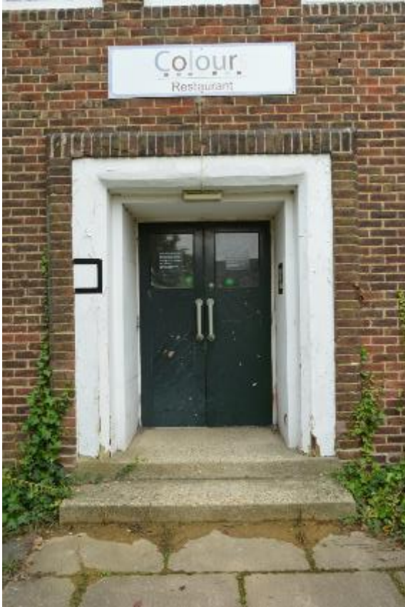
Plate 99: Building 12, east elevation, doorway (478)
