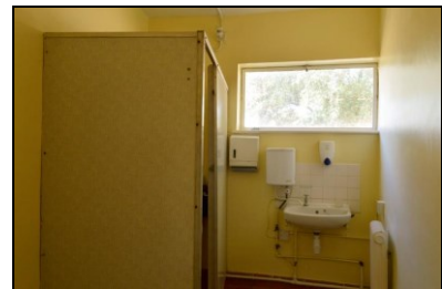
HOB16-0309 Building 5, WC
