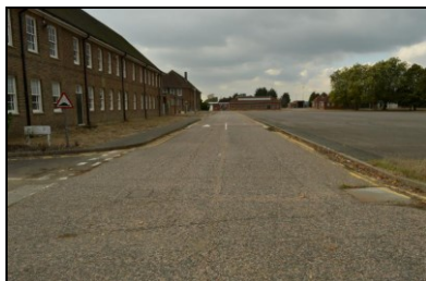
HOB16-0922 View of the Drill Yard to the north of Building 12
