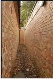
HOB16-0319 Building 6, north internal passage
