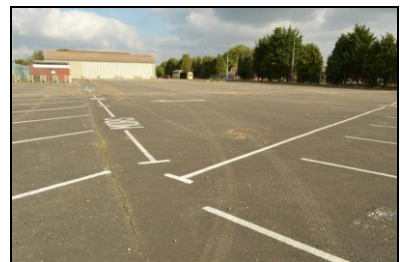
HOB16-0912 Car park to the south of Building 24
