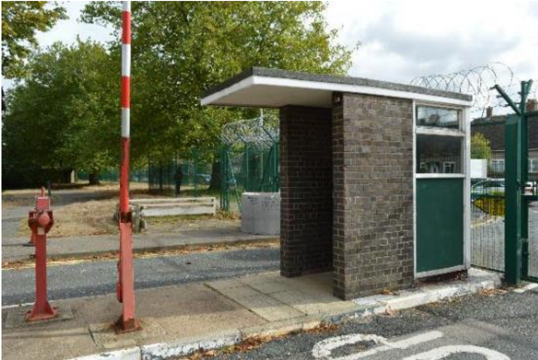
Plate 29: Building 2A, west elevation (224)
