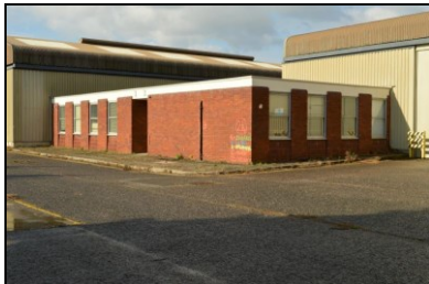
HOB16-0790 Building 24, central link structure
