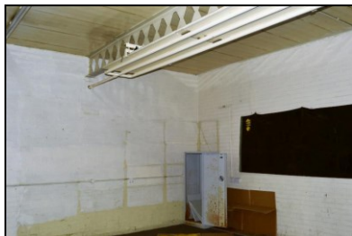
HOB16-0775 Building 23, original range, north coy
