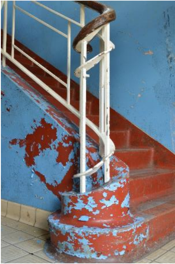
Plate 135: Building 17, north range, ground floor, lobby stair (662)
