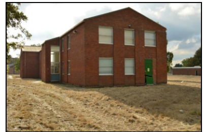
HOB16-0732 Building 21, north-east corner
