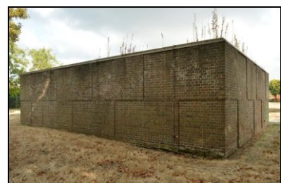
HOB16-0315 Building 6, west elevation
