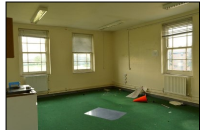
HOB16-0534 Building 12, east wing, first floor
