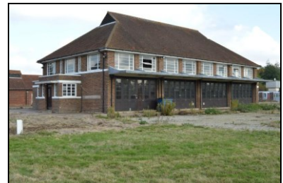
HOB16-0657 Building 17, south-west corner
