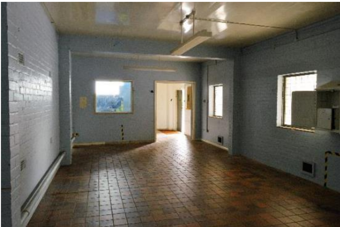
Plate 66: Building 8, southern store with office partition (344)
