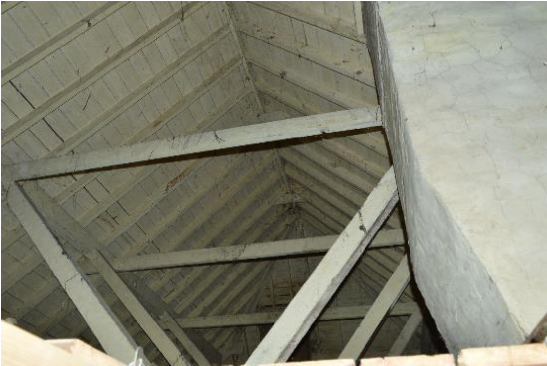
Plate 213: Building 90, roof and central chimney construction (875)
