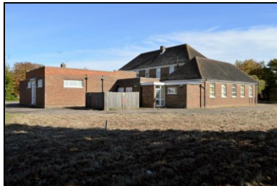
HOB16-0112 Building 2, south-west corner
