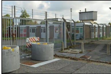
HOB16-0650 Building 16, south-west corner
