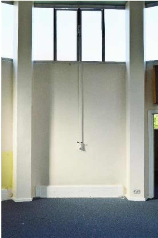
Plate 51: Building 5, band practice room, window panels (308)
