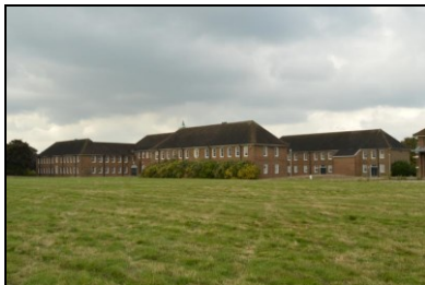
HOB16-0457 Building 12, south-east corner
