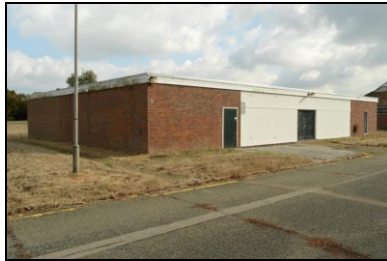
HOB16-0770 Building 23, north-west corner
