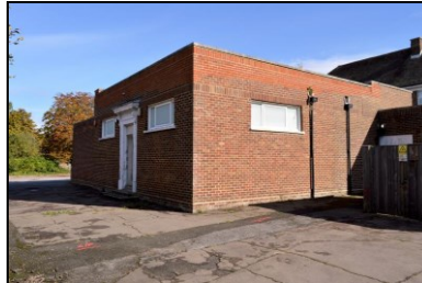
HOB16-0116 Building 2, west elevation
