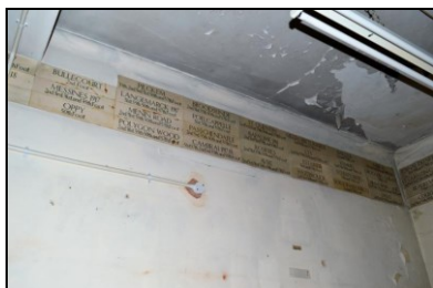
HOB16-0202 Building 2, west extension
