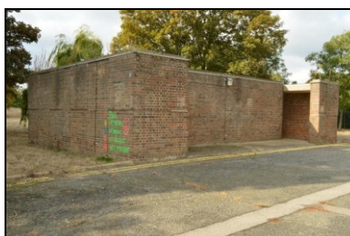
HOB16-0314 Building 6, south-east corner
