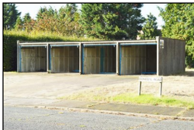
HOB16-0104 Building 1A, east extension
