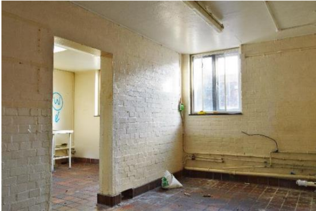
Plate 5: Building 1, original range, ground floor, kitchen prep area (51)
