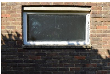
HOB16-0293 Building 5, typical window arrangement
