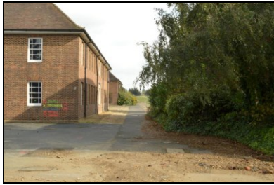
HOB16-0901 Building 9, west elevation
