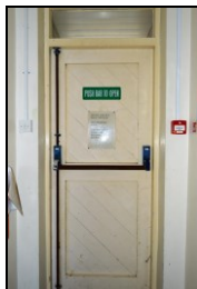
HOB16-0103 Building 1, interior, north range
