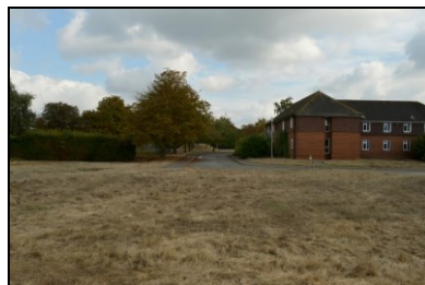
HOB16-0896 View of central access separating Buildings 1 and 9
