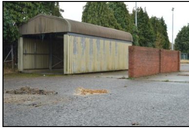
HOB16-0812 Building 24, south shed
