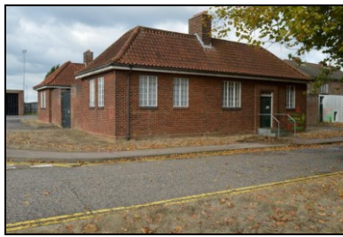
HOB16-0422 Building 11, south-east corner
