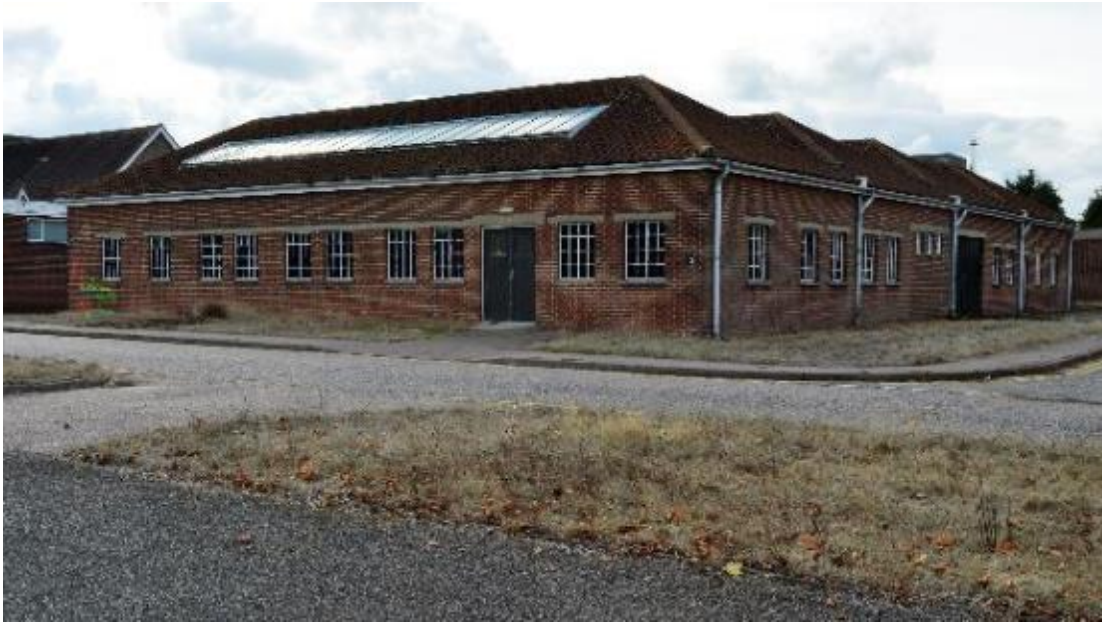
Plate 75: Building 10, north-east corner (404)
