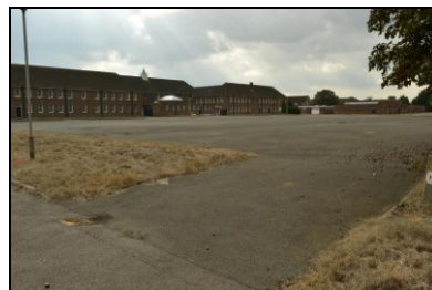
HOB16-0921 View of the Drill Yard to the north of Building 12
