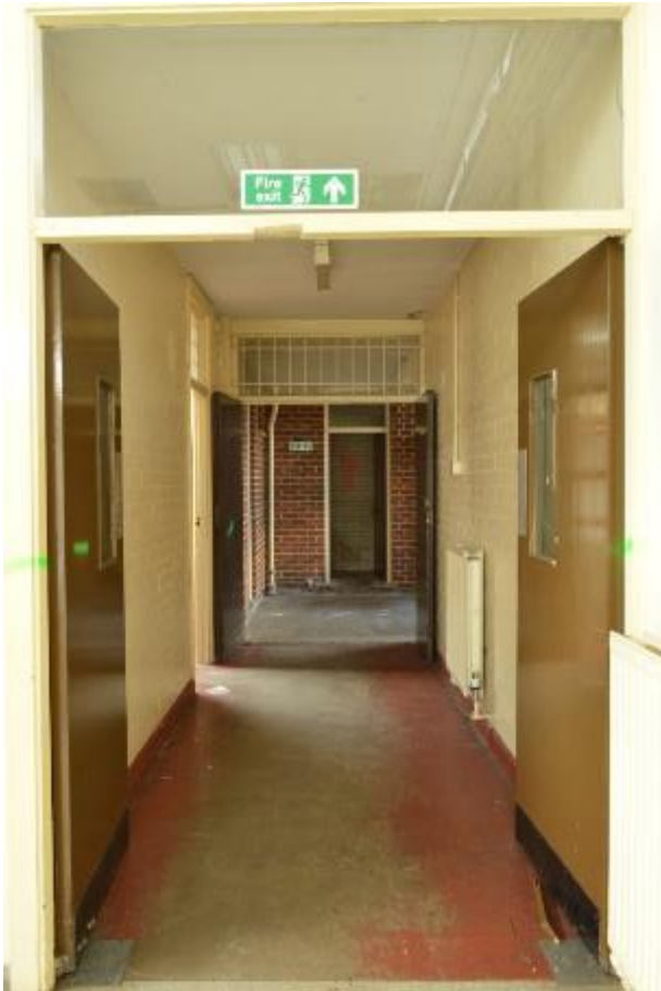
Plate 125: Building 15, access corridor (637)
