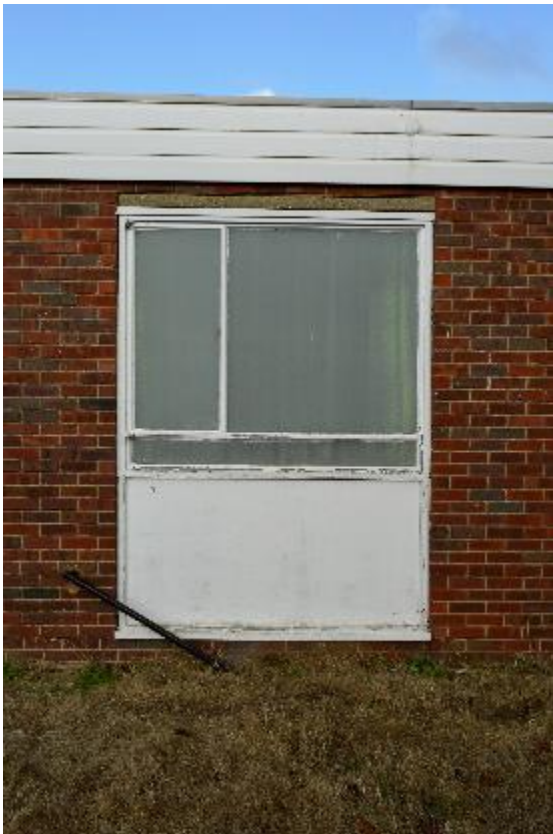
Plate 64: Building 8, south elevation, window arrangement (334)
