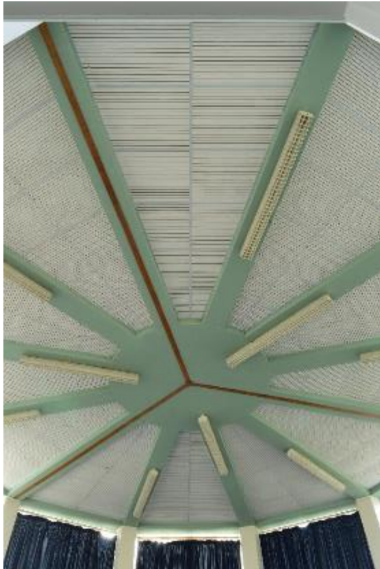
Plate 52: Building 5, band practice room, ceiling construction (297)
