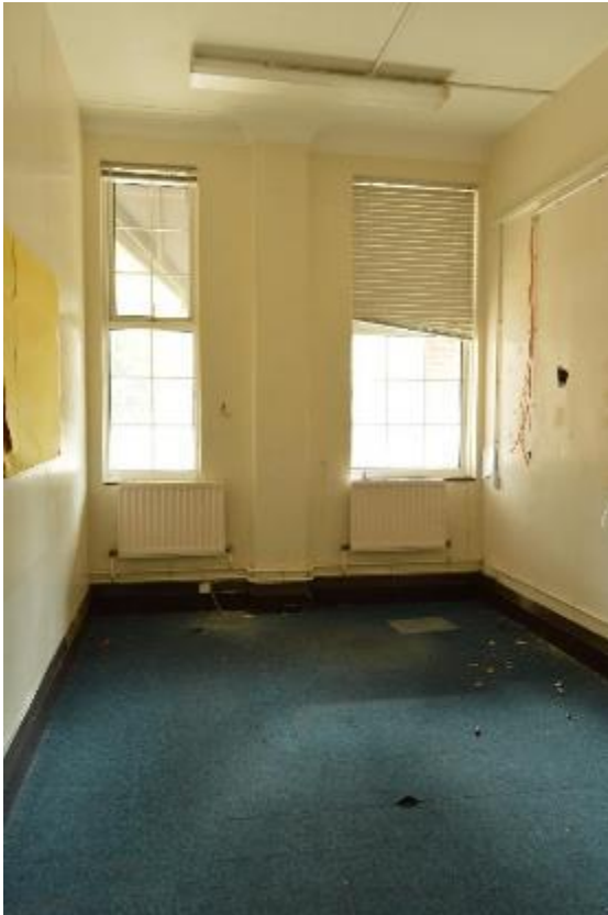
Plate 69: Building 9, original range, ground floor, office (354)
