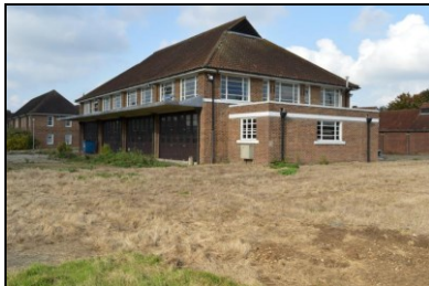
HOB16-0655 Building 17, south-east corner
