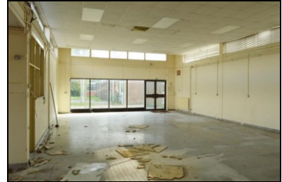
HOB16-0636 Building 15, sports hall
