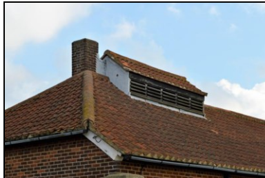
HOB16-0761 Building 22, south-west corner, roof vent and chimney detail
