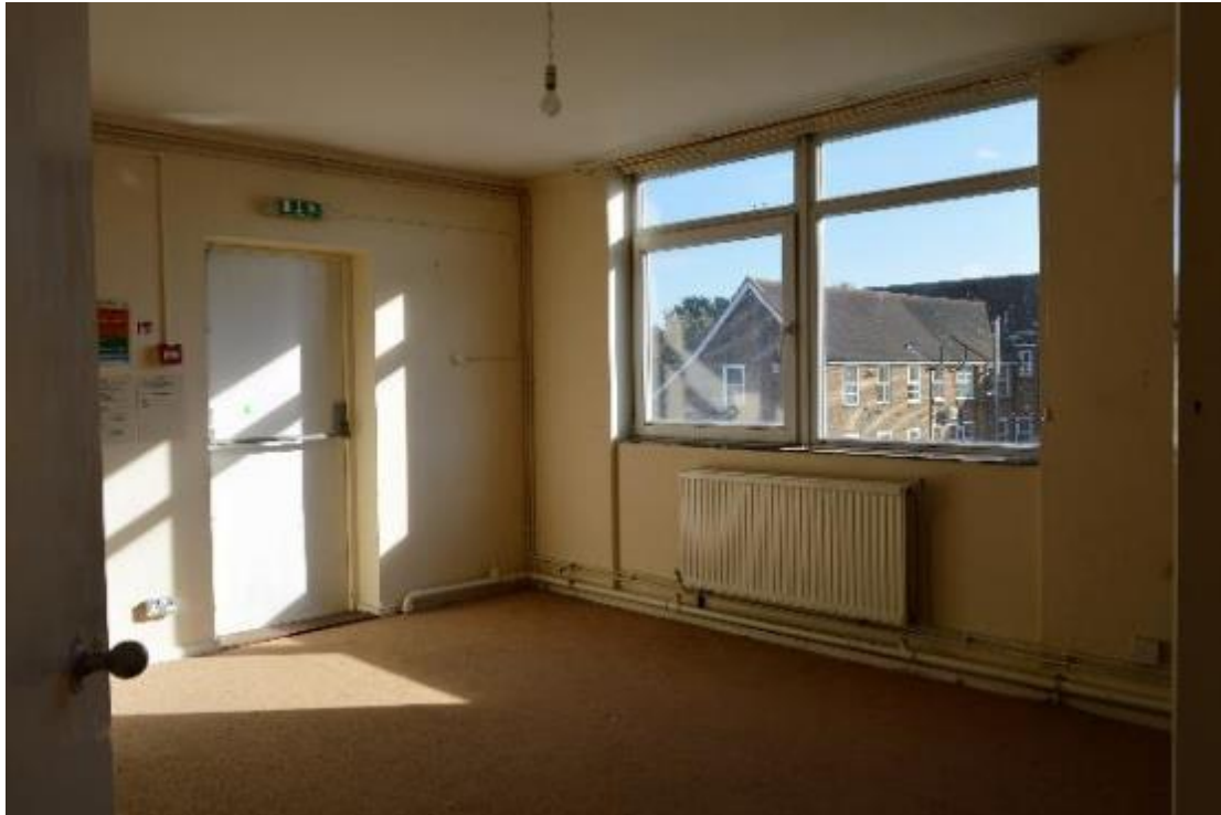
Plate 37: Building 3, north range, first floor, bedroom (257)
