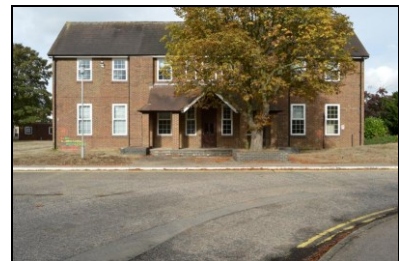
HOB16-0345 Building 9, south elevation, original range
