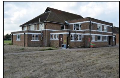
HOB16-0654 Building 17, north-east elevation
