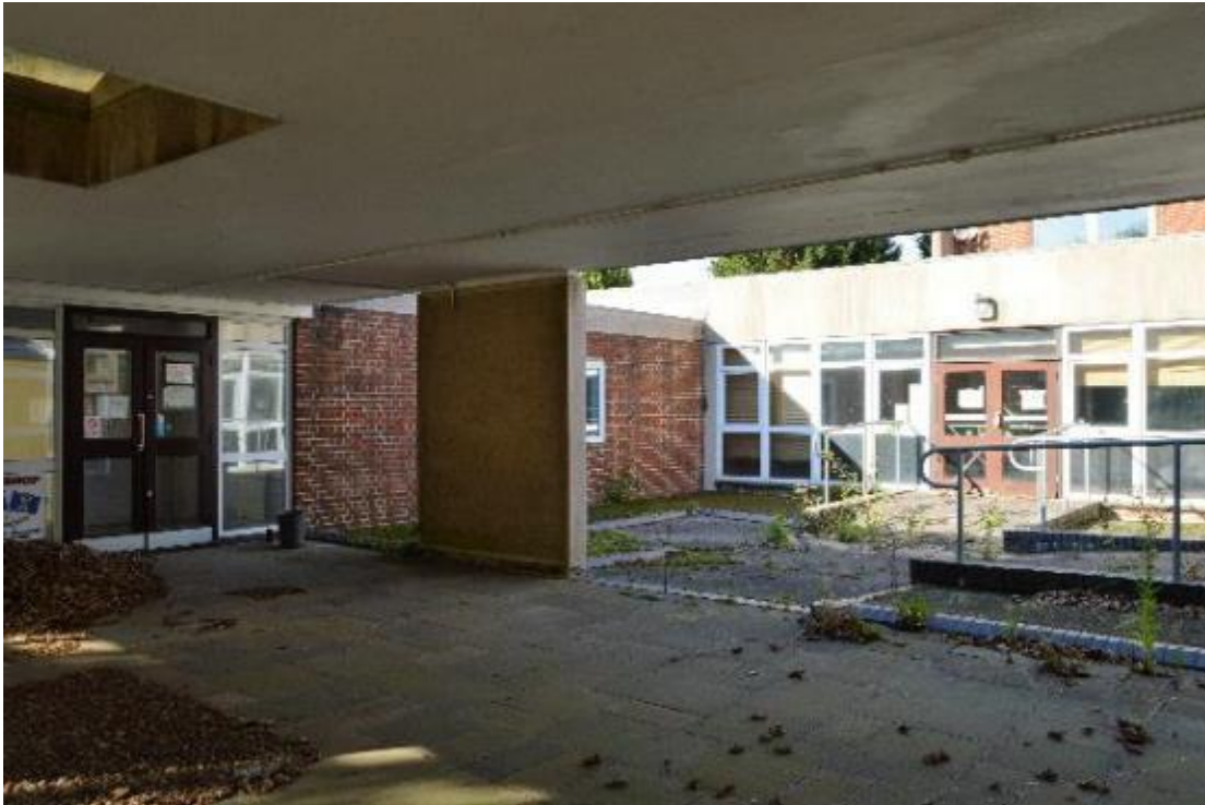
Plate 33: Building 3, internal courtyard (233)
