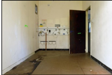
HOB16-0065 Building 1, interior, south extension
