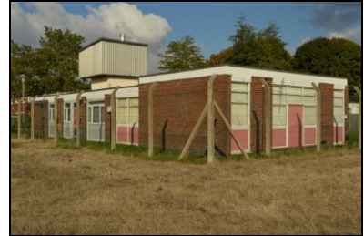
HOB16-0651 Building 16, west elevation
