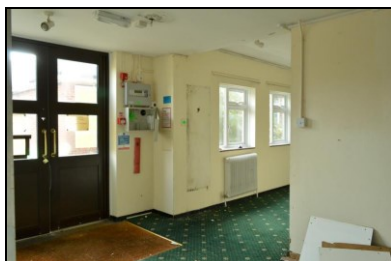
HOB16-0013 Building 1, interior, modern extension
