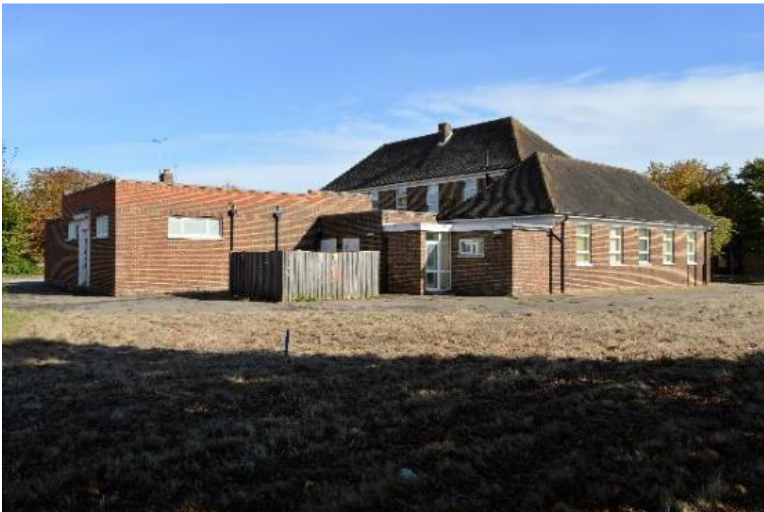
Plate 16: Building 2, south-west corner (112)
