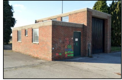
HOB16-0321 Building 7, south-east corner
