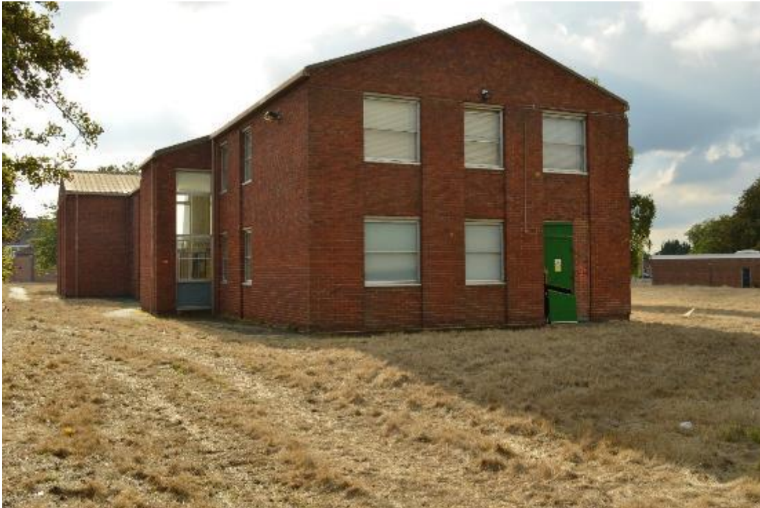
Plate 169: Building 21, north-east corner (732)
