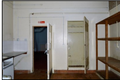
HOB16-0244 Building 3, ground floor
