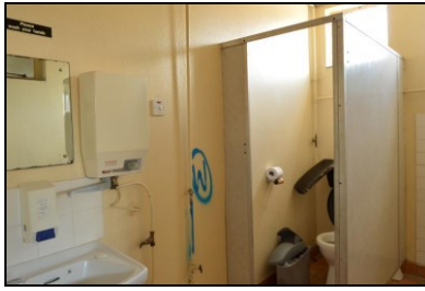
HOB16-0646 Building 15, WC
