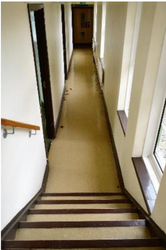
Plate 74: Building 9, north extension, first floor, access corridor (375)
