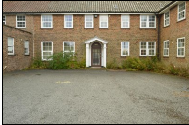
HOB16-0574 Building 14, original range, north elevation, entrance
