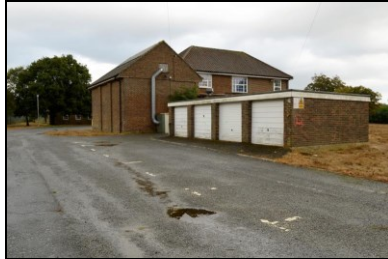
HOB16-0575 Building 14, west elevation
