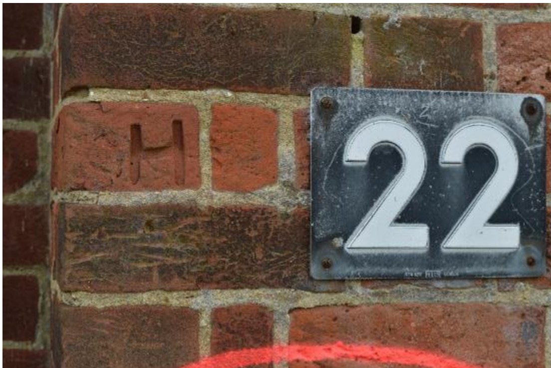
Plate 180: Building 22, north elevation, building identification signage (764)
