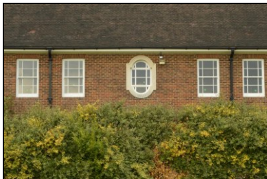
HOB16-0460 Building 12, south-east corner
