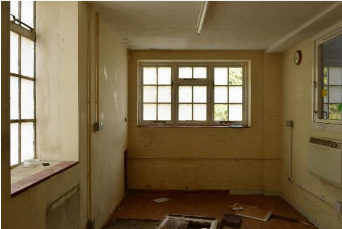
Plate 157: Building 18, west extension (701)
