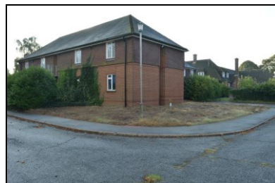
HOB16-0006 Building 1, north-west corner
