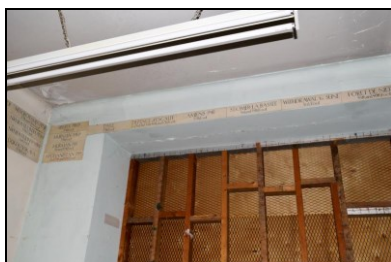
HOB16-0208 Building 2, west extension
