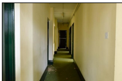
HOB16-0358 Building 9, original range, ground floor
