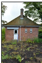
HOB16-0877 Building 90, west elevation and garden
