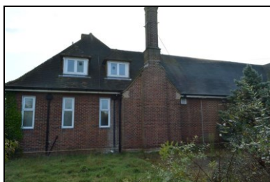
HOB16-0008 Building 1, west elevation
