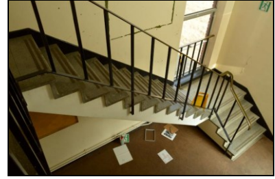
HOB16-0756 Building 21, north-east range, first floor
