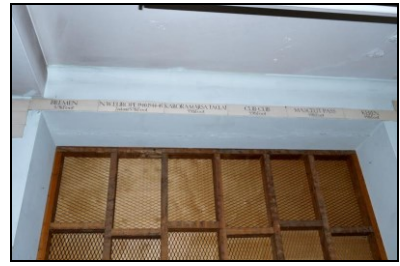
HOB16-0213 Building 2, west extension
