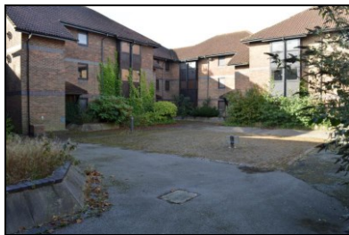
HOB16-0826 Building 25, typical exterior elevation detail and internal courtyard arrangement
