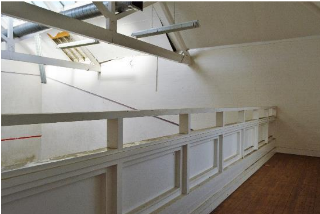
Plate 118: Building 14, original range, first floor, squash court gallery (625)
