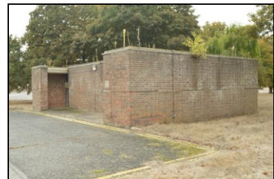
HOB16-0312 Building 6, north-east corner
