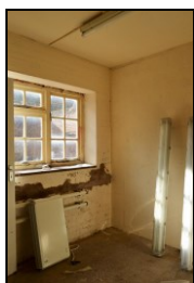
HOB16-0700 Building 18, original range
