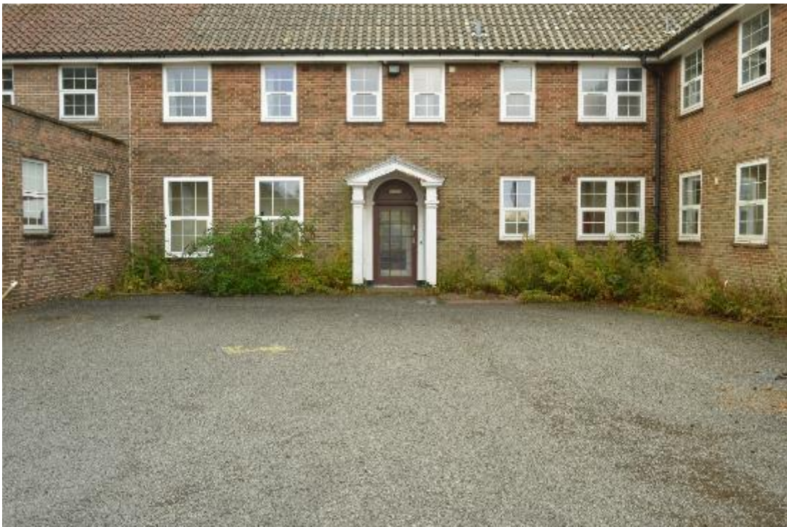
Plate 108: Building 14, original range, north elevation, entrance (574)
