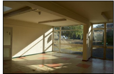
HOB16-0234 Building 3, ground floor
