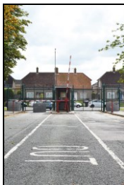
HOB16-0220 Building 2A, north elevation
