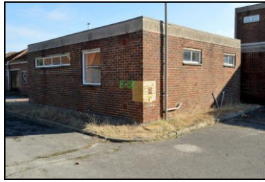
HOB16-0722 Building 20, north-west corner
