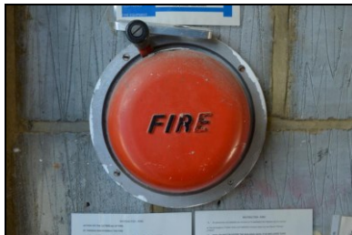
HOB16-0696 Building 18, original range, vehicle maintenance area
