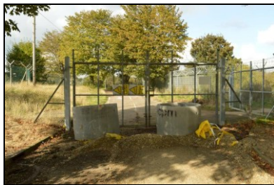
HOB16-0913 Access road at the northern end of the site providing access to Building 24
