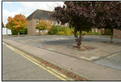
HOB16-0902 Building 12, west elevation
