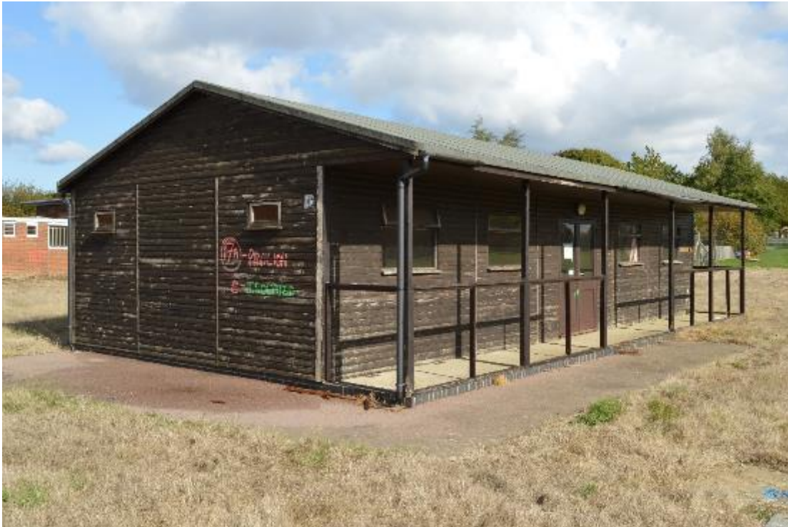
Plate 147: Building 17A, south-west corner (691)
