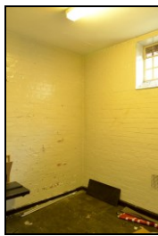
HOB16-0137 Building 2, interior, central range
