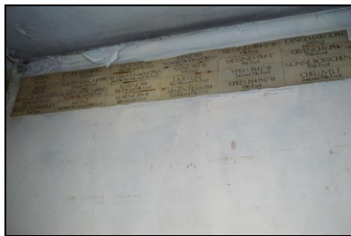
HOB16-0197 Building 2, west extension
