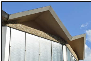
HOB16-0294 Building 5, roof and upper window arrangement
