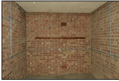
HOB16-0317 Building 6, internal store
