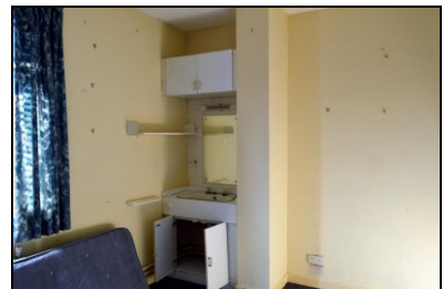
HOB16-0102 Building 1, interior, north range
