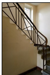
HOB16-0359 Building 9, original range, ground floor, western staircase
