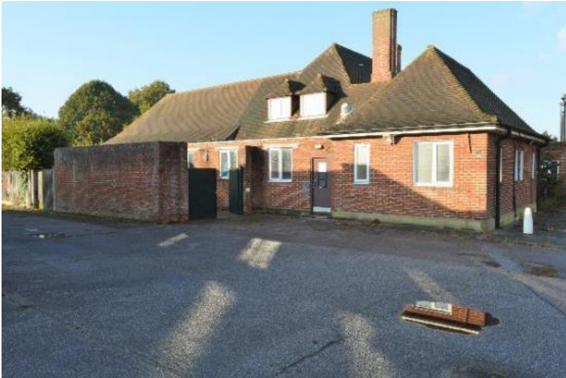
Plate 3: Building 1, original range, east elevation (1)
