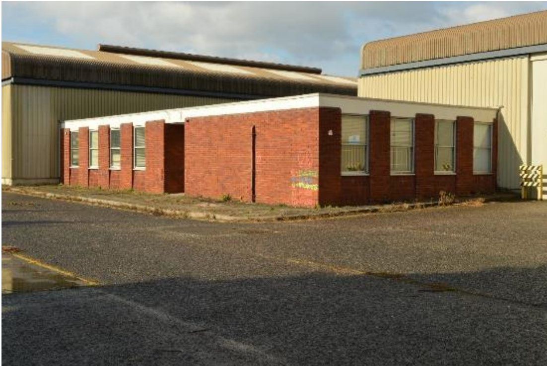
Plate 193: Building 24, central link structure (790)
