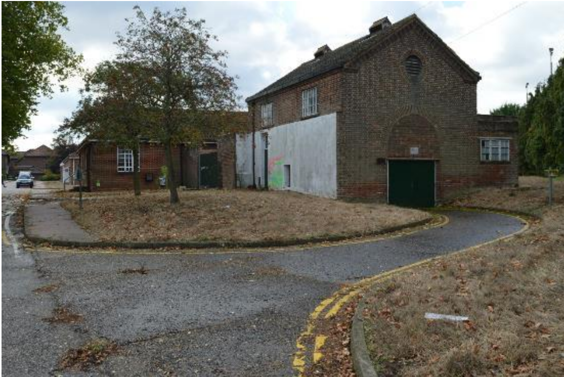
Plate 149: Building 18, north-east corner (429)
