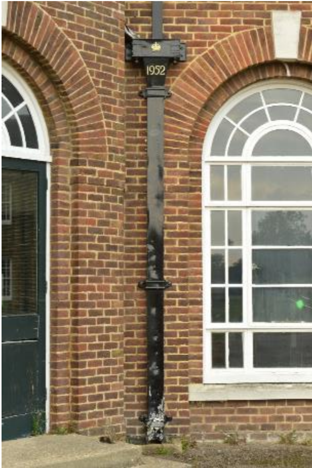
Plate 93: Building 12, south elevation, rainwater date stamp (465)
