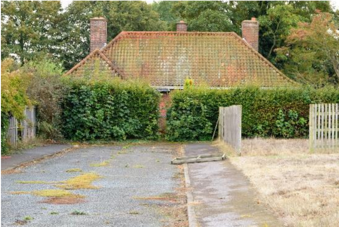
Plate 207: Building 90, north elevation (864)
