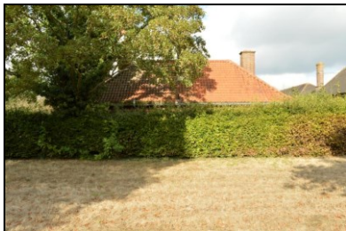
HOB16-0892 View of the west elevation of Building 90
