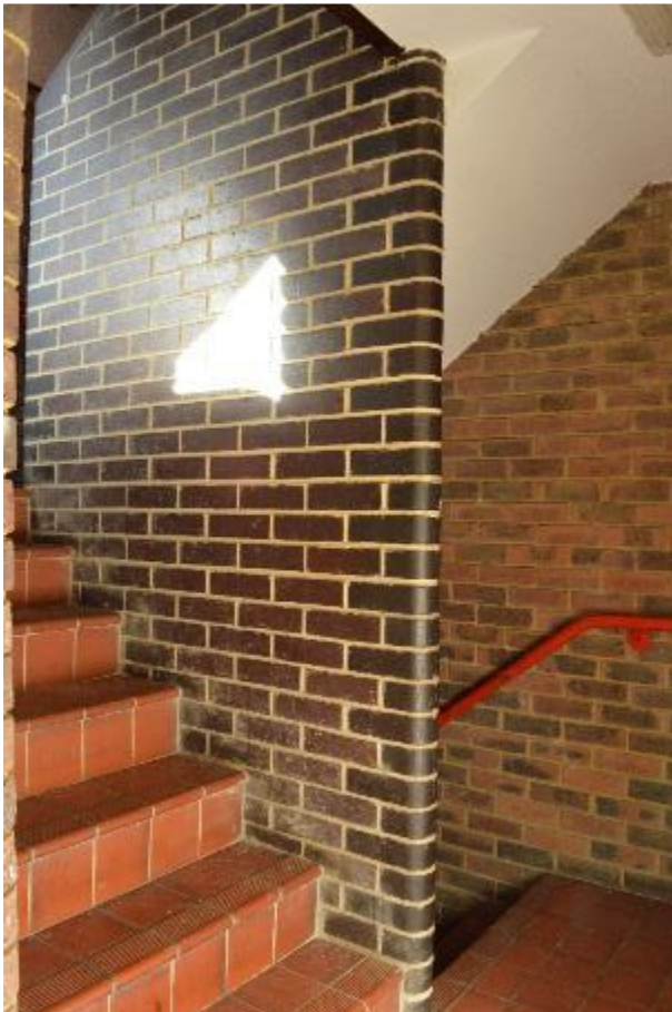
Plate 206: Building 25, typical stairwell arrangement within all blocks (840)
