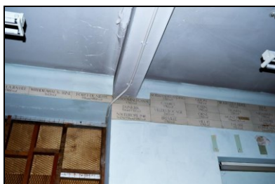
HOB16-0209 Building 2, west extension
