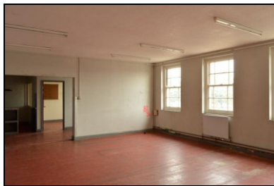
HOB16-0542 Building 12, east wing, first floor
