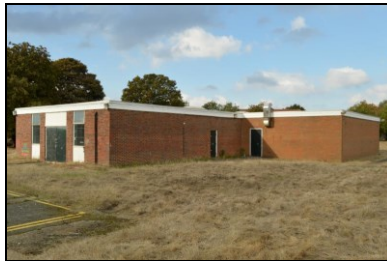
HOB16-0773 Building 23, south-east corner
