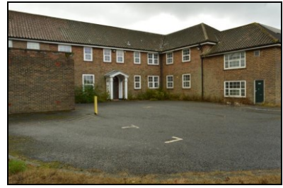
HOB16-0573 Building 14, original range, north elevation
