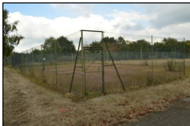
HOB16-0916 Tennis Court at the northern end of the site
