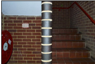
HOB16-0263 Building 4, block 23, ground floor
