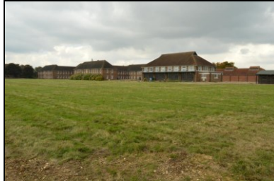
HOB16-0455 Building 12, north-west corner
