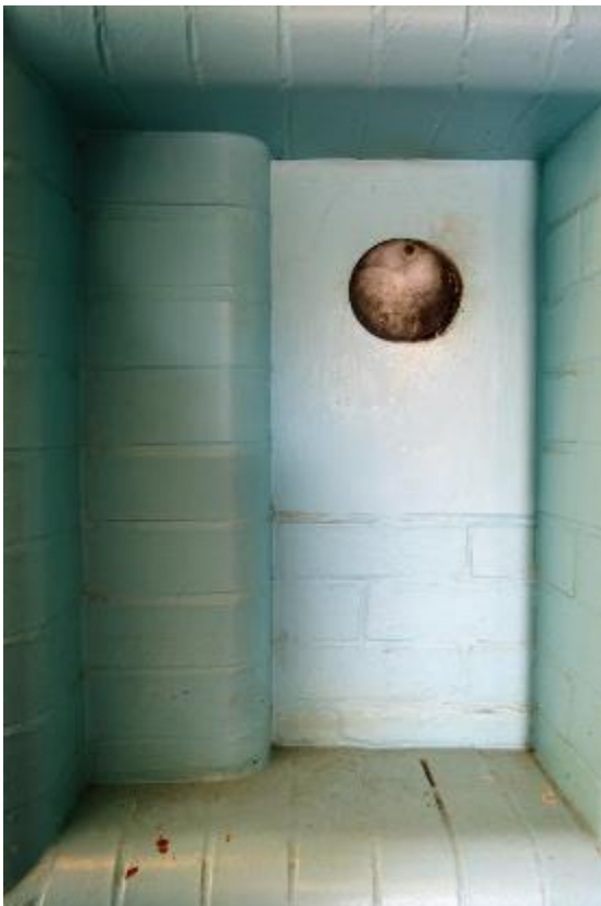
Plate 24: Building 2, north range, ground floor, cell inspection eyelet (150)
