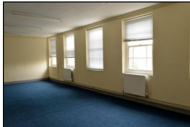
HOB16-0533 Building 12, east wing, first floor
