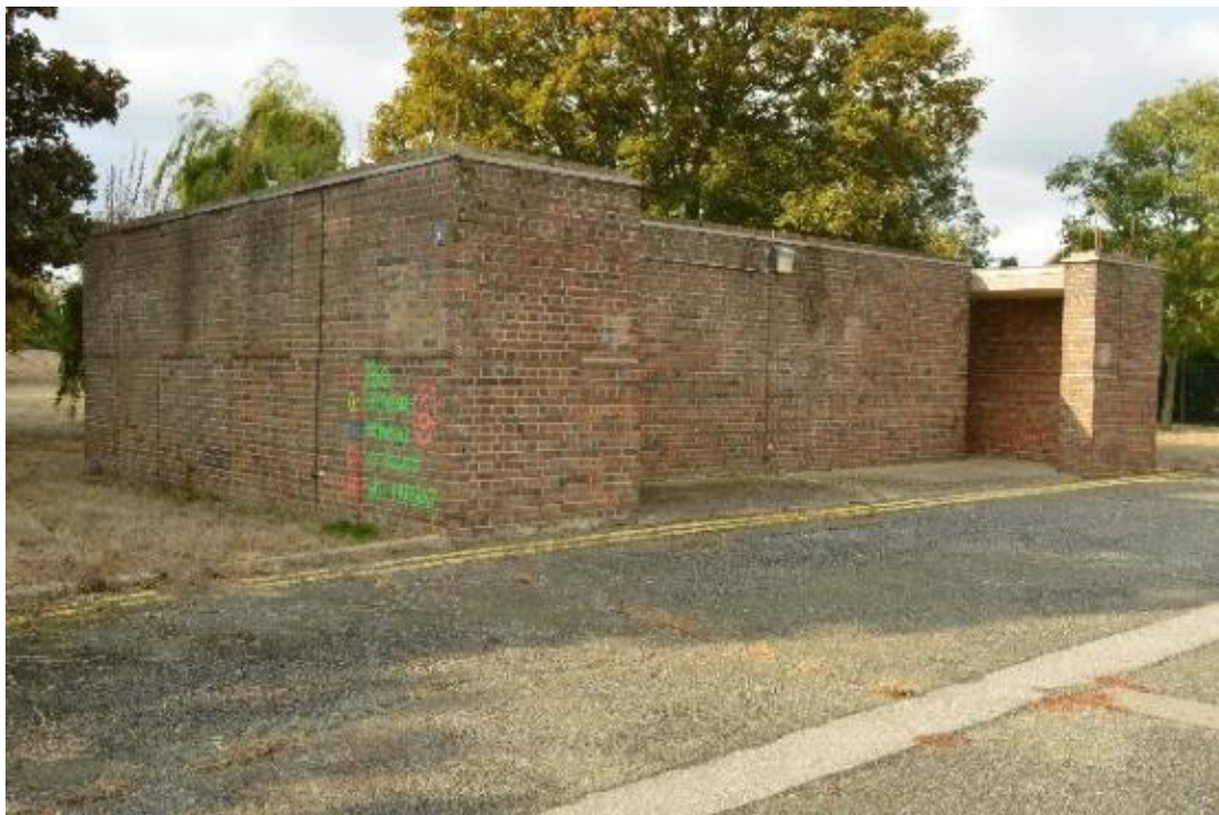
Plate 54: Building 6, east elevation (314)
