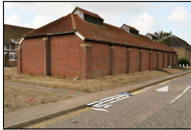
HOB16-0758 Building 22, north-east corner
