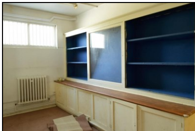
HOB16-0217 Building 2, west extension
