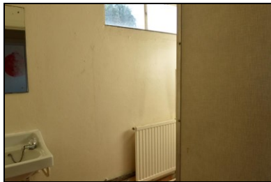
HOB16-0727 Building 20, WC
