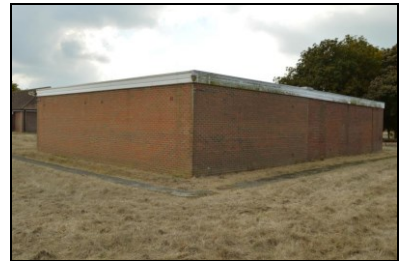
HOB16-0774 Building 23, south-east corner
