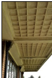
HOB16-0659 Building 17, south elevation, veranda detailing
