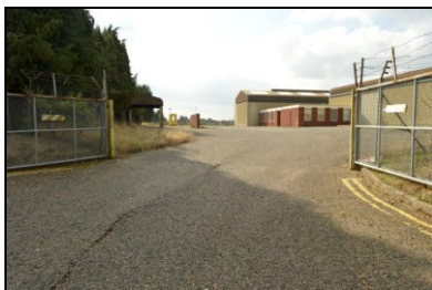
HOB16-0910 Access road at the northern end of the site providing access to Building 24
