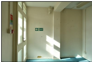
HOB16-0166 Building 2, central range
