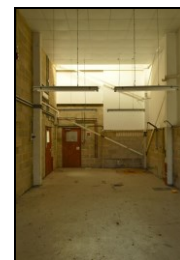
HOB16-0795 Building 24, west range, garage
