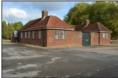
HOB16-0424 Building 11, south-west corner
