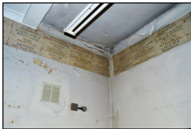
HOB16-0196 Building 2, west extension
