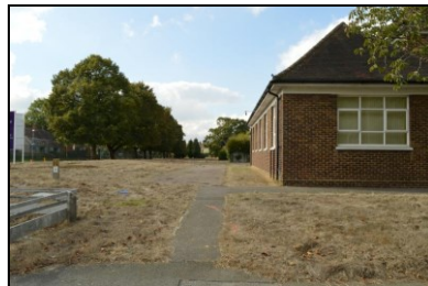
HOB16-0890 Site land separating Building 2 from Littlebourne Road
