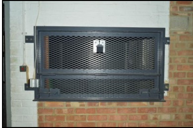
HOB16-0784 Building 23, original range, store service hatch
