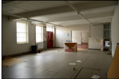
HOB16-0529 Building 12, east wing, ground floor
