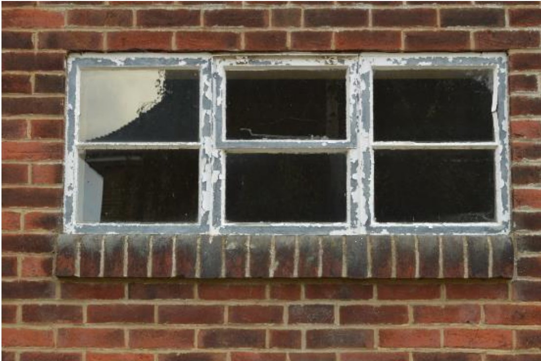
Plate 177: Building 22, west elevation, window arrangement (762)
