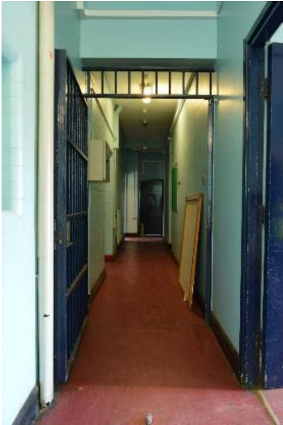
Plate 25: Building 2, north range, ground floor, corridor (121)
