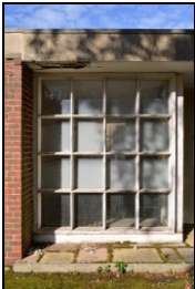
HOB16-0232 Building 3, south elevation, window arrangement
