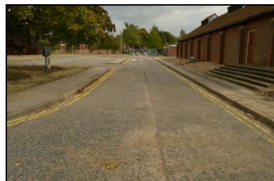
HOB16-0924 Access road to the north of Building 22
