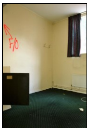
HOB16-0583 Building 14, east extension, ground floor
