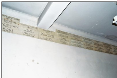
HOB16-0199 Building 2, west extension
