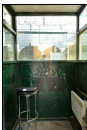
HOB16-0223 Building 2A, interior
