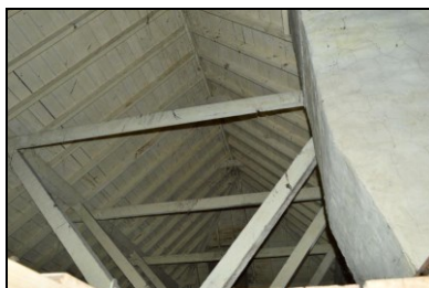
HOB16-0875 Building 90, roof and central chimney construction
