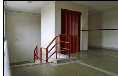
HOB16-0531 Building 12, east wing, first floor
