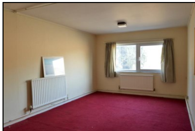
HOB16-0248 Building 3, north range
