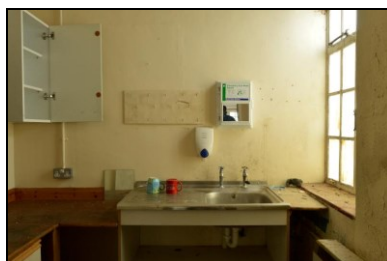
HOB16-0702 Building 18, west extension
