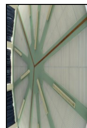
HOB16-0297 Building 5, band practice room, ceiling construction
