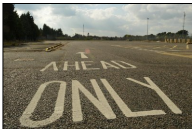
HOB16-0911 Access road at the northern end of the site providing access to Building 24
