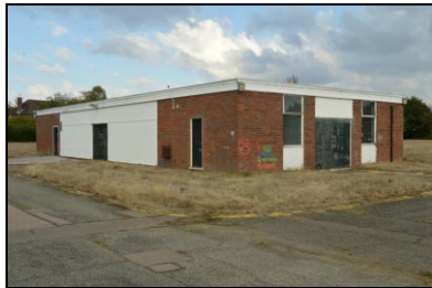
HOB16-0772 Building 23, south-west corner
