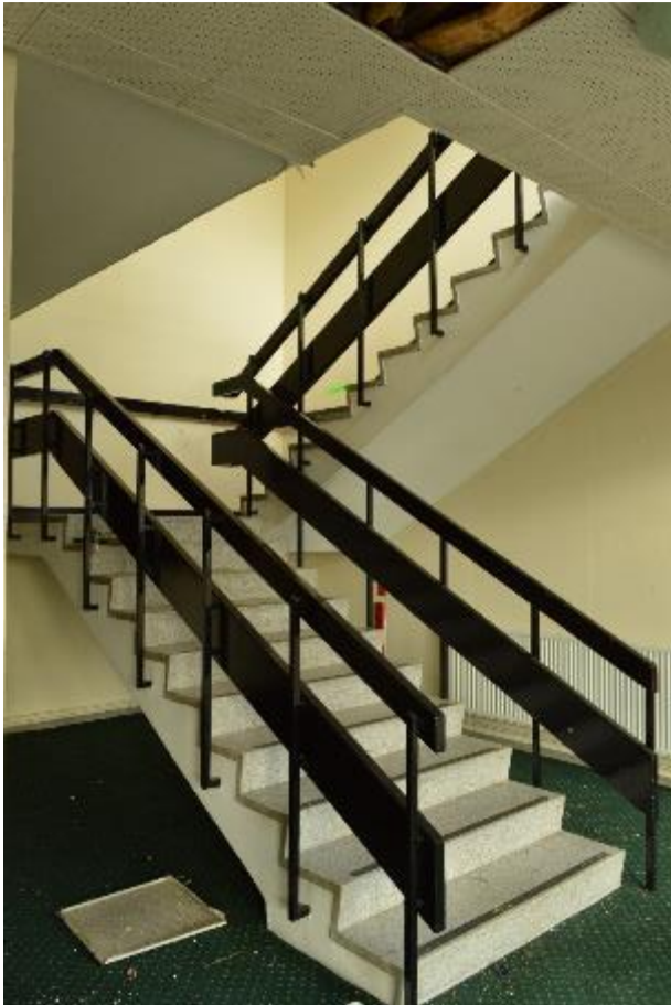
Plate 111: Building 14, east extension, ground floor, lobby (580)
