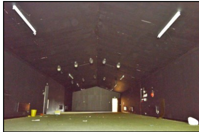
HOB16-0769 Building 22, interior firing range, facing east
