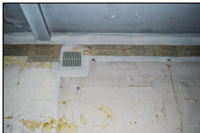
HOB16-0205 Building 2, west extension
