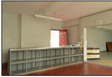
HOB16-0527 Building 12, east wing, ground floor
