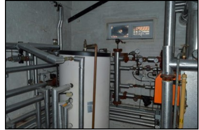
HOB16-0246 Building 3, ground floor
