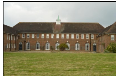
HOB16-0459 Building 12, south-east corner
