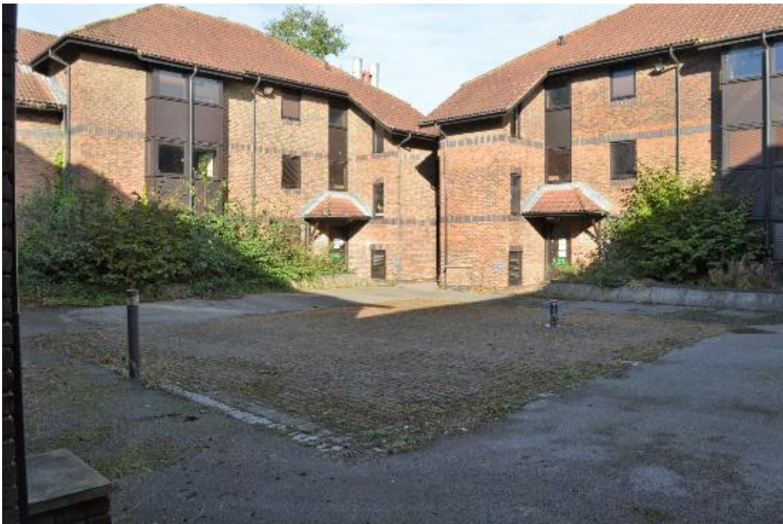
Plate 200: Building 25, typical exterior elevation detail and north courtyard arrangement (825)
