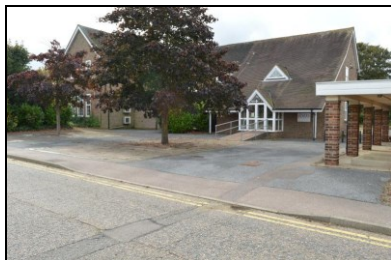
HOB16-0349 Building 9, east elevation, north extension
