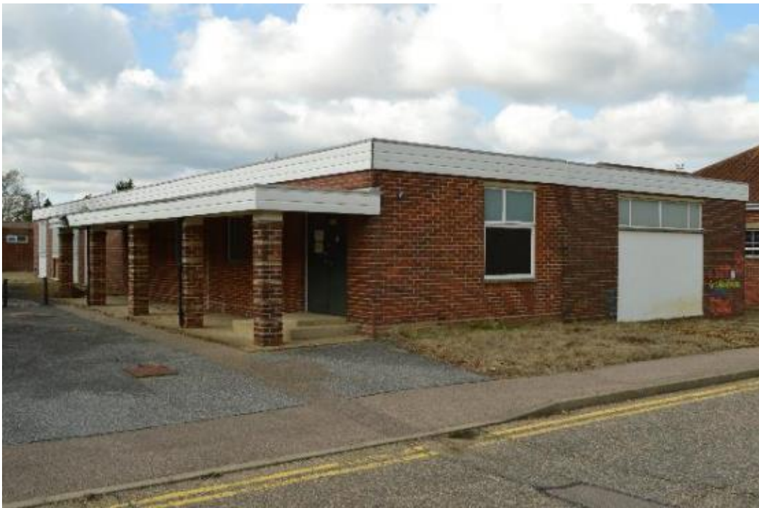
Plate 62: Building 8, south-east elevation (331)
