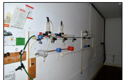
HOB16-0240 Building 3, ground floor
