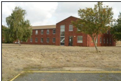
HOB16-0730 Building 21, west elevation
