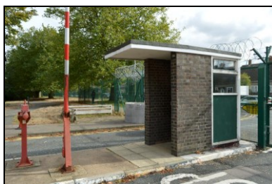
HOB16-0224 Building 2A, west elevation
