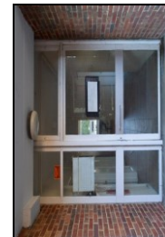
HOB16-0729 Building 20, southern entrance
