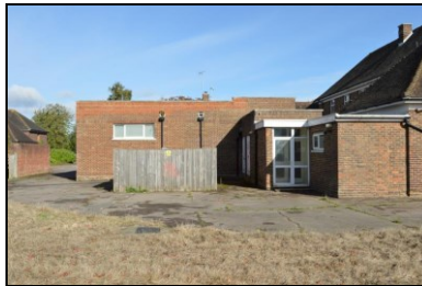
HOB16-0113 Building 2, west elevation
