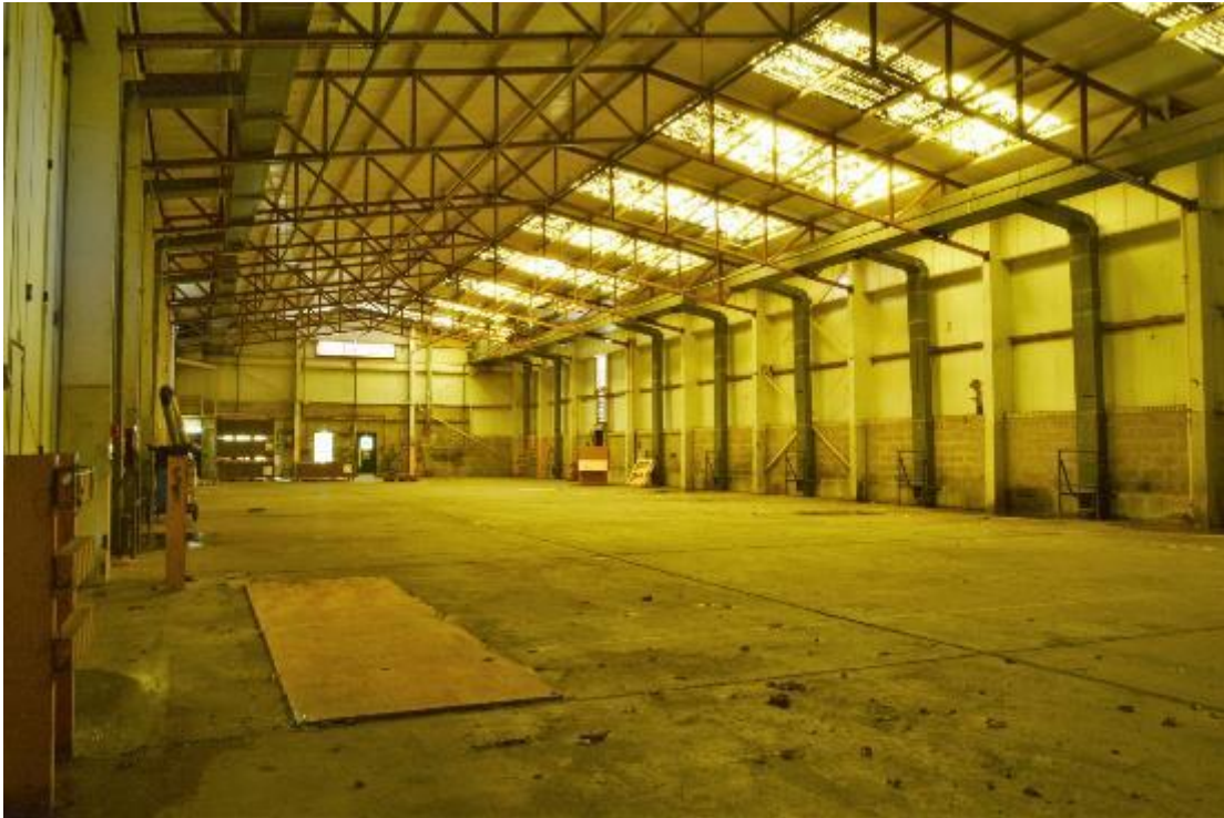
Plate 195: Building 24, east range, car hangar (810)
