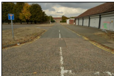
HOB16-0923 Access road to the west of Building 19
