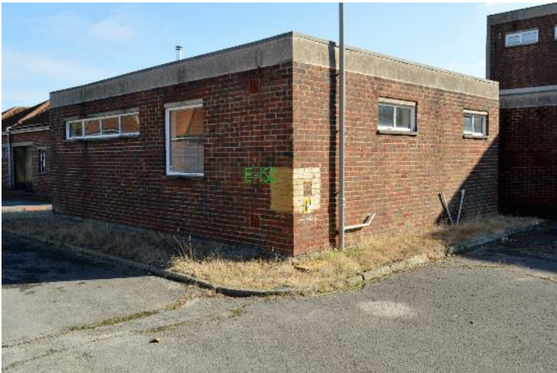
Plate 166: Building 20, north-west corner (722)
