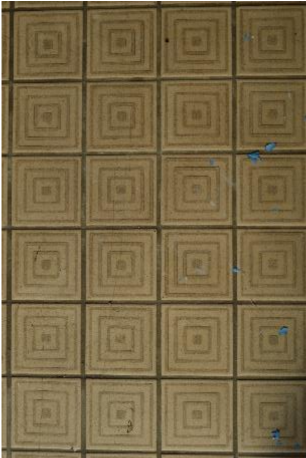
Plate 137: Building 17, north range, ground floor, lobby floor tiles (689)
