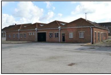
HOB16-0406 Building 10, north-west corner
