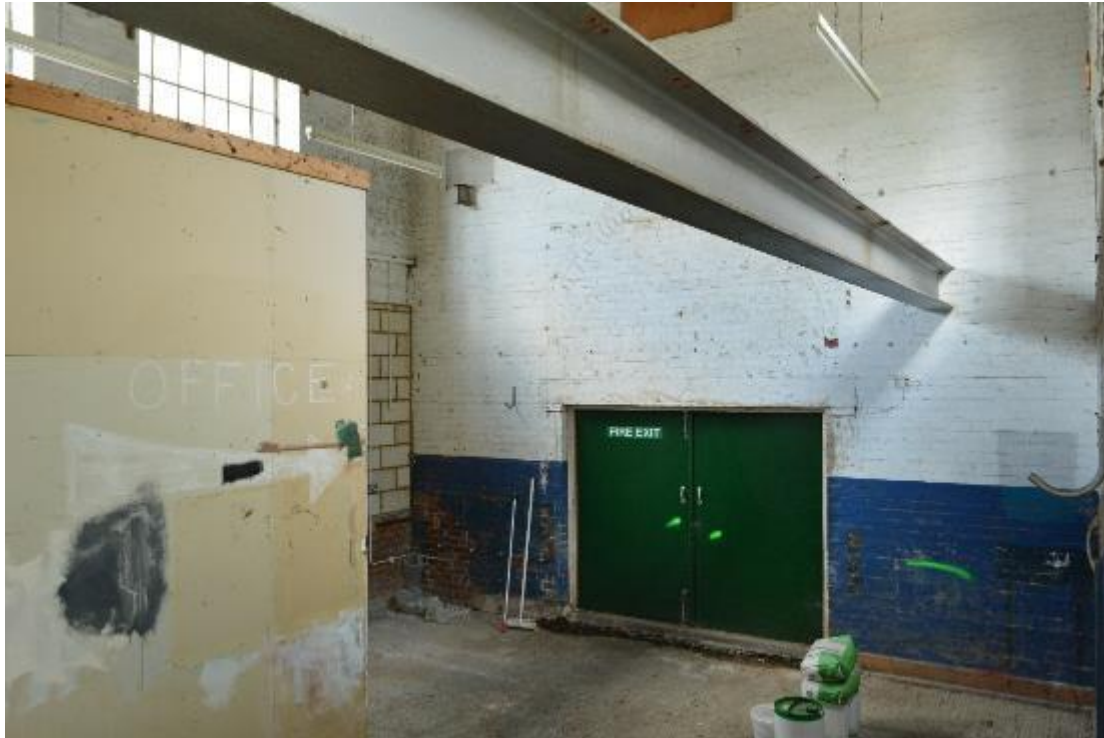
Plate 155: Building 18, original range, vehicle maintenance area (697)
