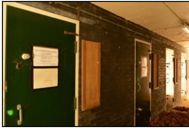
HOB16-0316 Building 6, eastern internal passage
