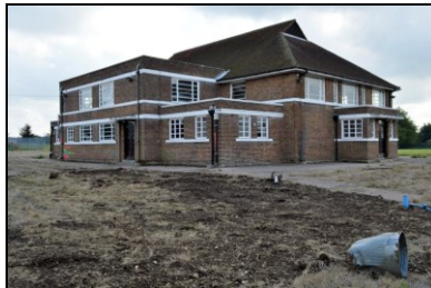
HOB16-0653 Building 17, north-west corner
