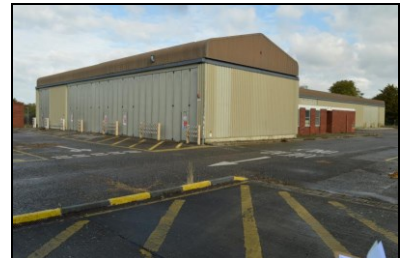
HOB16-0792 Building 24, west elevation
