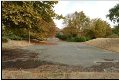
HOB16-0898 View of the car park to the north of Building 2, south elevation of Bunker 2 (right)
