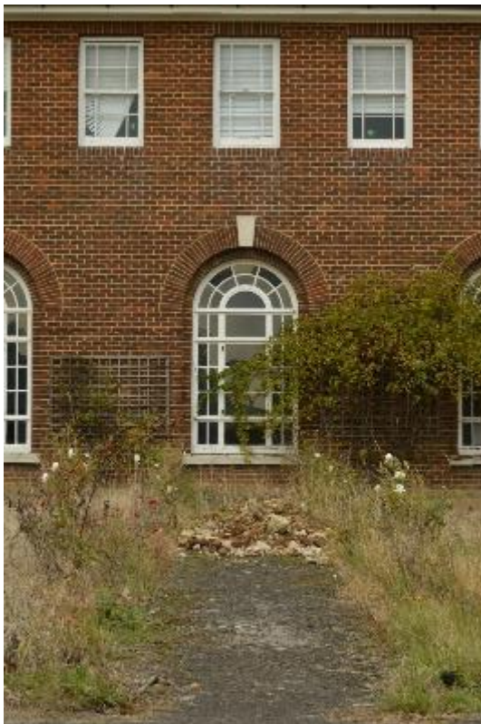
Plate 96: Building 12, south elevation, landscaping and window arrangement (462)
