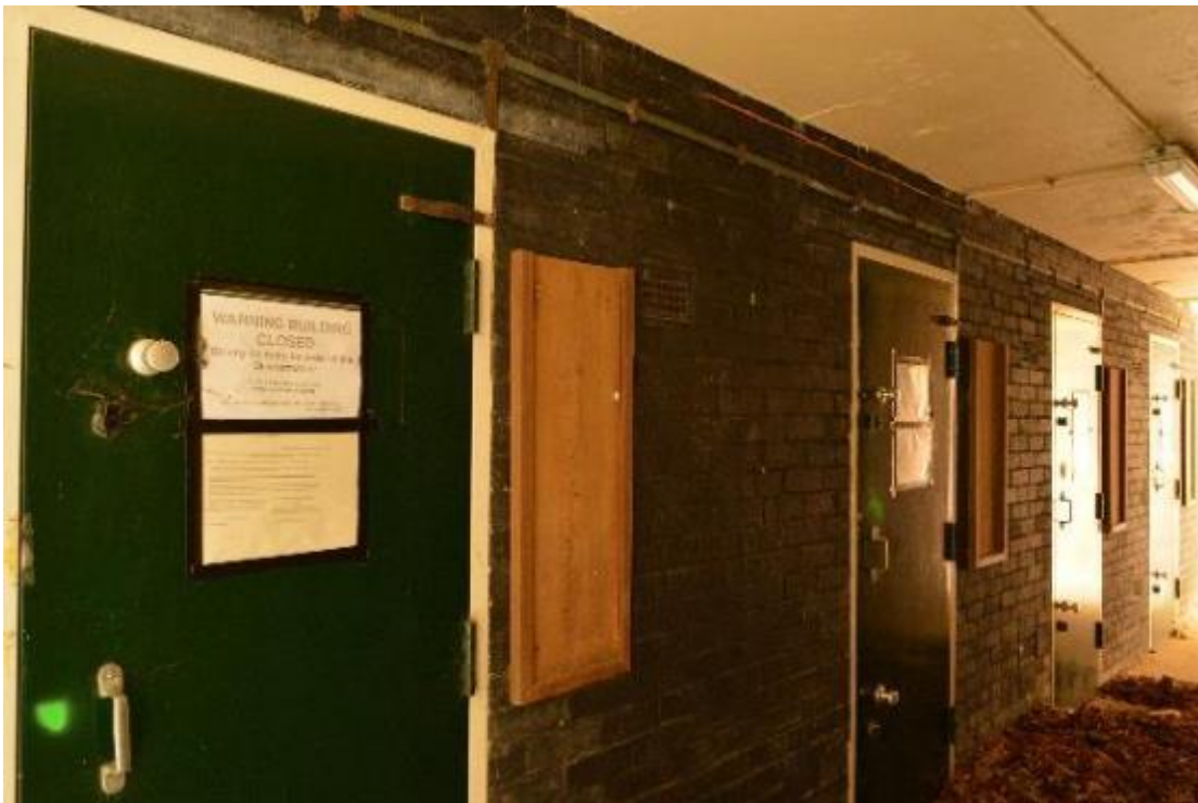
Plate 58: Building 6, eastern internal passage (316)
