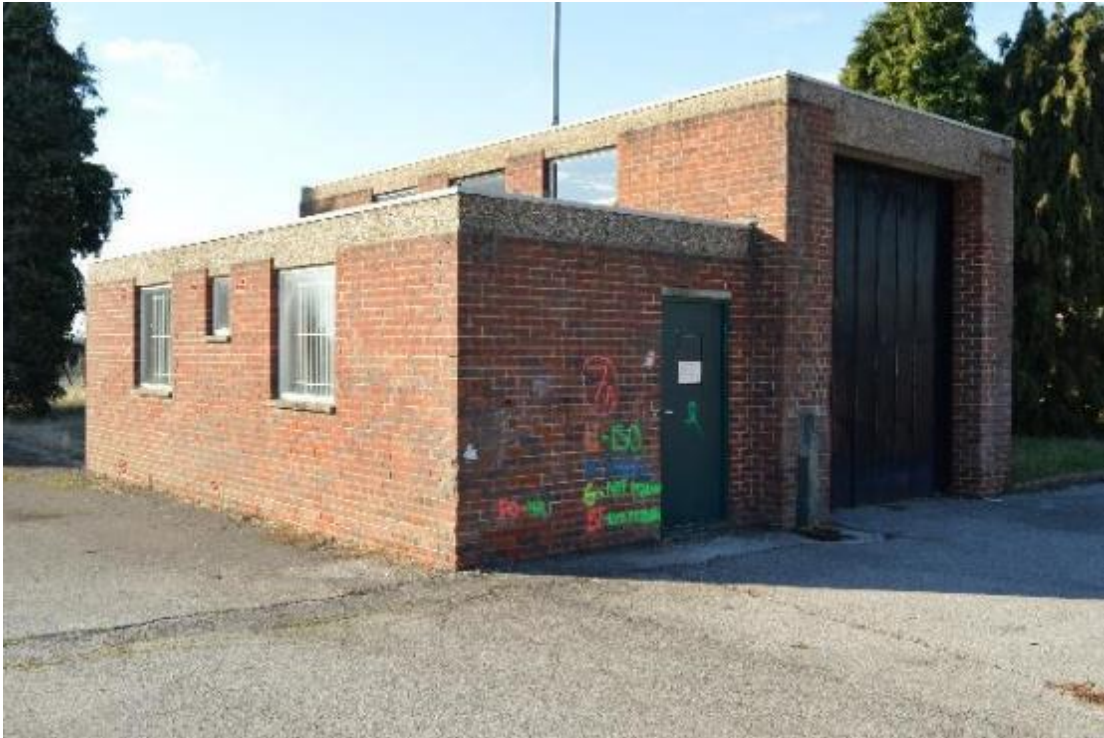
Plate 59: Building 7, south-east elevation (321)
