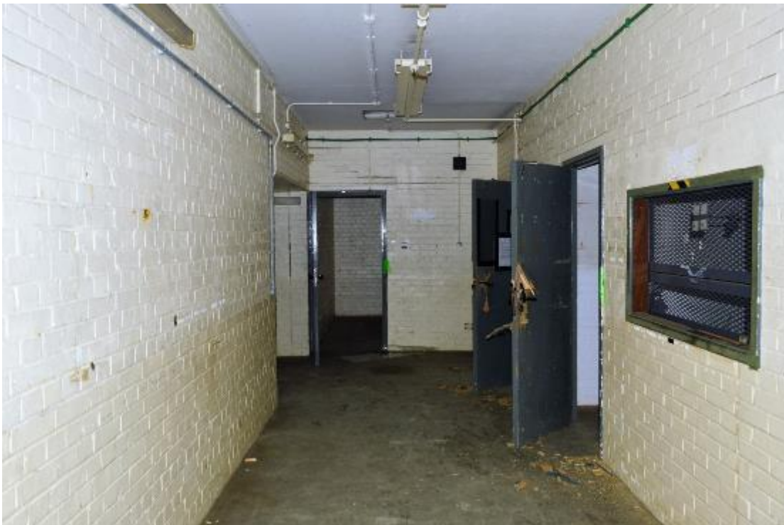
Plate 188: Building 23, east extension corridor (782)
