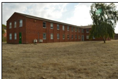
HOB16-0733 Building 21, north-west corner
