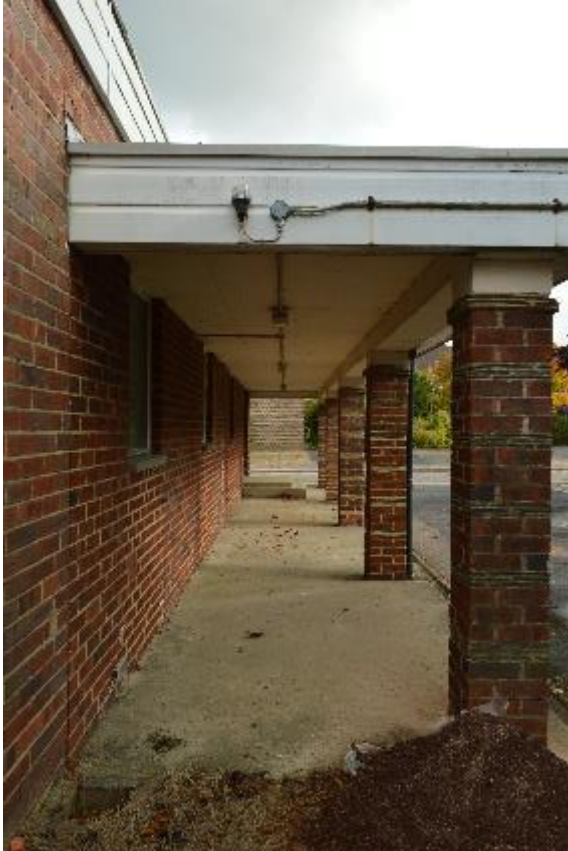
Plate 63: Building 8, south-east elevation (333)
