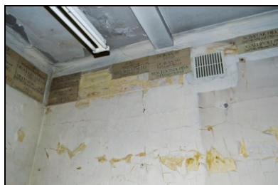
HOB16-0204 Building 2, west extension
