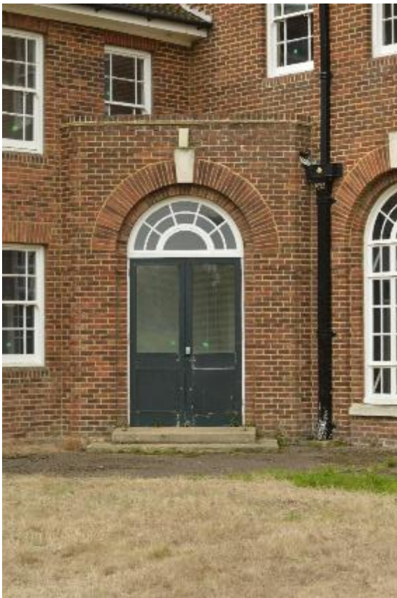
Plate 100: Building 12, south elevation, doorway into central range (463)
