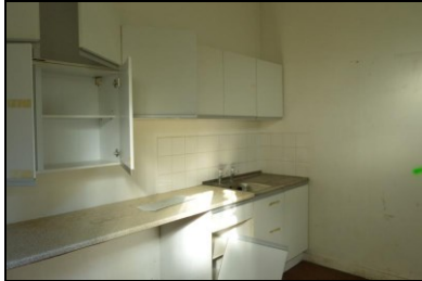
HOB16-0064 Building 1, interior, south extension
