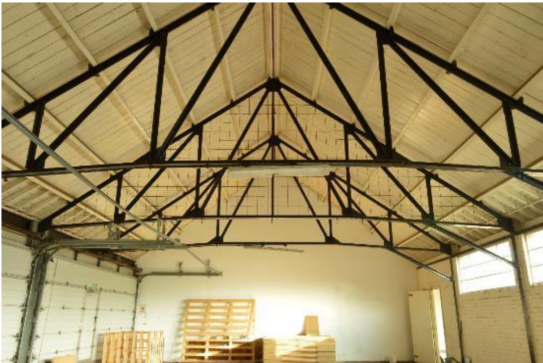
Plate 162: Building 19, original range, southern garage, roof truss arrangement (713)
