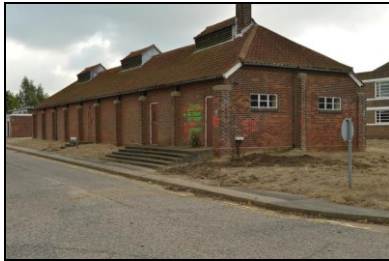
HOB16-0757 Building 22, north-west corner
