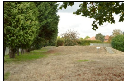
HOB16-0894 View of Bunker 1, south elevation
