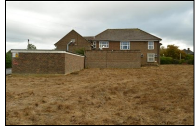
HOB16-0576 Building 14, west elevation
