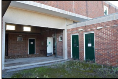
HOB16-0245 Building 3, north courtyard
