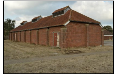
HOB16-0759 Building 22, south-east corner
