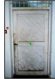
HOB16-0066 Building 1, interior, south extension
