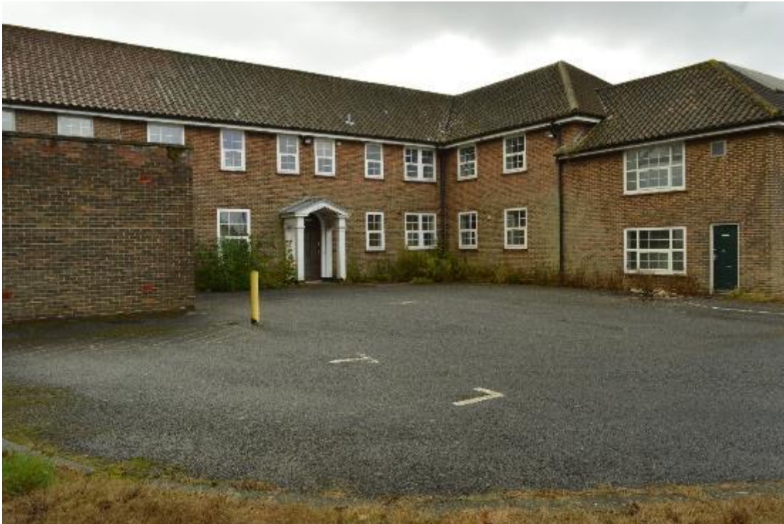
Plate 107: Building 14, original range, north elevation (573)
