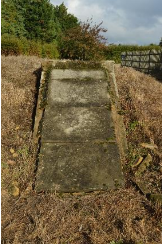
Plate 215: Bunker 1, south entrance (880)
