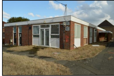
HOB16-0335 Building 8, south-west corner
