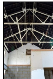
HOB16-0699 Building 18, original range, vehicle maintenance area
