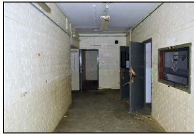
HOB16-0782 Building 23, east extension corridor
