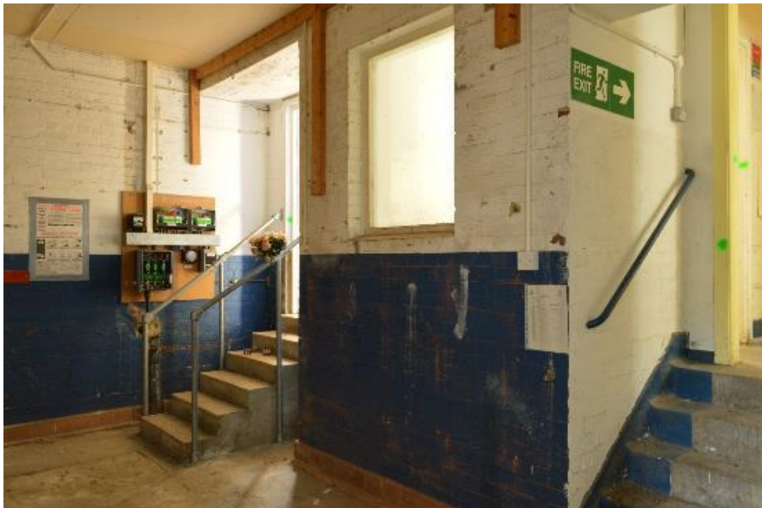
Plate 156: Building 18, original range, inserted lobby (703)
