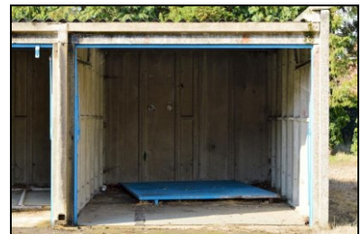
HOB16-0105 Building 1A, east extension
