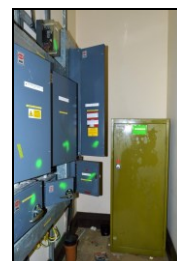
HOB16-0360 Building 9, original range, ground floor
