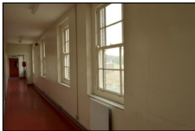
HOB16-0541 Building 12, east wing, first floor
