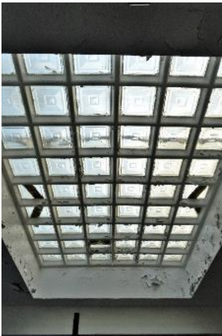
Plate 146: Building 17, north range, first floor, additional gym facility, skylight detailing (686)
