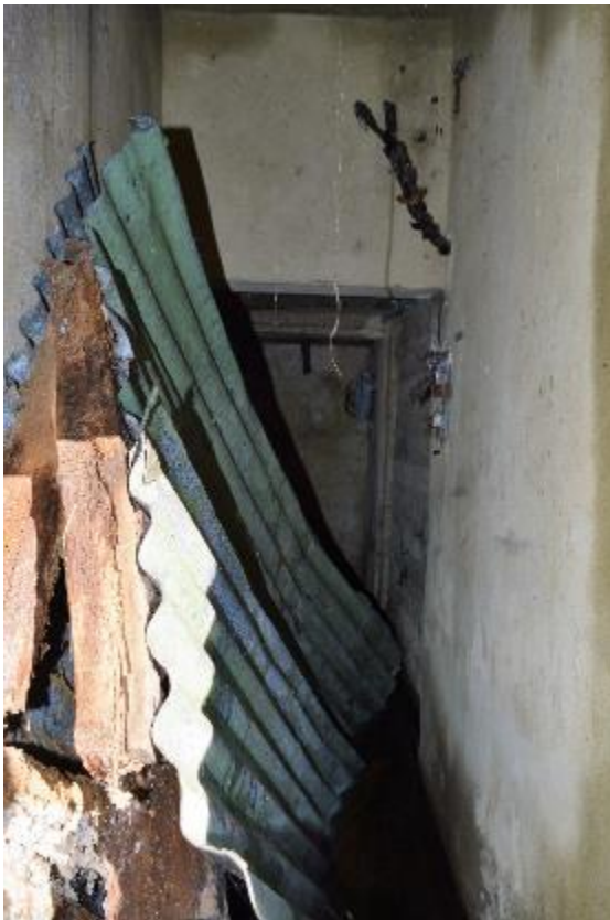
Plate 216: Bunker 1, south entrance, interior passage (881)
