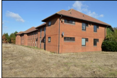
HOB16-0259 Building 4, south-west corner
