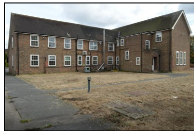
HOB16-0348 Building 9, west elevation, north extension
