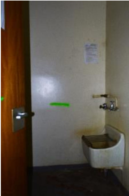
Plate 171: Building 21, north-east range, ground floor, store (746)
