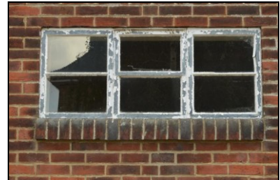
HOB16-0762 Building 22, west elevation, window arrangement
