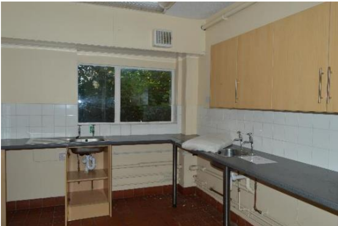
Plate 42: Building 4, block 24, first floor, kitchen (280)
