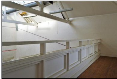
HOB16-0625 Building 14, original range, first floor, squash court gallery
