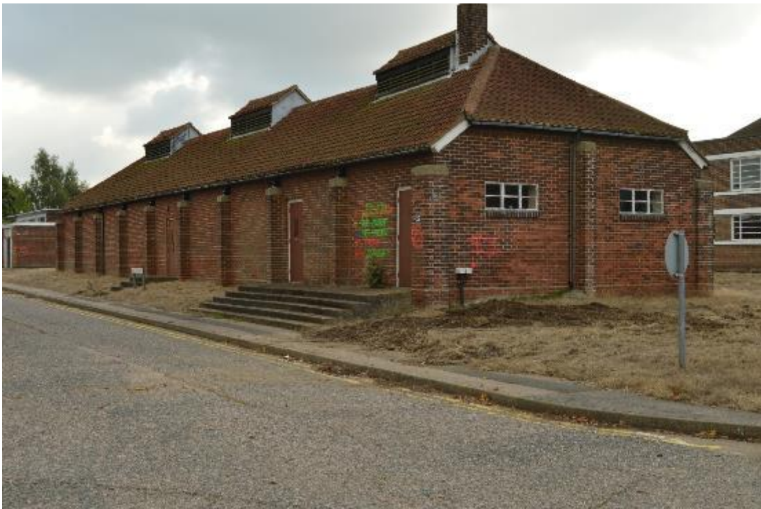
Plate 178: Building 22, north-west corner (757)
