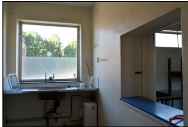
HOB16-0725 Building 20, reception
