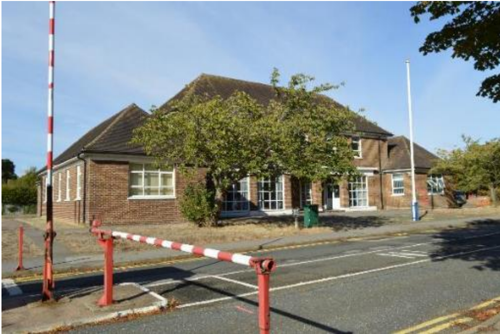
Plate 17: Building 2, east elevation (109)
