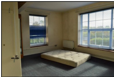
HOB16-0622 Building 14, original range, first floor
