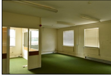
HOB16-0755 Building 21, north-east range, ground floor
