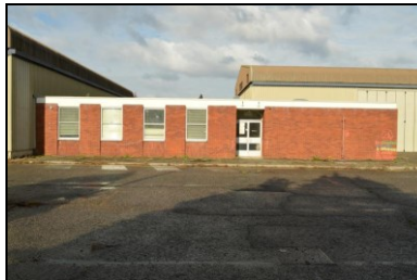
HOB16-0791 Building 24, central link structure
