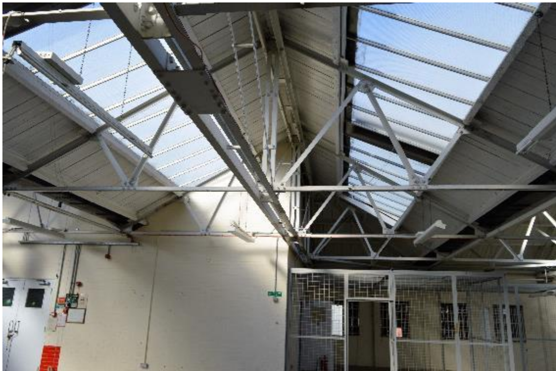
Plate 80: Building 10, principal store, truss arrangement (417)
