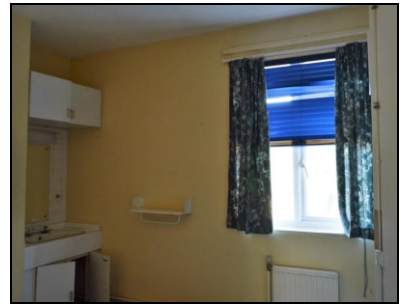
HOB16-0093 Building 1, interior, north range
