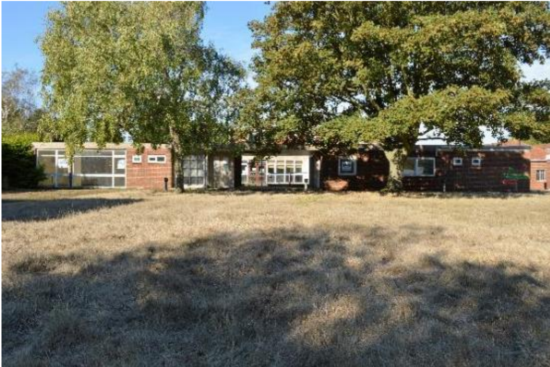
Plate 31: Building 3, south elevation (225)
