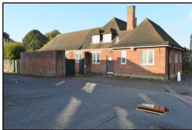
HOB16-0001 Building 1, original range, east elevation
