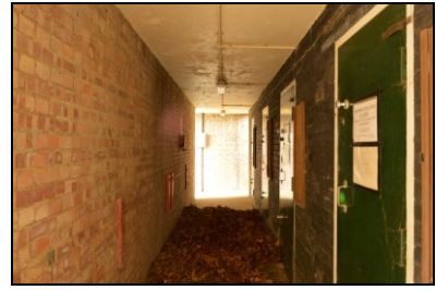
HOB16-0318 Building 6, north internal passage
