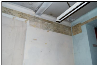
HOB16-0207 Building 2, west extension
