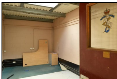
HOB16-0800 Building 24, west range, office
