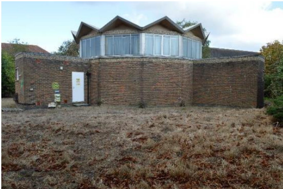
Plate 44: Building 5, south side (291)
