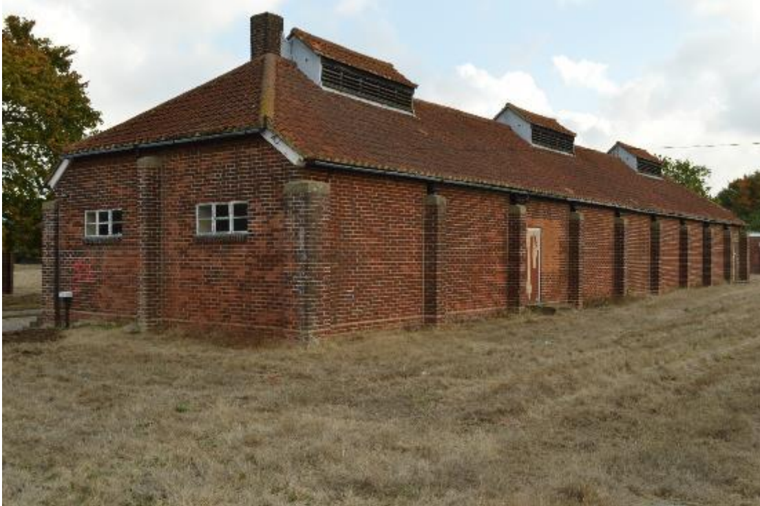
Plate 175: Building 22, south-west corner (760)
