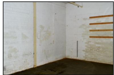
HOB16-0777 Building 23, original range
