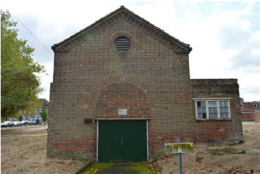
Plate 152: Building 18, north elevation (428)
