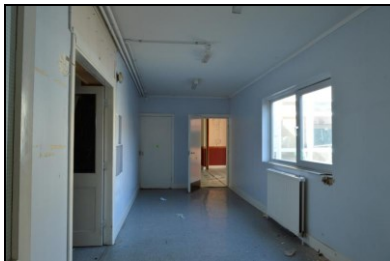
HOB16-0235 Building 3, ground floor
