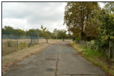
HOB16-0917 Access road to Building 14
