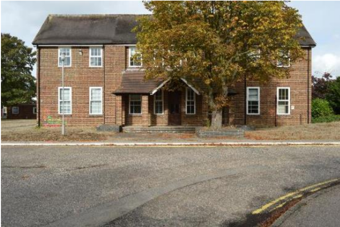
Plate 67: Building 9, south elevation, original range (345)
