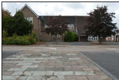
HOB16-0350 Building 9, east elevation, north extension
