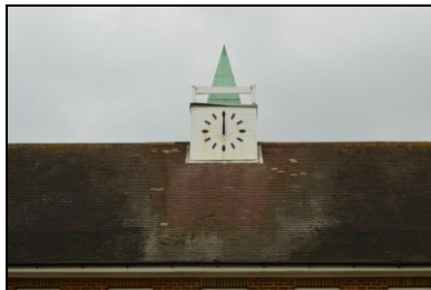
HOB16-0461 Building 12, south elevation, central clock tower
