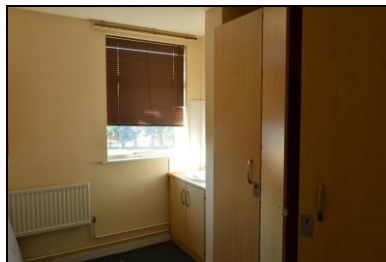
HOB16-0288 Building 4, block 24, first floor
