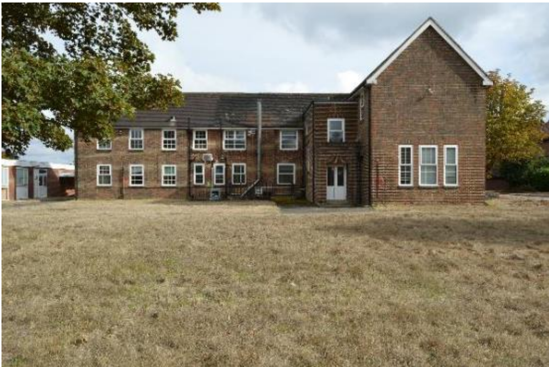
Plate 68: Building 9, west elevation, north extension (347)
