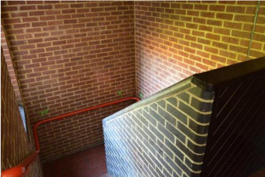
Plate 41: Building 4, block 23, first floor, staircase (272)
