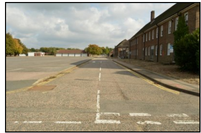
HOB16-0906 View of the Drill Yard to the north of Building 12
