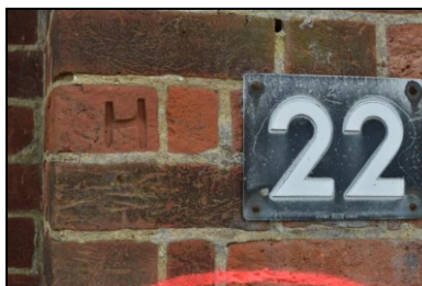
HOB16-0764 Building 22, north elevation, building identification signage
