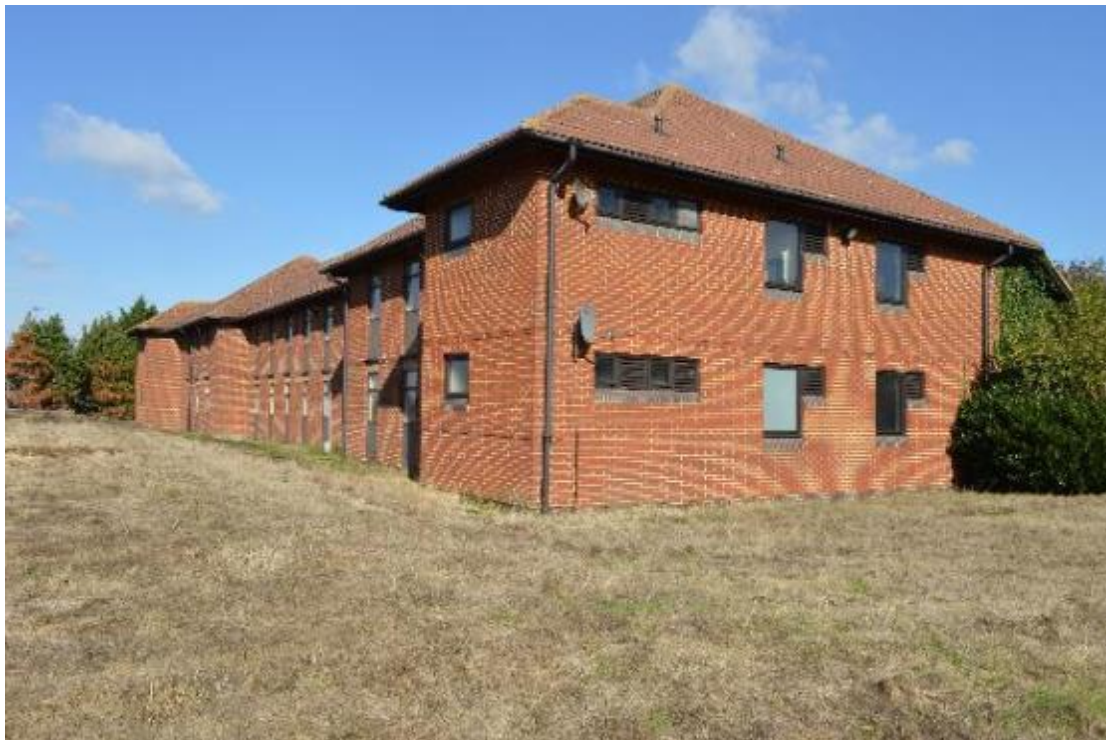
Plate 38: Building 4, south-west corner (259)
