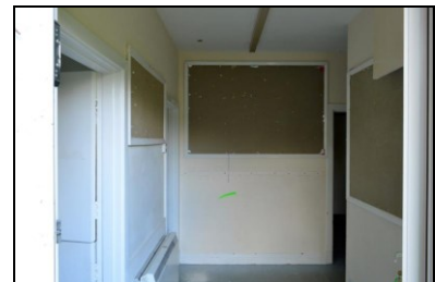
HOB16-0867 Building 90, access corridor
