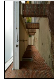
HOB16-0333 Building 8, south-east elevation
