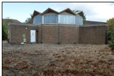
HOB16-0291 Building 5, south side
