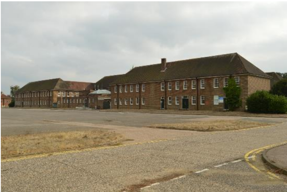
Plate 92: Building 12, rear north elevation and parade ground (469)
