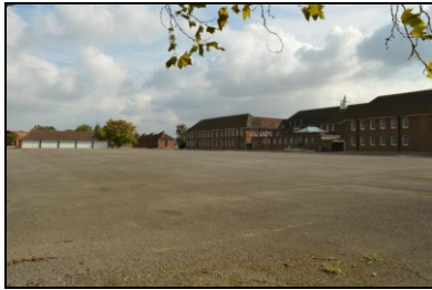
HOB16-0907 View of the Drill Yard to the north of Building 12
