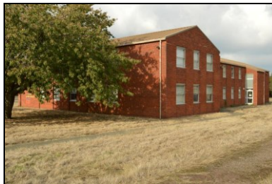
HOB16-0731 Building 21, south-west corner
