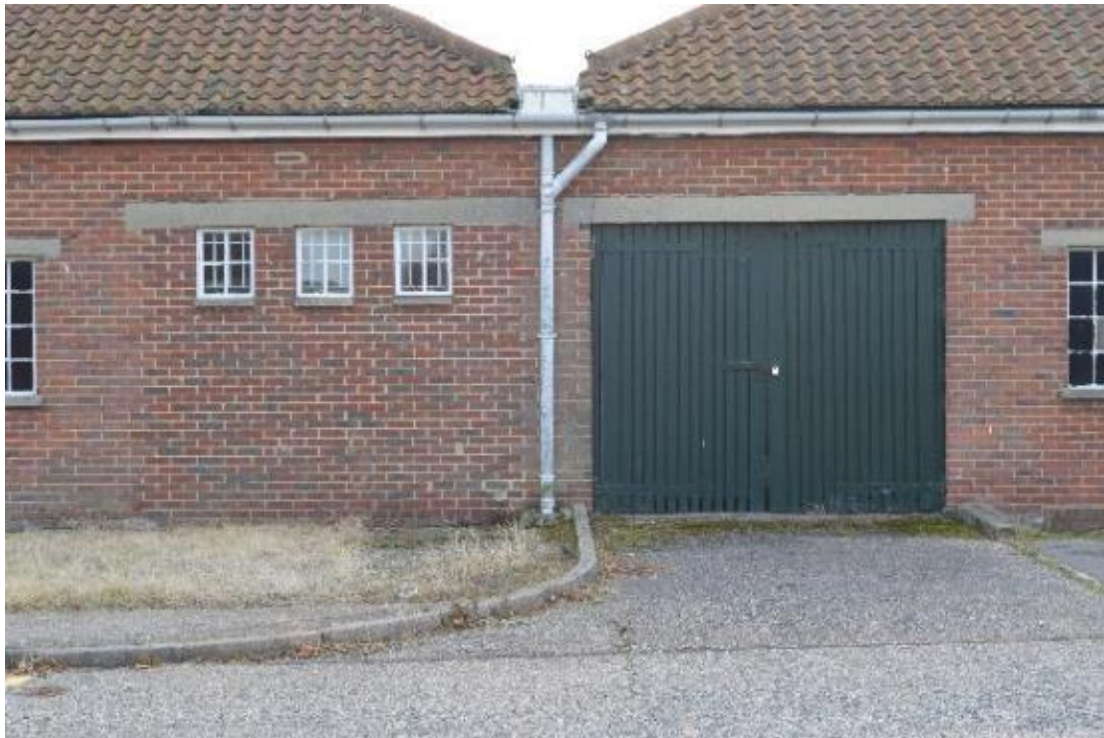
Plate 78: Building 10, north elevation, central doorway (405)
