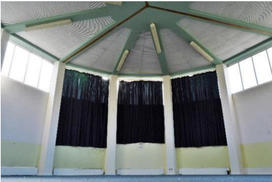
Plate 48: Building 5, band practice room (298)
