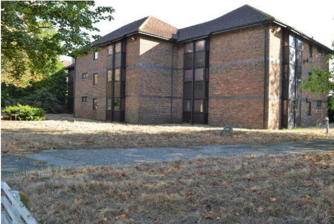
Plate 199: Building 25, north-east corner (823)
