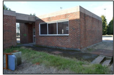
HOB16-0723 Building 20, south-east corner
