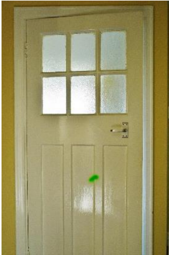
Plate 11: Building 1, original range, first floor (75)
