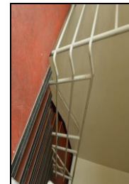
HOB16-0537 Building 12, east wing, first floor
