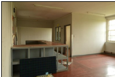
HOB16-0535 Building 12, east wing, first floor
