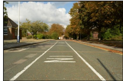
HOB16-0888 Principal site throughfare from Building 2A
