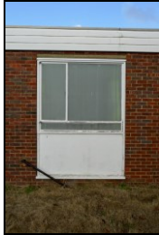
HOB16-0334 Building 8, south elevation, window arrangement
