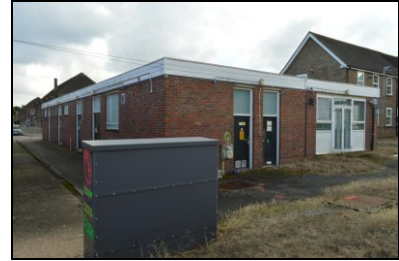
HOB16-0336 Building 8, north-west corner
