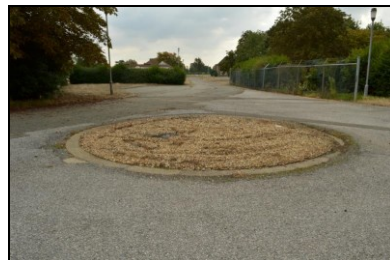
HOB16-0918 Access road adjacent Building 14
