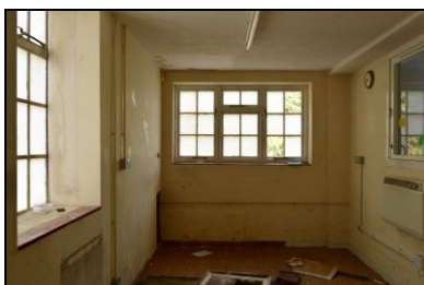
HOB16-0701 Building 18, west extension
