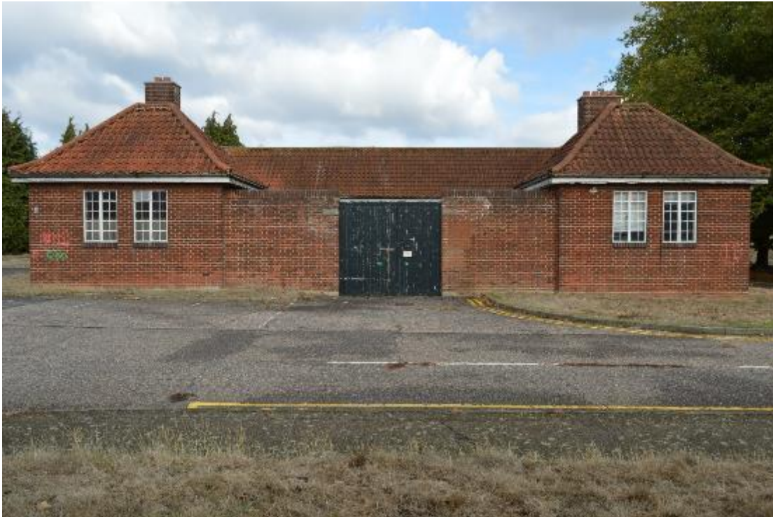
Plate 87: Building 11, south elevation (423)
