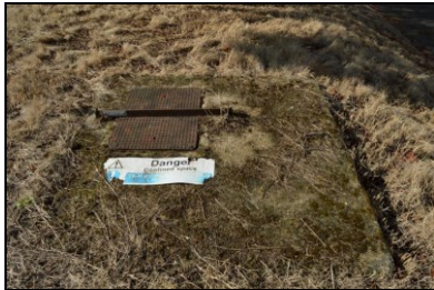
HOB16-0886 Bunker 2, entrance hatch
