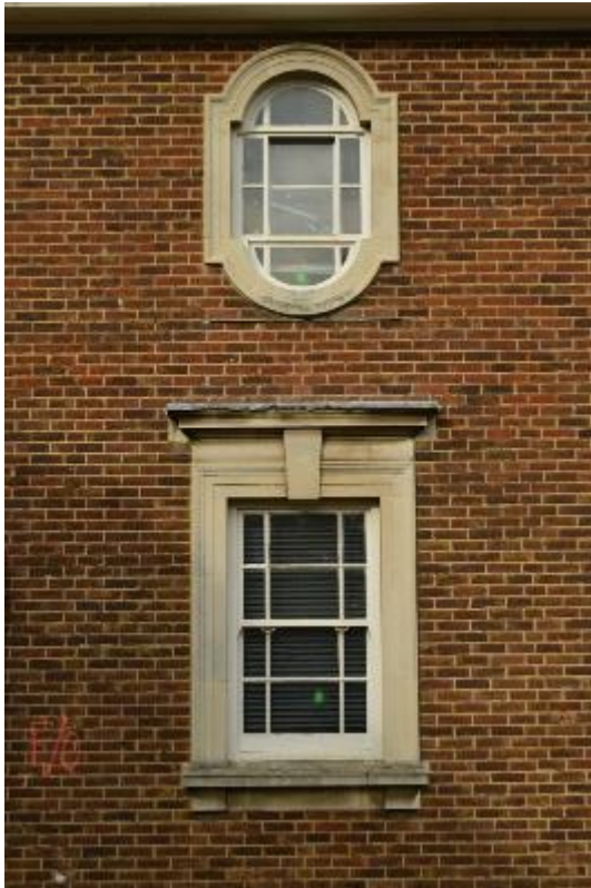
Plate 97: Building 12, south elevation, window arrangement (466)
