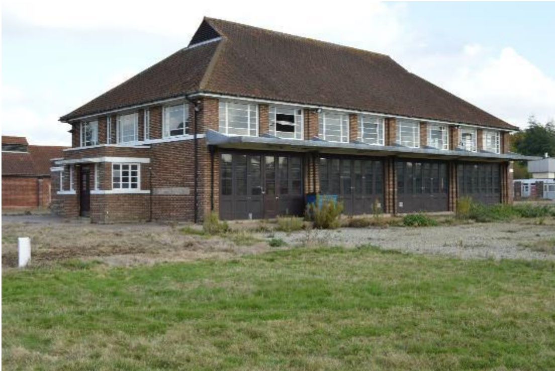
Plate 133: Building 17, south-west corner (657)
