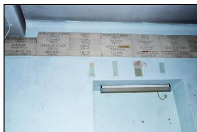
HOB16-0210 Building 2, west extension
