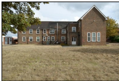
HOB16-0347 Building 9, west elevation, north extension
