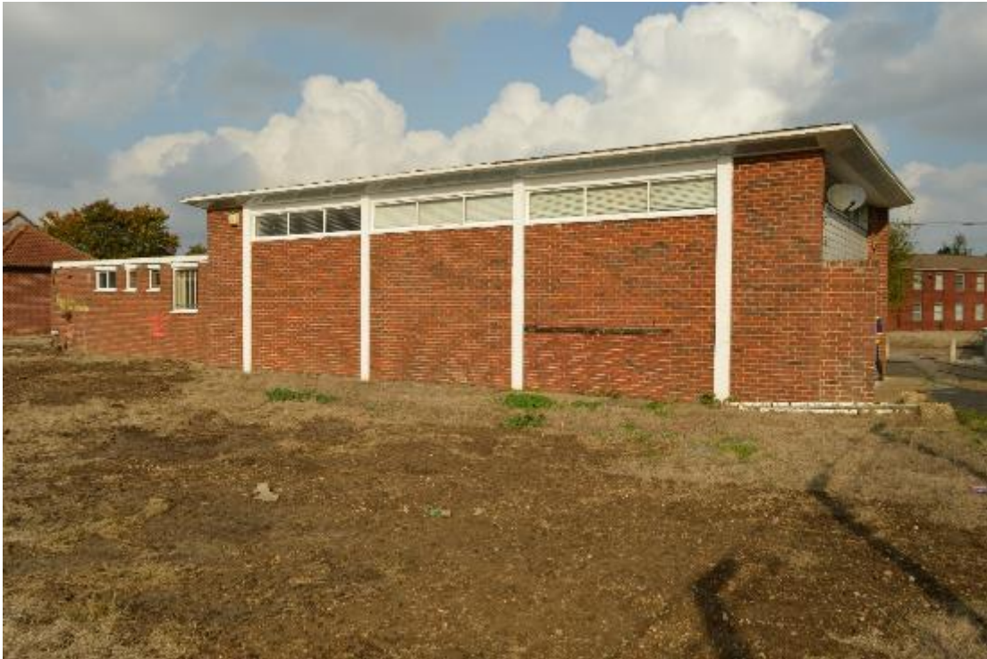
Plate 123: Building 15, south elevation (634)
