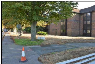
HOB16-0824 Building 25, west elevation
