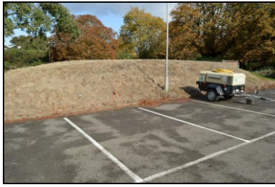
HOB16-0883 Bunker 2, south elevation
