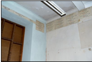
HOB16-0214 Building 2, west extension
