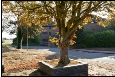
HOB16-0814 Building 25, north-west corner
