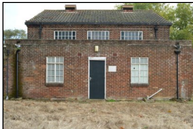
HOB16-0427 Building 18, west elevation
