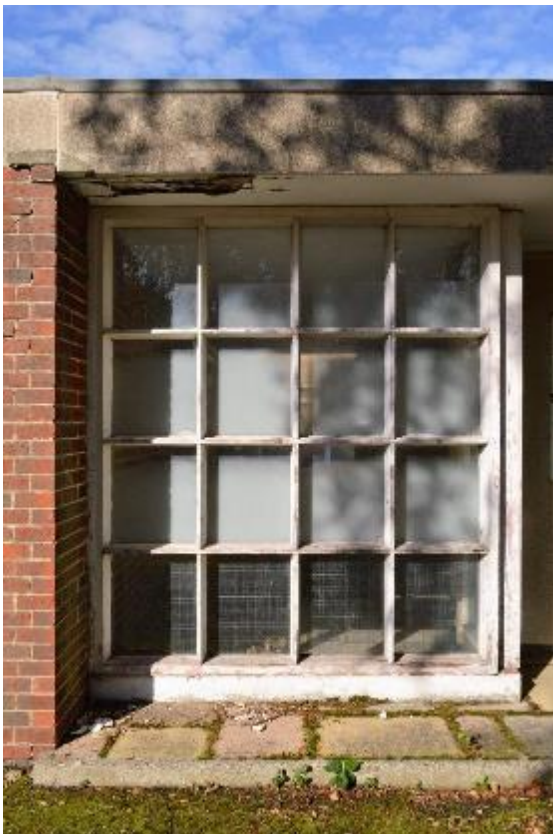
Plate 34: Building 3, south elevation, window arrangement (232)
