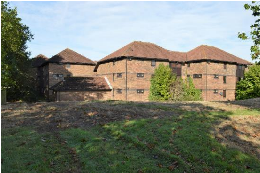
Plate 198: Building 25, east elevation (821)
