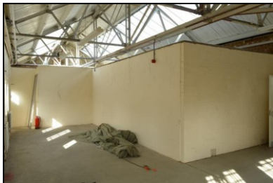
HOB16-0418 Building 10, south-west store
