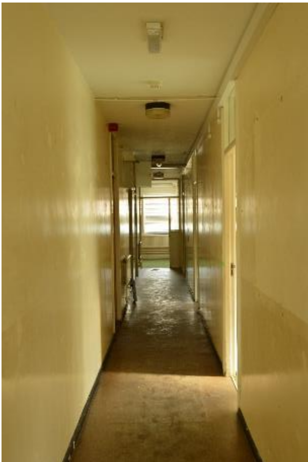
Plate 170: Building 21, north-east range, first floor, corridor (743)
