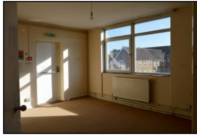
HOB16-0257 Building 3, north range, first floor, bedroom
