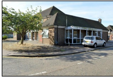
HOB16-0107 Building 2, north-east elevation
