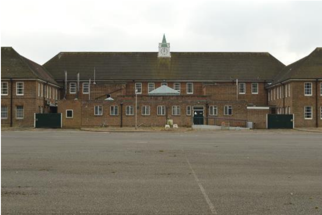
Plate 95: Building 12, north elevation, central kitchen block (470)
