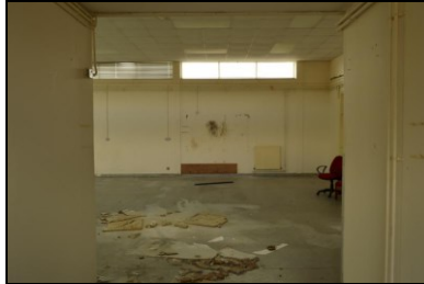
HOB16-0635 Building 15, sports hall
