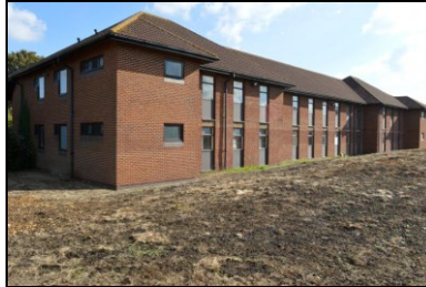
HOB16-0260 Building 4, west elevation
