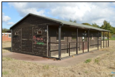
HOB16-0691 Building 17A, south-west corner
