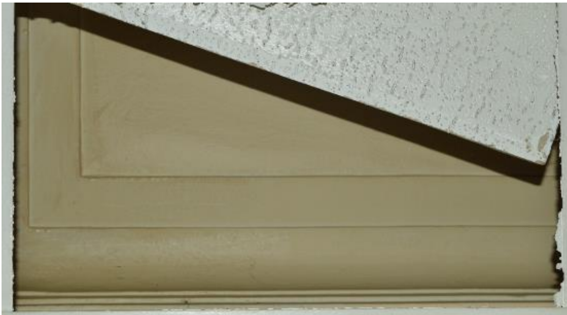
Plate 106: Building 12, central range, ground floor, dining room, ceiling cornice (501)
