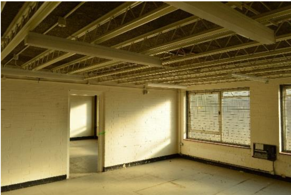
Plate 164: Building 19, north-east extension, southern room (715)
