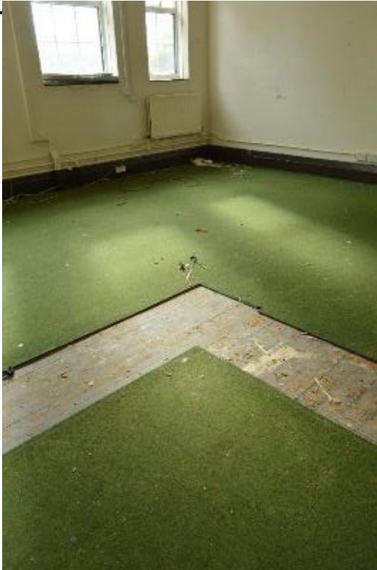
Plate 71: Building 9, original range, first floor, timber floorboards (371)
