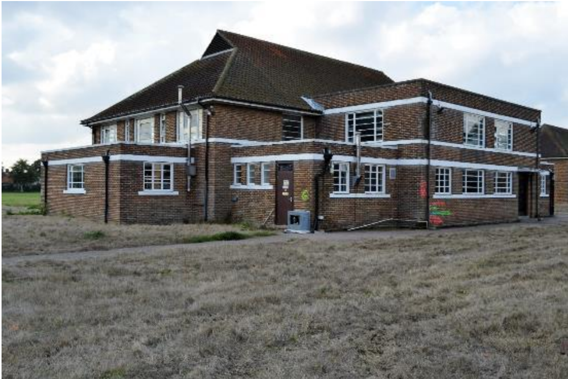
Plate 131: Building 17, north-east elevation (654)
