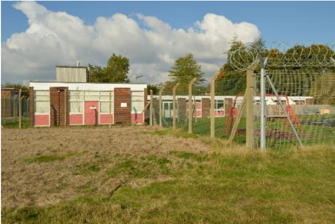
Plate 129: Building 16, south elevation (652)
