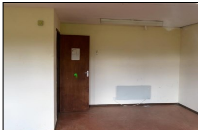
HOB16-0694 Building 17A, east changing room
