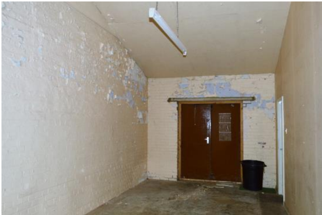
Plate 184: Building 22, east room (767)
