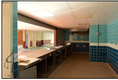
HOB16-0241 Building 3, ground floor
