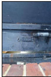
HOB16-0326 Building 7, east elevation, shutter
