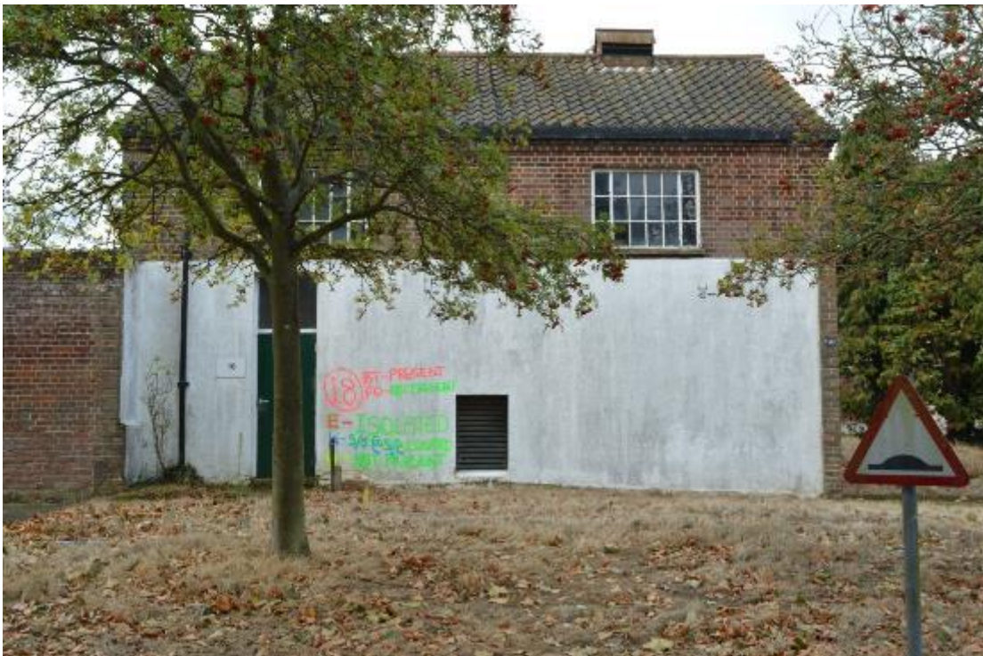
Plate 150: Building 18, east elevation (430)
