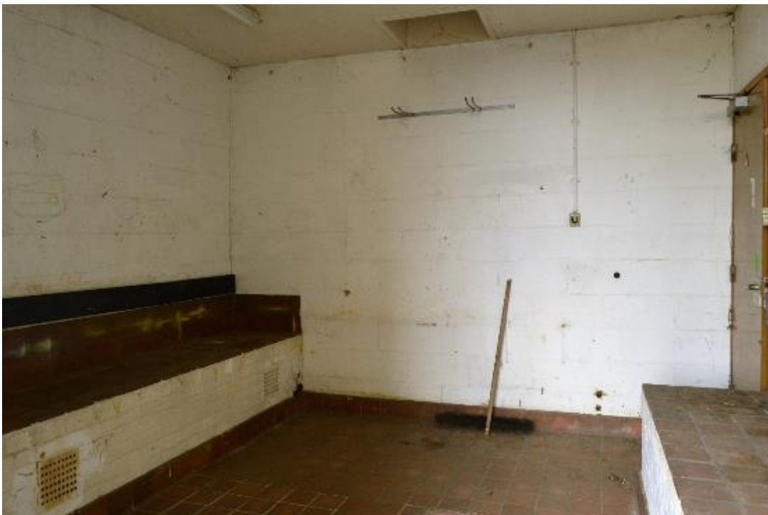
Plate 196: Building 24, central link, acid store (801)
