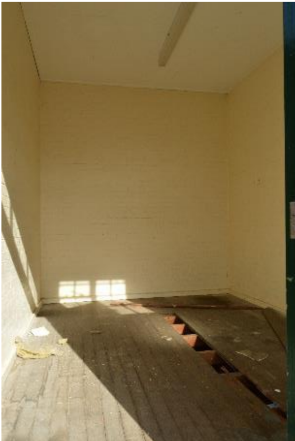
Plate 90: Building 11, Painters Shop (447)
