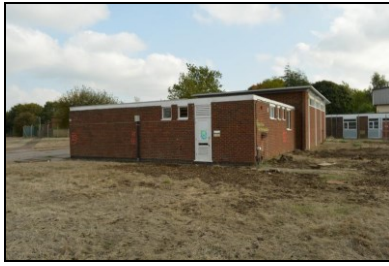
HOB16-0631 Building 15, west elevation
