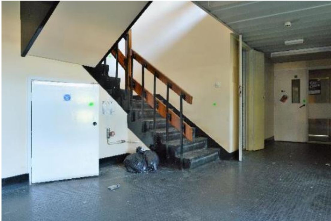
Plate 43: Building 4, block 24, central lobby, ground floor (276)
