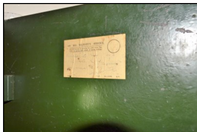
HOB16-0584 Building 14, east extension, ground floor
