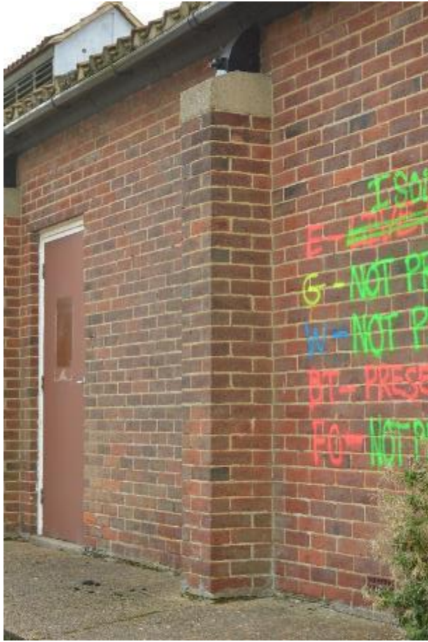
Plate 179: Building 22, north elevation, pilaster detailing (763)
