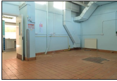
HOB16-0242 Building 3, ground floor
