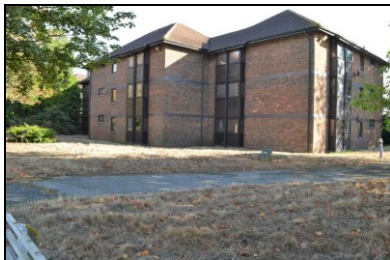
HOB16-0823 Building 25, south-west corner
