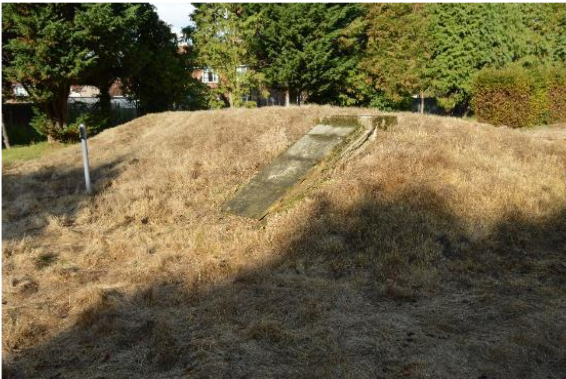
Plate 214: Bunker 1, south-east corner (879)
