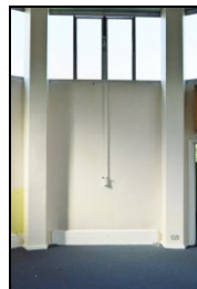
HOB16-0308 Building 5, band practice room, window panels
