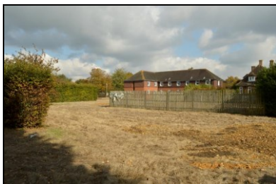
HOB16-0895 Distant view of Building 1, west elevation
