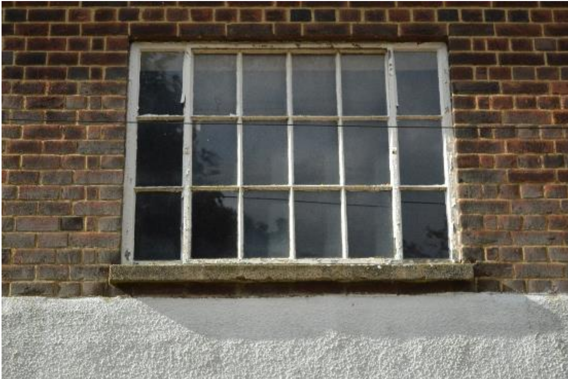
Plate 151: Building 18, east elevation, window arrangement (706)
