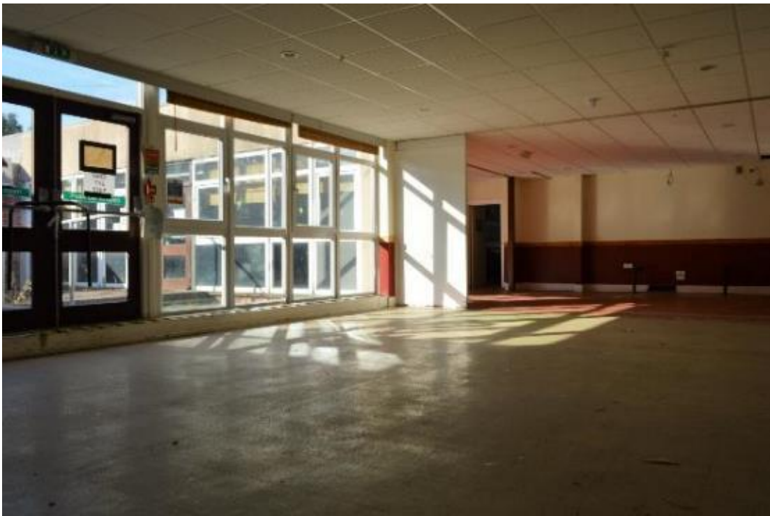
Plate 36: Building 3, ground floor, social area (249)
