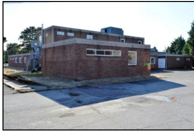
HOB16-0721 Building 20, north-east corner
