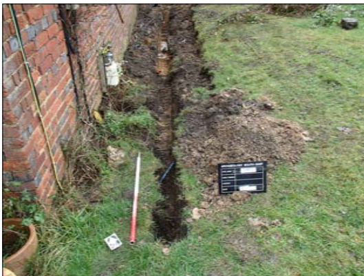
Service trench, north-east facing
