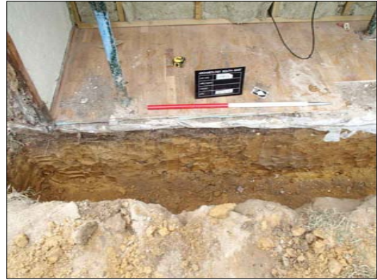
North-east facing section of Timber support (N end)
