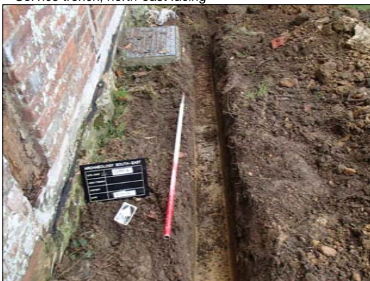
Service Trench, north-east facing
