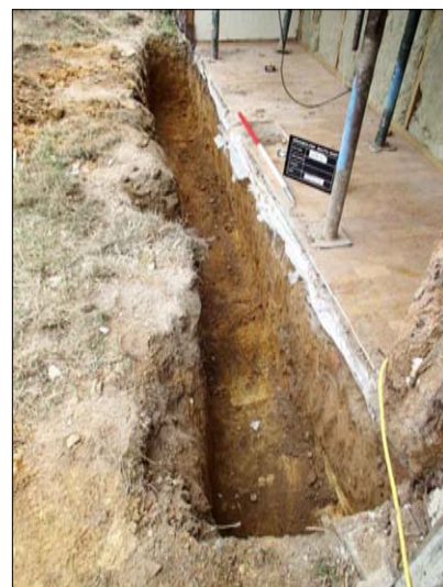
Timber support trench, looking south
