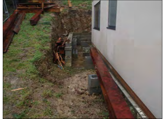
General location of Balcony post 4 facing north
