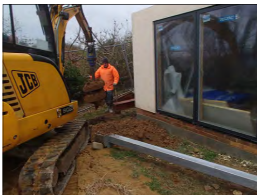
Undertaking pile auguring
