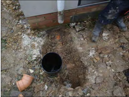
Drainage trench in the north-east
