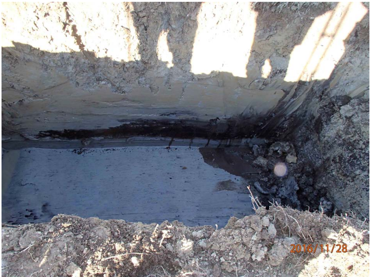
South side of sewer excavation, south-east facing section
