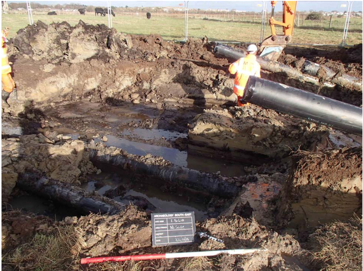
North side of sewer excavation, looking north-east
